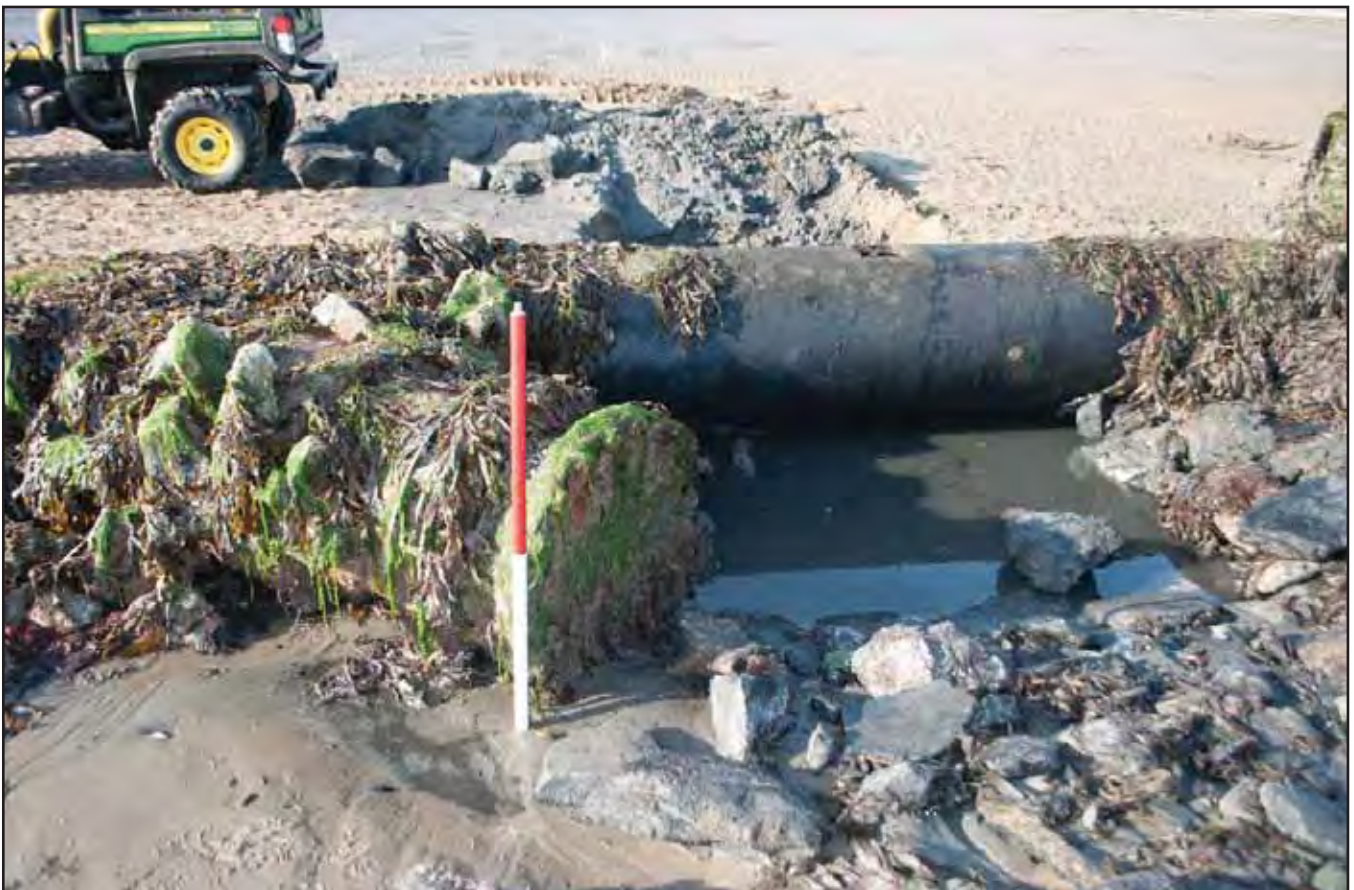
Plate 14: Stones encrusted to outfall pipe; scale: 1x1m (archive reference: G2619_019).
