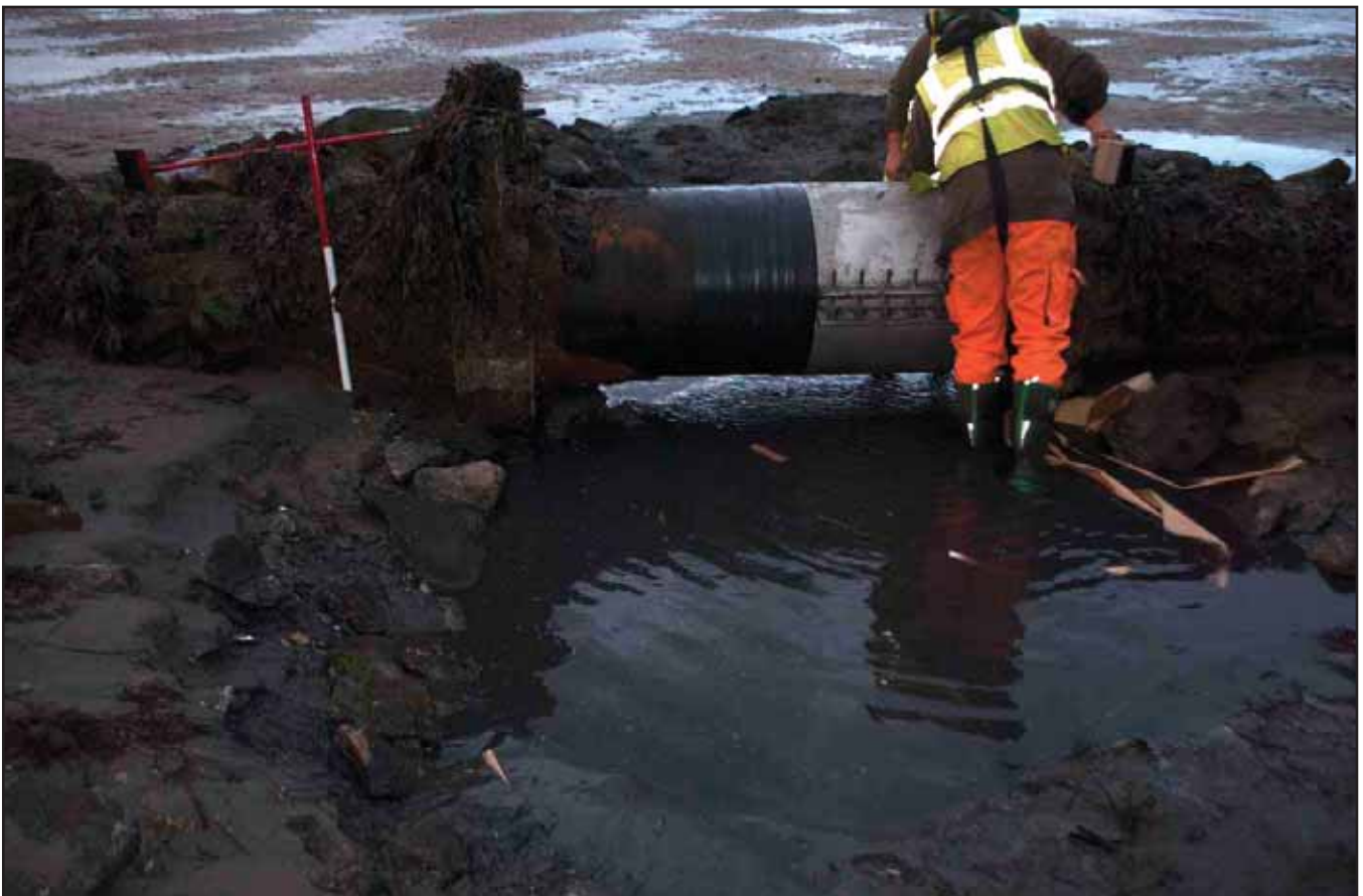
Plate 20: Excavation 11 showing repair; scale: 1x1m (archive reference: G2619_061).
