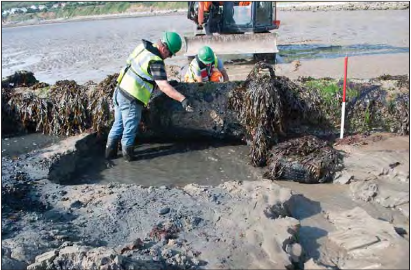
Plate 01: Cleaning a section of outfall; scale: 1x1m (archive reference: G2619_010).
