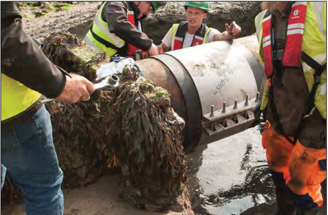
Plate 04: Fitting the repair section; no scale (archive reference: G2619_045).
