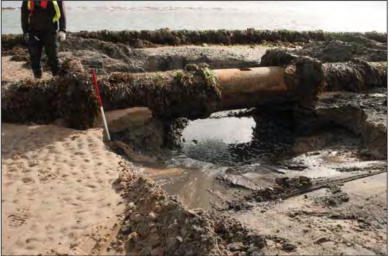
Plate 11: Excavation 6; scale: 1x1m (archive reference: G2619_041).
