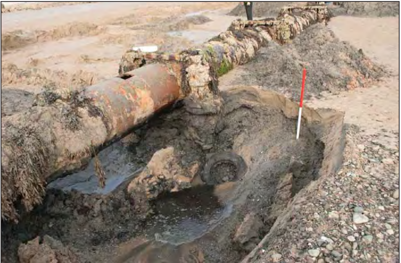
Plate 12: Excavation 7; scale: 1x1m (archive reference: G2619_043).
