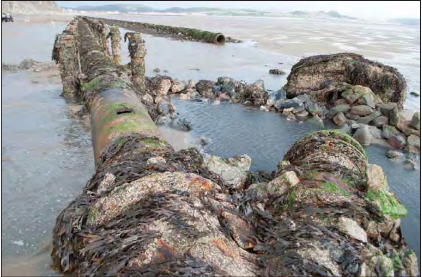
Plate 15: Stones collecting around obsolete pipe connexion; no scale (archive reference: G2619_052).
