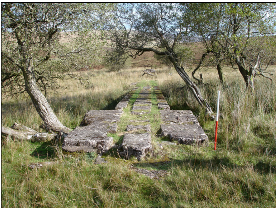
Plate 33: A concrete machine base or ramp (NPRN 267148), to the south of the dam.
