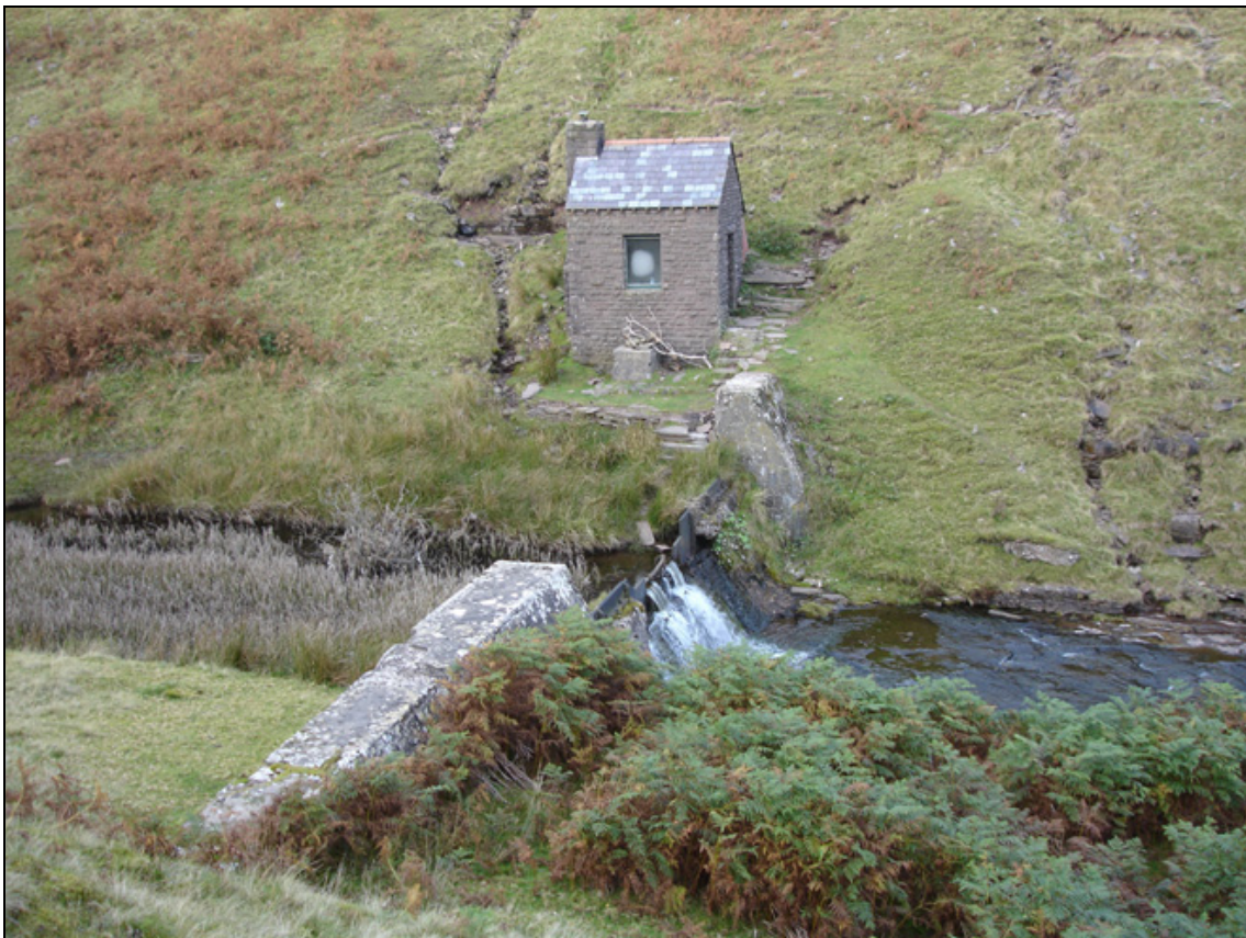
Plate 29: The Water Meter House and weir of the original, temporary Grwyne Fawr reservoir (NPRNs 267356 & 267357).
