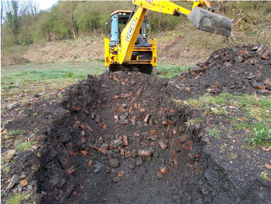
Photo 1: Trench 1. West facing shot of trench during excavation, showing large quantity of brick rubble 1003.
