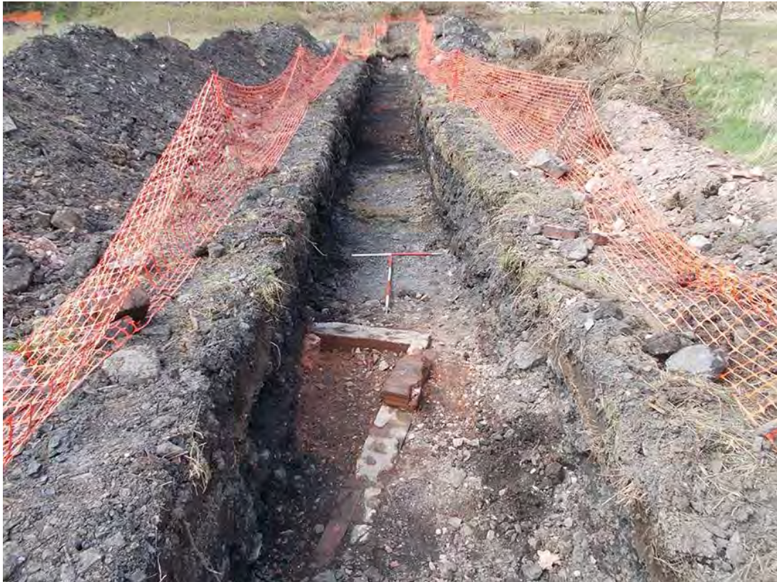
Photo 5: Trench 2. WNW facing shot along the Trench. 1m & 2m scales.
