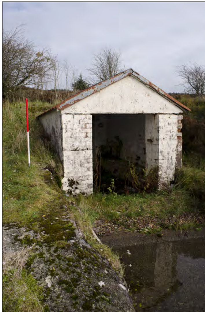
Plate 10: View of boathouse (Feature 2); scale: 1x1m (archive reference: G2580_014).
