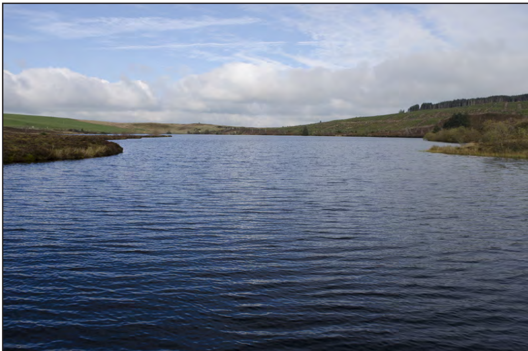
Plate 6: General view of the reservoir looking northwards from the dam wall; scale: not used (archive reference: G2580_006).
