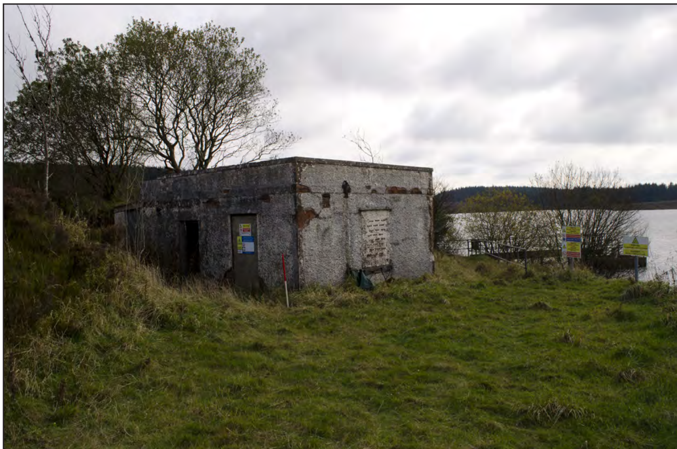
Plate 13: View of brick and concrete building to the north of the DCWW jetty (Feature 3); scale: 1x1m (archive reference: G2580_017).
