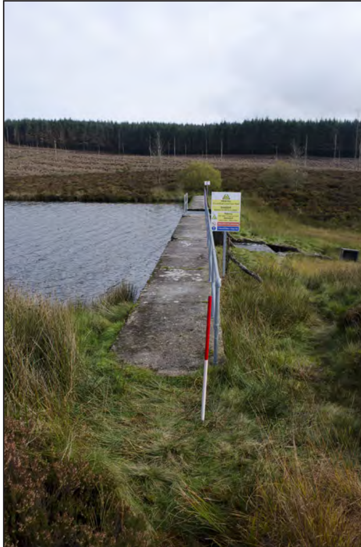
Plate 5: View along the dam parapet; scale: 1x1 m (archive reference: G2580_005).
