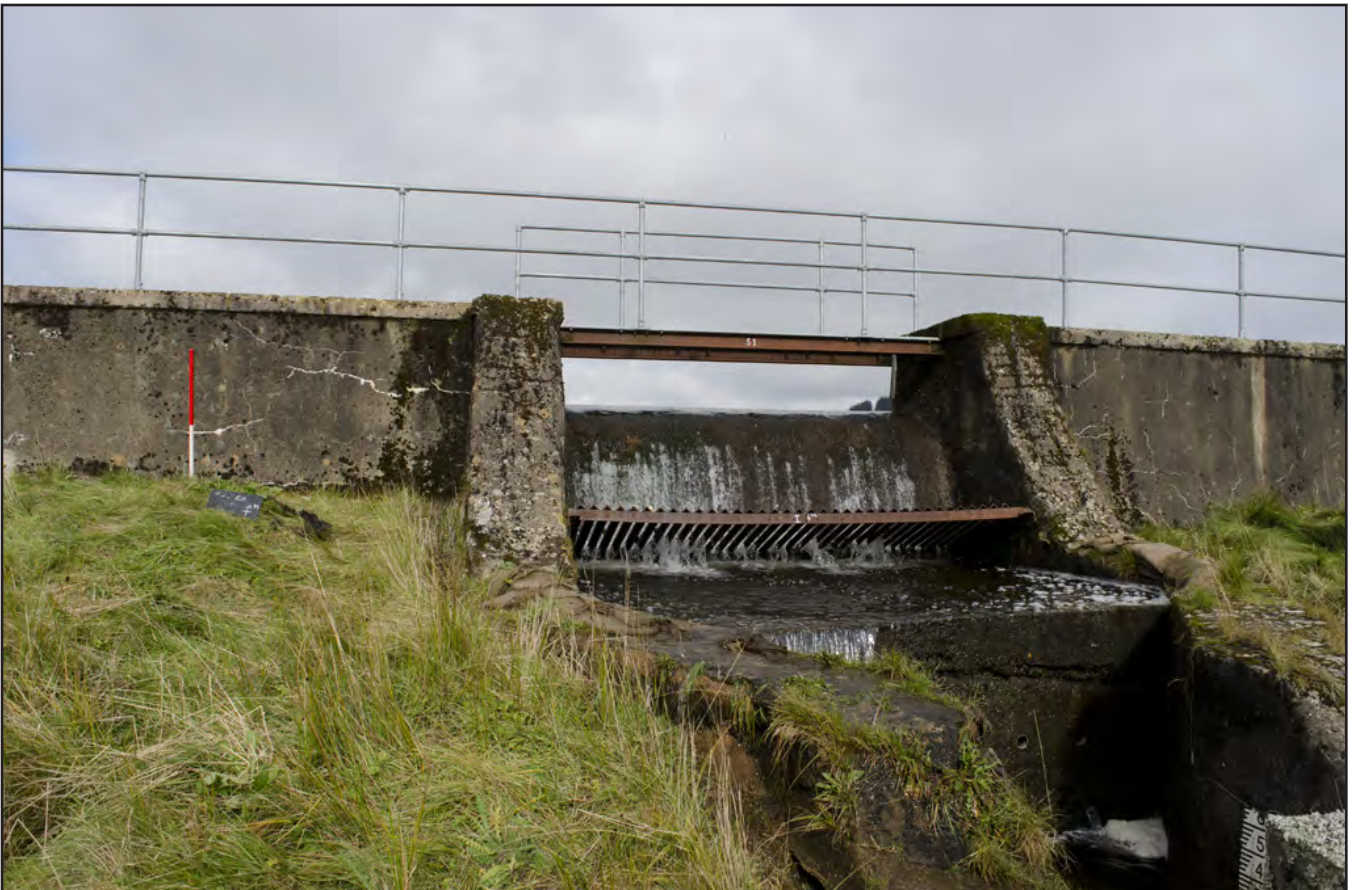
Plate 2: View of weir in the dam wall; scale: 1x1m (archive reference: G2580_002).
