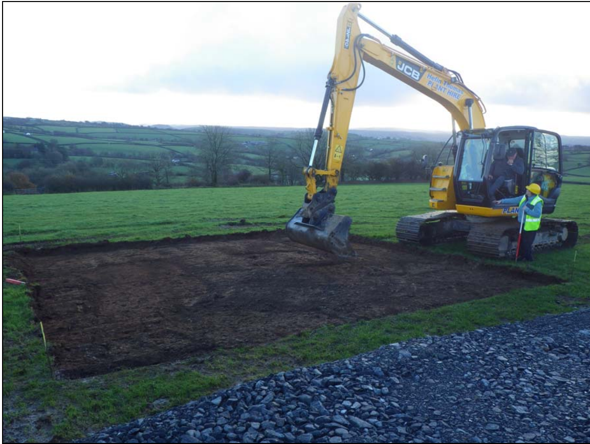
Plate 1: CCF2014_101, After the topsoil removed from the trench, looking southeast.
