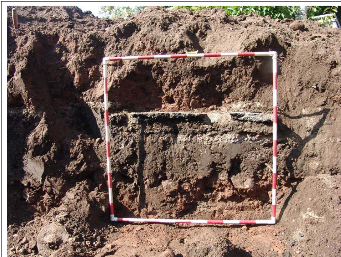
Plate 11: View of two tarmac road surfaces within western bank. Scale 1sqm Looking west
