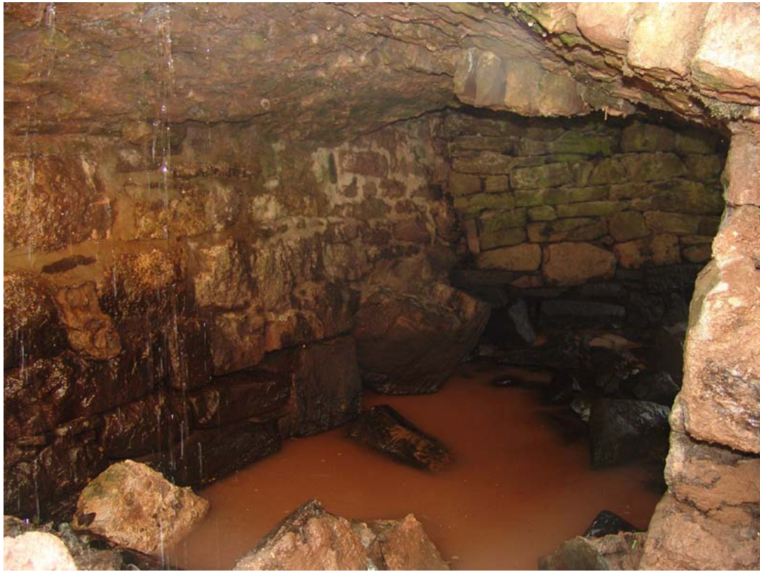
Plate 5: View of unbonded bridge stonework with later cement pointing. Looking south east
