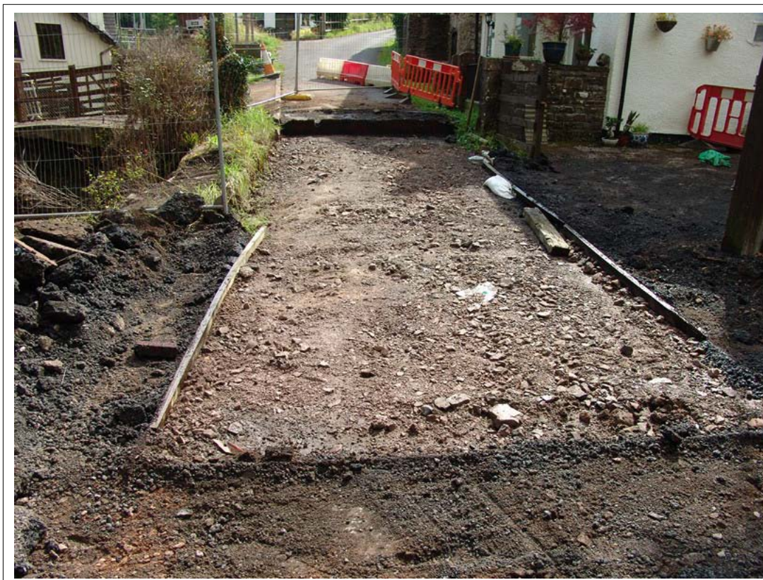
Plate 2: View of hardcore deposit (001) beneath steel road plate. Looking east
