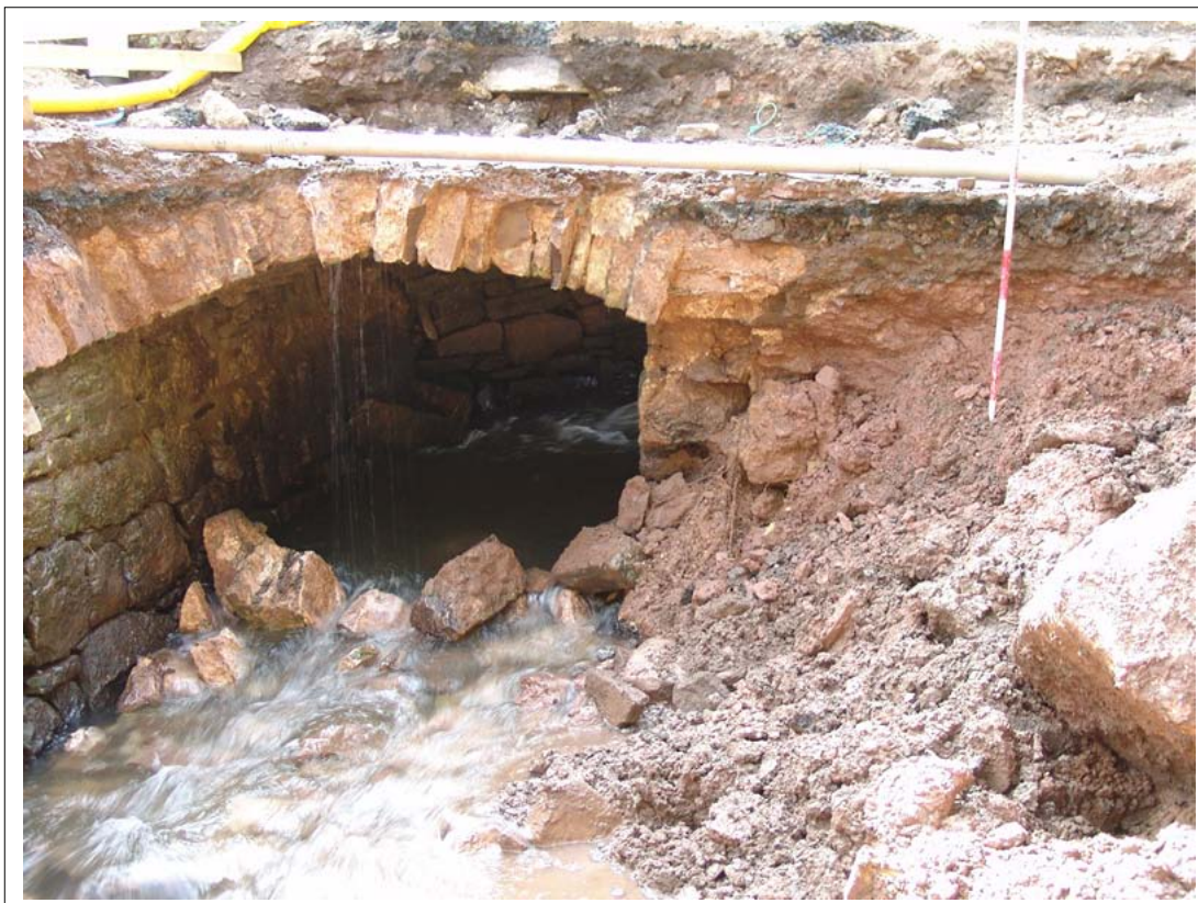
Plate 3: View of bridge arch stones with hardcore (001) above. Scale 1x2m. Looking south
