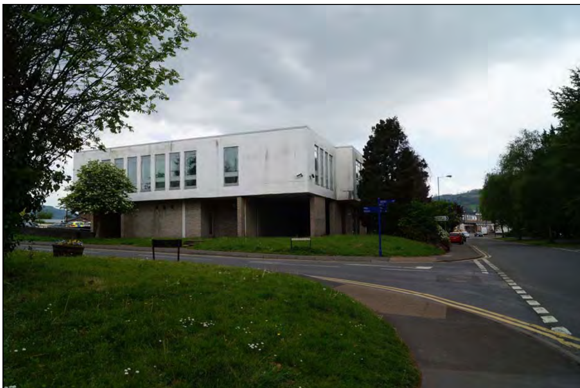
Plate 1: A view towards the Magistrates Court (ID number 1001), looking east-northeast along Tudor Street at the Baker Street junction. Baker Street runs to the left.
