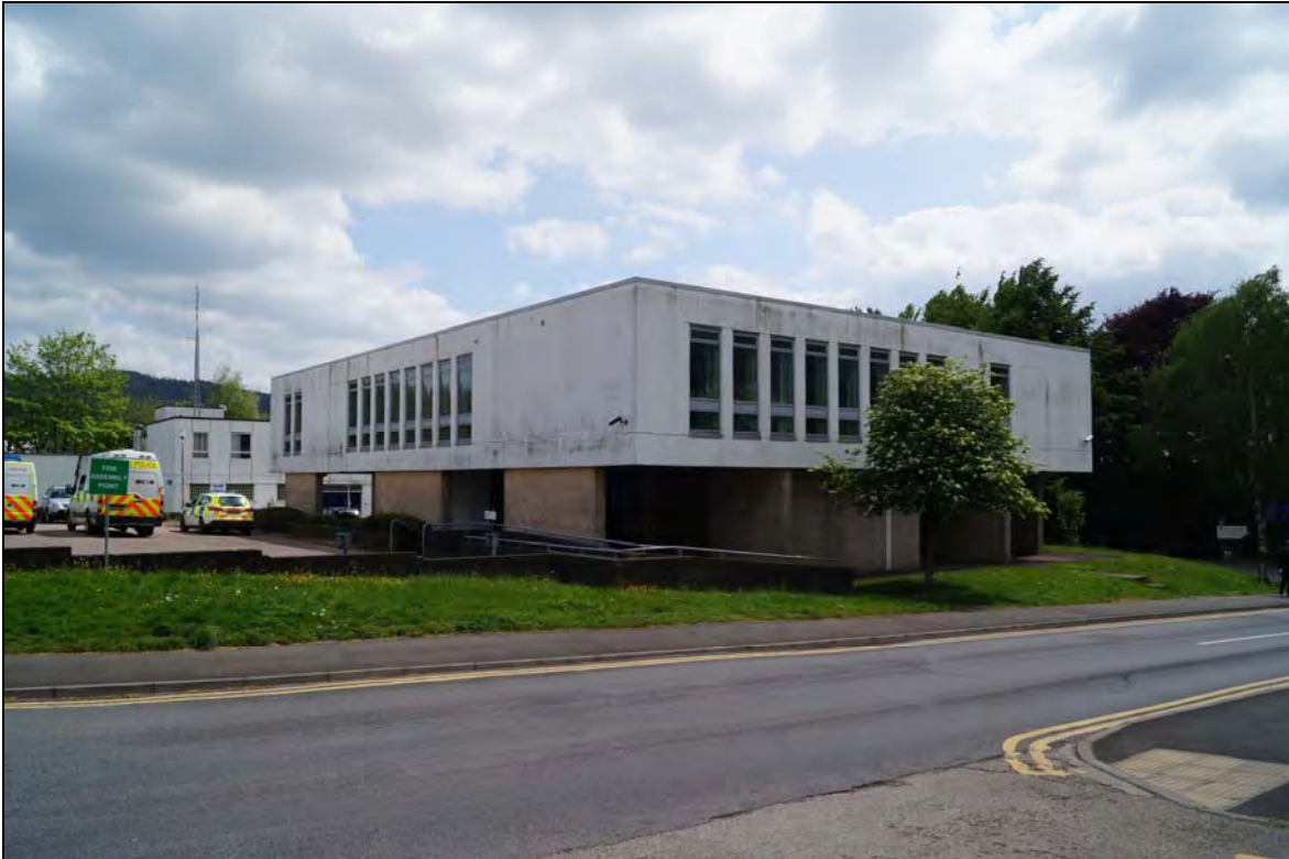
Plate 15: A view of the Magistrates Court (ID number 1001), from Baker Street, looking southeast.
