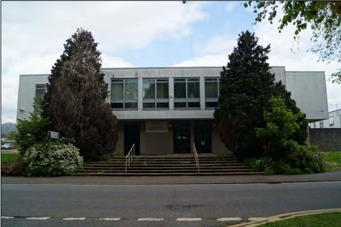
Plate 7: A view of the front of the Magistrates Court (ID number 1001), looking north. Note that the building is raised above road level.
