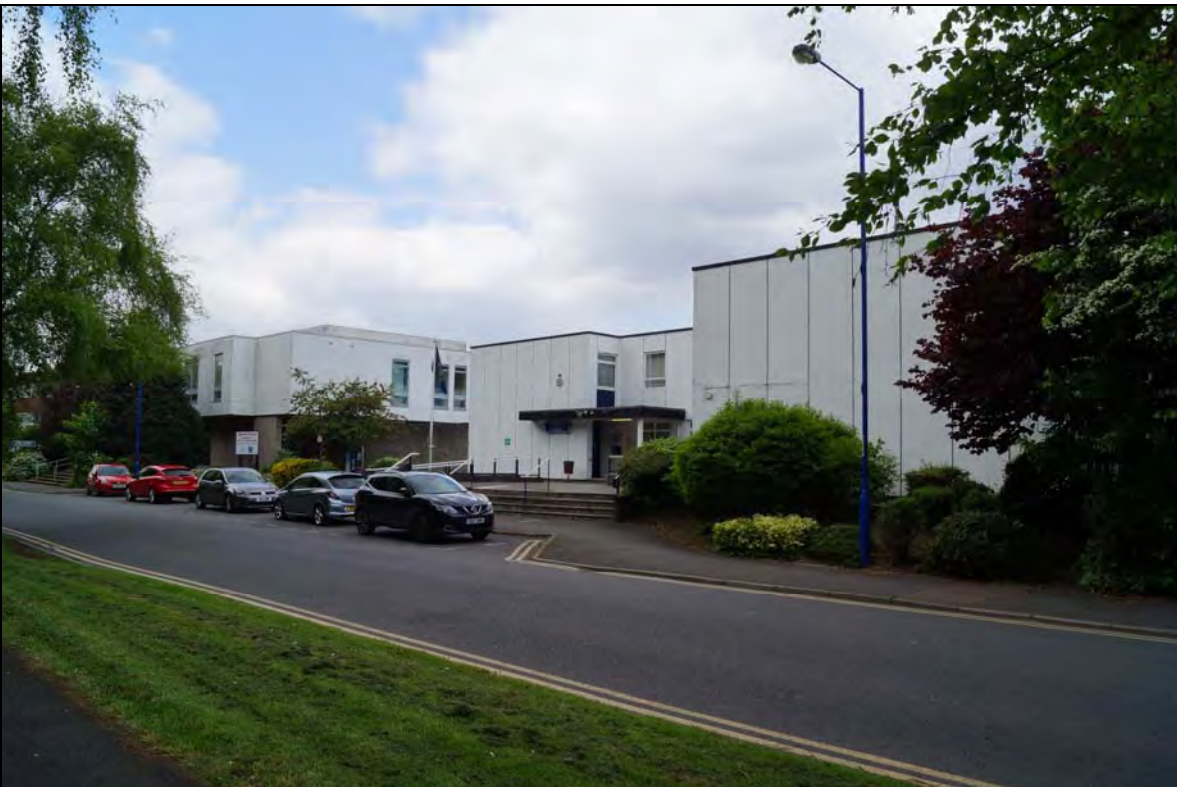
Plate 12: A view northwestwards of the Police Station and Magistrates Court from the southern side of Tudor Street.
