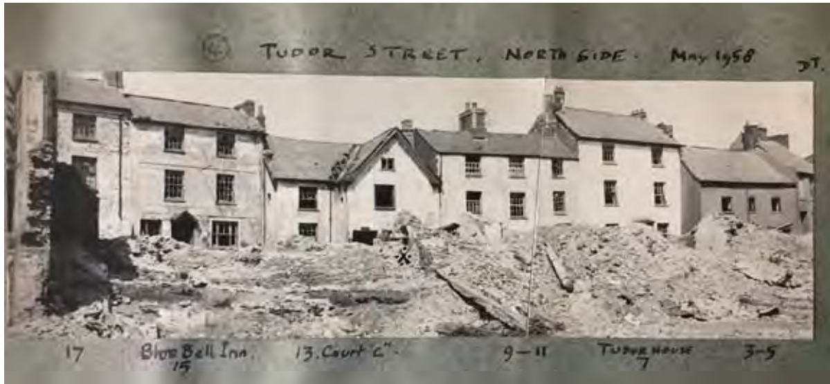
Figure 8; A view across the partially demolished Tudor Street in 1958. The buildings to the left, numbers 15 (The Bell Inn) and 17 (ID numbers 1003 & 1004) would roughly correspond with the eastern side of the modern police station (D.M. Thacker Collection, NMR Archive).
