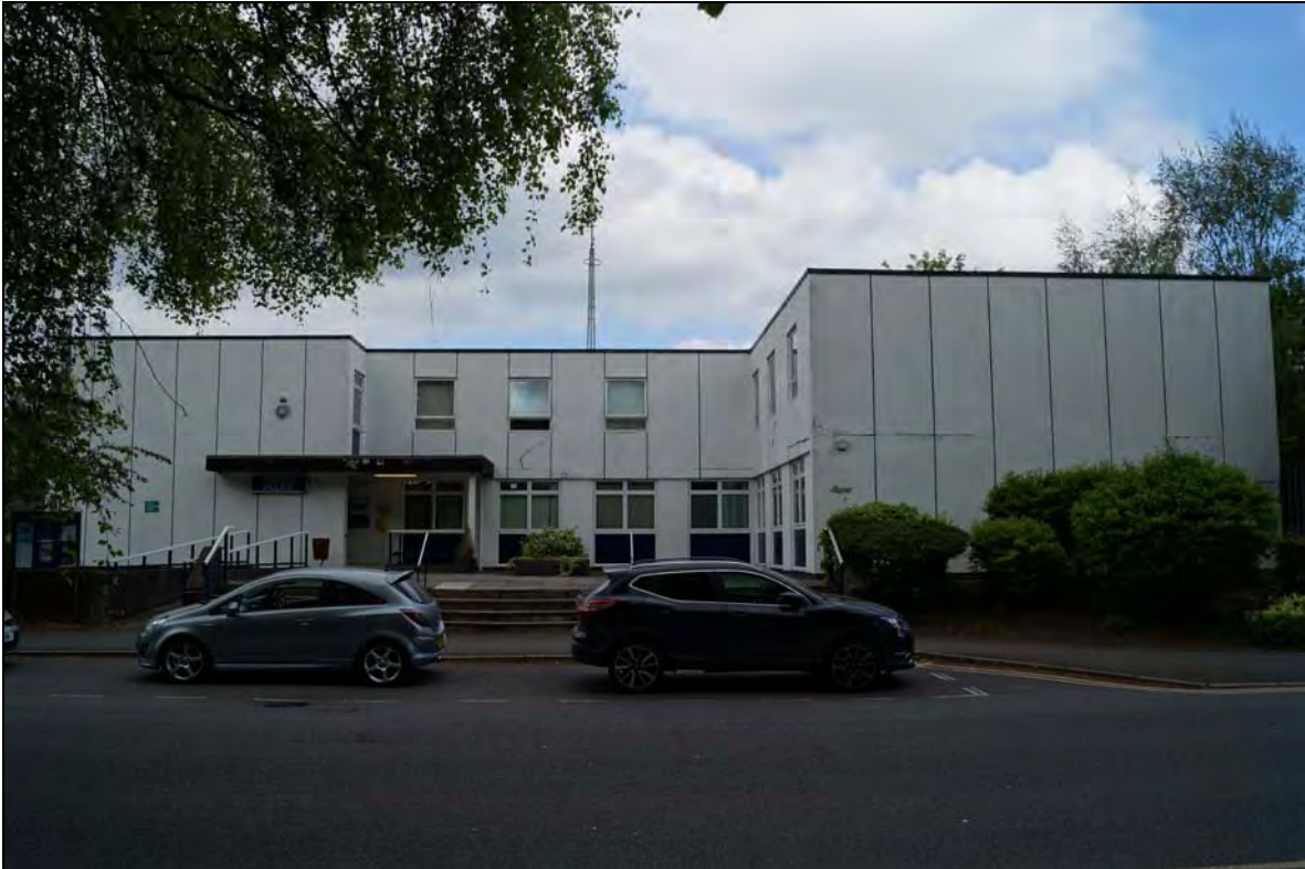
Plate 13: A view of the Police Station (ID number 1002), looking north from the southern side of Tudor Street.
