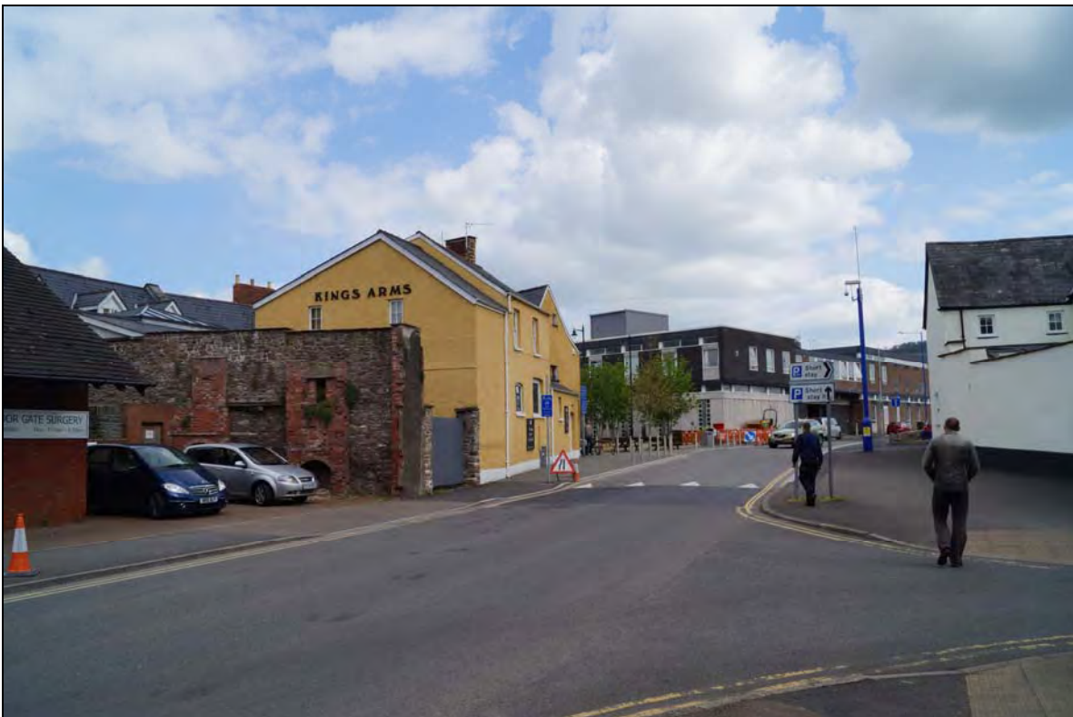
Plate 10: A section of the post-medieval town wall (ID number 1), seen here centre left, looking northeast from the eastern end of Tudor Street. The Tudor Gate would have stood here. The listed Kings Arms inn (ID number 75) stands behind the wall and the modern Post Office beyond that.
