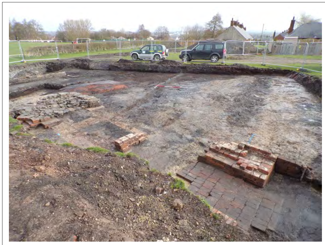
Plate 12. General view across excavated area. Looking north-east. Scales 1m & 2m
