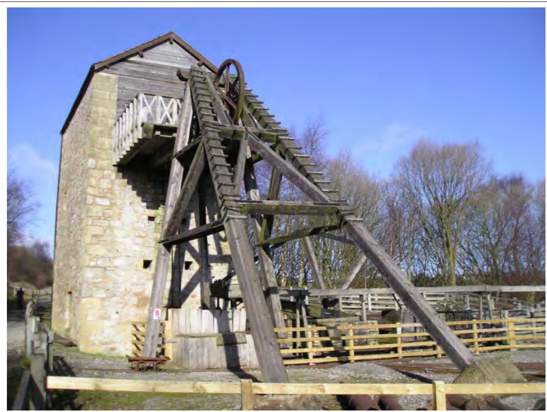
Plate 2. Example of Engine House at Minera, Wrexham
