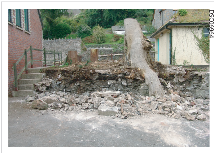
Plate 01: Retaining wall dismantles to remove tree. [101], [102], [104], [105], [129].
