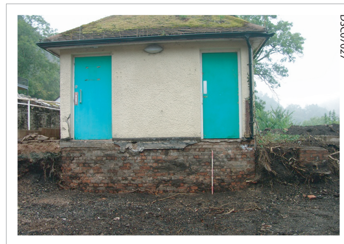
Plate 08: South side of toilet block on 1.2m high brick foundation. [101], [103], [104], [105], [114].
