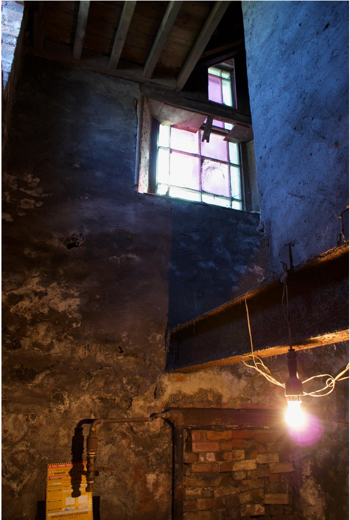
046CCPS Basement under east stairs
