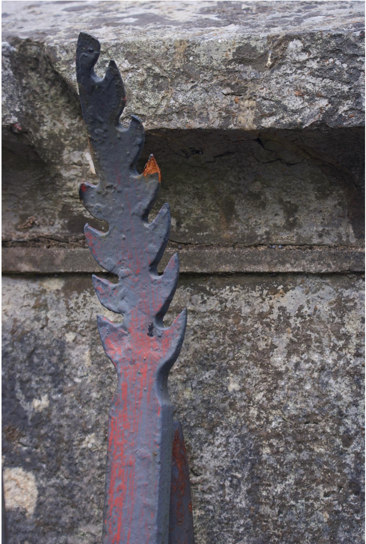
050CCPS Gate detail
