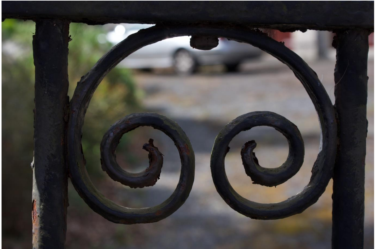
051CCPS Gate detail
