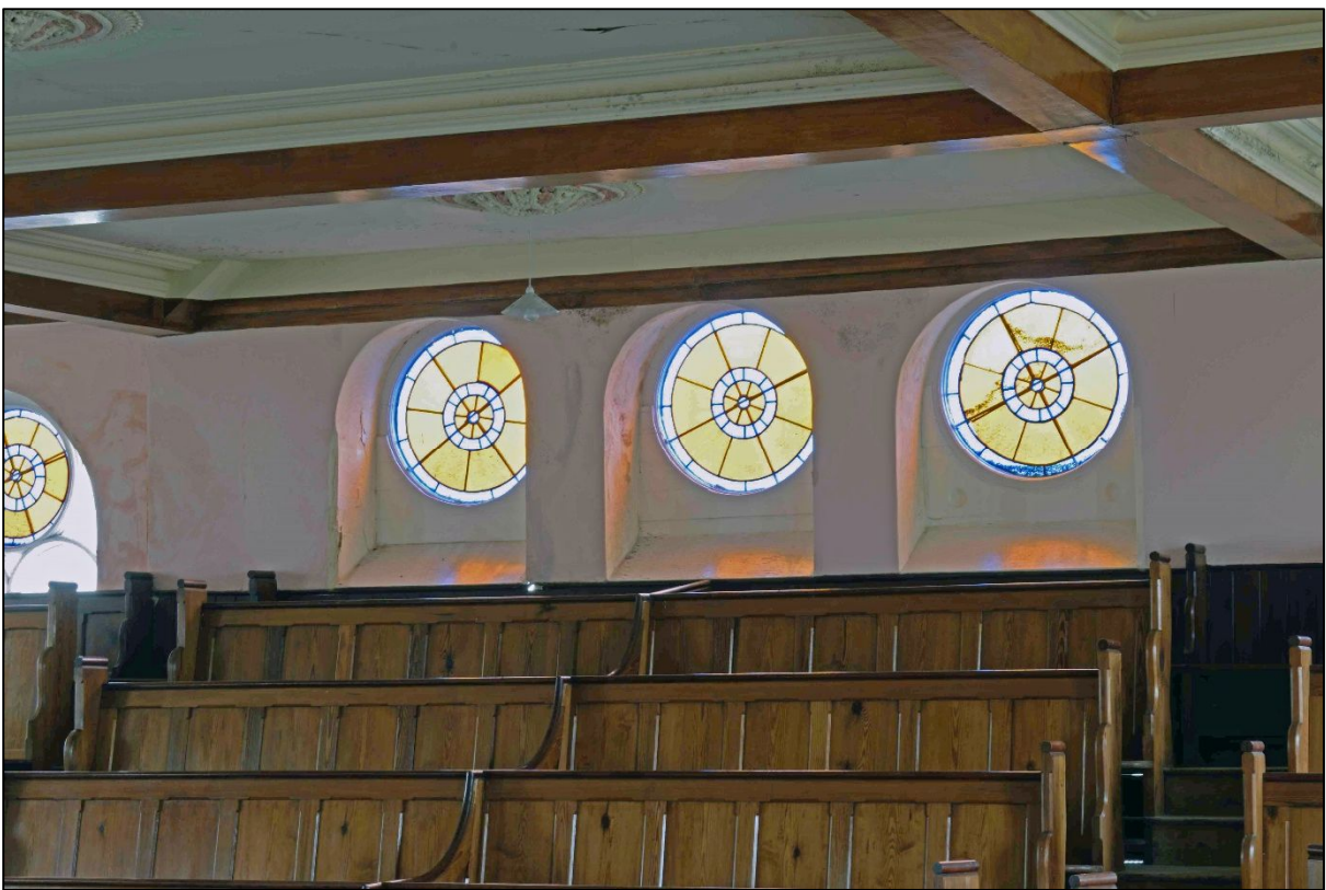
Plate 34: Stained glass windows in south western gable.
