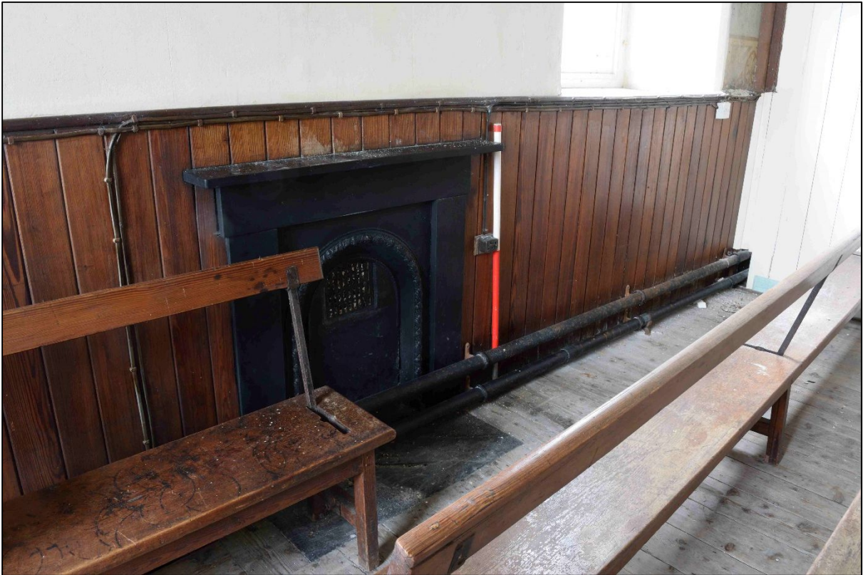
Plate 49: Fireplace in the Sunday School room
