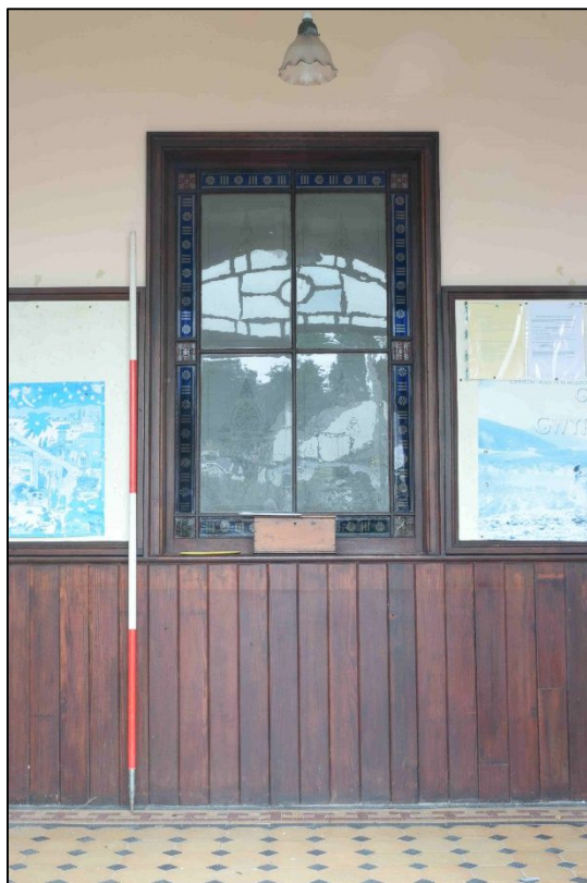
Plate 16: Window between the lobby and the nave
