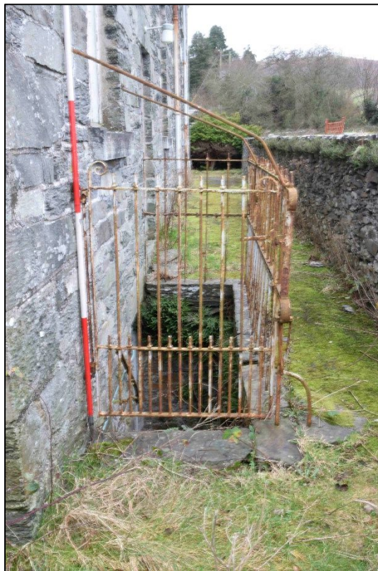
Plate 12: Enclosure around the access to the cellar
