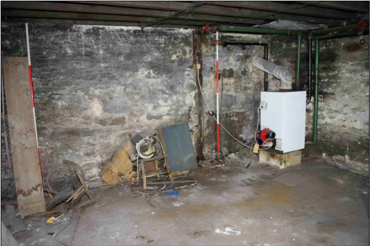
Plate 61: Cellar, looking east
