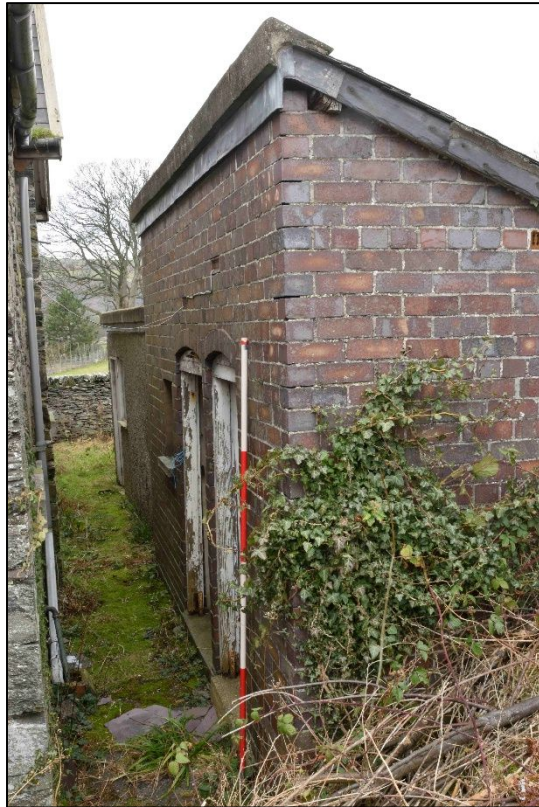
Plate 15: Toilet blocks looking north west
