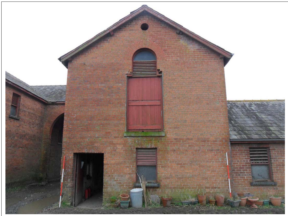
Plate 12:View of gable end adjacent to archway courtyard entrance Scales 2x2m, Looking south east
