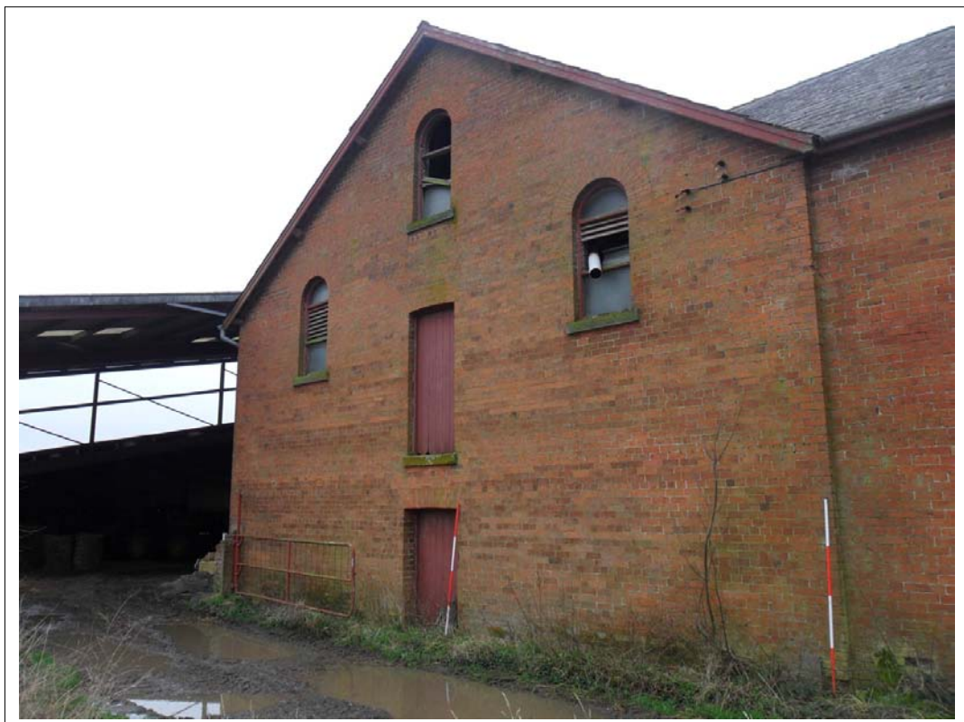
Plate 46: Oblique view of main building gable end Scales 2x2m, Looking west
