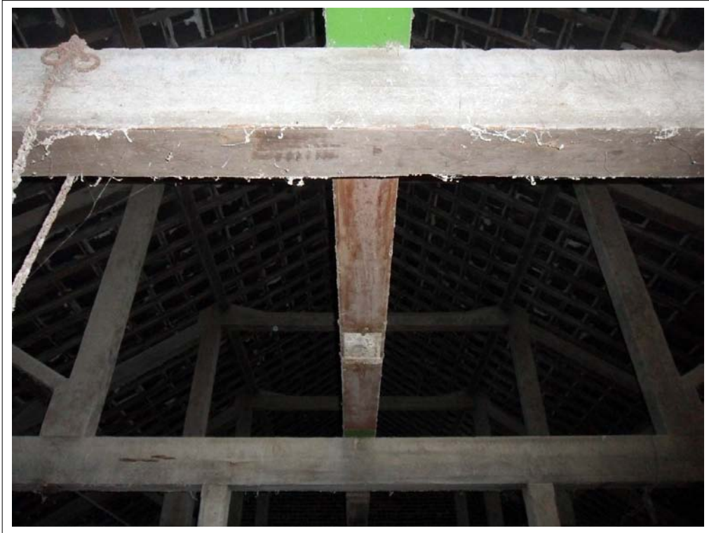
Plate 179: View of roof construction within provender storage area above cart store
