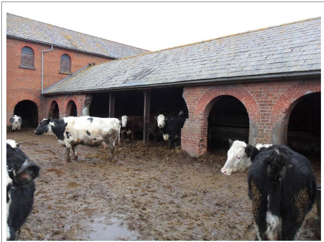
Plate 24: Note two brick archway pillars removed from this animal range also Repair made in same steel bars. Looking east
