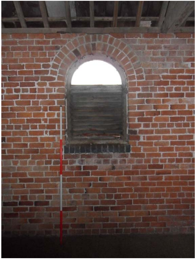
Plate 145: Example of an arched, slatted, window in upper level, Scale 1x2m
