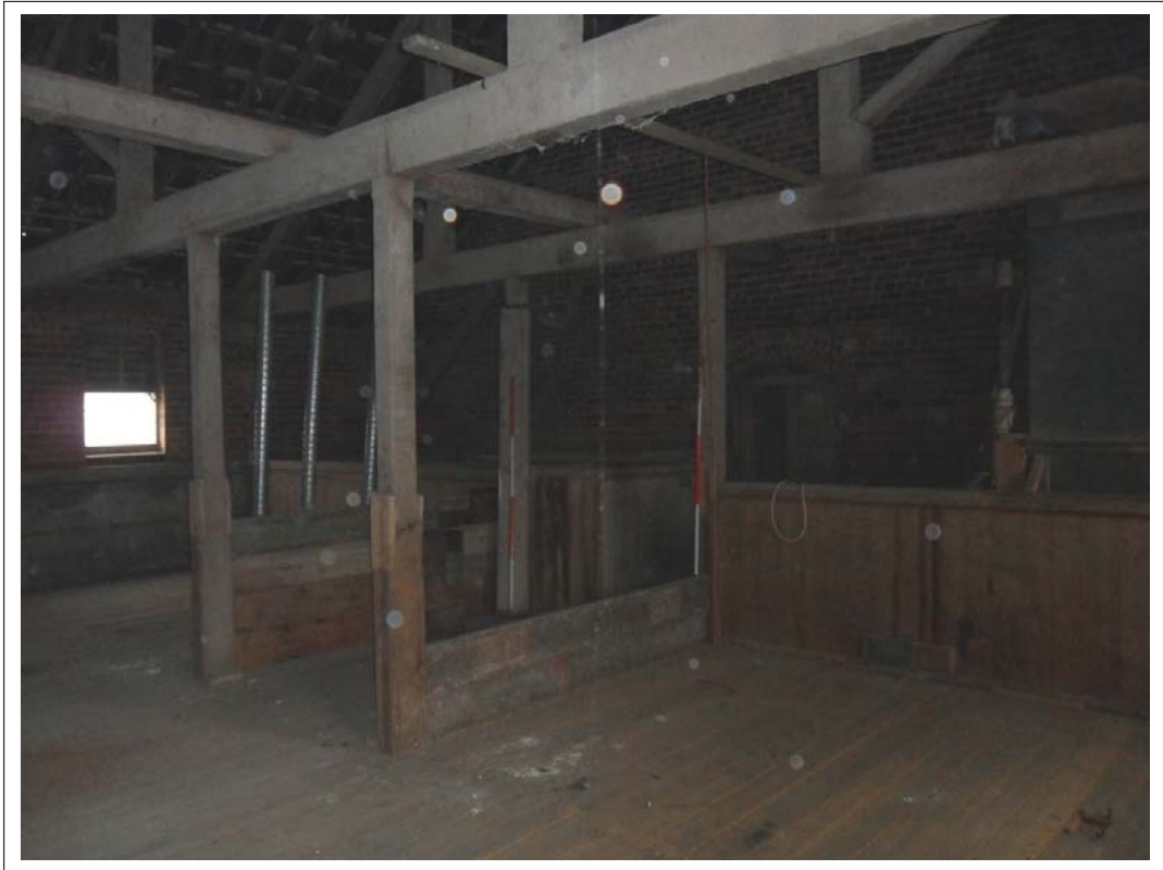
Plate 171: View of storage area above cart store Scales 2x2m
