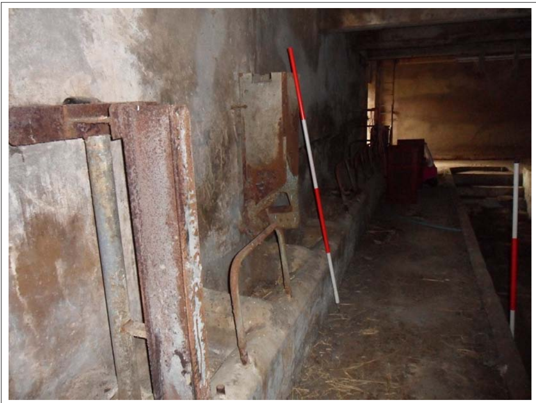
Plate 164: Feed stalls installed at base of each wall. Scales 2x2m
