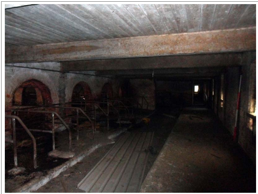
Plate 126: View of feeding stalls within corridor facing into courtyard area, note recessed floor for effluent removal. Scale 1x2m
