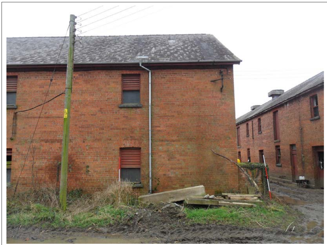
Plate 44: View of rear wall of cart store, now a workshop (lower floor). Scales 2x2m, Looking south west
