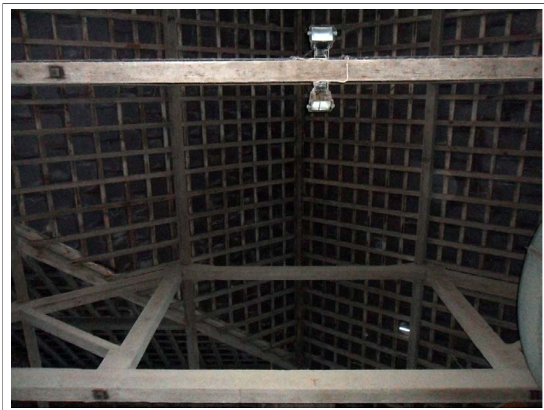
Plate 88: View of roof and rafter construction
