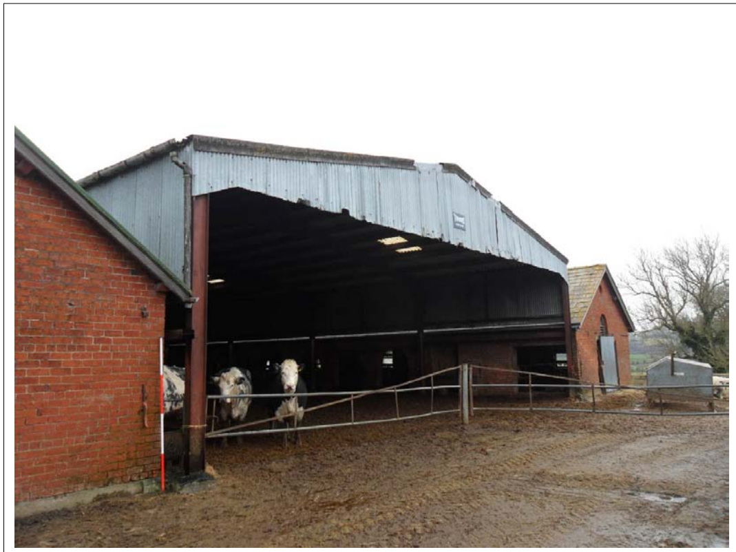
Plate 38: View of further modern steel addition in space between animal ranges 4 and 5. Scale 1x2m, Looking east
