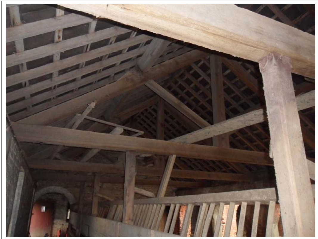
Plate 113: View of roof construction and ceiling trusses within animal range 1
