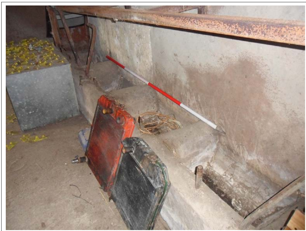
Plate 162: Individual feed stalls within milking area. Scale 1x2m
