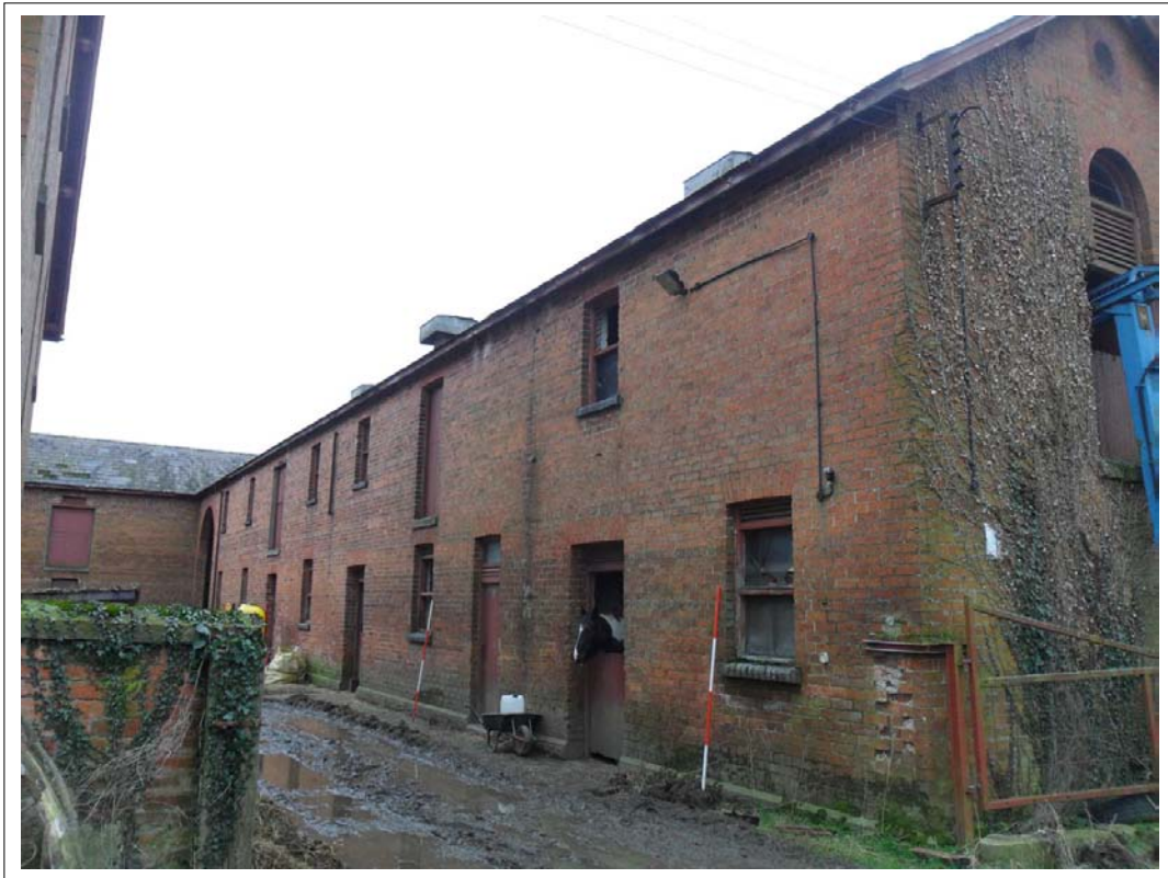
Plate 57: Oblique view of entrances to stable block facing into internal courtyard Scales 2x2m, Looking west
