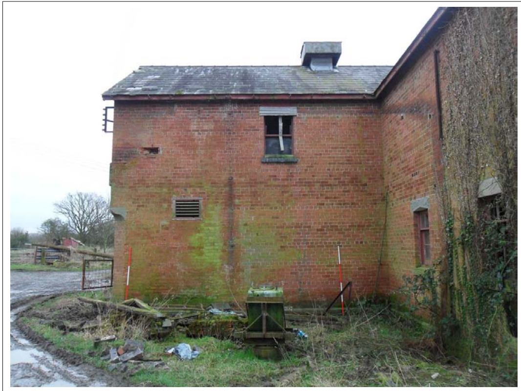
Plate 41: View of gable end side wall of stable block, Scales 2x2m Looking south east
