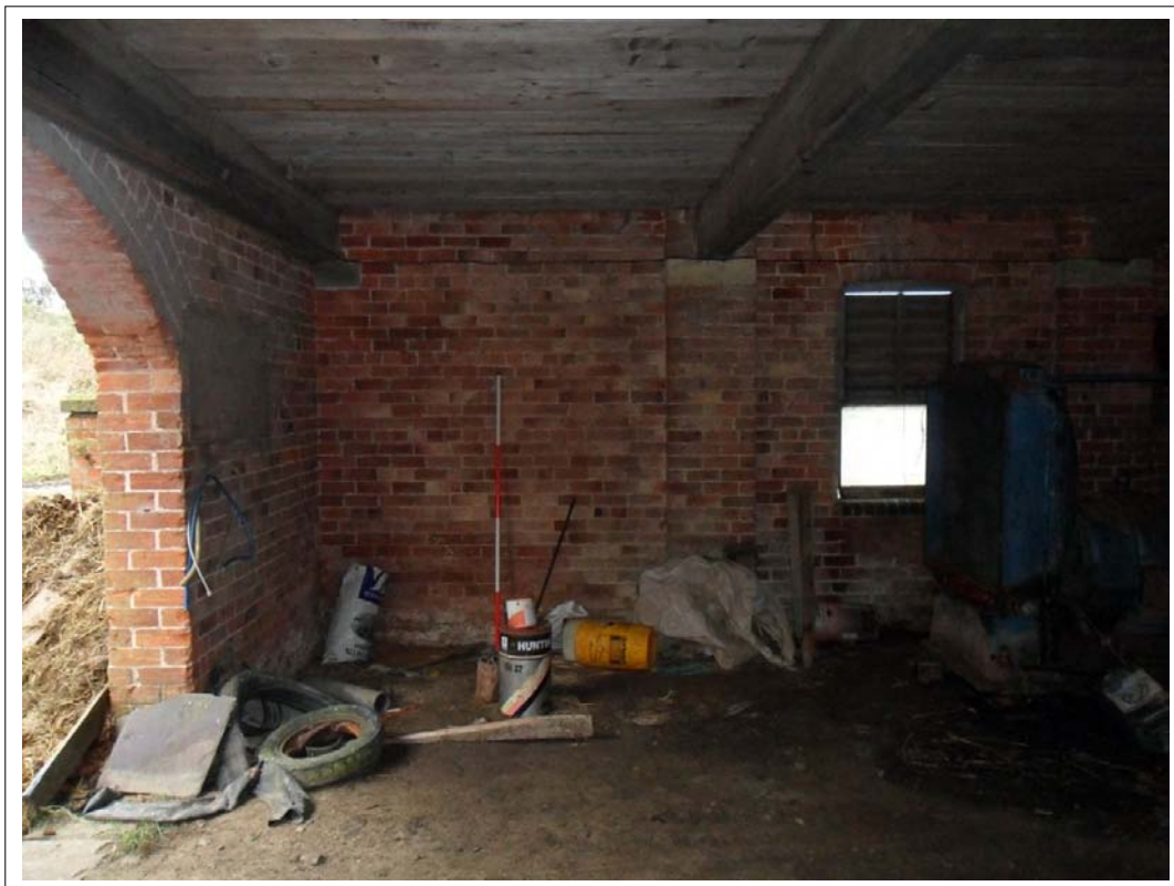
Plate 79: View on inside of cart store, now a workshop. Scale 1x2m
