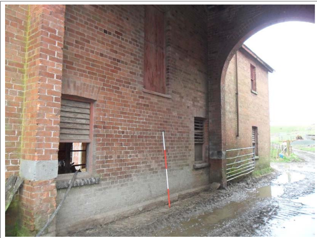
Plate 62: Oblique view of wall beneath courtyard archway. Scales 1x2m Looking west
