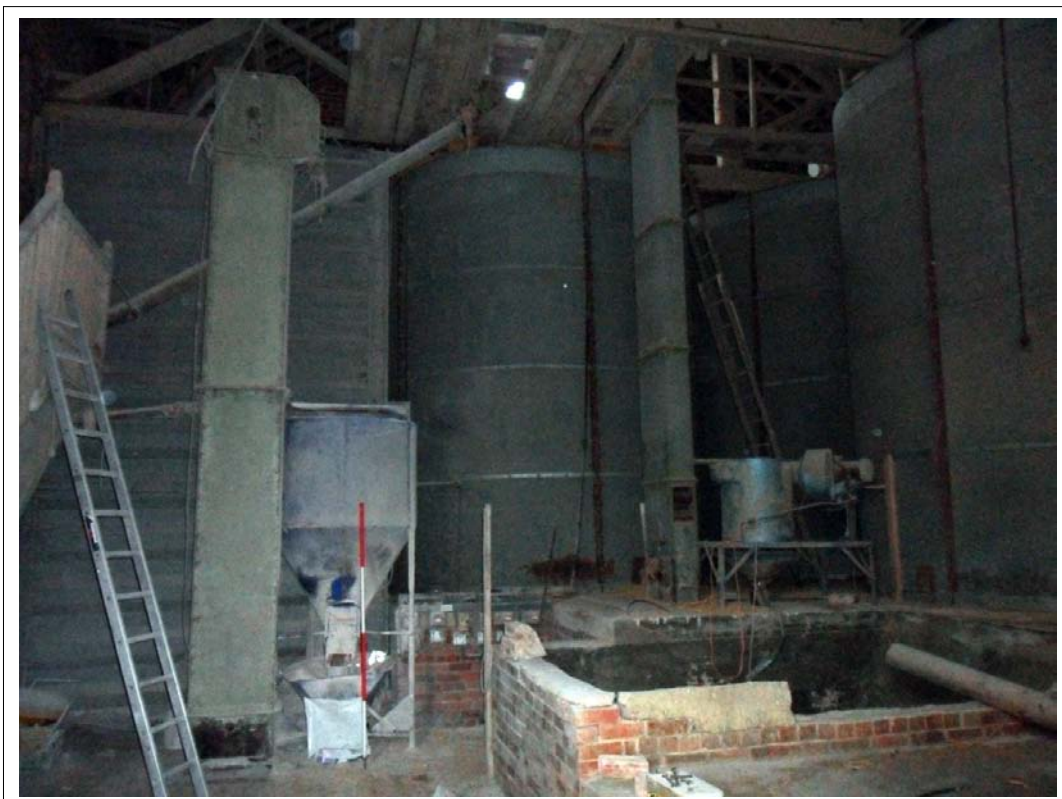
Plate 86: View of storage silos within main section of building Scale 1x2m
