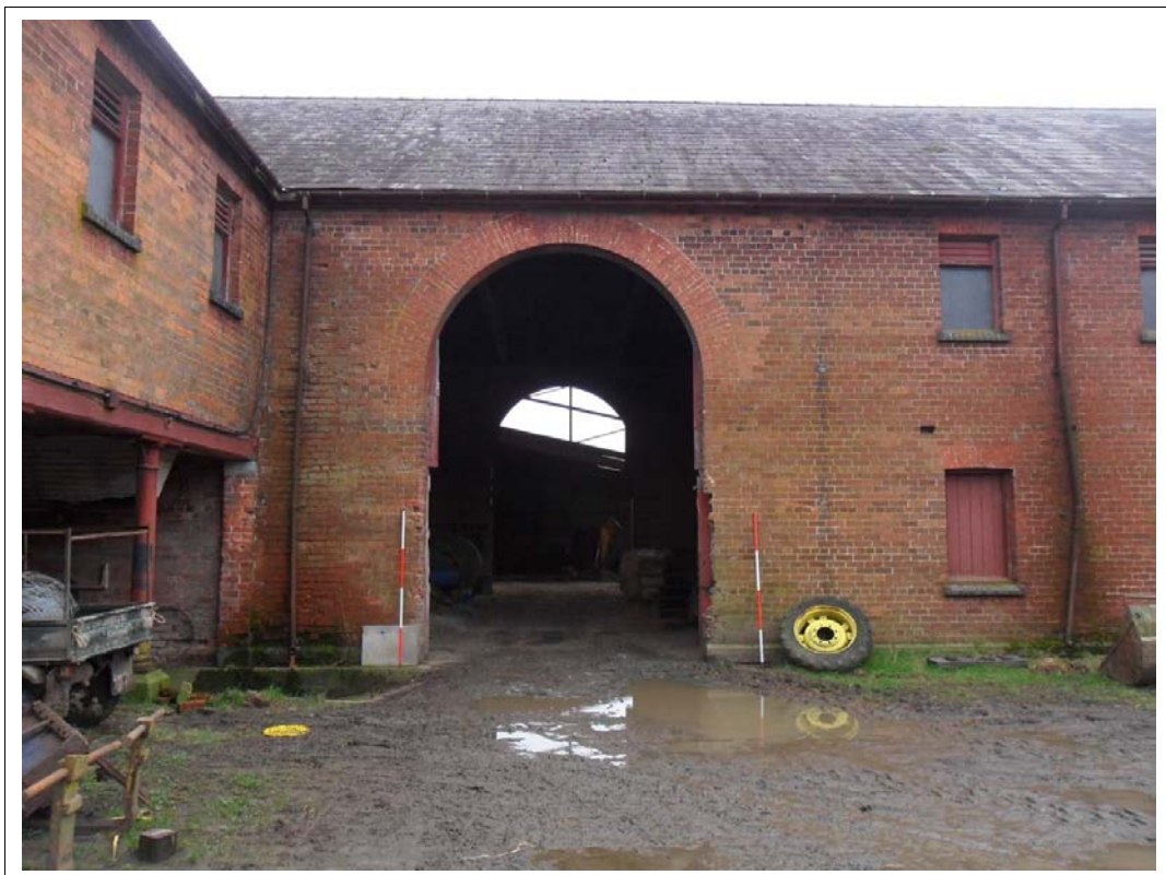
Plate 70: View of arched entrance into main building section Scales 2x2m, Looking south east
