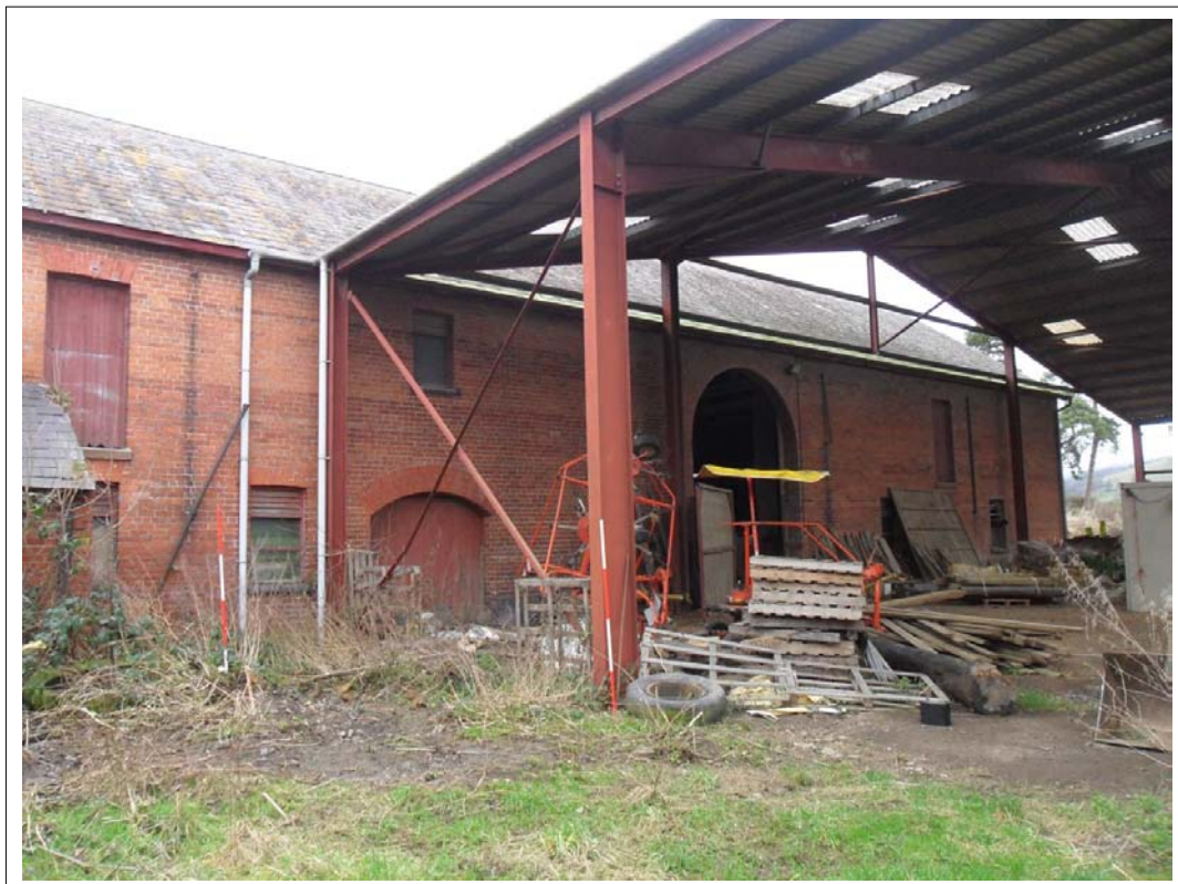
Plate 50: Oblique view of south east wall of main building including modern steel structure, Scales 2x2m, Looking north
