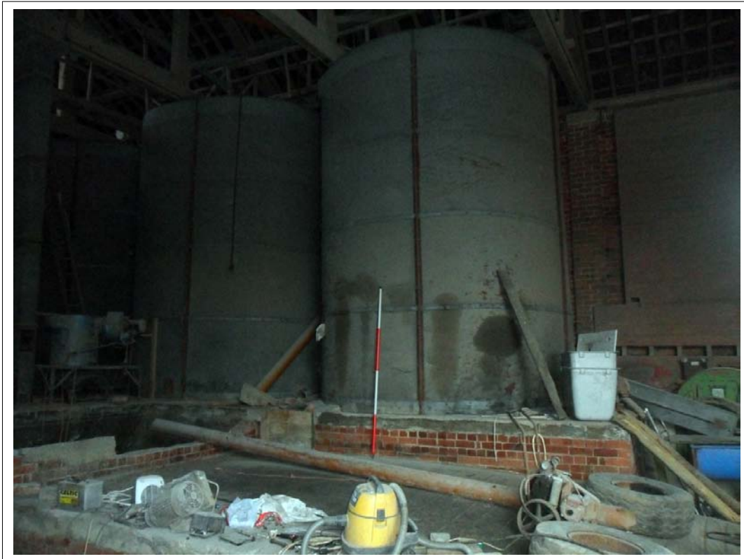
Plate 85: View of storage silos within main section of building Scale 1x2m
