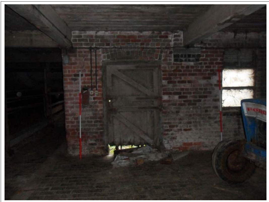
Plate 96: Door between vehicle storage area out into central courtyard Scales 2x2m
