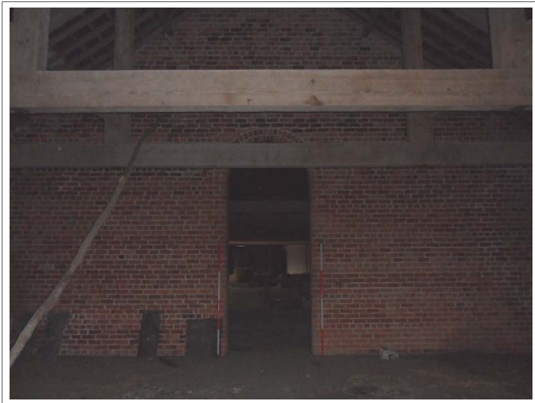
Plate 156: View of doorway into hay storage area from upper floor of animal range 3 Scales 2x2m
