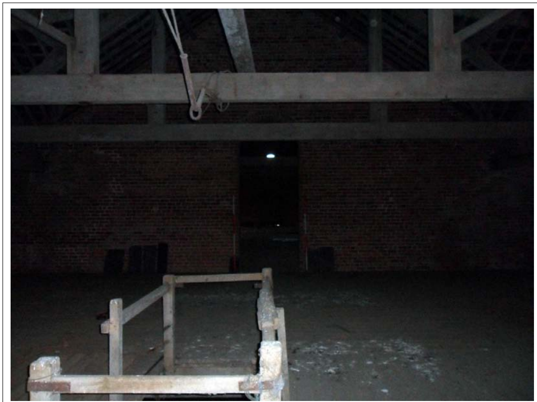
Plate 144: View south west from hay storage area. Access door to upper floor of animal range 3 in background. Stepped access from lower floor in foreground Scales 2x2m
