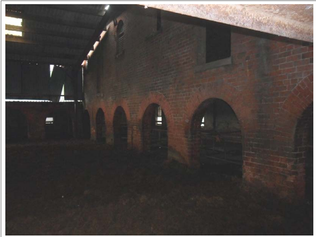
Plate 130: View across covered courtyard (beneath steel frame structure) between animal ranges 4 and 5.
