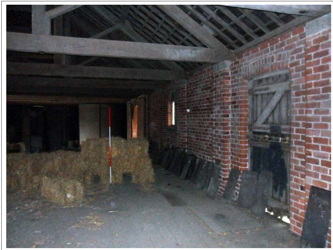
Plate 139:View of door within upper floor wall, Scale 1x2m
