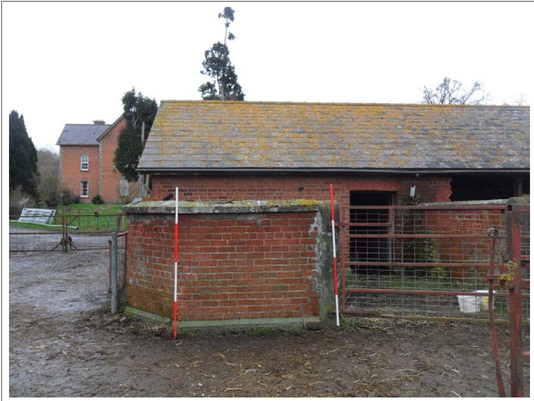
Plate 17: View of small yard enclosure wall at end of animal range Scales 2x2m, Looking north west
