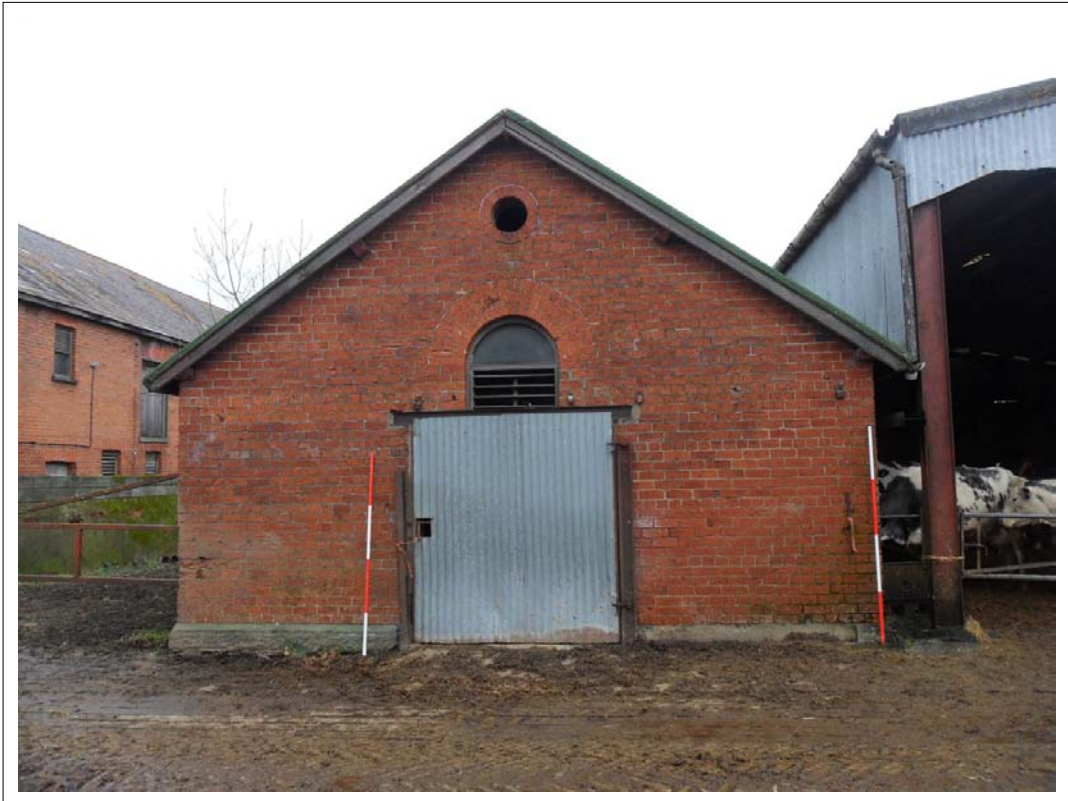
Plate 37: View of gable end of animal range 4. Note later door insertion beneath window. Scales 2x2m, Looking north east
