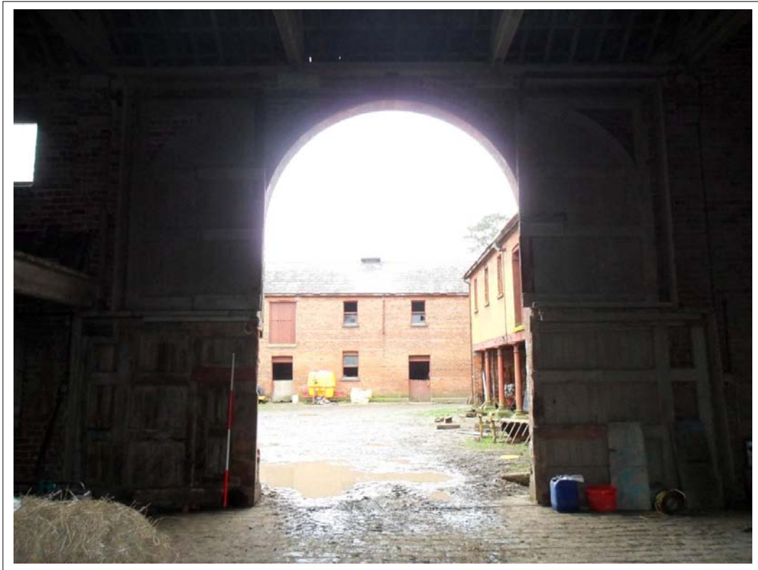
Plate 91: View through arched doorway into central courtyard Scale 1x2m
