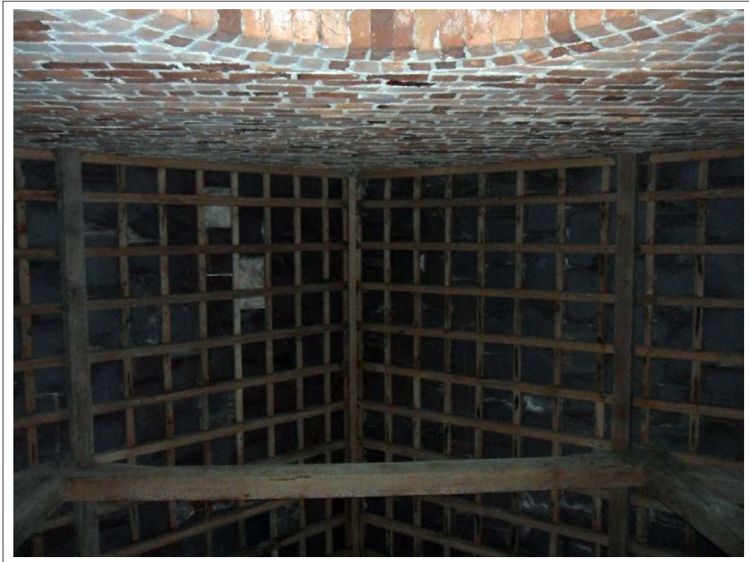
Plate 155: View of roof construction above upper floor of animal range 3
