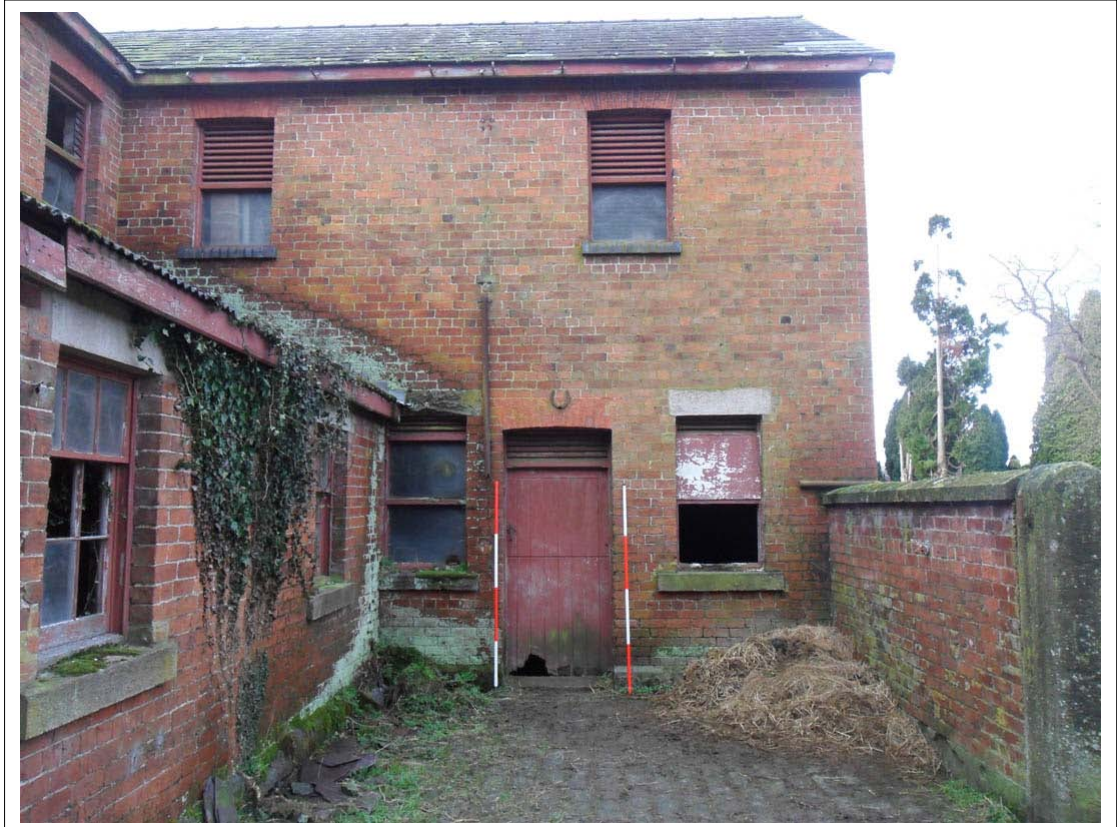
Plate 7: View of single block stable, Scales 2x2m, Looking south west
