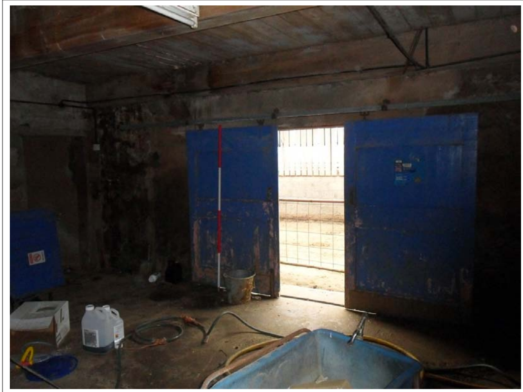
Plate 157: Oblique view out of double doors from boiler room at end of animal range 3 ground floor, Scale 1x2m
