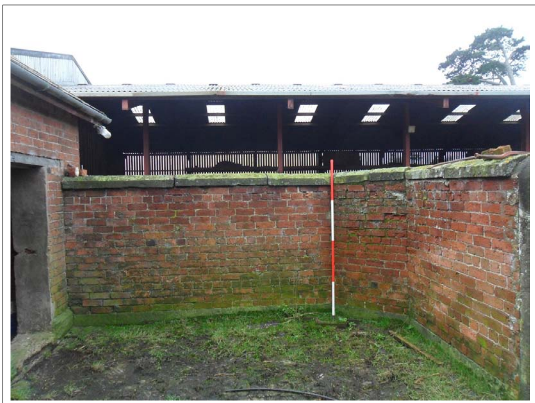
Plate 26: Inside face of enclosed yard wall, Scale 1x2m, Looking south west
