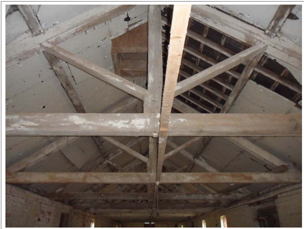
Plate 186: View of roof construction in stable block upper floor
