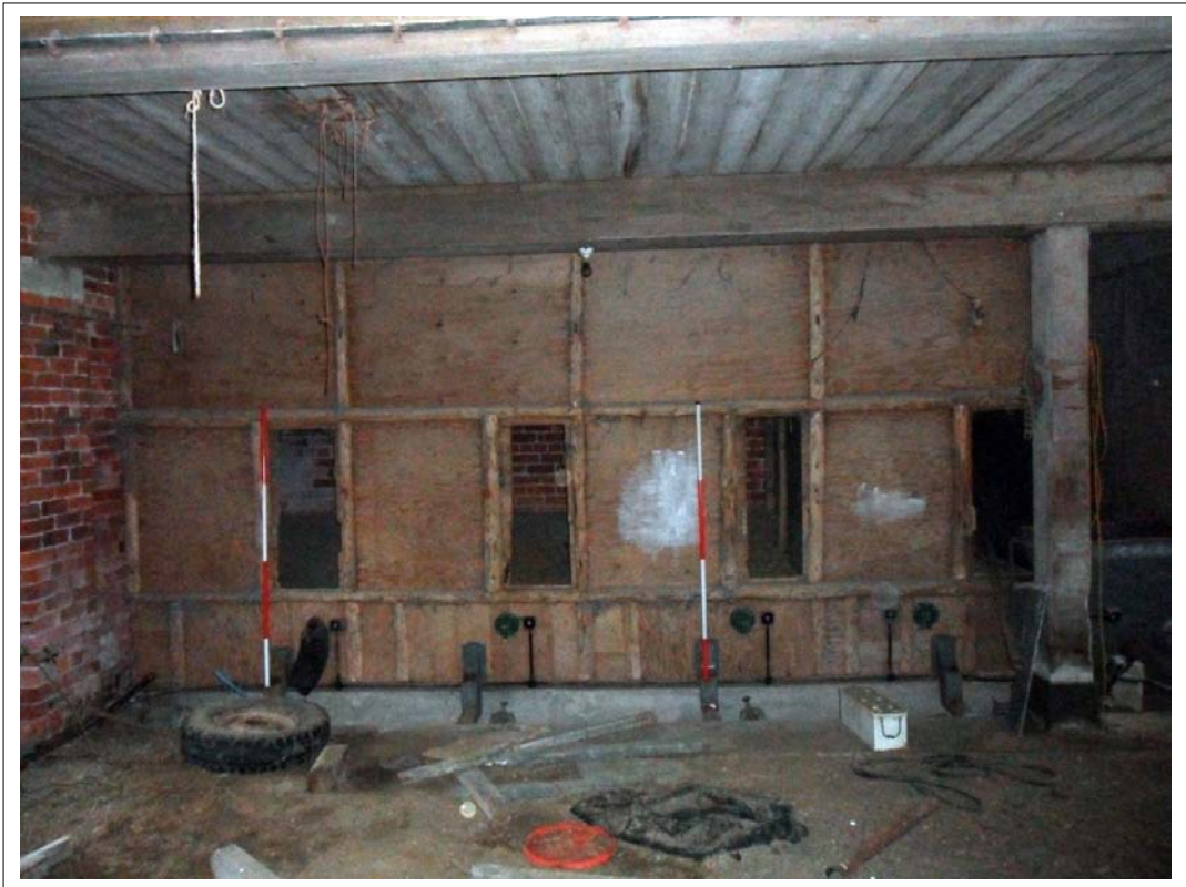
Plate 82: View of feed dispenser within cart store. Scales 2x2m
