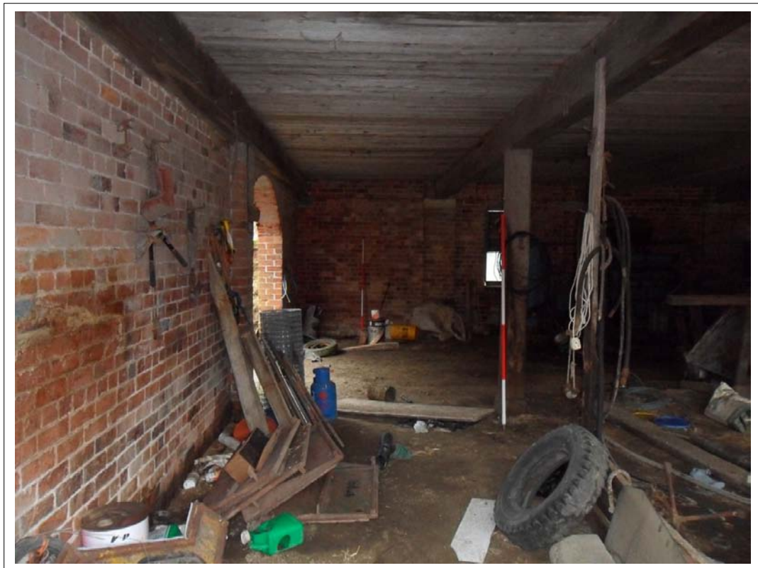
Plate 78: View inside cart store area, now a workshop. Scales 2x2m
