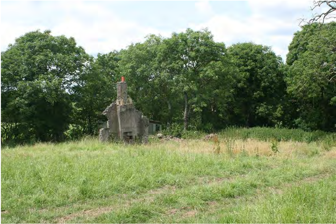
Photo 3: Looking northwest at the remains of North Fenton Farm, with a modern static caravan behind.
