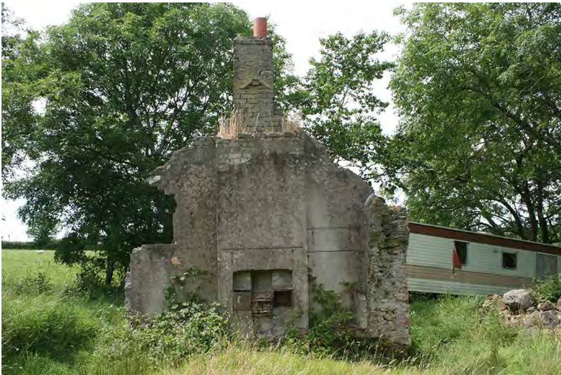
Photo 4: Looking west at the surviving gable wall of North Fenton.
