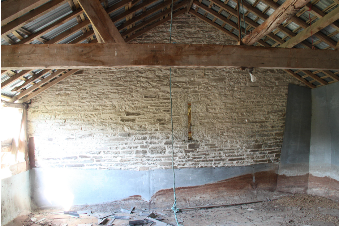
Plate 63 - AD011_063: Ventilation slit in south-west gable of barn.
