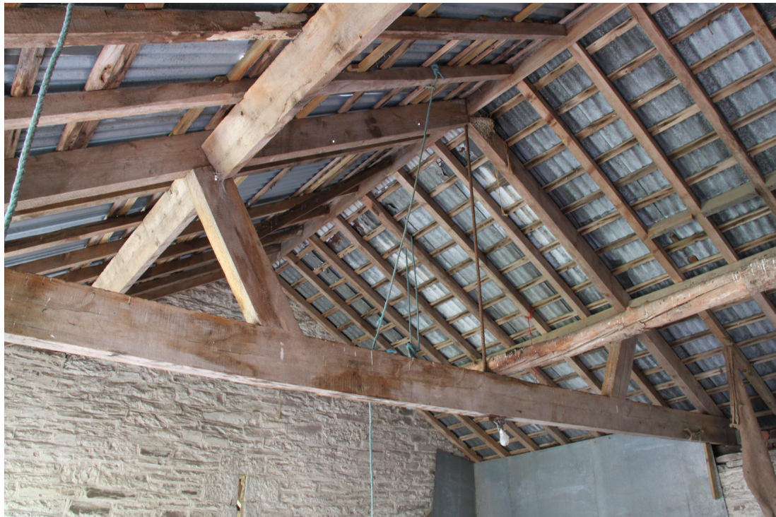
Plate 58 - AD011_058: Truss to granary/hay loft with clapsed purlins and raking struts.
