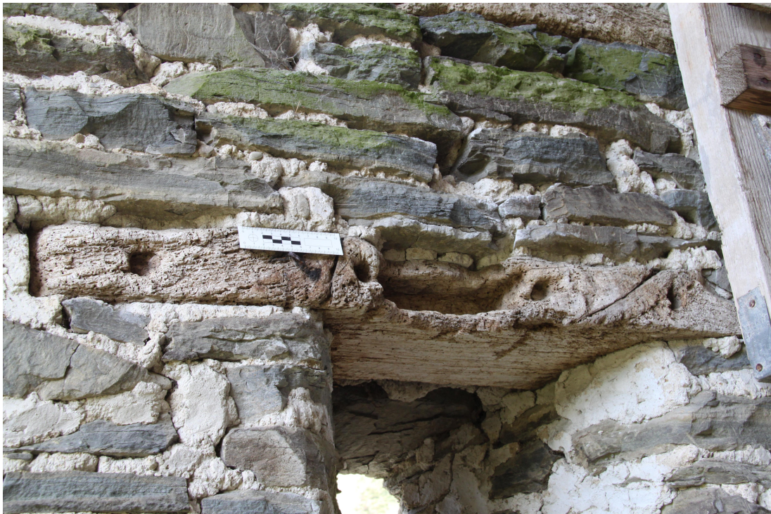
Plate 28 - AD011_028: Detail of reused timber lintel in north-east gable, showing mortice and stave holes.
