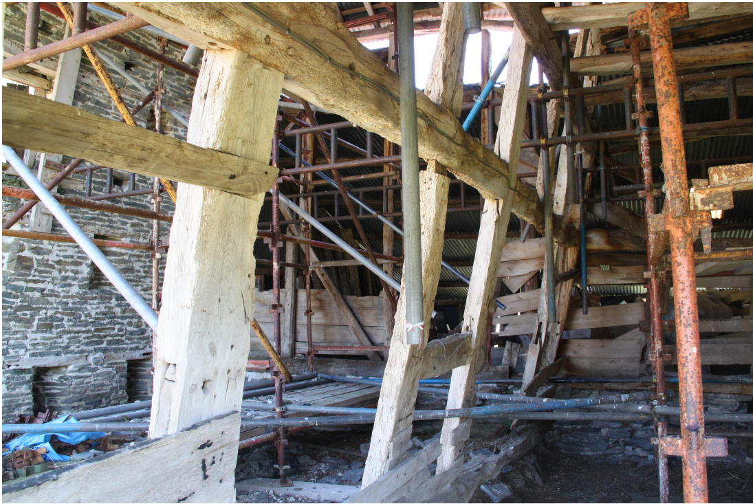
Plate 17 - AD011_017: Reverse face of Truss 1.
