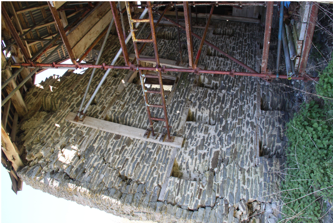
Plate 10 - AD011_010: Internal view of north-east gable, showing ventilation slits.
