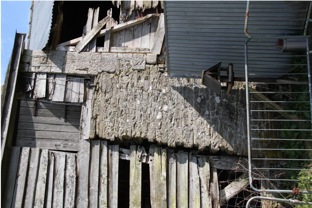
Plate 54 - AD011_054: Stone wall and stub to south-west gable.
