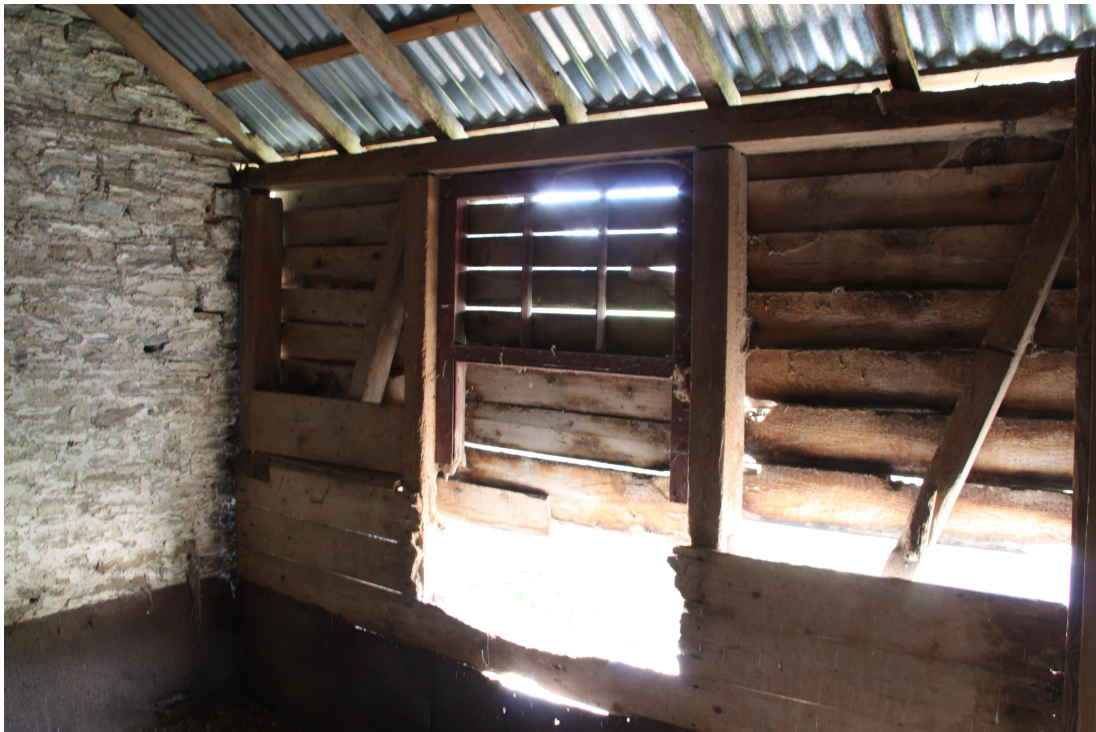
Plate 62 - AD011_062: Remains of 9 light casement window.
