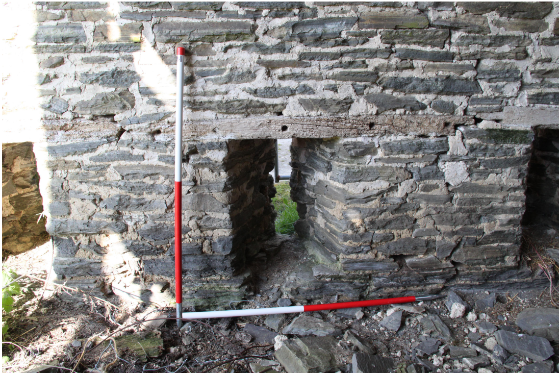
Plate 27 - AD011_027: Ventilation slit in north-east gable.
