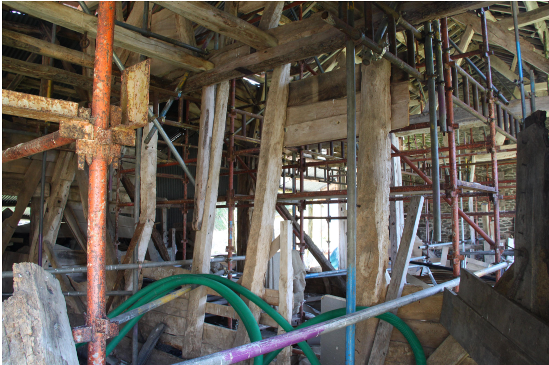
Plate 16 - AD011_016: Later studs in bay 2.
