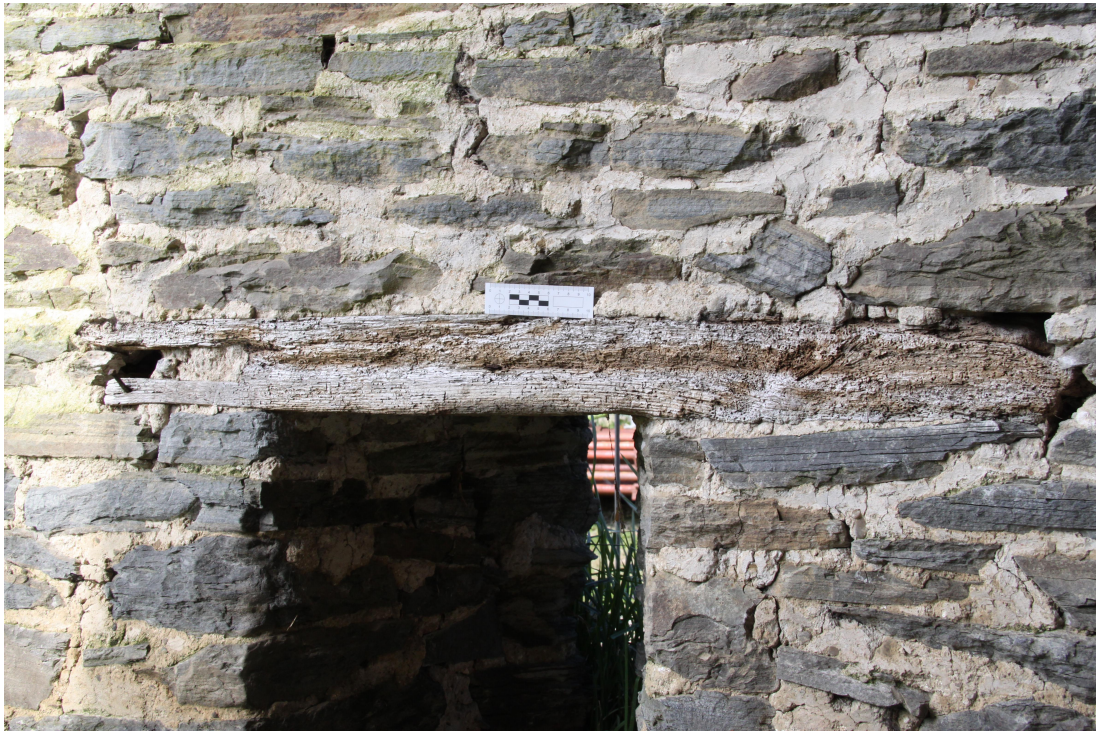
Plate 29 - AD011_029: Detail of reused timber lintel in north-east gable, showing stave groove.
