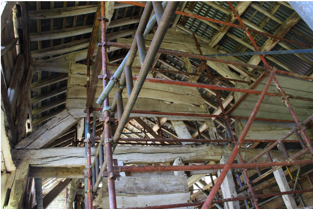
Plate 18 - AD011_018: Internal weatherboarding to subdivide barn; to rear of truss 2.
