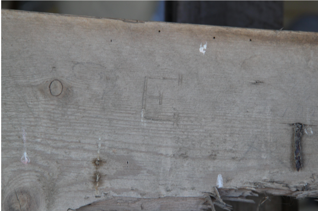
Plate 39 - AD011_039: Carved initial in weatherboarding to rear of bay 2.
