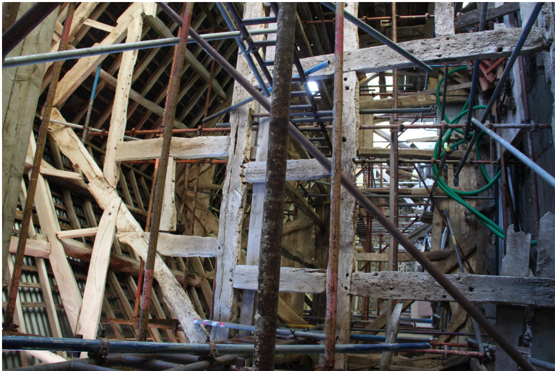
Plate 12 - AD011_012: Truss 1, viewing towards south, showing square panelled box framing.
