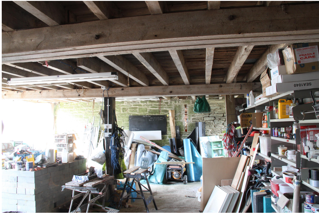
Plate 57 - AD011_057: Cart shed.
