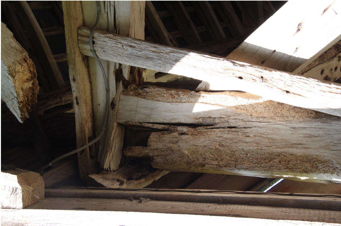
Plate 48 - AD011_048: Gunstock head to posts.
