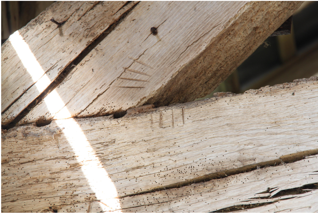
Plate 43 - AD011_043: Carpenters marks on tie beam and principle rafter of truss 2.
