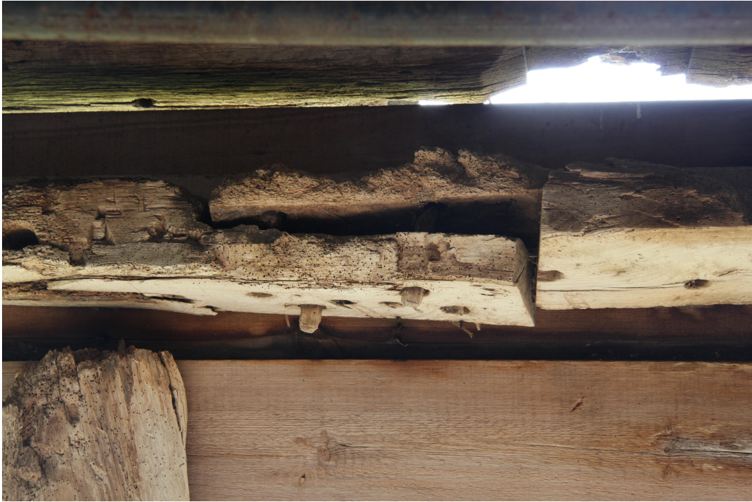
Plate 47 - AD011_047: Side halved lap join in rail.
