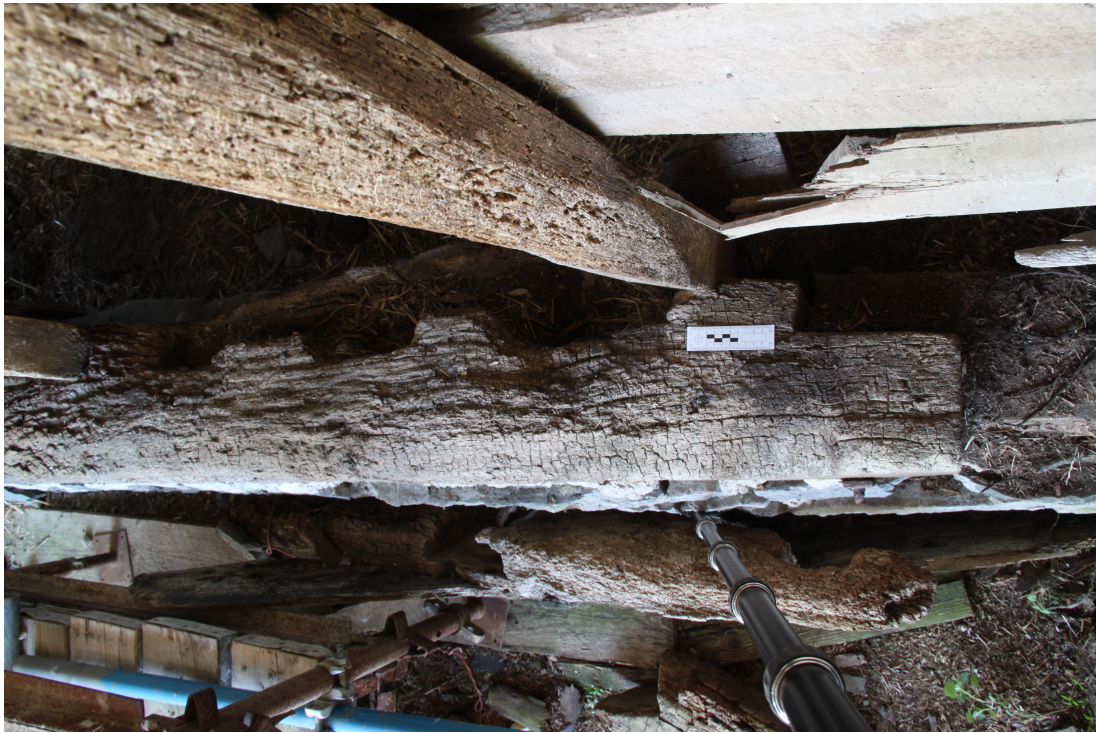
Plate 35 - AD011_035: Reused floor beam, circa late C16th. Showing central joist mortises.
