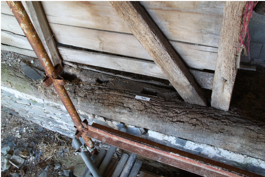
Plate 34 - AD011_034: Reused floor beam, circa late C16th. Showing central joist mortises.
