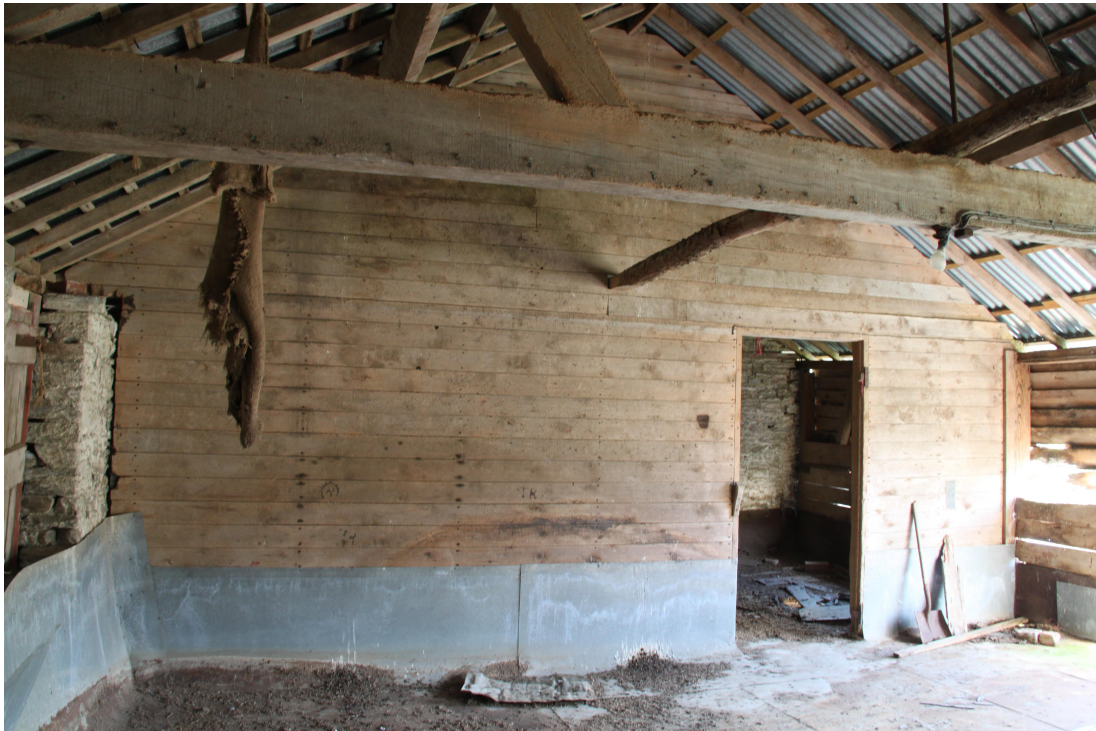
Plate 61 - AD011_061: Panelled wall between granary and hay loft.
