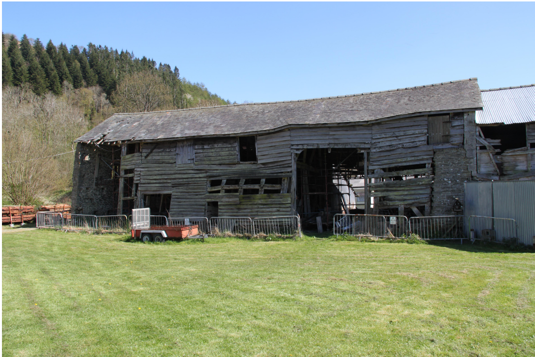
Plate 1 - AD011_001: General view of north-west elevation; Barn.
