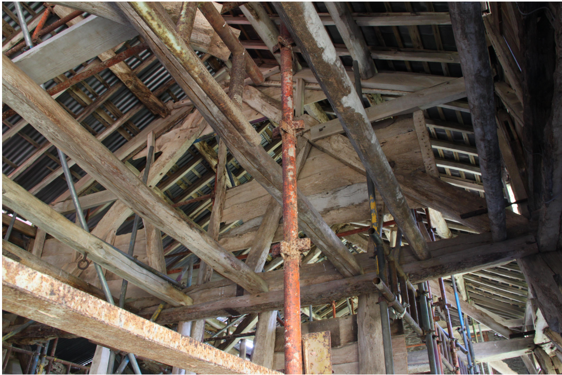
Plate 15 - AD011_015: Truss 2 and joists over bay 2.
