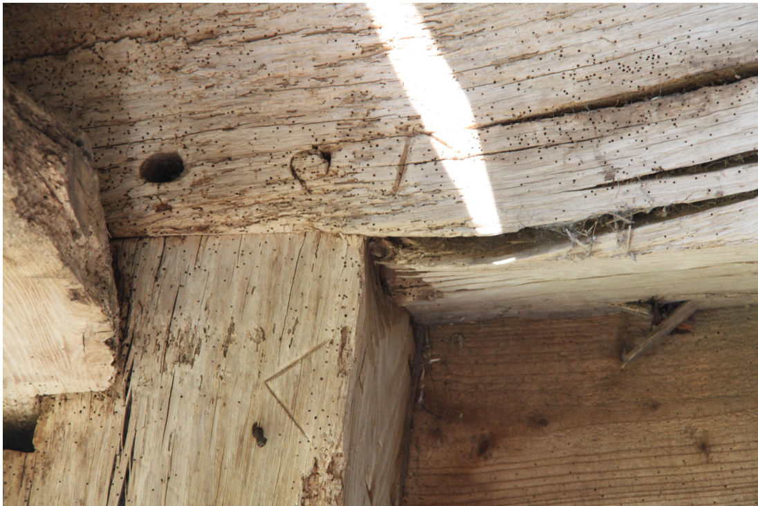
Plate 44 - AD011_044: Carpenters marks on post and tie beam of truss 2.
