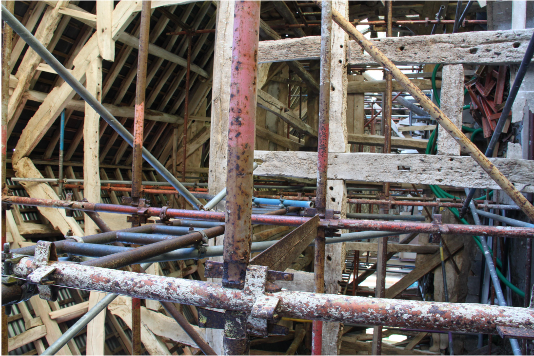
Plate 13 - AD011_013: Truss 1 viewing towards south.
