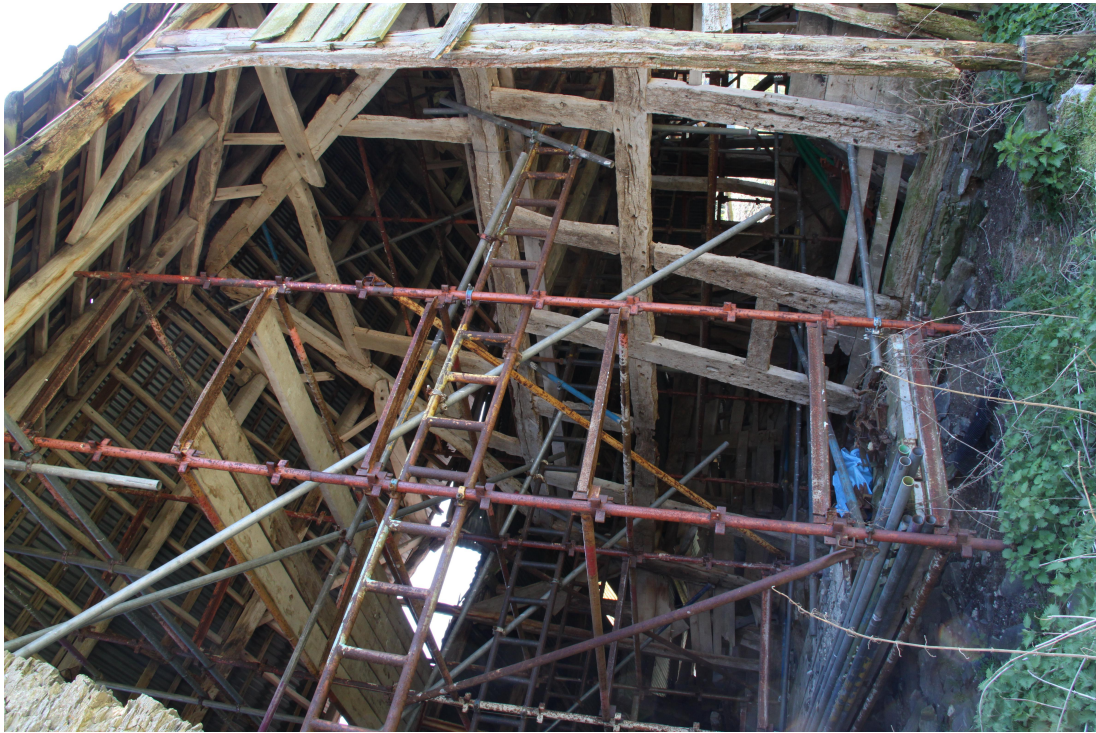
Plate 11 - AD011_011: Truss 1, viewing towards south-east.
