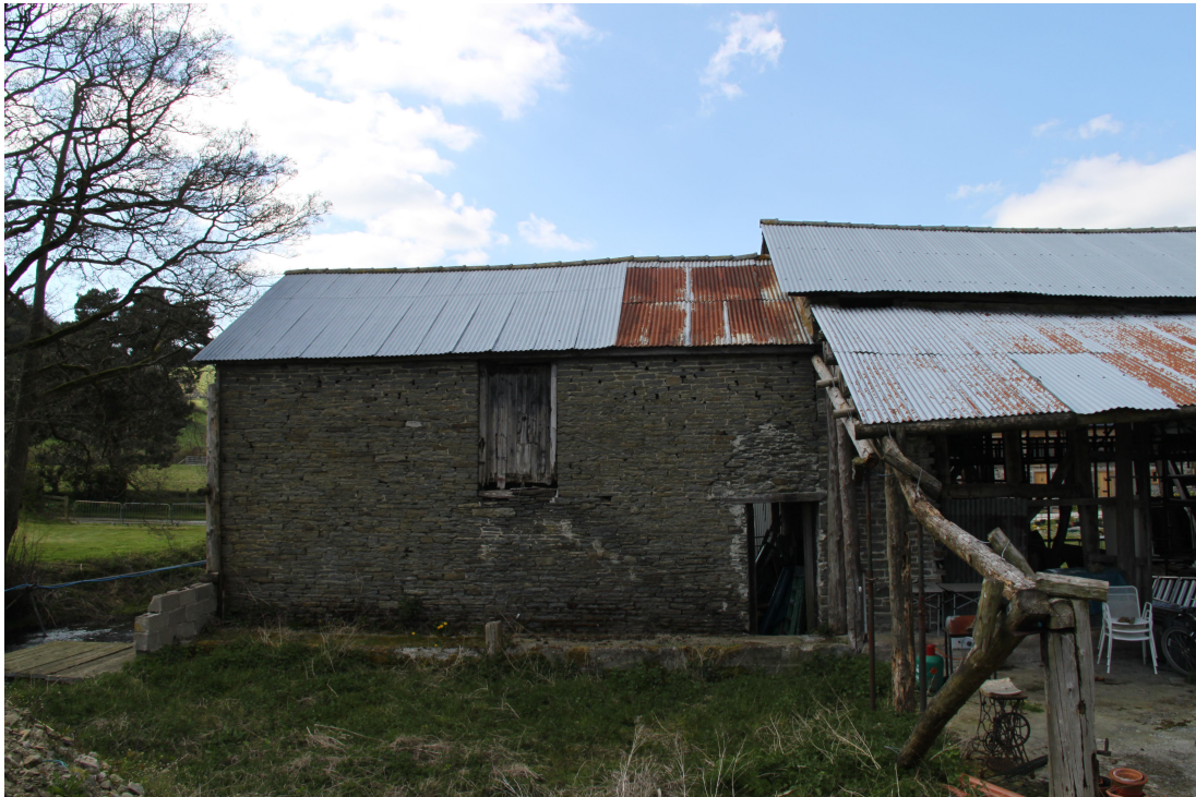
Plate 7 - AD011_007: South-east elevation of cart shed and granary.
