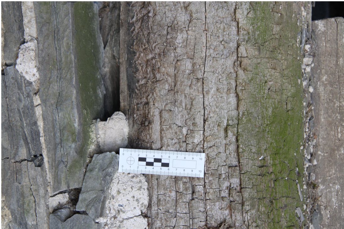
Plate 32 - AD011_032: Reused floor beam, circa late C16th. Showing deep chamfer.
