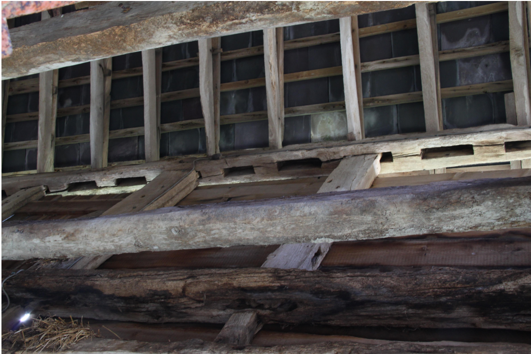
Plate 38 - AD011_038: Detail of reused timber; mortice holes indicate reuse from close studded building.
