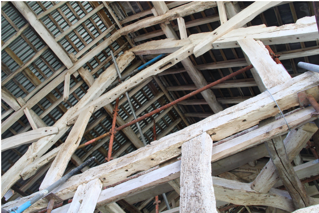
Plate 30 - AD011_030: Detail of stave holes in truss 1.
