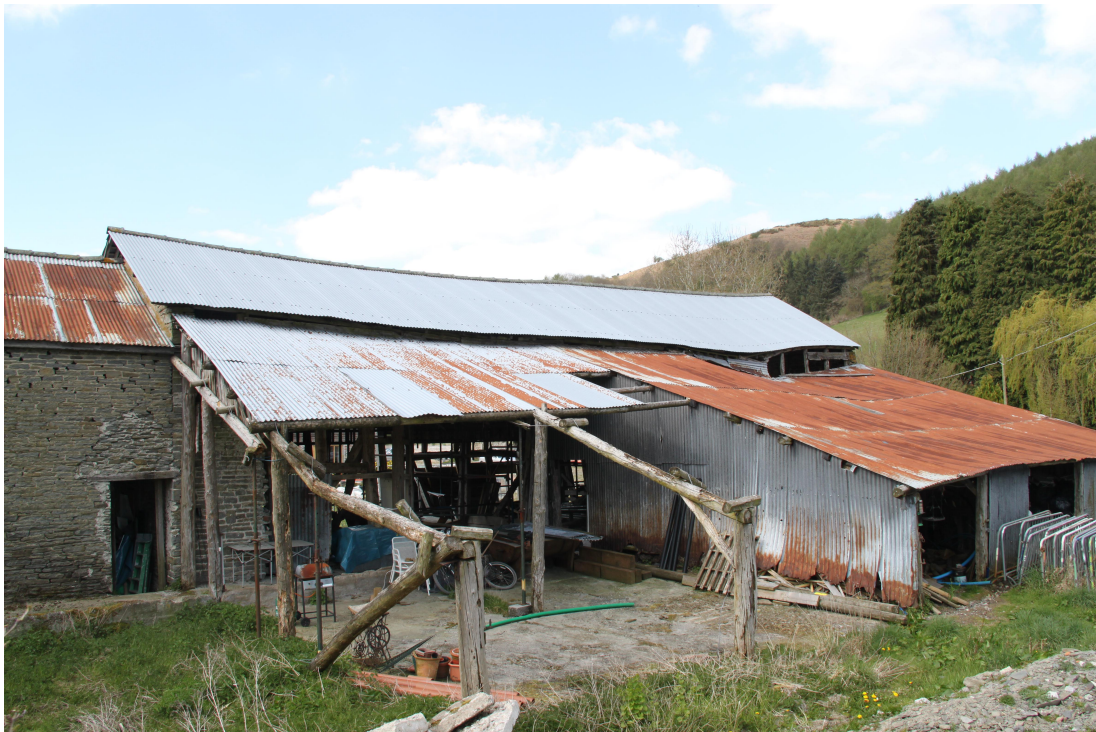
Plate 6 - AD011_006: South-east elevation of barn and rear lean-to.
