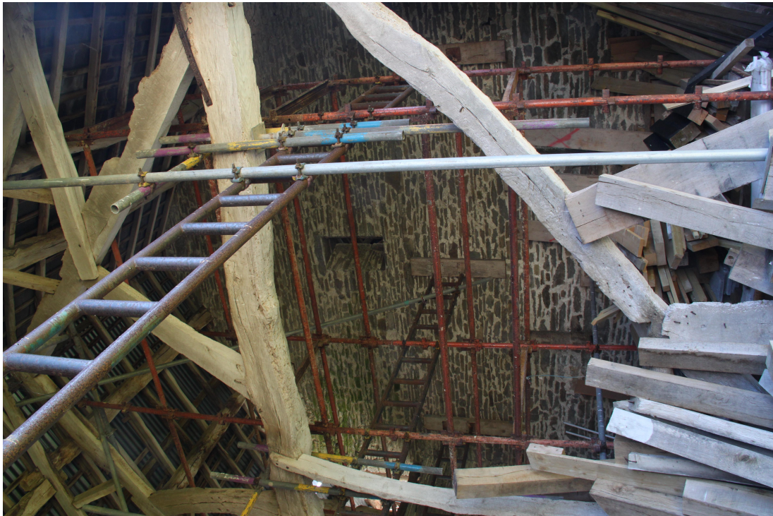
Plate 25 - AD011_025: Ventilation slit in south-west gable.
