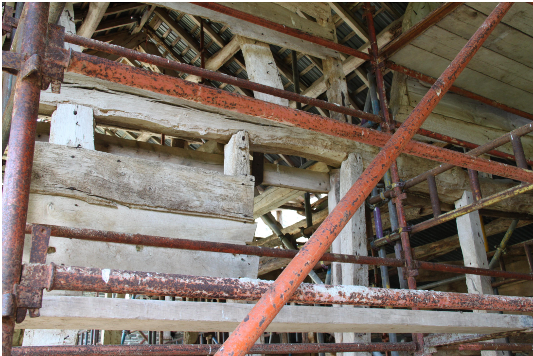
Plate 20 - AD011_020: Internal weatherboarding to subdivide barn; to rear of truss 2.
