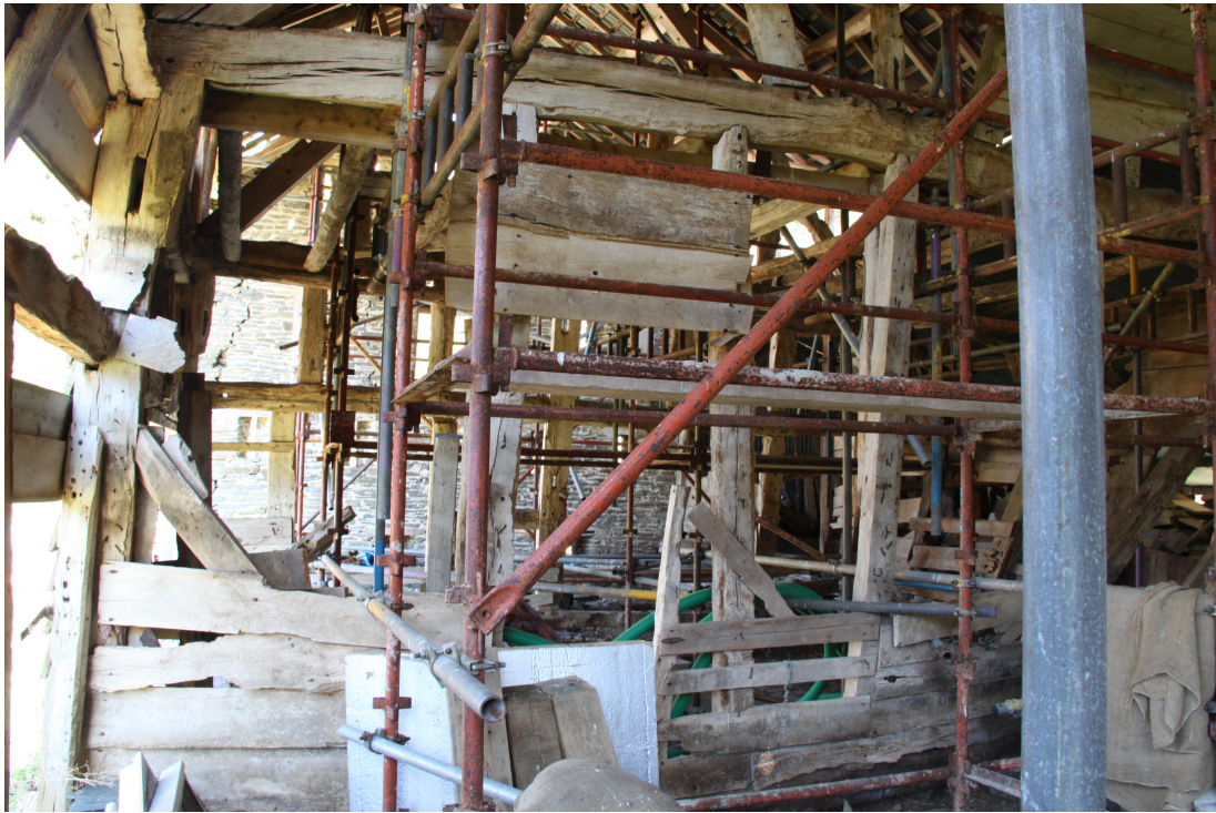
Plate 19 - AD011_019: Internal weatherboarding to subdivide barn; to rear of truss 2.
