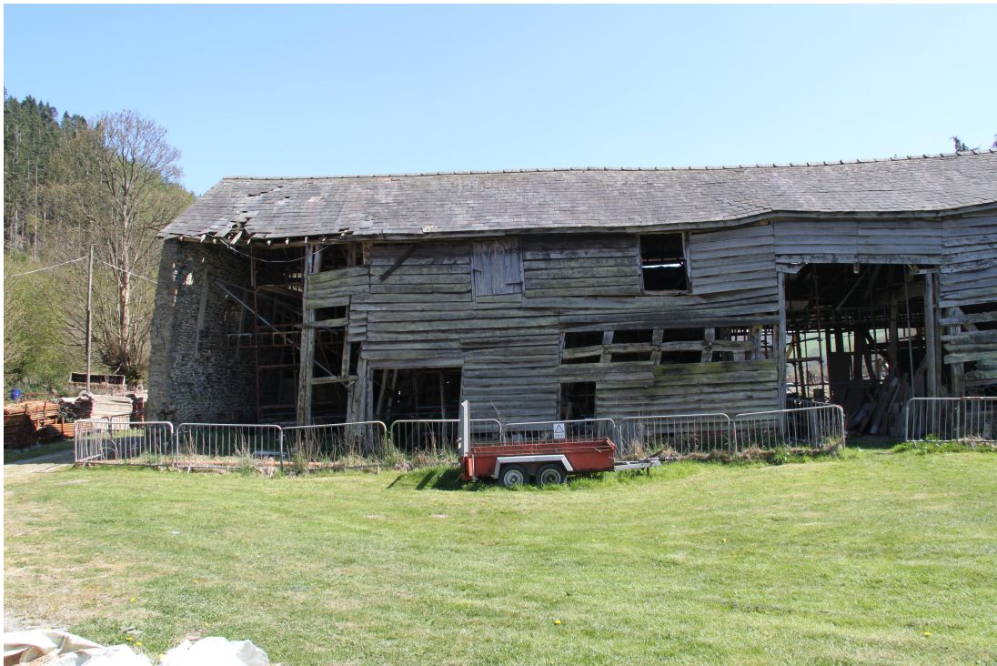
Plate 2 - AD011_002: General view of north-west elevation.
