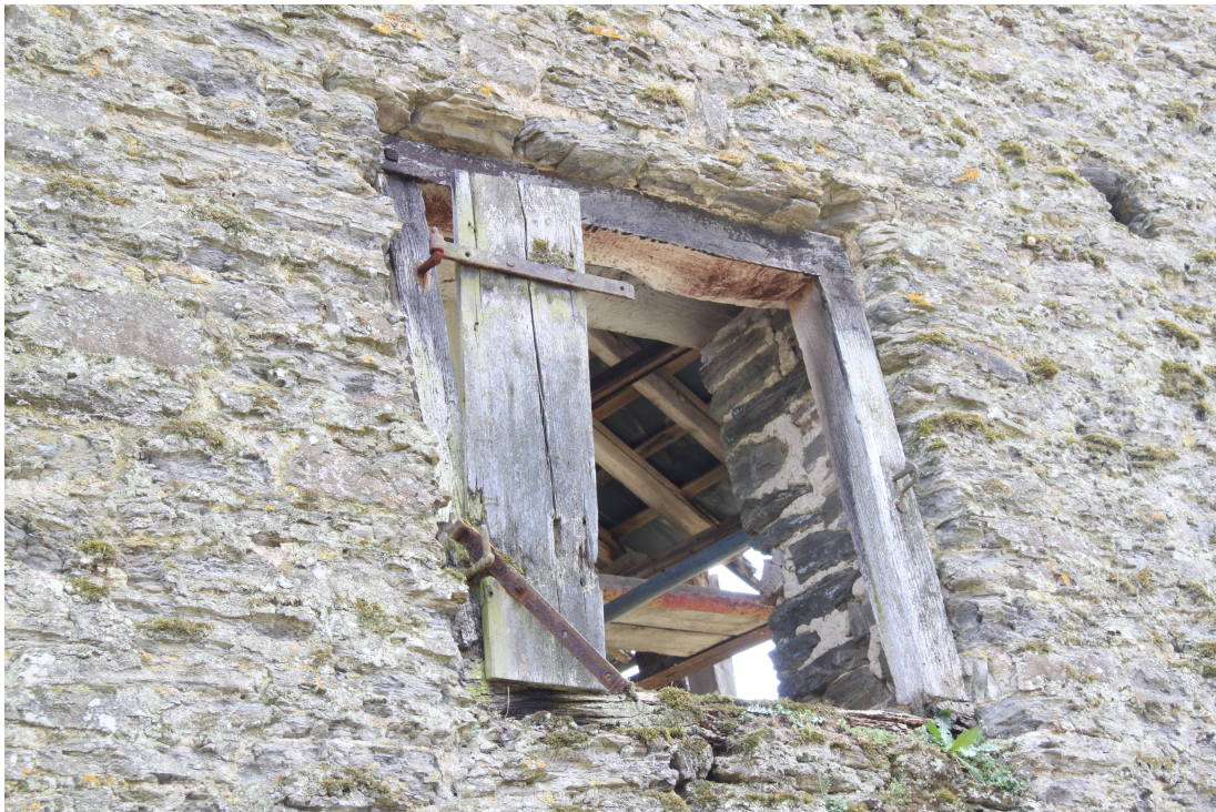
Plate 26 - AD011_026: Window in north-east gable.
