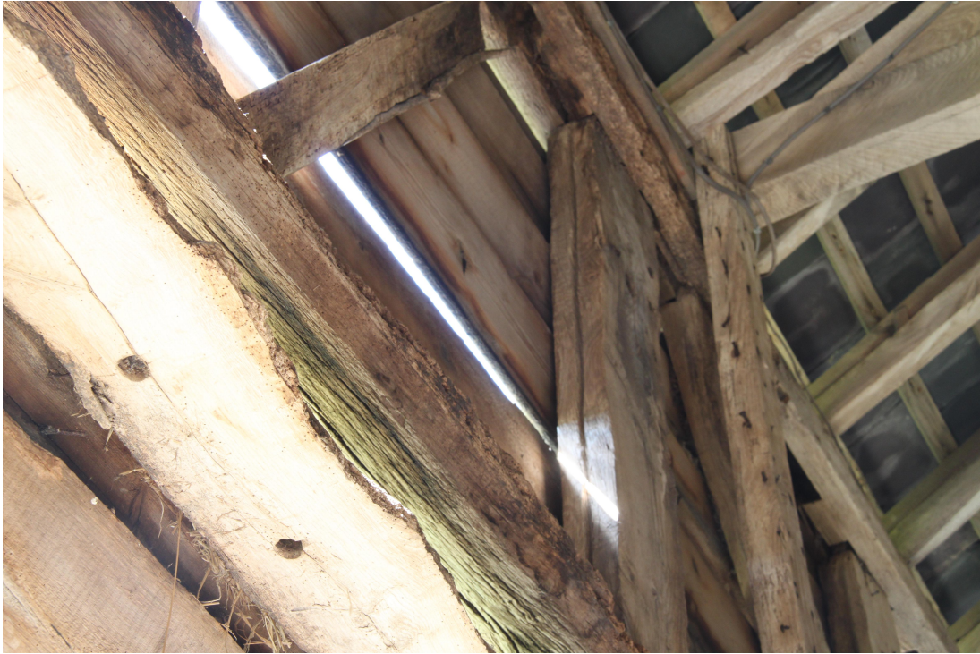
Plate 45 - AD011_045: Stud to raised eave, showing groove, indicating its reuse from a rail.
