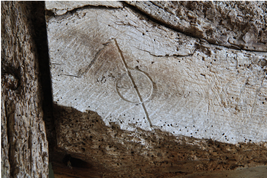
Plate 41 - AD011_041: Carpenters mark on tie beam of truss 1.
