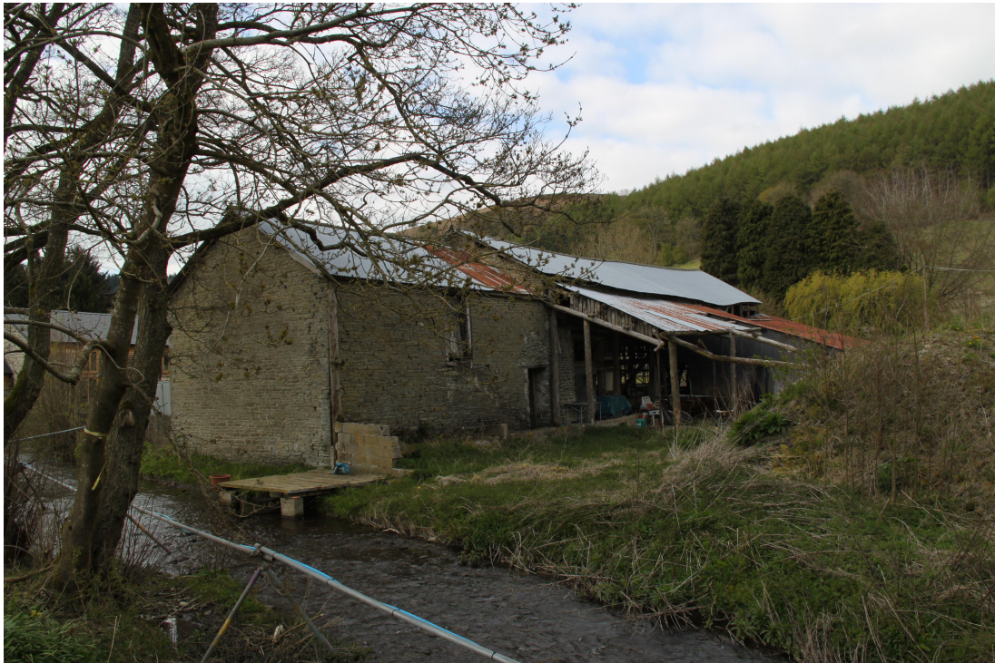
Plate 9 - AD011_009: ¾ view of south-west and south east elevations.
