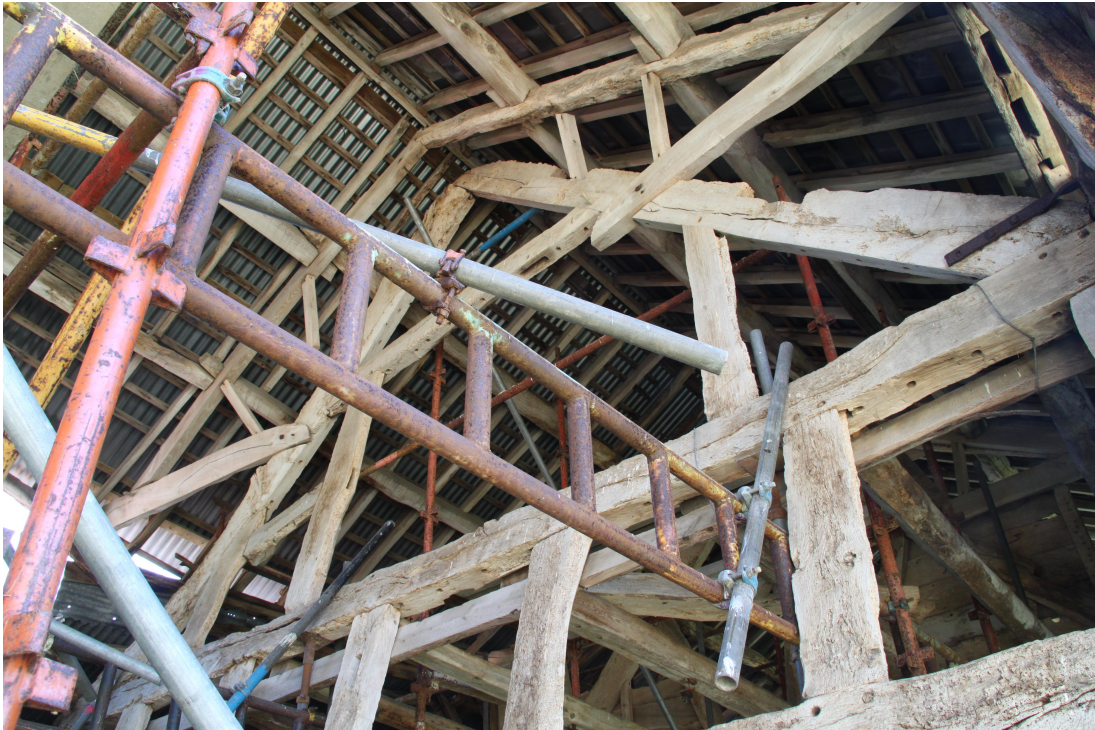
Plate 14 - AD011_014: Truss 1, showing principle rafter roof with later raising.
