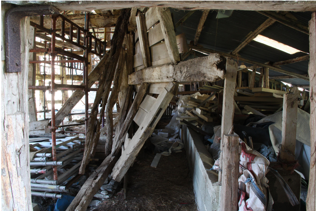
Plate 50 - AD011_050: Rear lateral wall to bay 3.
