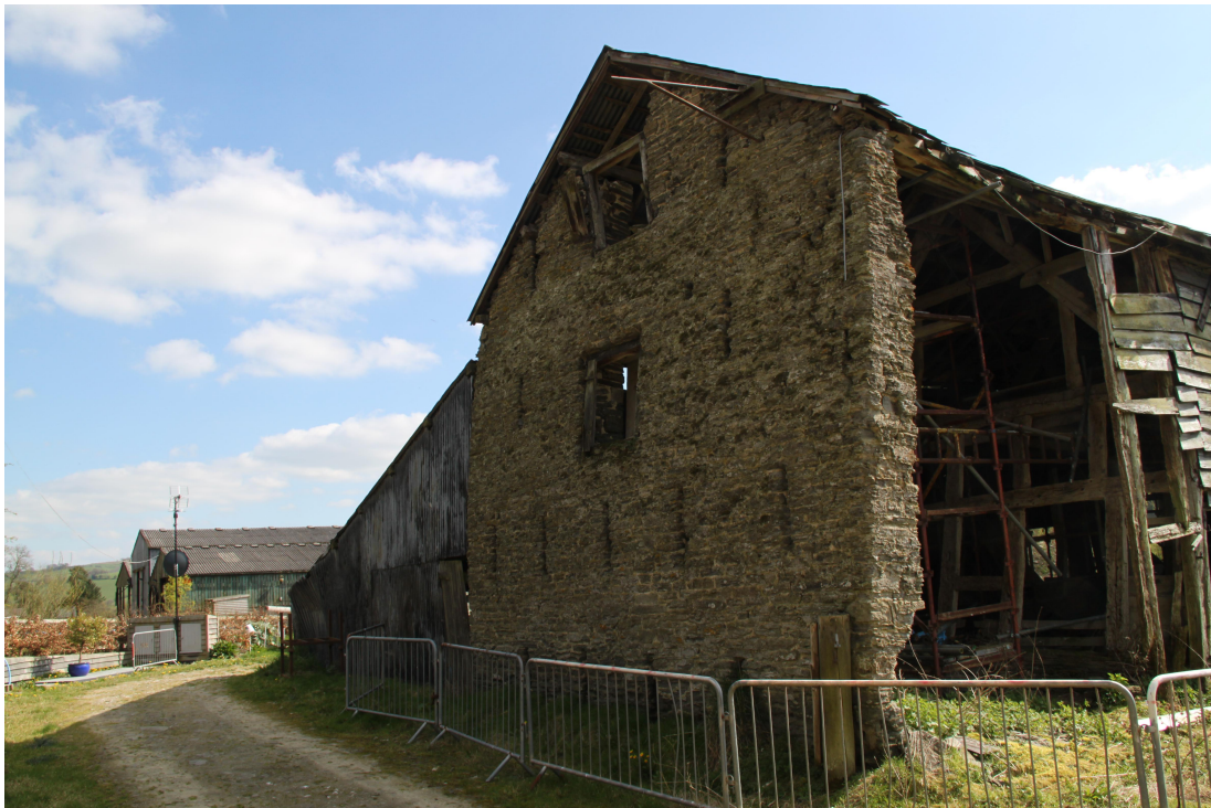
Plate 4 - AD011_004: North-east limestone elevation of barn.
