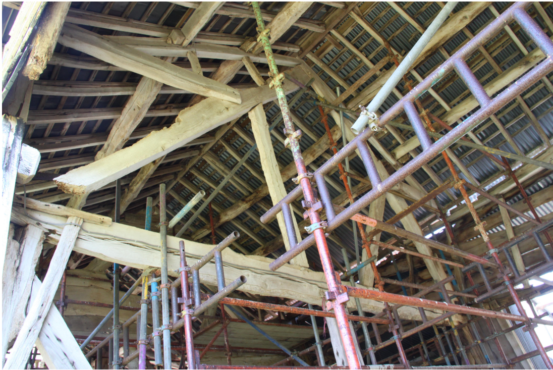
Plate 21 - AD011_021: Truss 3, principle rafters with raking struts. Also showing later raised roof.
