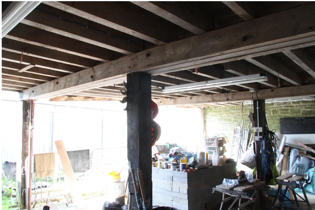
Plate 56 - AD011_056: Cart shed.
