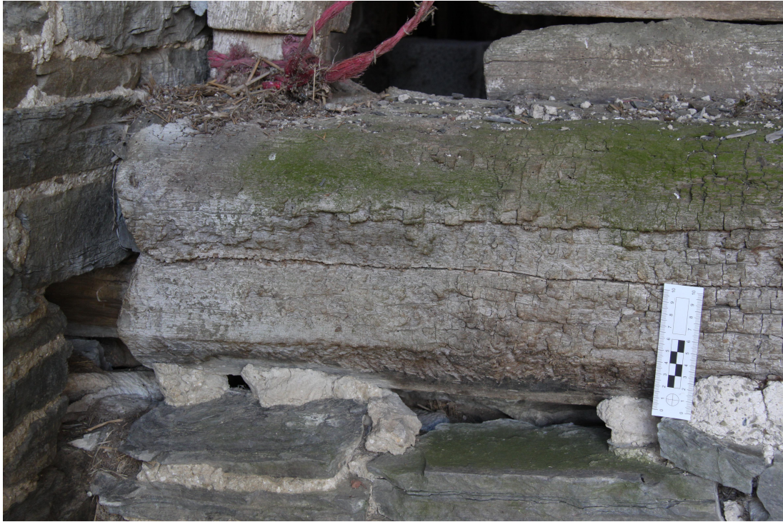
Plate 33 - AD011_033: Reused floor beam, circa late C16th. Showing deep chamfer.
