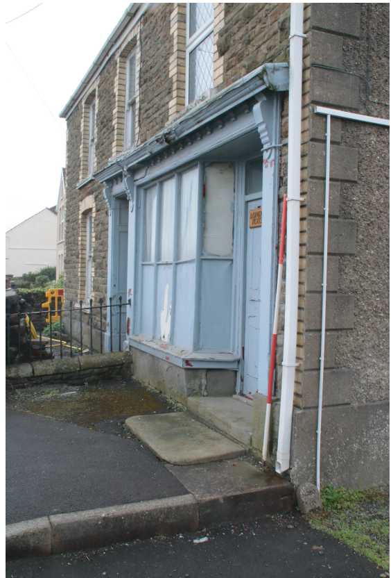
Plate 14. London House, Beach Road, Penclawdd. Shopfront. Oblique view. Looking southeast.
