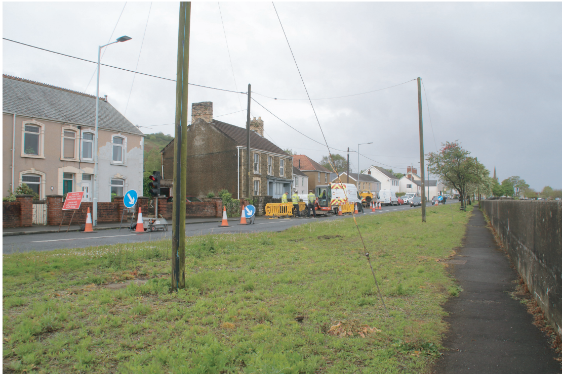
Plate 01. London House, Beach Road, Penclawdd. Looking southwest.
