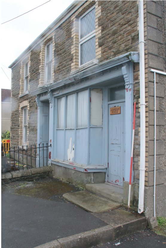
Plate 13. London House, Beach Road, Penclawdd. Shopfront. Oblique view. Looking southeast.
