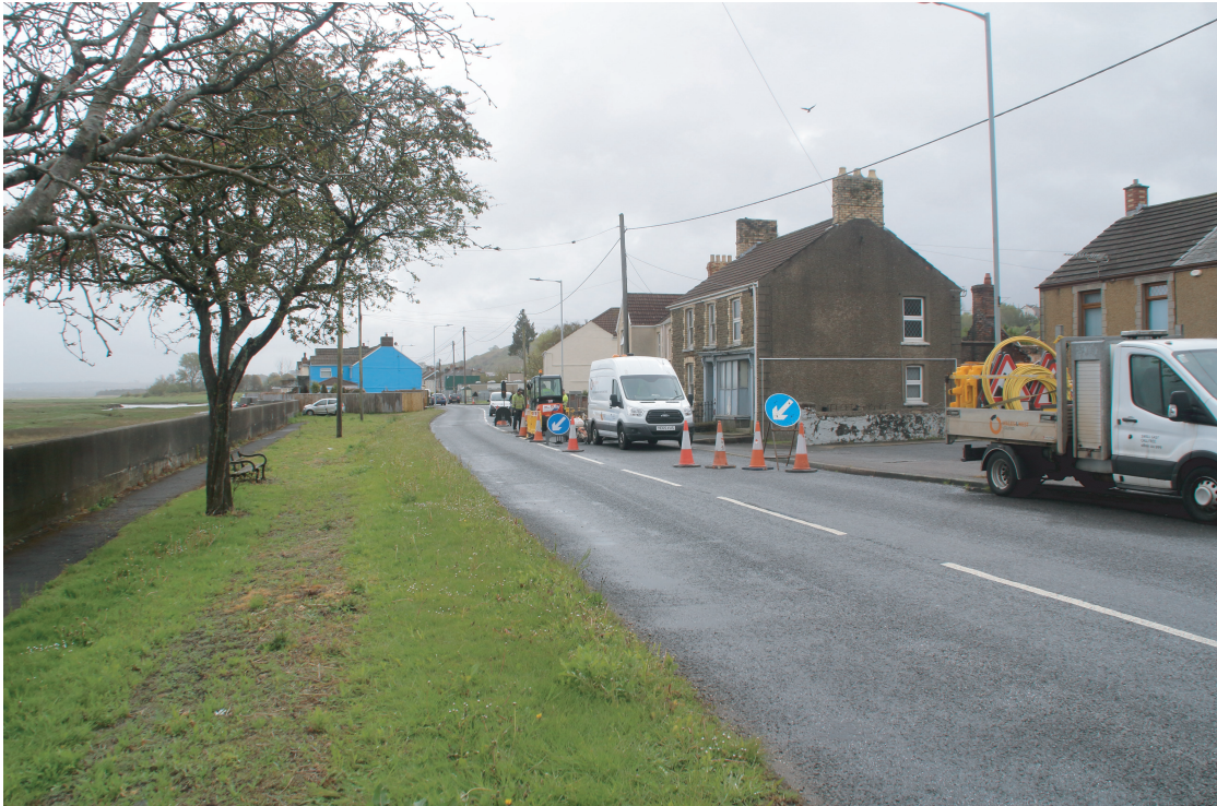
Plate 03. London House, Beach Road, Penclawdd. Looking eastwards.
