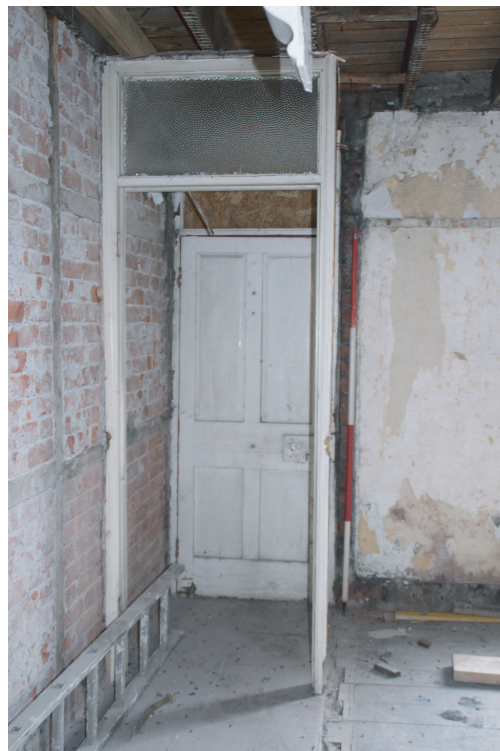
Plate 22. London House, Beach Road, Penclawdd. Internal view of House doorway. Looking north.
