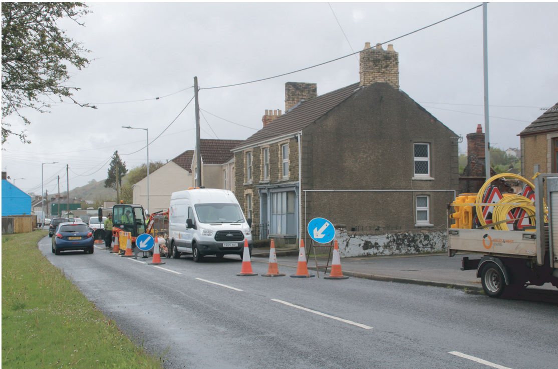
Plate 04. London House, Beach Road, Penclawdd. Looking eastwards.
