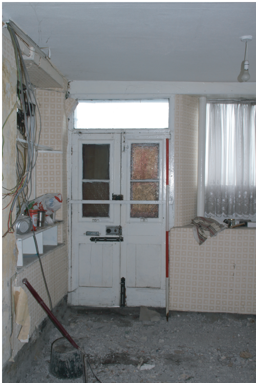
Plate 21. London House, Beach Road, Penclawdd. Internal view of shopfront. Doorway. Looking north.
