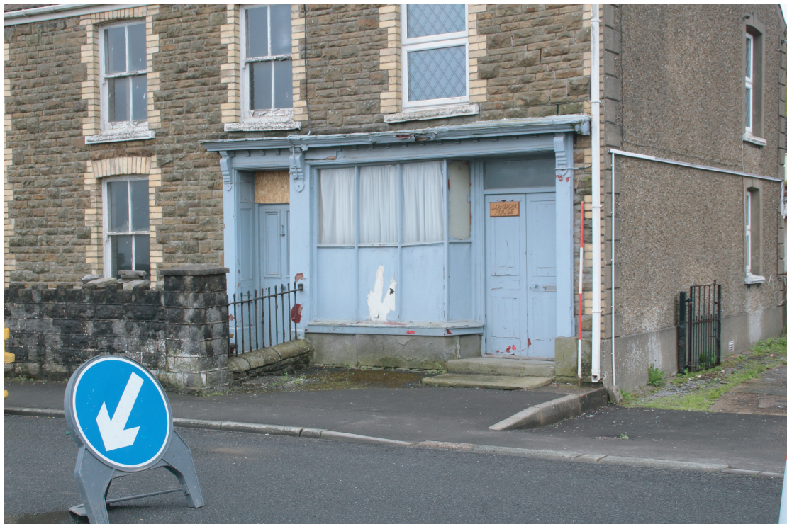
Plate 08. London House, Beach Road, Penclawdd. Early shopfront. Looking southeast.
