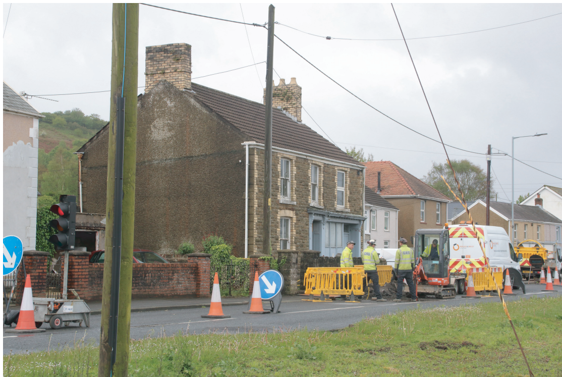
Plate 02. London House, Beach Road, Penclawdd. Looking southwest.
