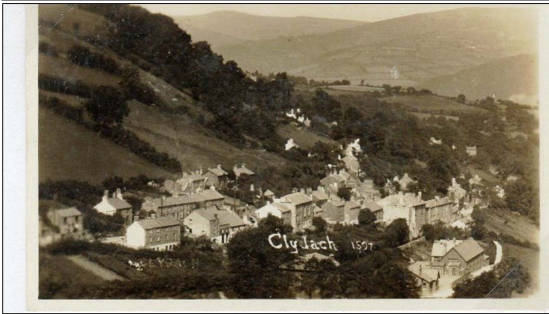
Fig. 6 Clydach North viewed from the south-east in 1897 (the primary school and infant school are visible in the bottom right hand corner)
