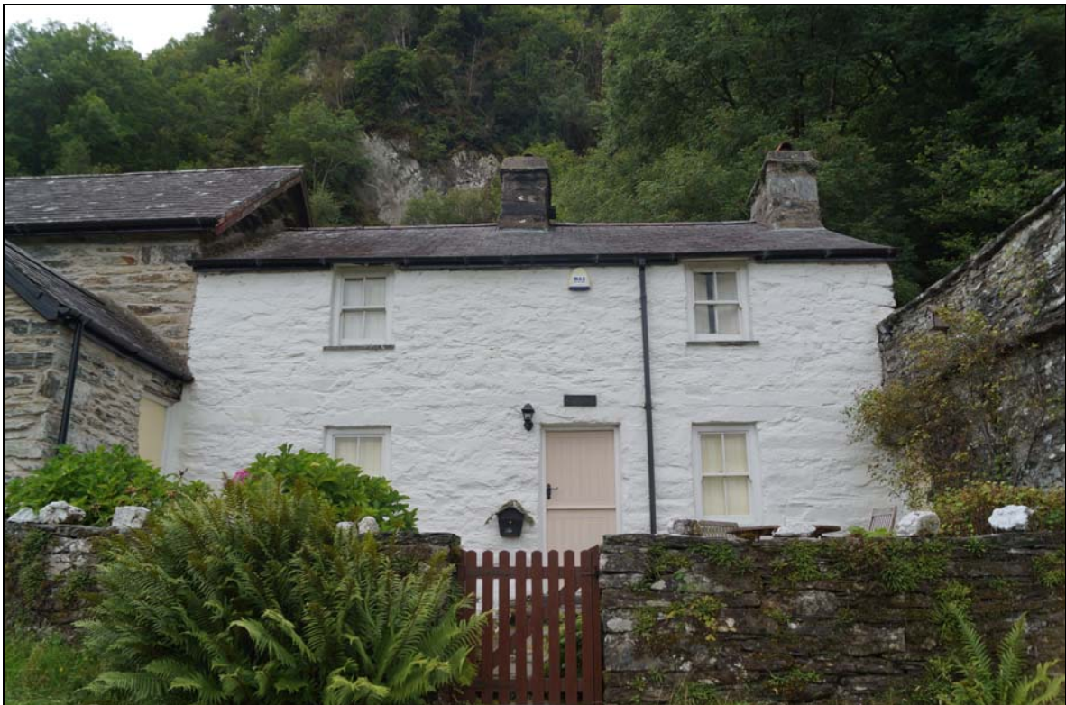
Plate 6: TYC2016_106 – Cyfyng cottage, ID number 9, looking west. It was once two cottages, with the lintel of a blocked up doorway still visible at the extreme left hand side of the front elevation.
