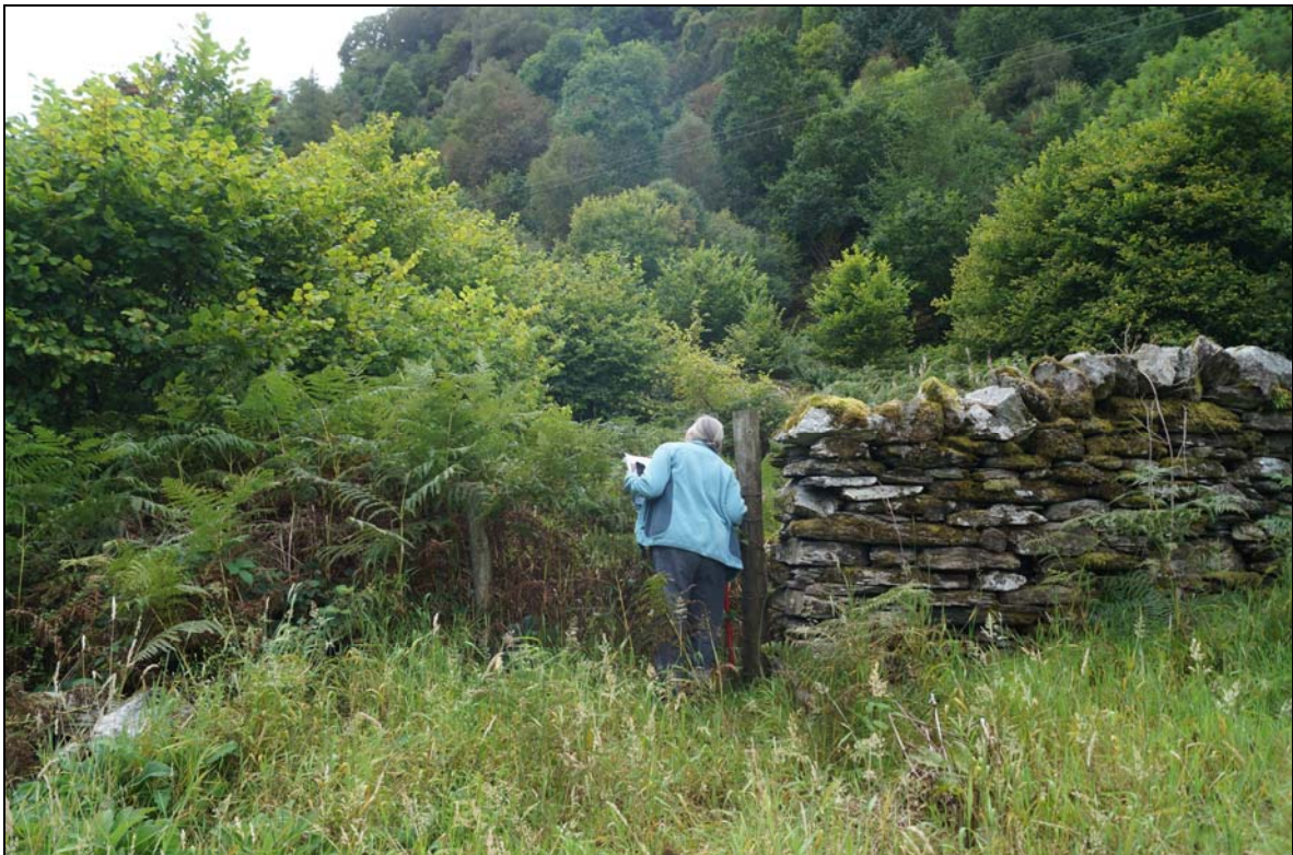
Plate 10: TYC2016_112 – the pipeline would pass through this former gateway through Wall ID number 2, looking southwest. Note the density of the scrub beyond the wall, in a field which would have been pasture a century ago.
