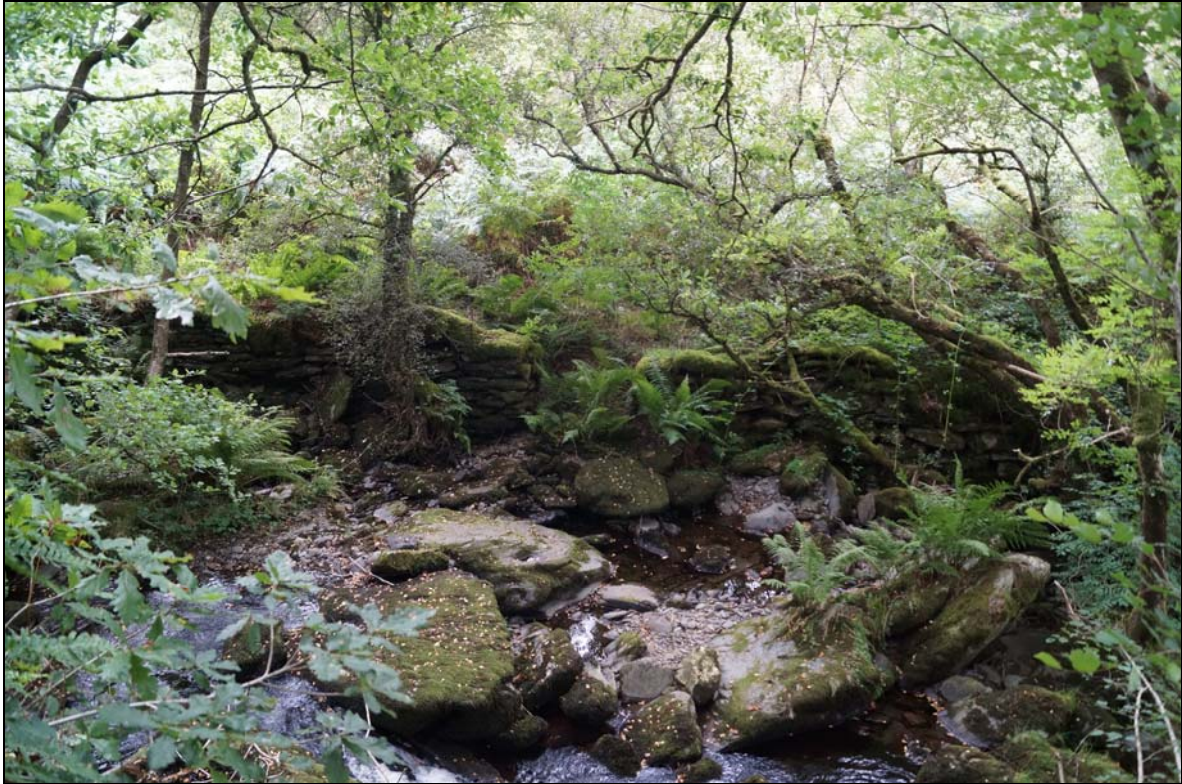
Plate 13: TYC2016_115 – the western riverbank below the proposed site of the intake tank has been revetted (ID number 6). This revetment may be a continuation of Wall Id number 5.
