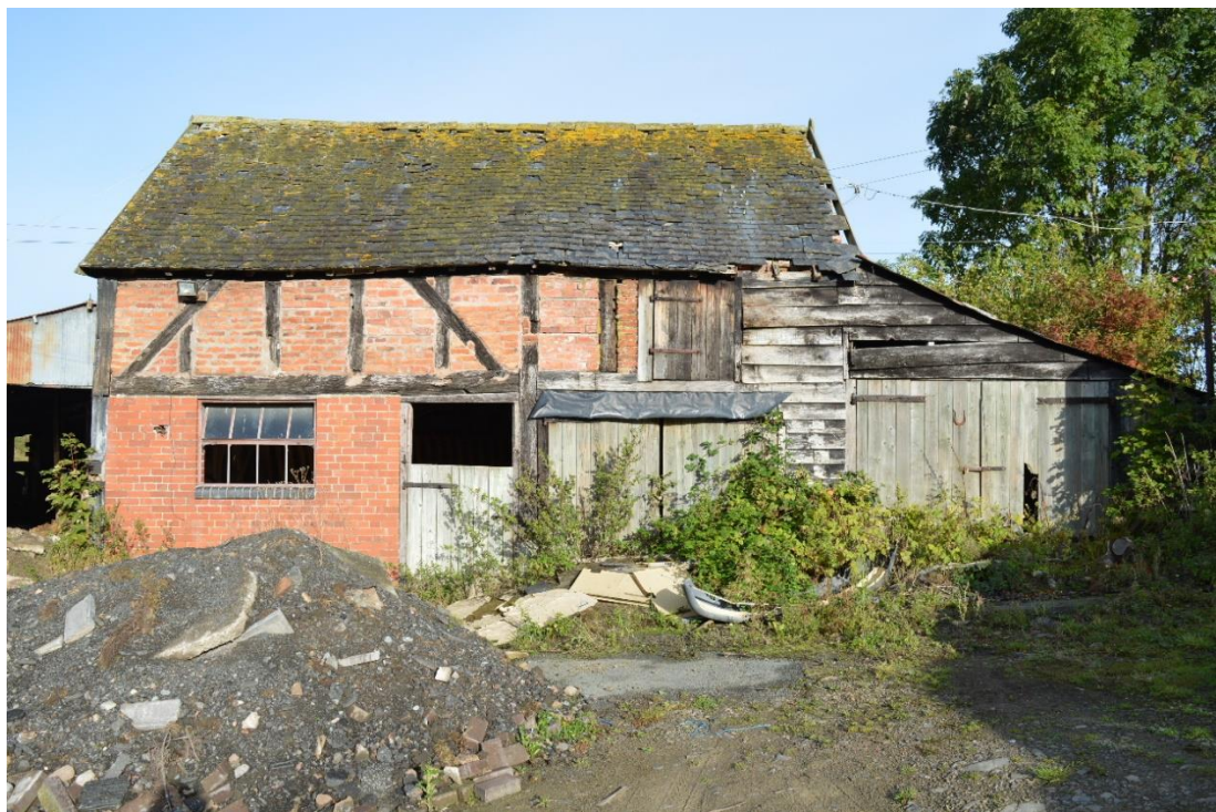
Fig. 7 Building B viewed from the south-east. Photo CPAT 4697-0001
