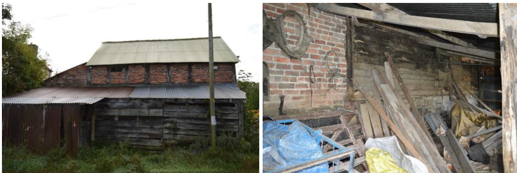
Fig. 11 Building B, north-west elevation. Photo CPAT 4697-0013 / 4697-0015
