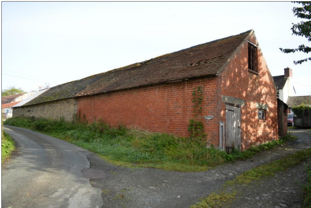
Fig. 4 Building A, south-west elevation. Photo CPAT 4697-0009
