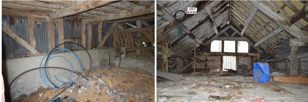
Fig. 8 Building B, south-west internal elevations. Photo CPAT 4697-0053 / 4697-0057
