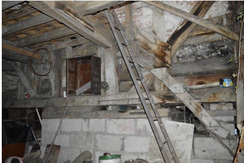
Fig. 10 Building B internal view of the north-east gable. Photo CPAT 4697-0066
