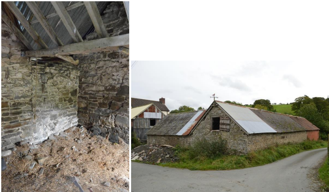
Fig. 6 Building A and the smaller stone building viewed from the north-west. Photo CPAT 4697-0048 and Building A internally showing the join in the stone work beside the north-west gable. Photo CPAT 4697-0028
