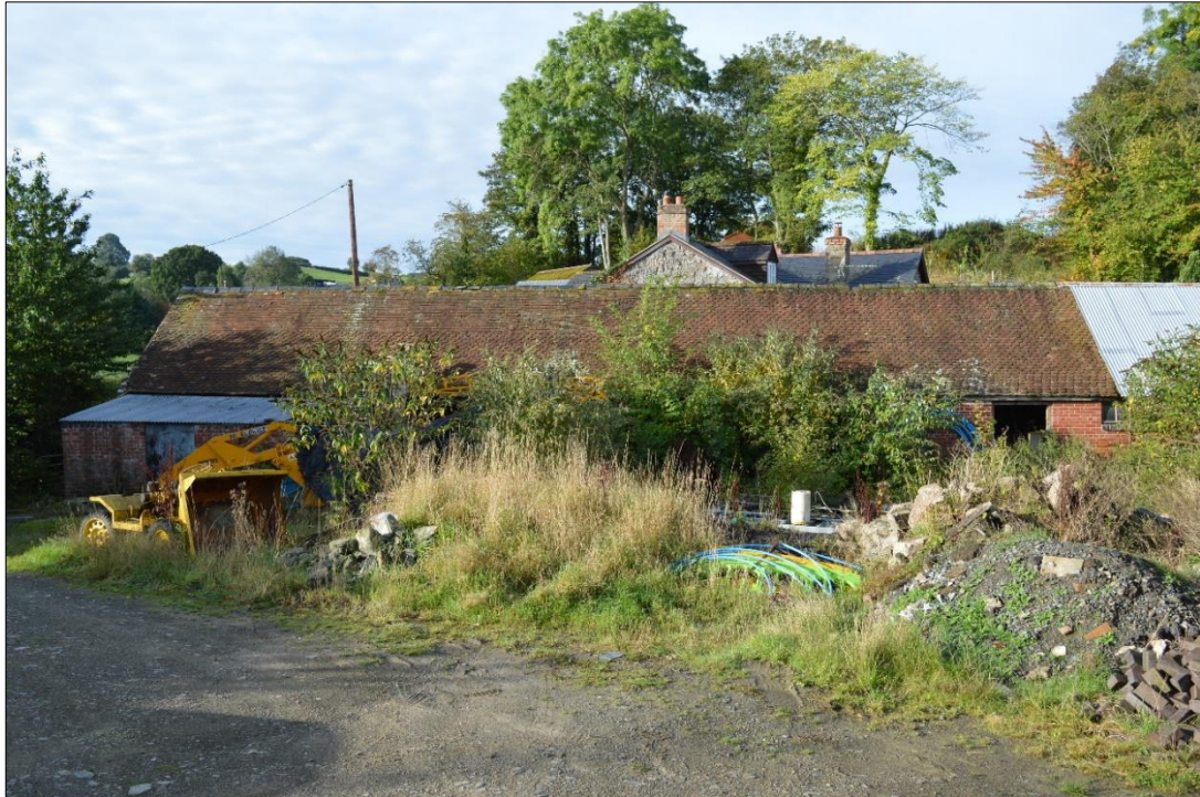
Fig. 5 Building A, viewed from the north-east. Photo CPAT 4697-0002
