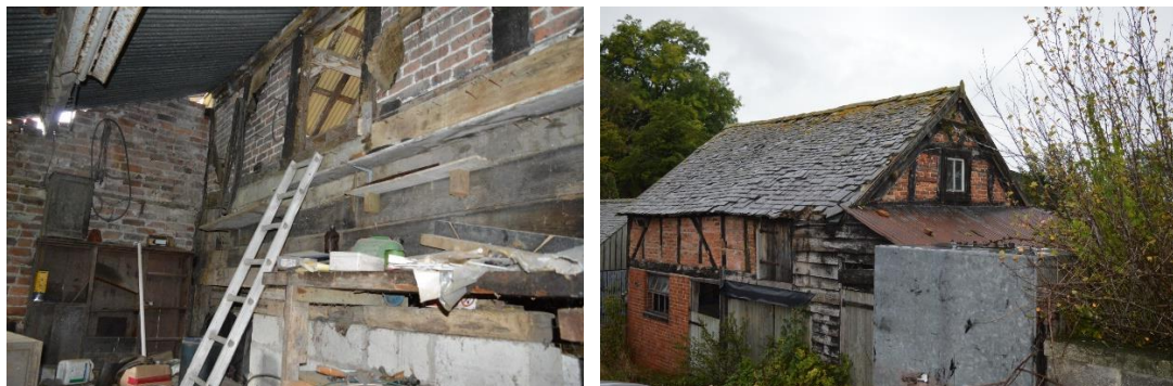
Fig. 9 Building B, north-east gable. Photo CPAT 4697-0055 / 4697-0067
