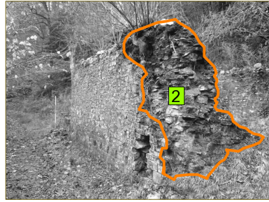
W44.05 North elevation - Exposed wall core and invasive roots to be removed and wall consolidated as clause C41/830
