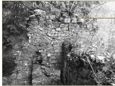
W44.05 North elevation - Evidence of dual pitched roofs Tree saplings to be removed as clause C41/127
