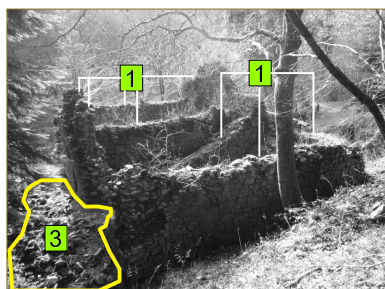
W44.04 West elevation - Exposed wall core at collapsed opening to be rough raked as clause C41/121
