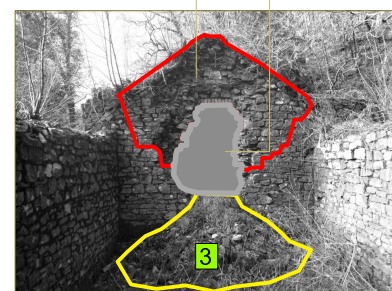
W44.02 North elevation - Unstable masonry to gable. Carefully dismantle, store and rebuild as clause C41/121. Collapsed material to be removed and stored as clause C41/140
