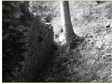
W44.04 West elevation - Close proximity of tree to wall. Tree clearance by others.
