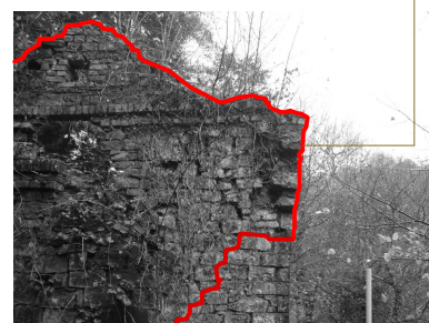
W44.02 South elevation - Displaced stonework to east end of wall
