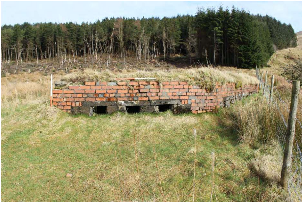
Plate 4: View north of Pill box installation NPRN115061
