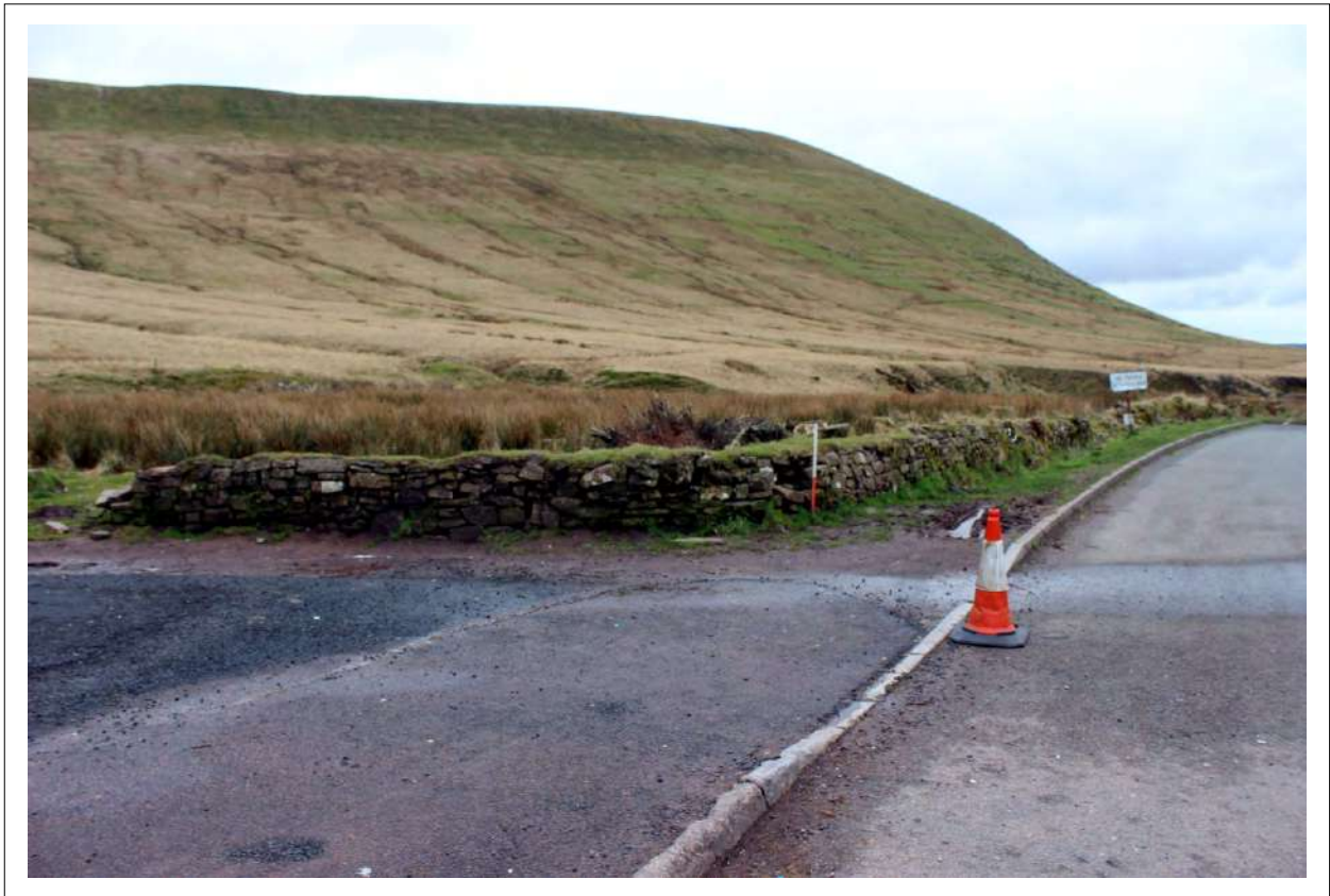
Plate 7: View south of wall NT860986
