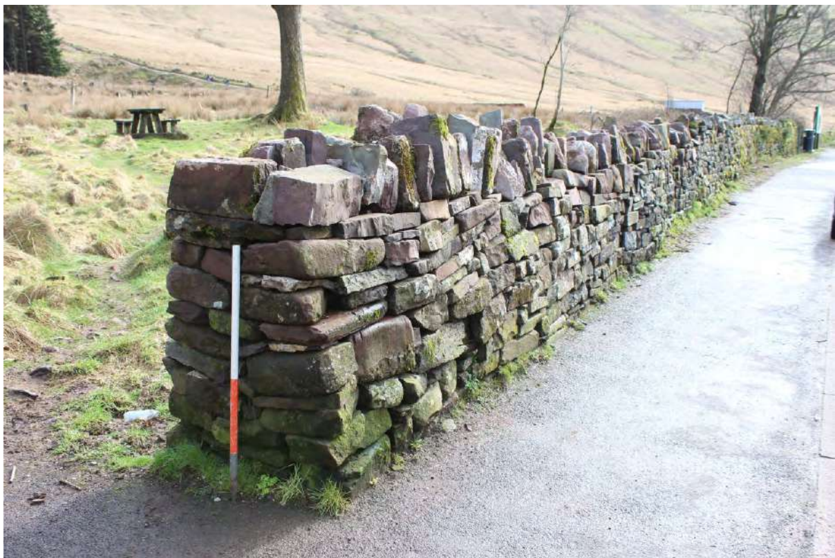
Plate 10: View south of wall NT860994
