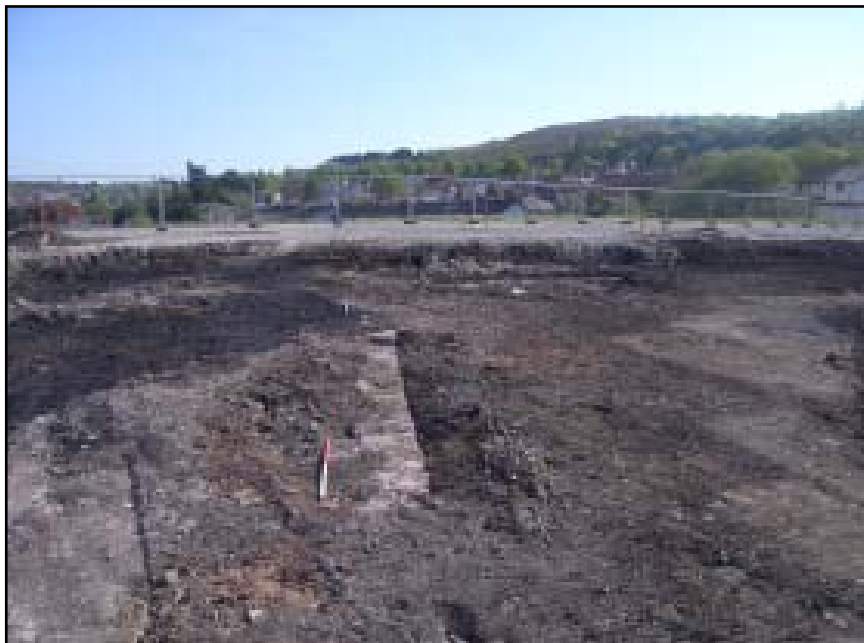
Plate 53 Looking south-east along the line of the eastern exterior wall of the rail mill, located beneath the former rugby club car park
