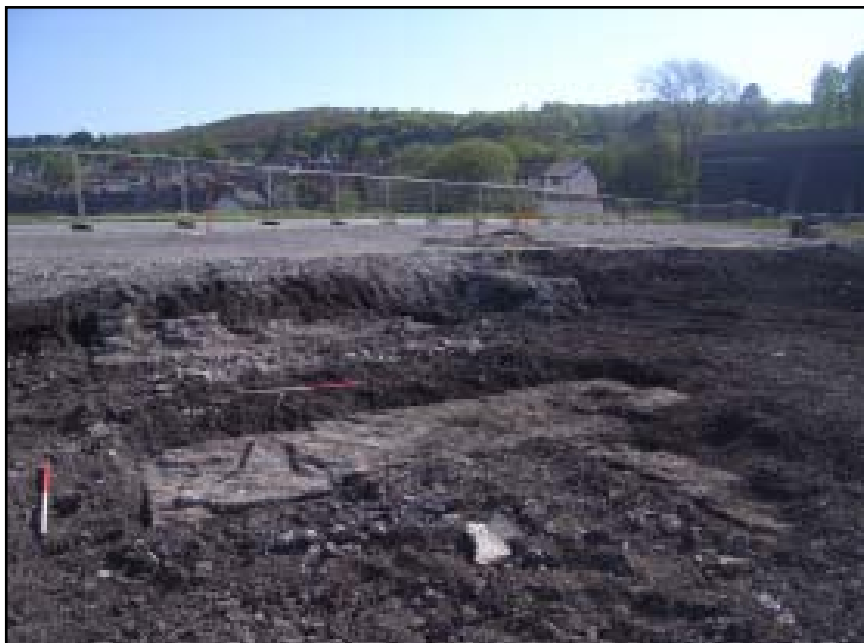
Plate 54 Two stone-built machine plinths, complete with cast iron holding down pins, located towards the south-east corner of the former rail mill, looking south-west
