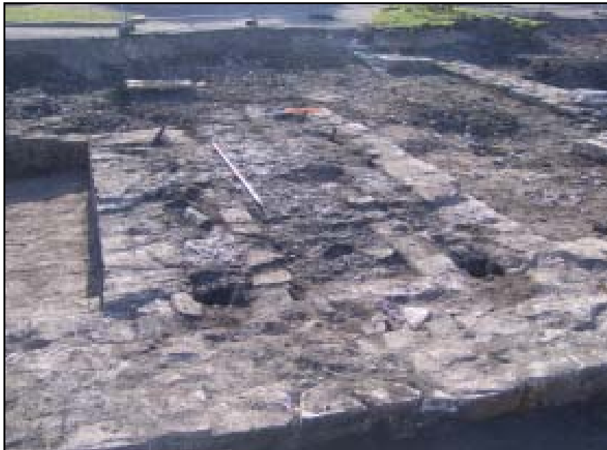
Plate 50 Looking south-west at the remains of the north end of the 'new mill' (Rail Mill). In the centre of the photograph is a massive structure, built using Pennant sandstone masonry, complete with seven integral cast iron holding down pins attached to which was a machine or machines used in the process of manufacturing iron rails
