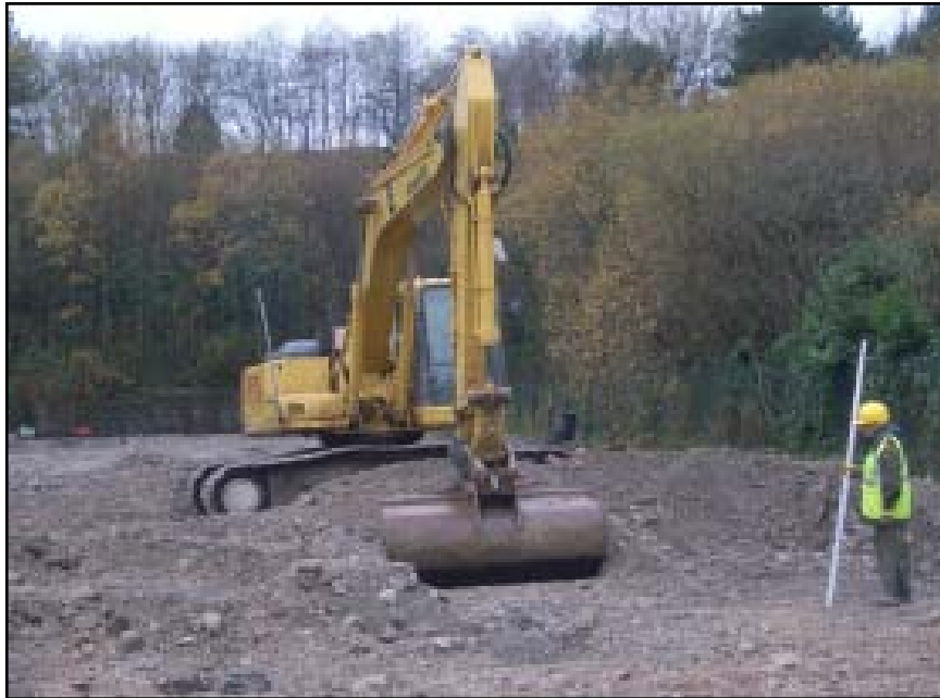
Plate 16 Initial excavation work in progress in late November 2006 – looking west
