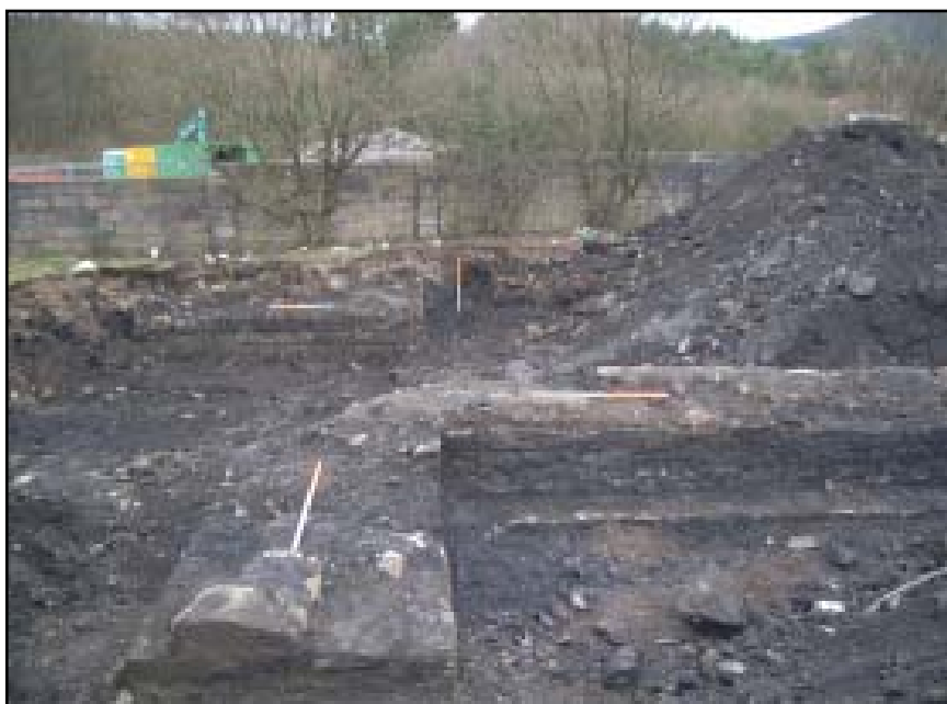
Plate 51 Looking north-west (the main excavation site was beyond the concrete block wall) at the remains of stone piers belonging to a railway bridge (see Figs. 12 – 14) that carried the G. W. R. line over a branch line leading to sidings
