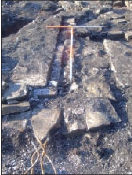
Plate 19 View north-west along the line of a 'flue-like' structure formed by walls 116 (left) and 114 (right) in 'new puddling' (forge). Note remnant of fire brick lining to left
