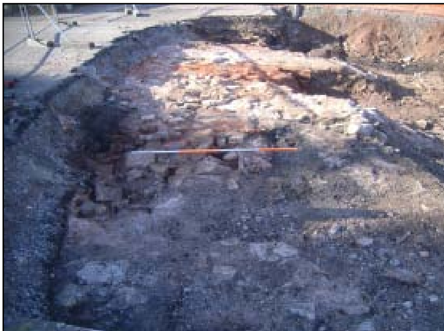
Plate 38 Looking west at the remains of the 'boilers' (Boiler House), showing three thermal halos caused by the intense heat generated by furnaces used to heat the boilers
