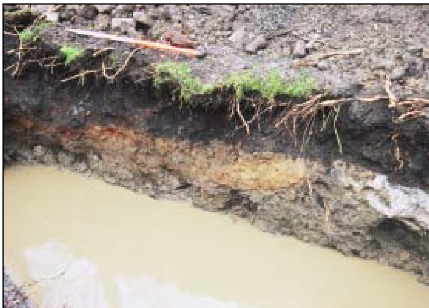
Plate 6 Trench 3, Casting House floor at western limit of trench
