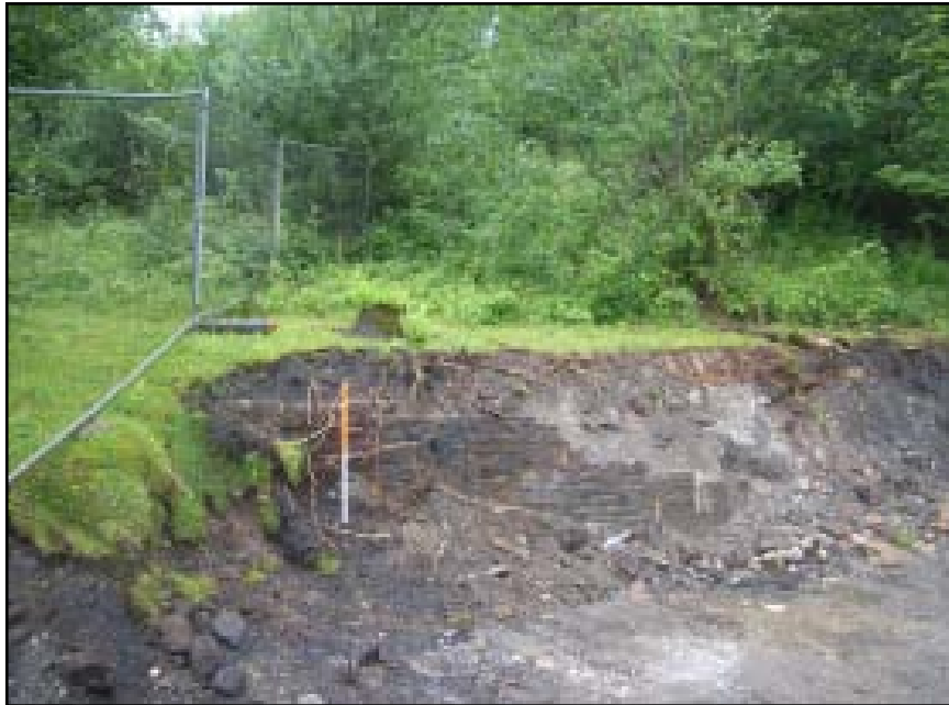
Plate 64 Looking north-west at part of the surviving east wall of Blast Furnace No. 3
