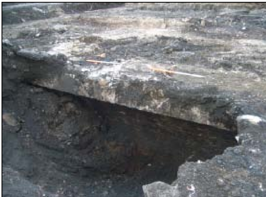
Plate 33 West-facing elevation of east wall (339) of N-S oriented tunnel located between 'boilers' (Boiler House) and 'new mill' (Rail Mill)
