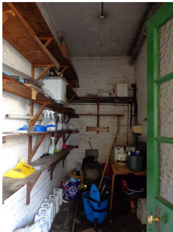
Plate 77: View of storing room (8), same than storing room (13); shot facing west.
