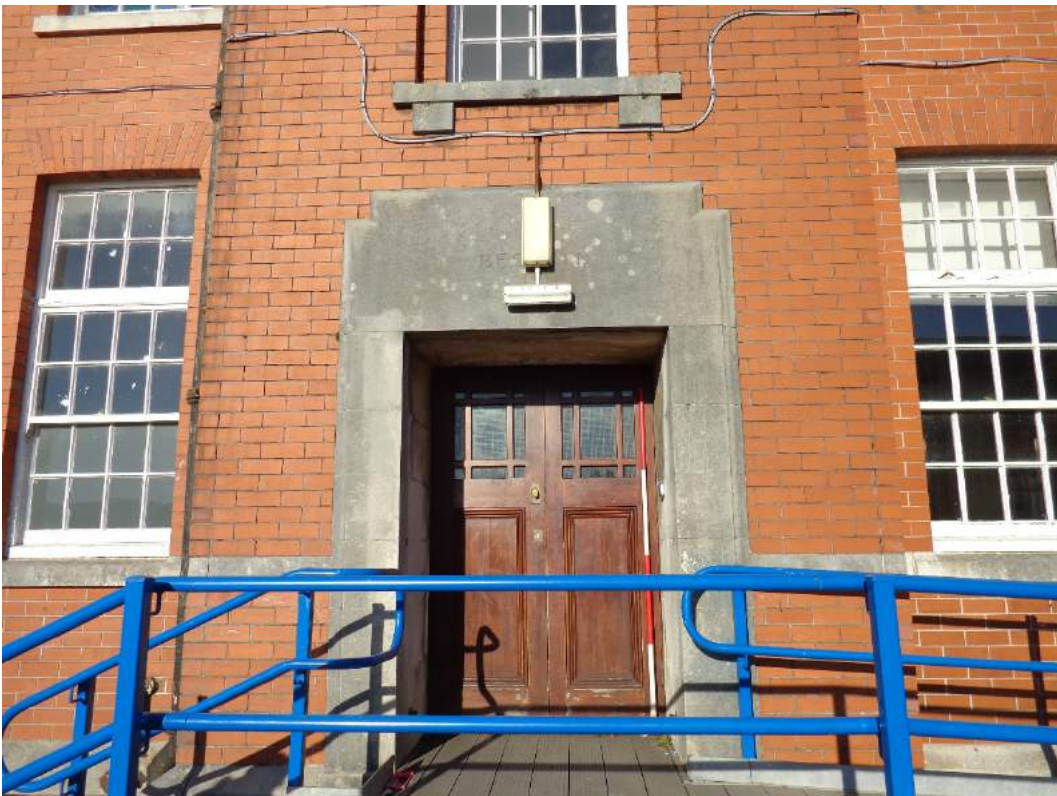
Plate 8: Boys S façade, view of western entry; shot facing north.
