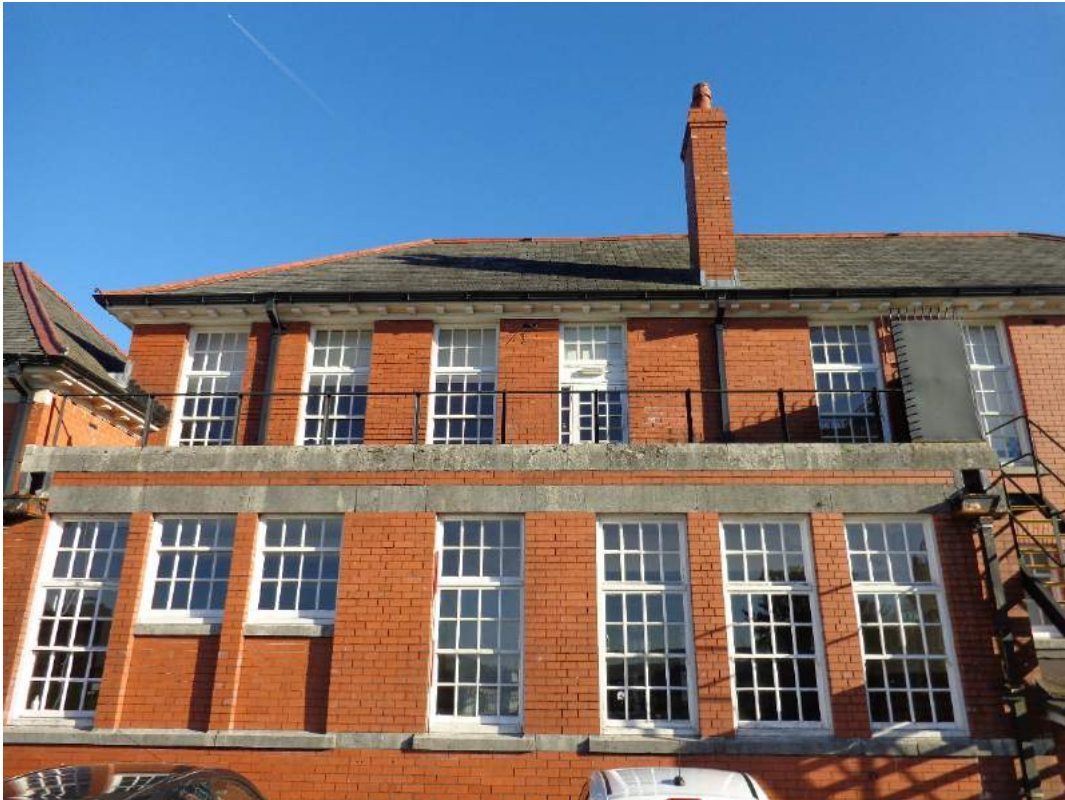
Plate 17: Back W façade, southern section; shot facing east.
