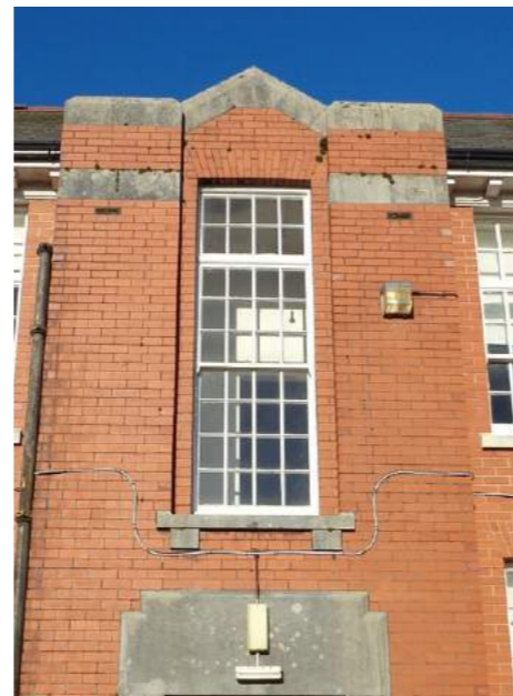
Window Type 8: 12-over-16-panel + 8-panel overhead
