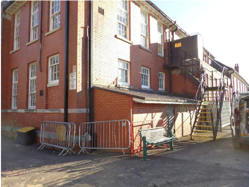
Plate 21: Back W façade, view of north-western corner; shot facing southeast.
