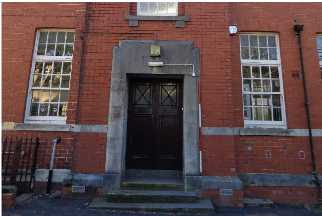
Plate 26: Girls N façade, view of eastern entry; shot facing south.
