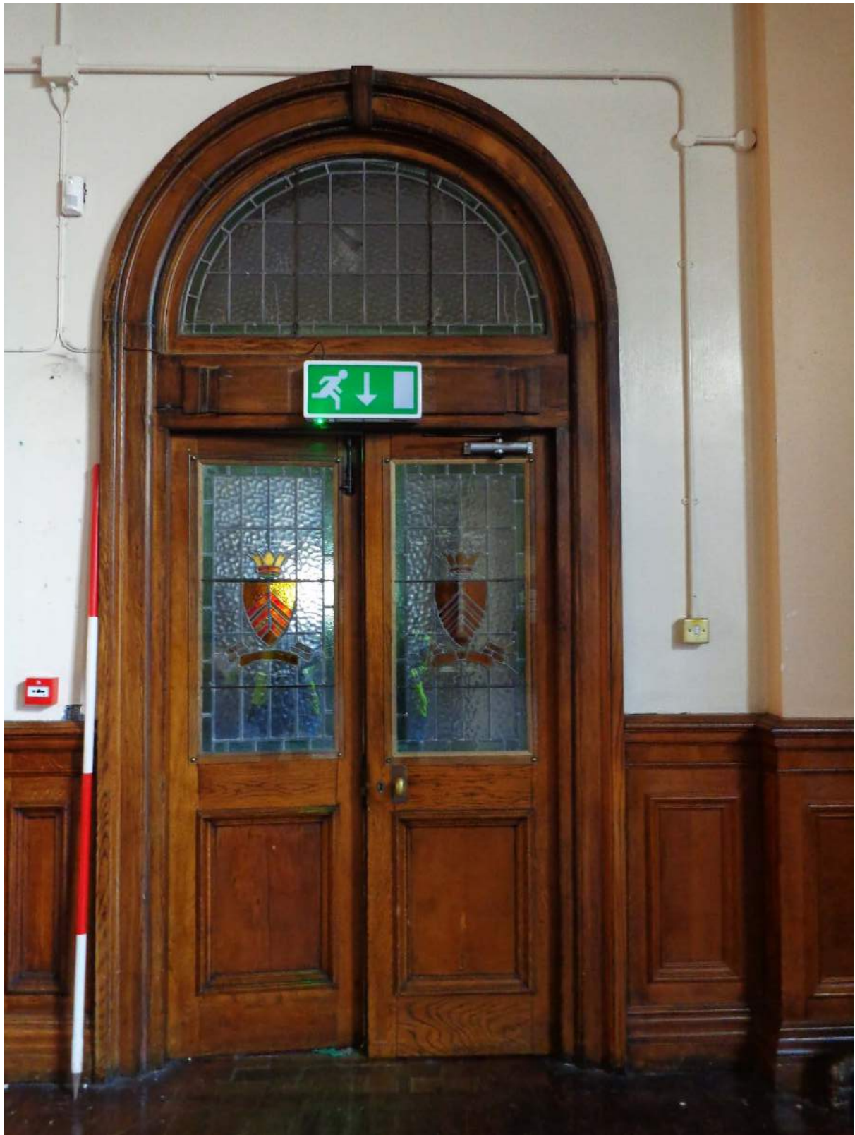
Plate 101: Drama Studio (33), detail of double gate entry from main entrance hall (29); shot facing east.
