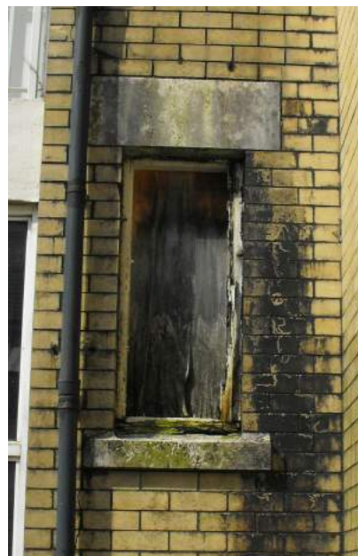
Window Type 7: single panel casement window
