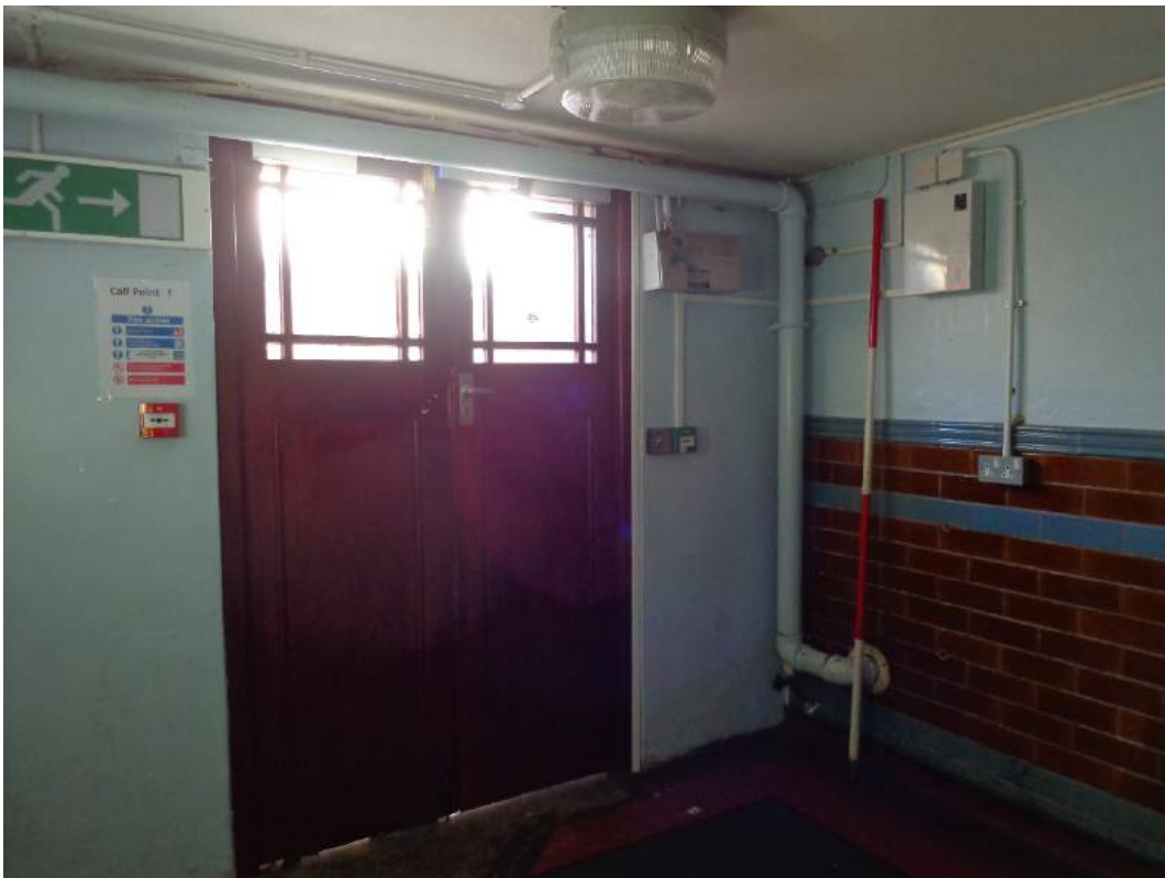
Plate 85: View of boys' eastern entry hall (101); shot facing southwest.
