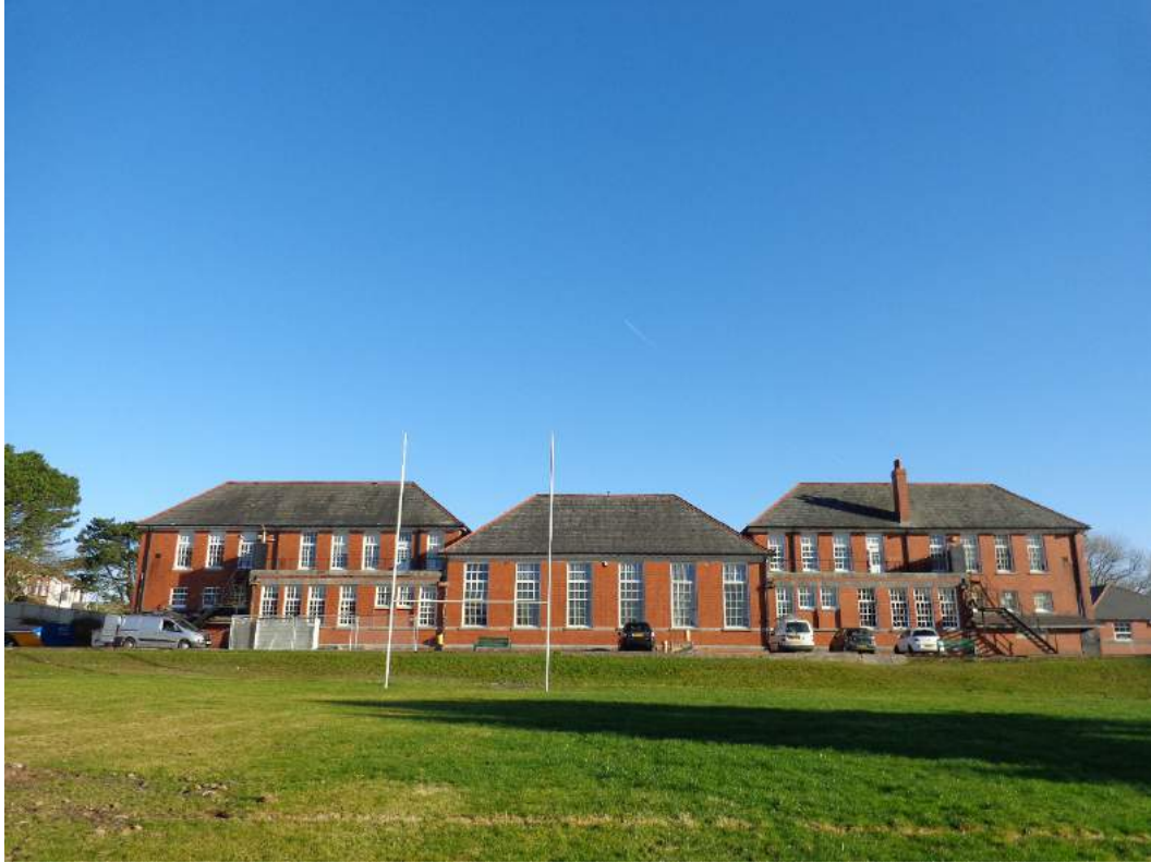
Plate 13: Back W façade, general view; shot facing east.
