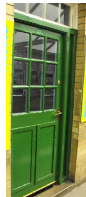
Door Type 10: wider single panel, glazed, lightover
