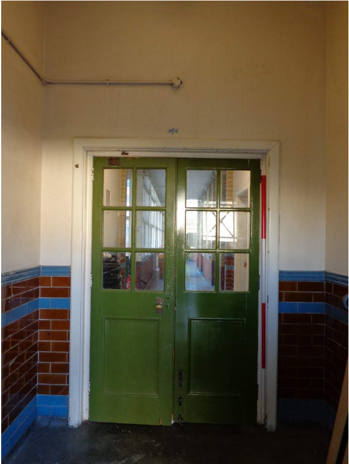
Plate 58: View of girls' western entry hall, lobby (85), and access to corridor (63) west; shot facing south.
