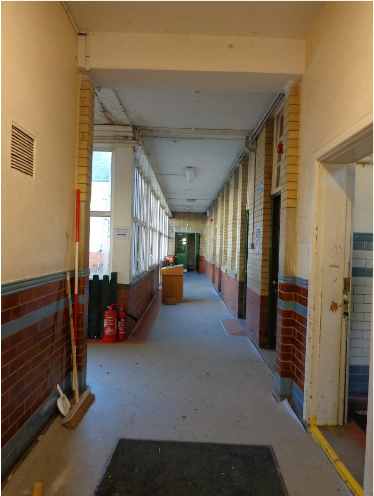
Plate 59: View of corridor (63) west, which gives access to (34), (13), (12), (11) and (10); also access to lobby (64) at the end; shot facing south.
