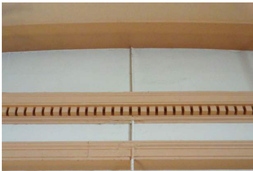
Plate 103: Drama Studio (33), detail of dentil decoration of roof cornice, same in all sides.
