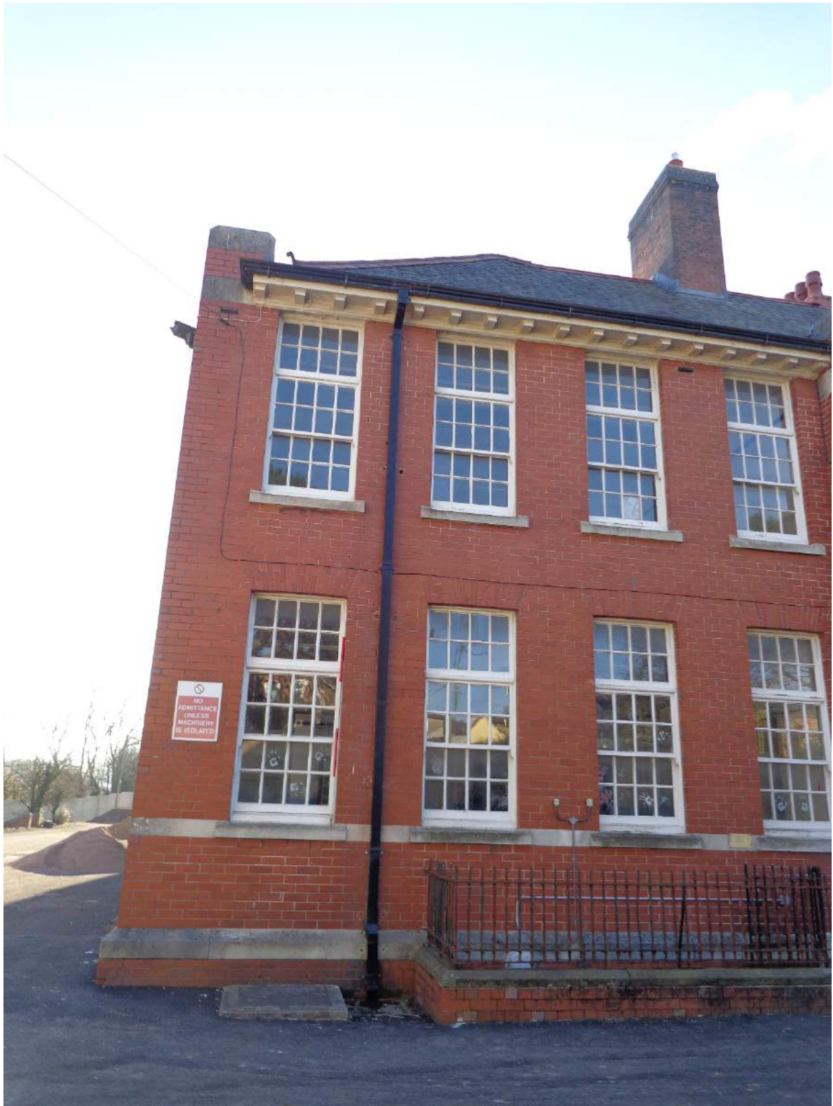
Plate 29: Girls N façade, view of eastern section; shot facing south.
