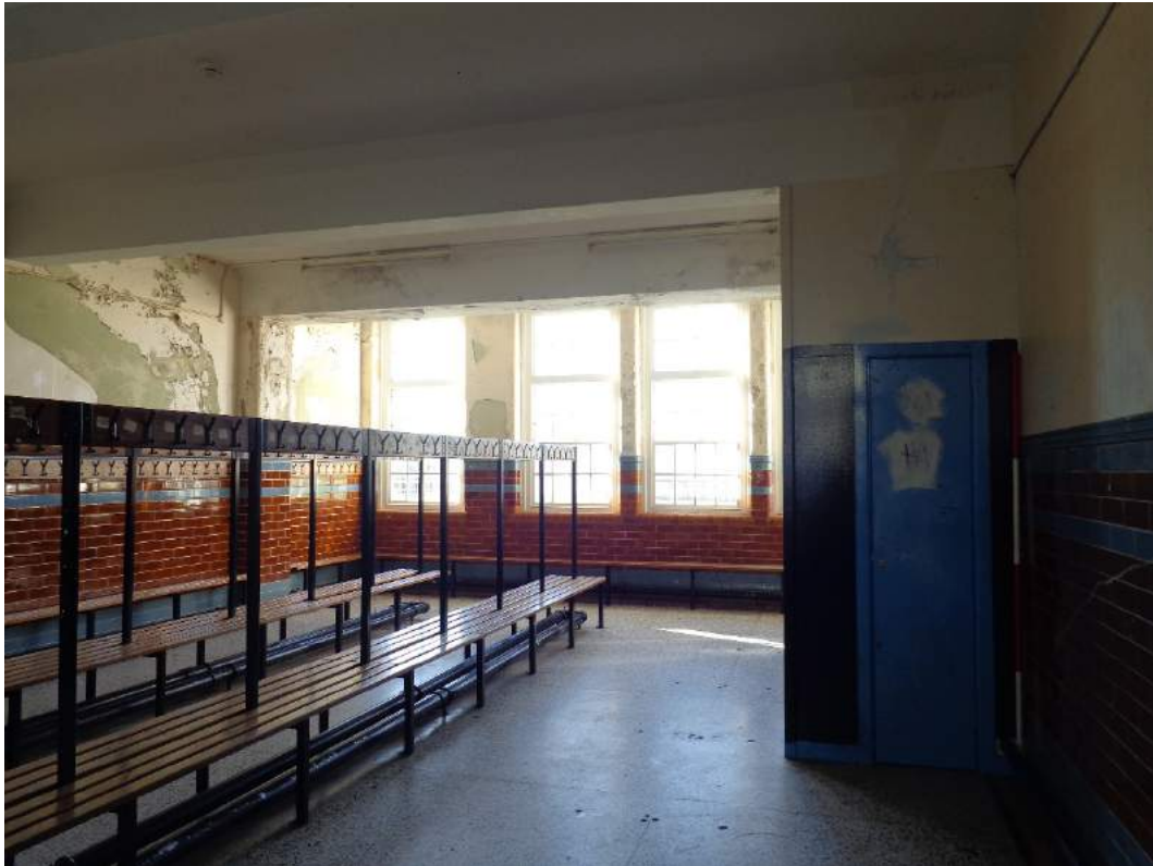
Plate 62: View of girls' changing room (12), with original tiling; shot facing west.
