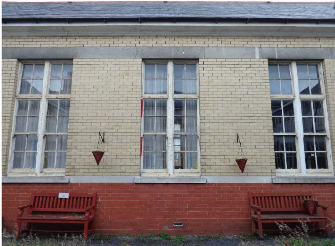
Plate 148: Courtyard 2, mid-section built of red and yellow brick and 6x4 panel windows; shot facing north.
