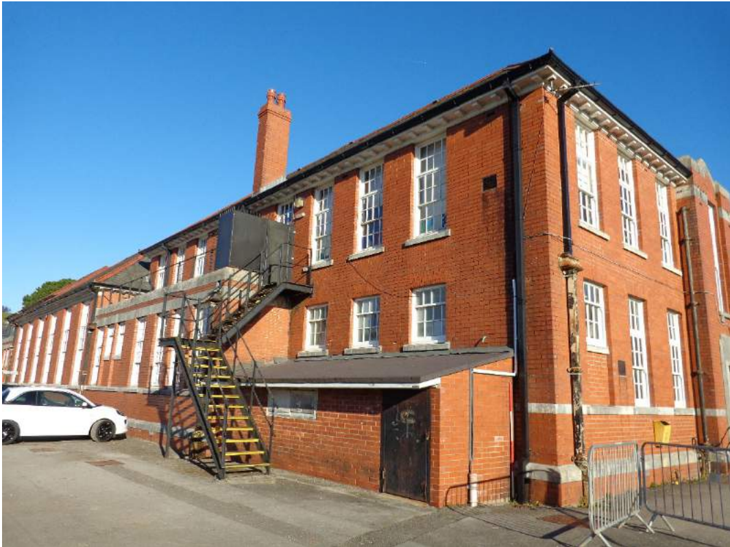
Plate 15: Back W façade, view of southwest corner; shot facing northeast.
