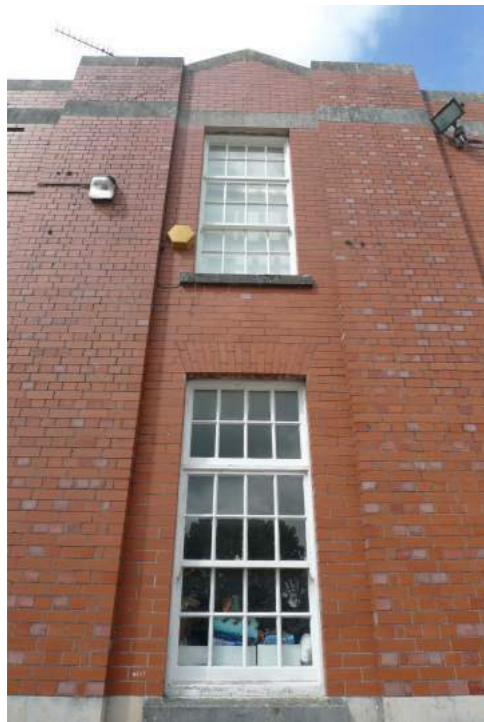
Window Type 1: 8-over-8-panel + 8-panel overhead
