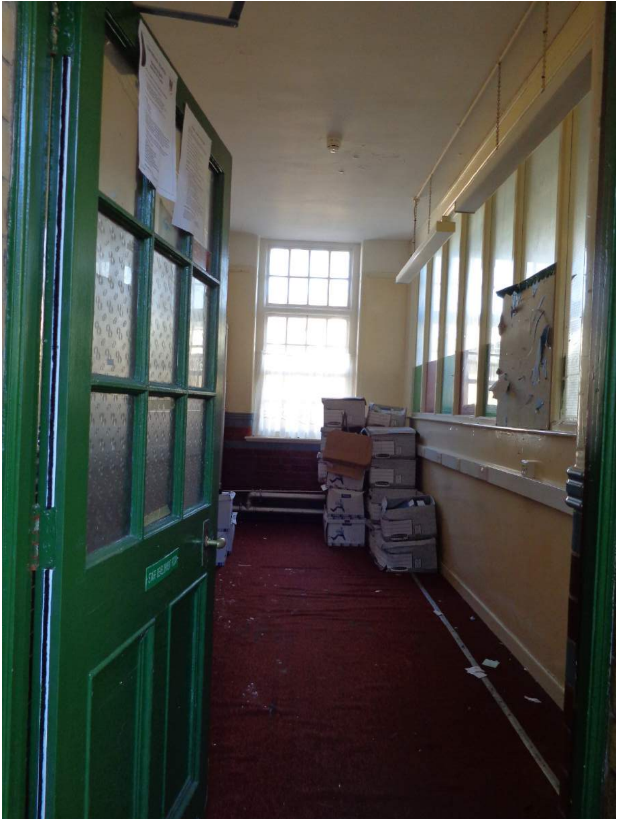
Plate 57: View of Staff Room (16), current canteen, with access to staff room (17); shot facing north.
