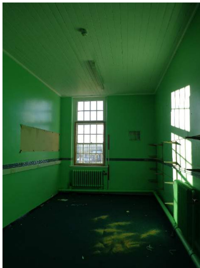
Plate 113: First Floor, view of Storage room 2 with original and new fittings; shot facing west.
