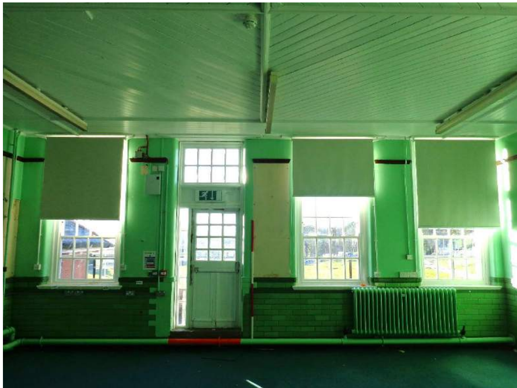
Plate 115: First Floor, view of Breakout area 1 with fitted door for fire exit; shot facing west.
