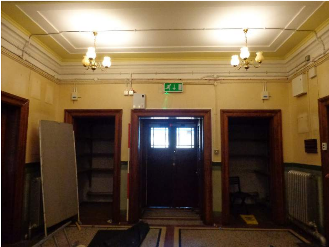
Plate 42: Main entrance hall (29), view of indoors; shot facing east.
