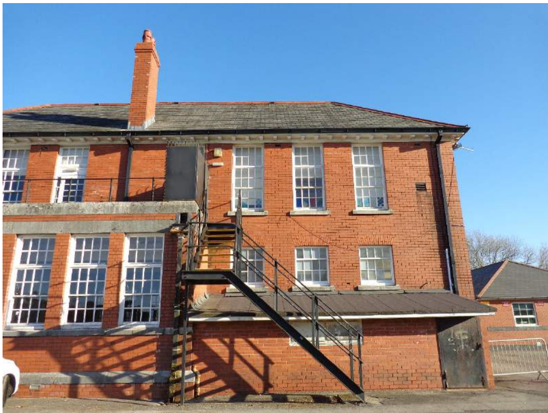
Plate 16: Back W façade, view of southern section; shot facing east.
