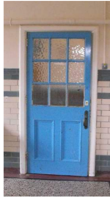
Door Type 4: single panel, glazed simple
