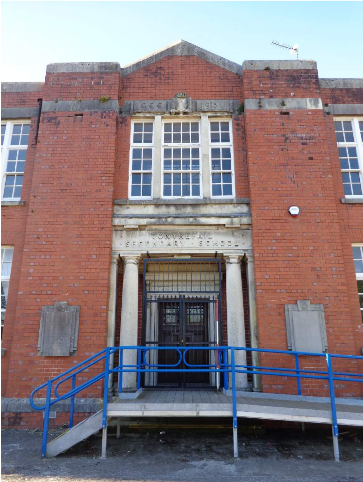
Plate 4: Frontal E façade, central area; shot facing west.
