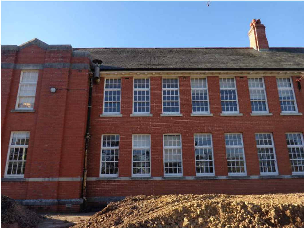
Plate 5: Frontal E façade, view of southern side; shot facing west.
