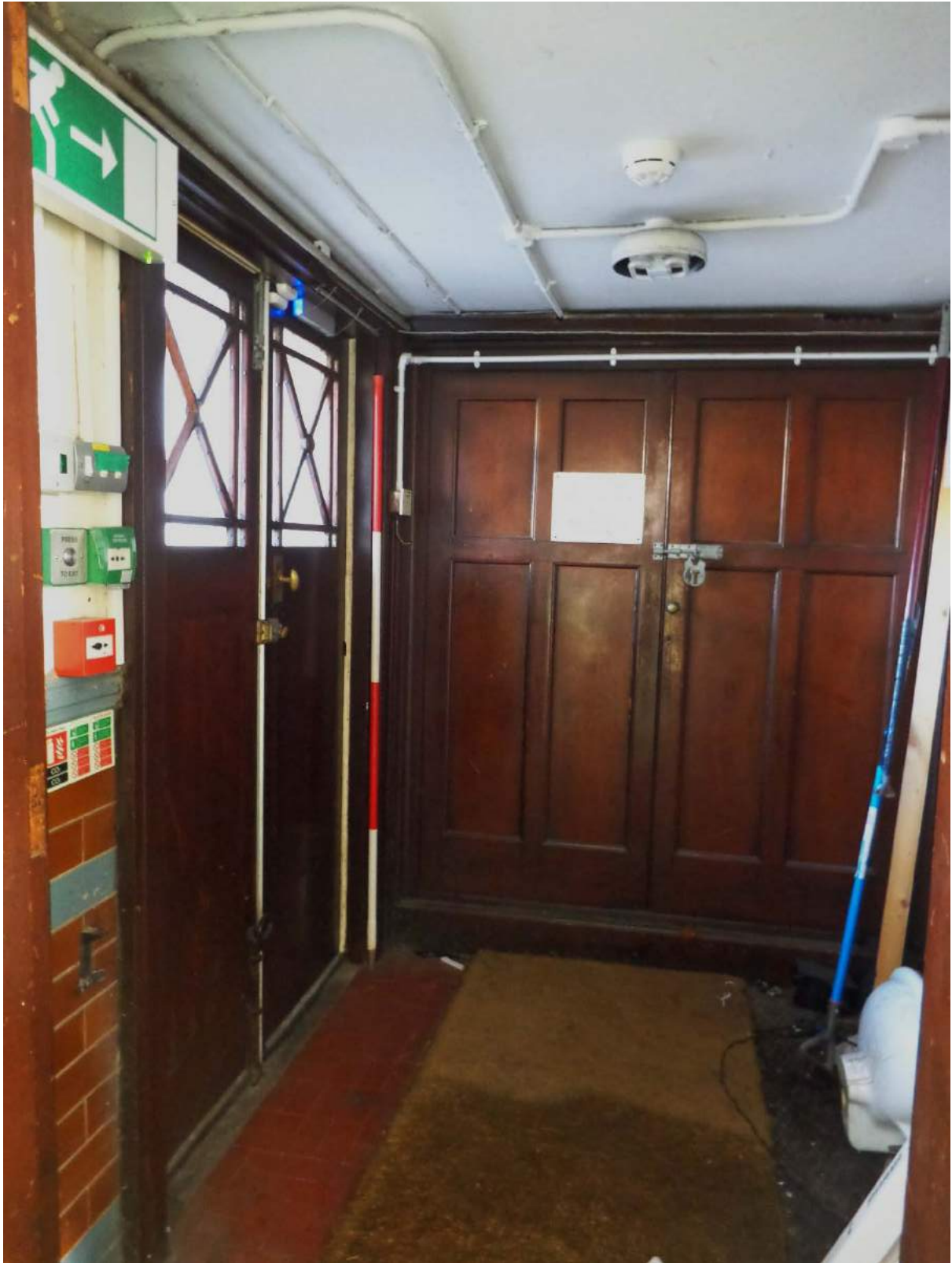
Plate 54: View of girls' eastern entry lobby (100), indoors; shot facing northeast.
