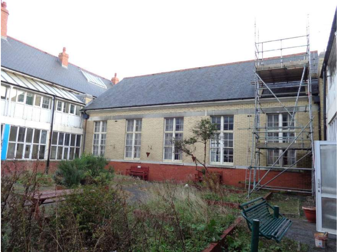
Plate 149: Courtyard 1, general view with scaffolding and overgrown shrubs; shot facing southeast.
