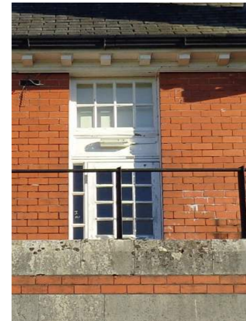
Type 9: former Type 1 window turned into a fire exit door
