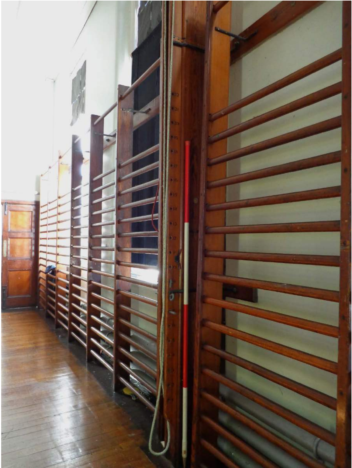
Plate 71: Detail of original fittings at the gymnasium (10); shot facing southeast.
