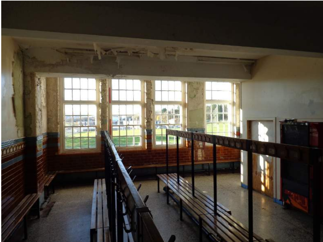
Plate 76: View of boys' changing room (9), with original fittings; shot facing west.
