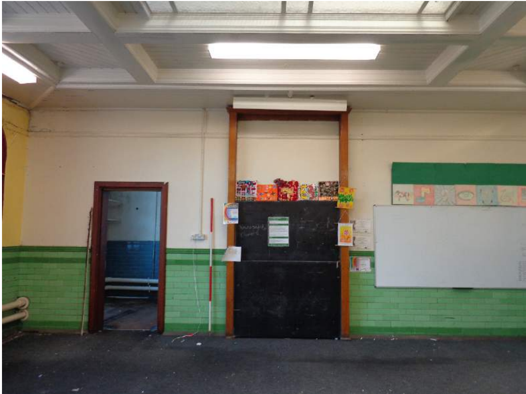
Plate 125: First Floor, Staff Work room with original fittings and access to Storage room 3; shot facing south.
