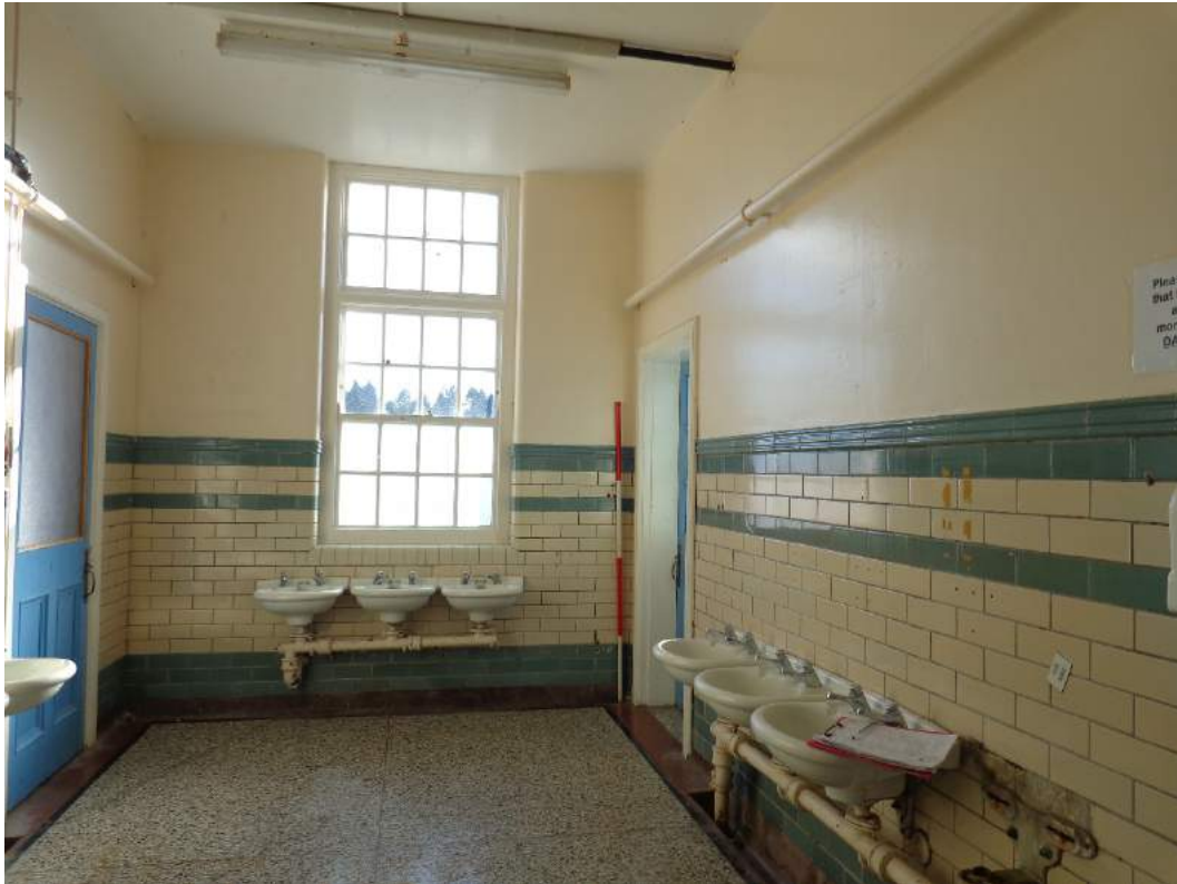
Plate 78: View of boys' WC lobby (7), with original fittings; shot facing south.
