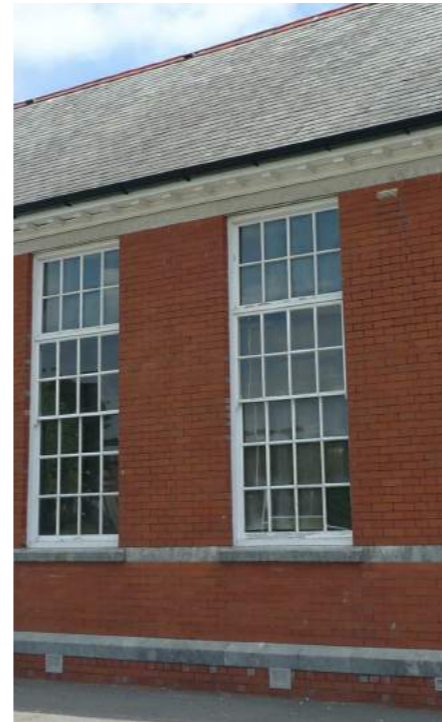
Window Type 3: 8-over-12-panel + 8-panel overhead
