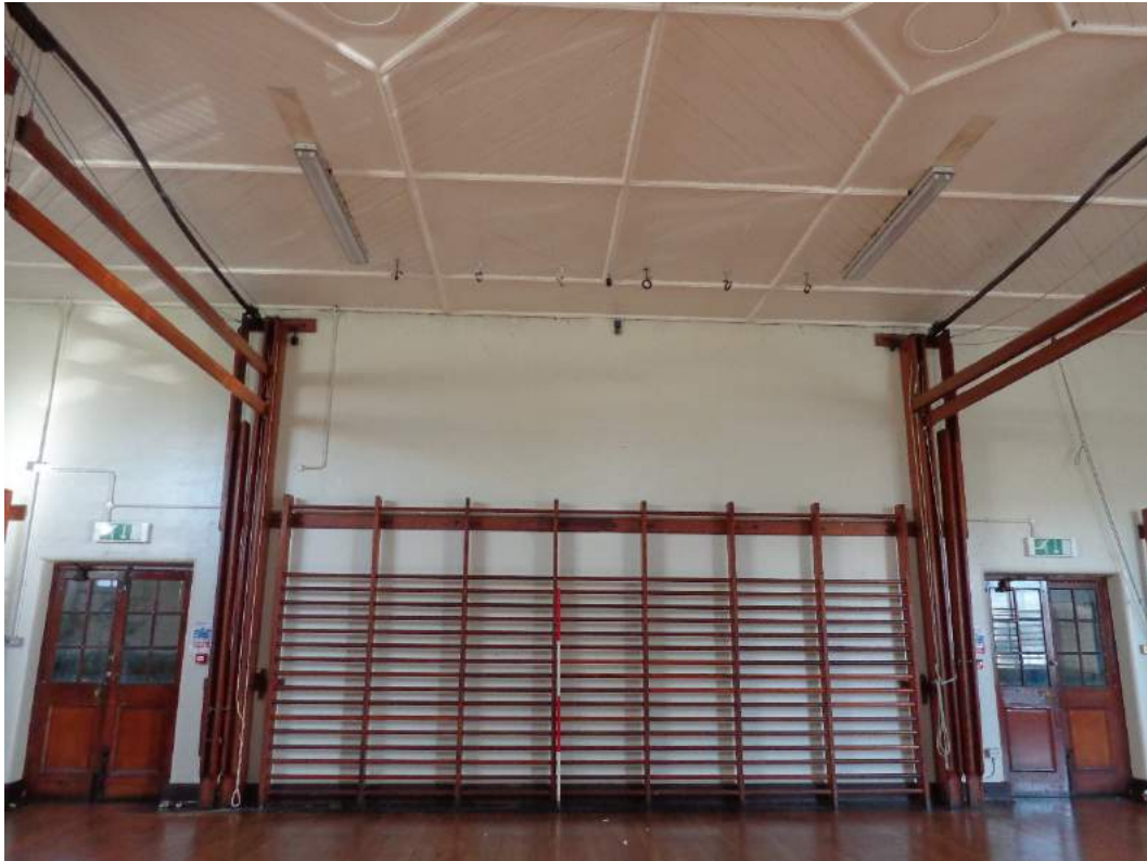
Plate 69: View of gymnasium (10) with original fittings and accesses to corridor (63) west; shot facing east.
