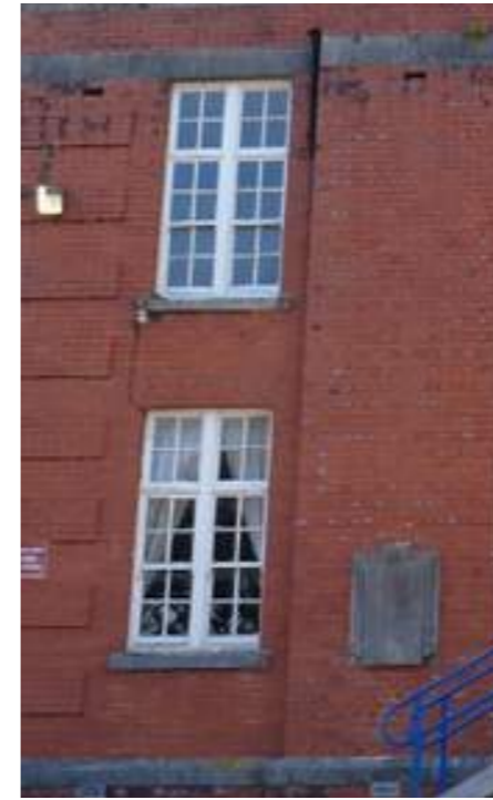
Window Type 4: double 4-over-4-panel + double 4-panel overhead
