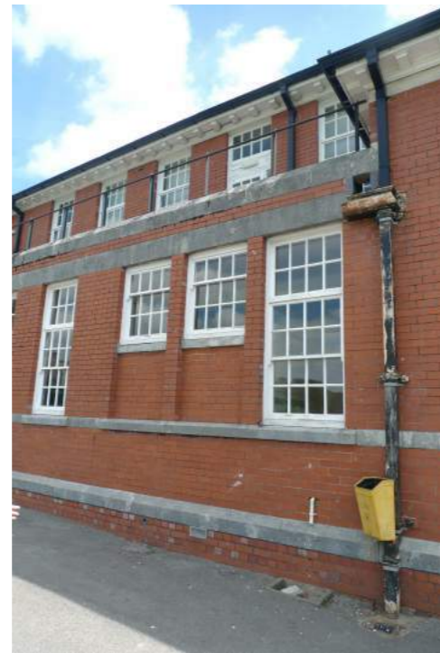
Window Type 2: 8-panel sash + 8-panel overhead
