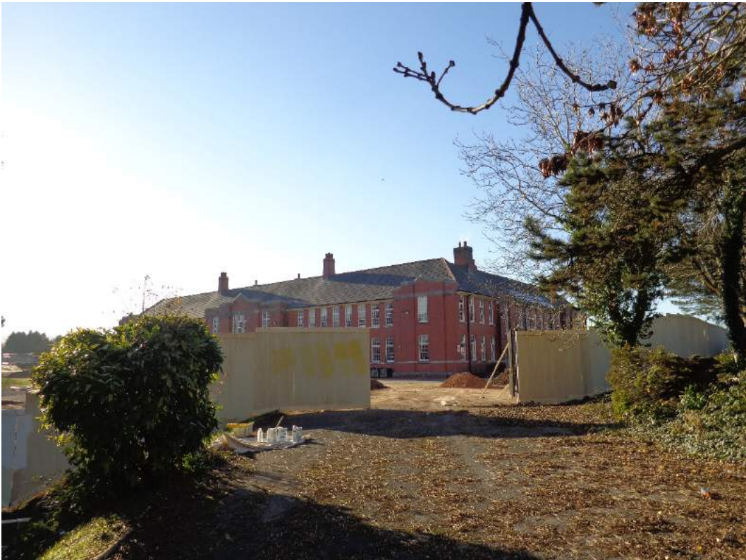
Plate 160: View of northeast gate area towards the street and wooden fencing; shot facing southwest.
