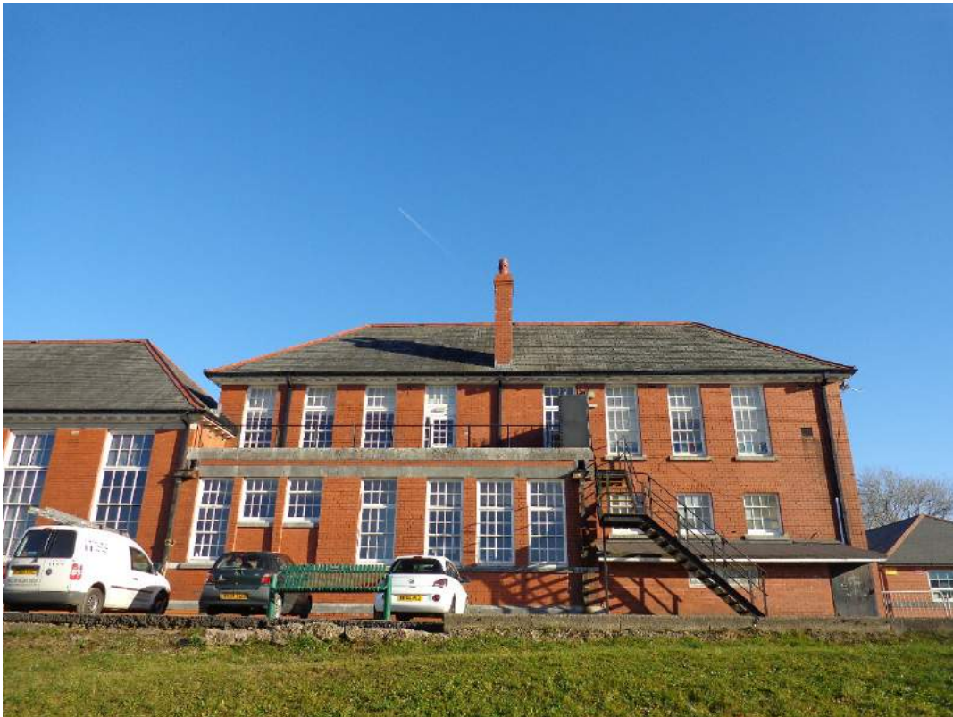
Plate 14: Back W façade, view of southern section; shot facing east.
