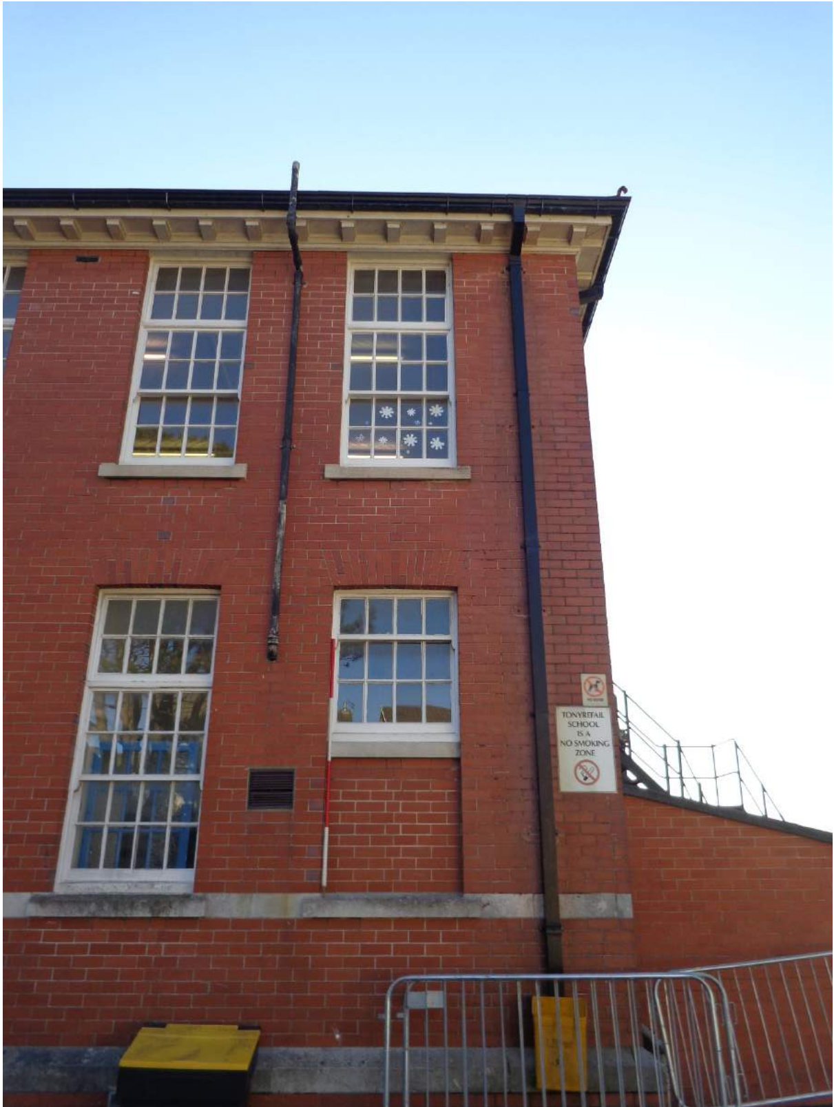
Plate 23: Girls N façade, view of western section; shot facing south.
