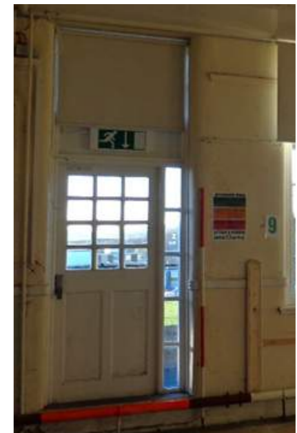
Type 9: former Type 1 window turned into a fire exit door
