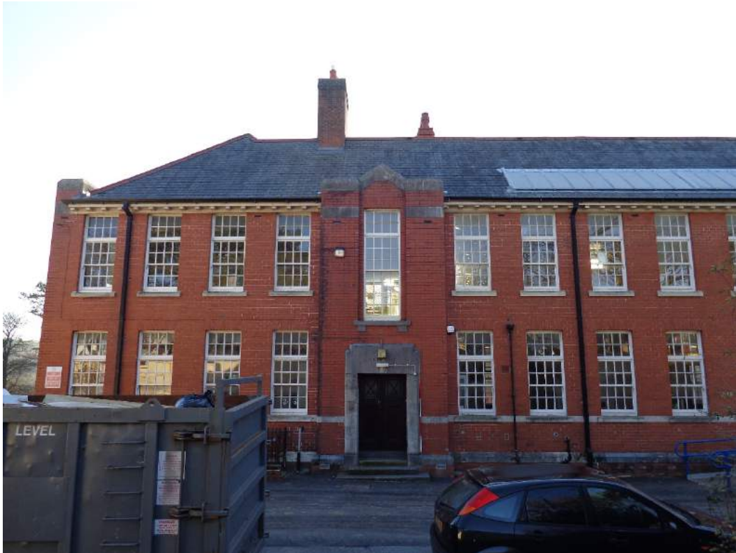
Plate 25: Girls N façade, eastern section and entry; shot facing south.
