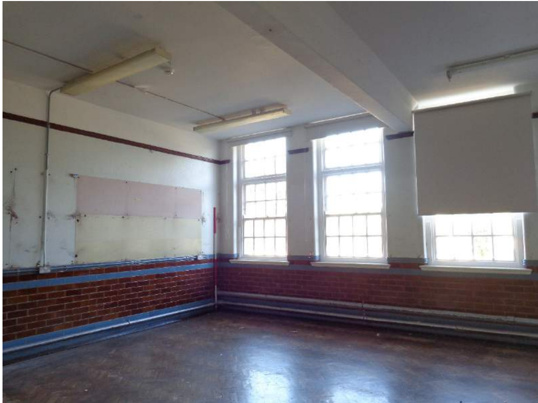
Plate 90: View of Seminar Room (1) with original fittings; shot facing northeast.
