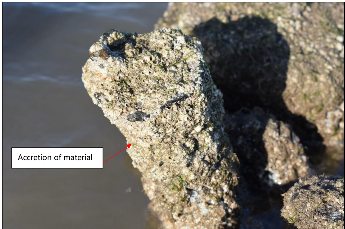
Fig. 7 Accretion materials of timber. Photo CPAT 4674-0023
