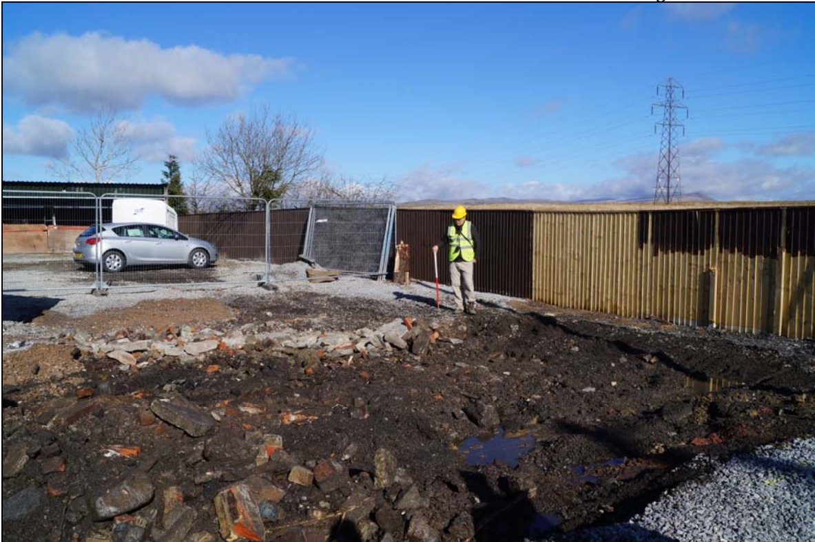
Plate 2: GVB2016_102, during removal of building rubble, 001, looking north northwest.
