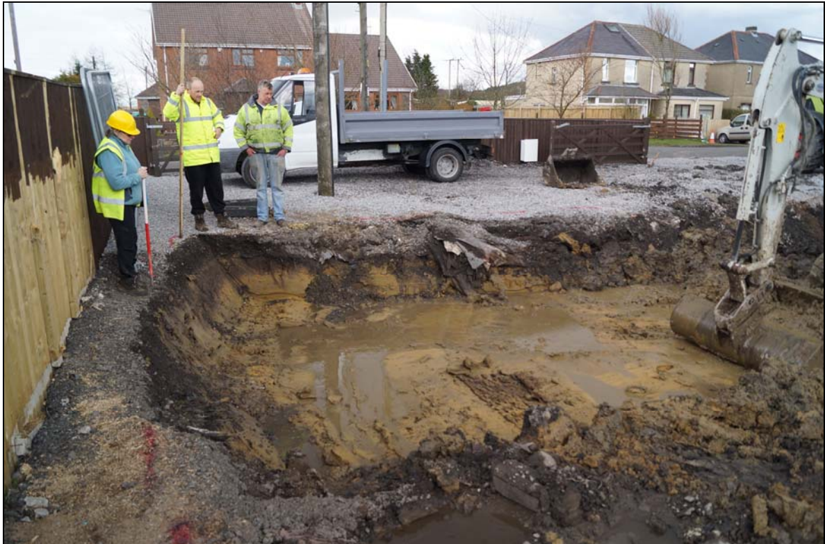
Plate 6: GVB2016_106, Building rubble removed and clay 002 and 003 visible in base, groundwater seeping in fast, looking southeast.
