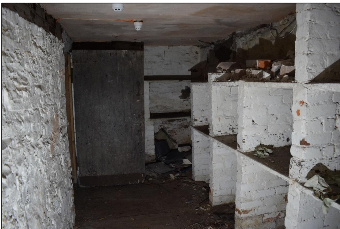
Fig. 45: Eastern of the three adjoining cellar rooms (Fig. 10, B6). CPAT 4537-0159
