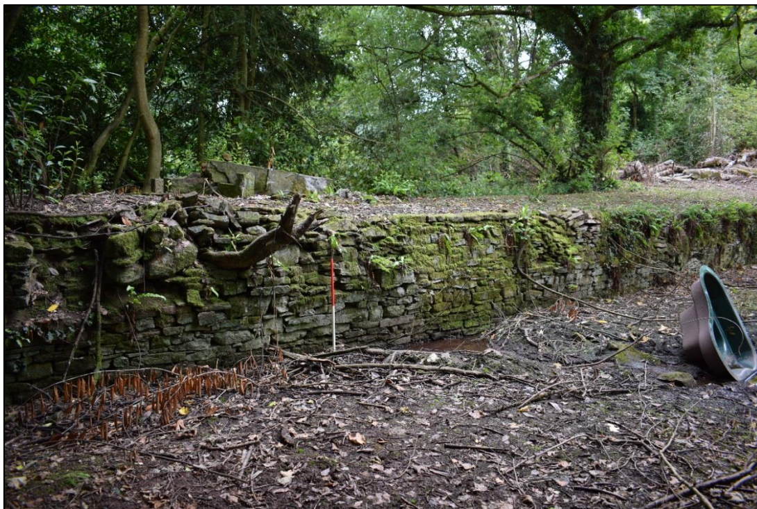
Fig. 52: The causeway/dam for the ornamental pond to the east of the hall. CPAT 4537-0019
