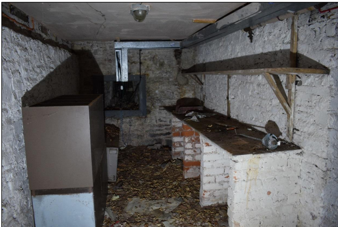
Fig. 44: Central of the three adjoining cellar rooms (Fig. 10, B5). CPAT 4537-0157
