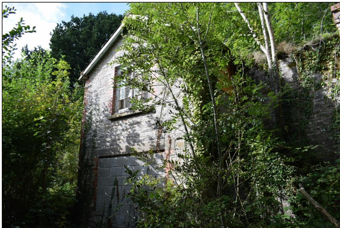
Fig. 50: The gardener's cottage. CPAT 4537-0163
