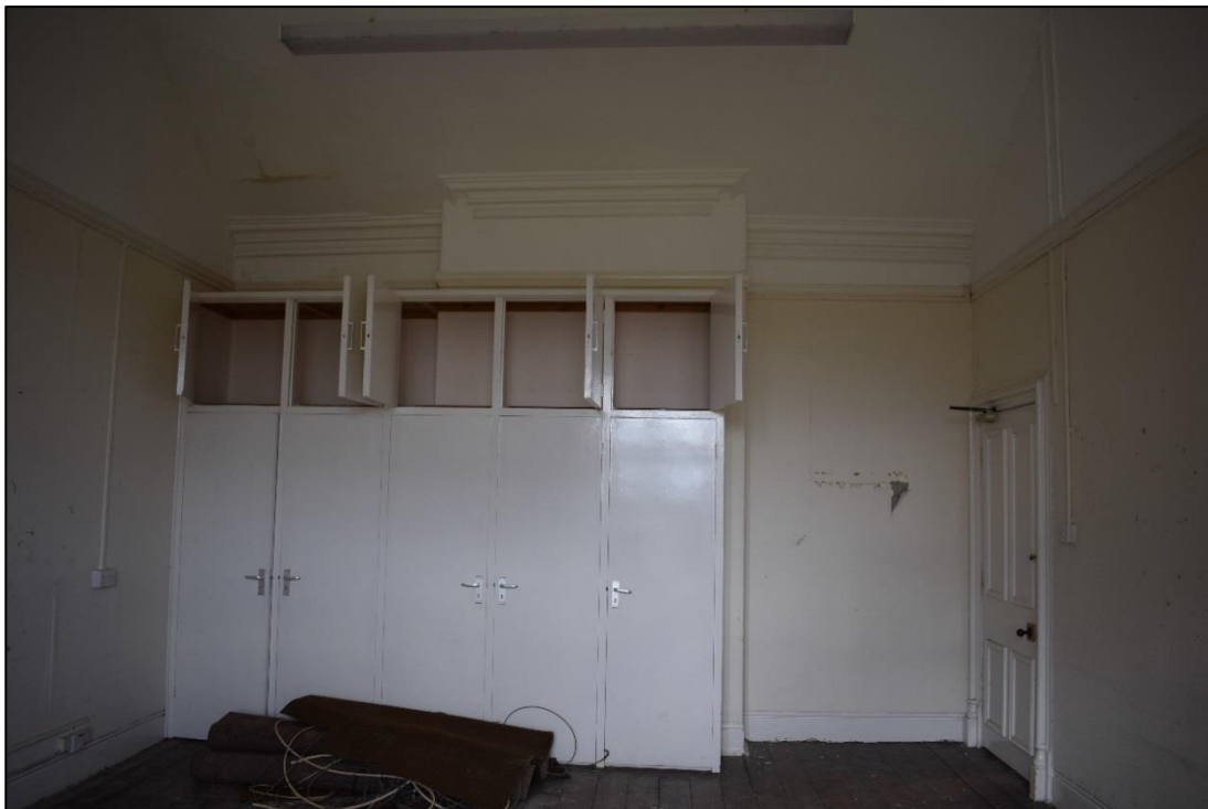
Fig. 37: Ornamental door surround and roof mouldings typical of the first floor in the historic core of the building (Fig. 12, F19). CPAT 4537-0095
