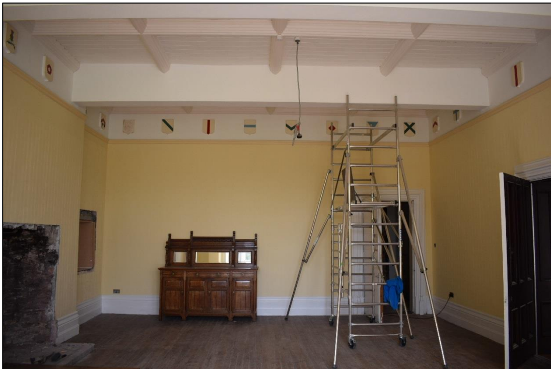
Fig. 29: Decorative shields and wooden ceiling in the western ground floor room of the historic core (Fig.11, G21). CPAT 4537-0140
