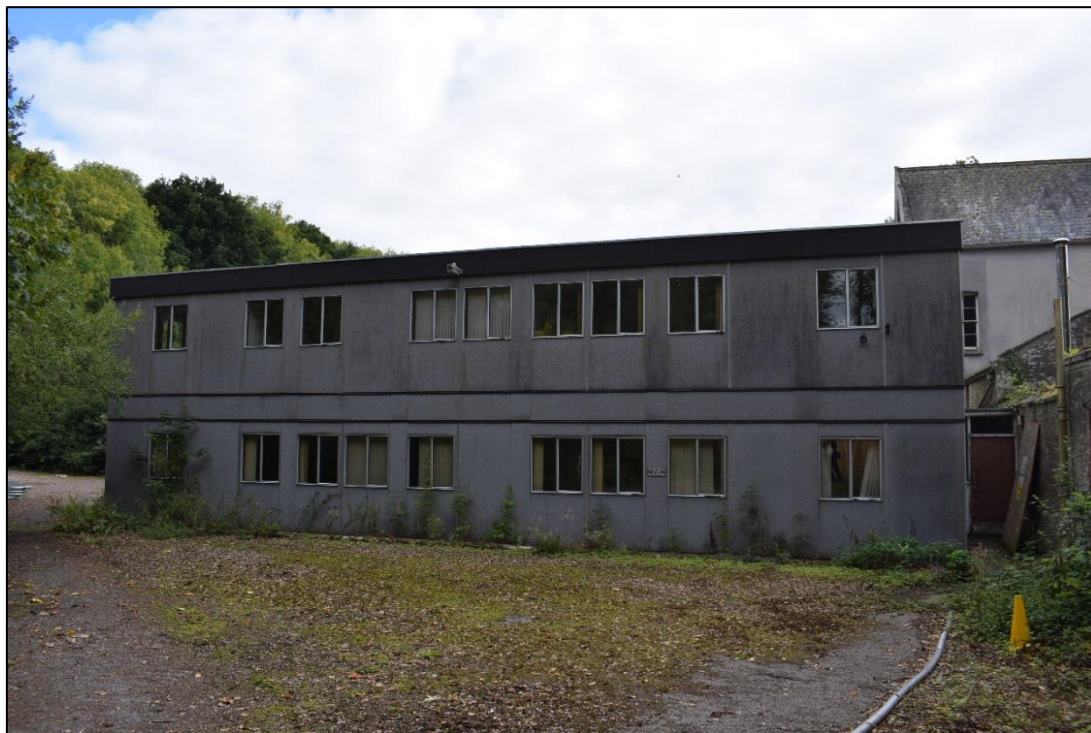
Fig. 22: The prefabricated 20 th -century wing to the north of the service court. CPAT 4537-0020
