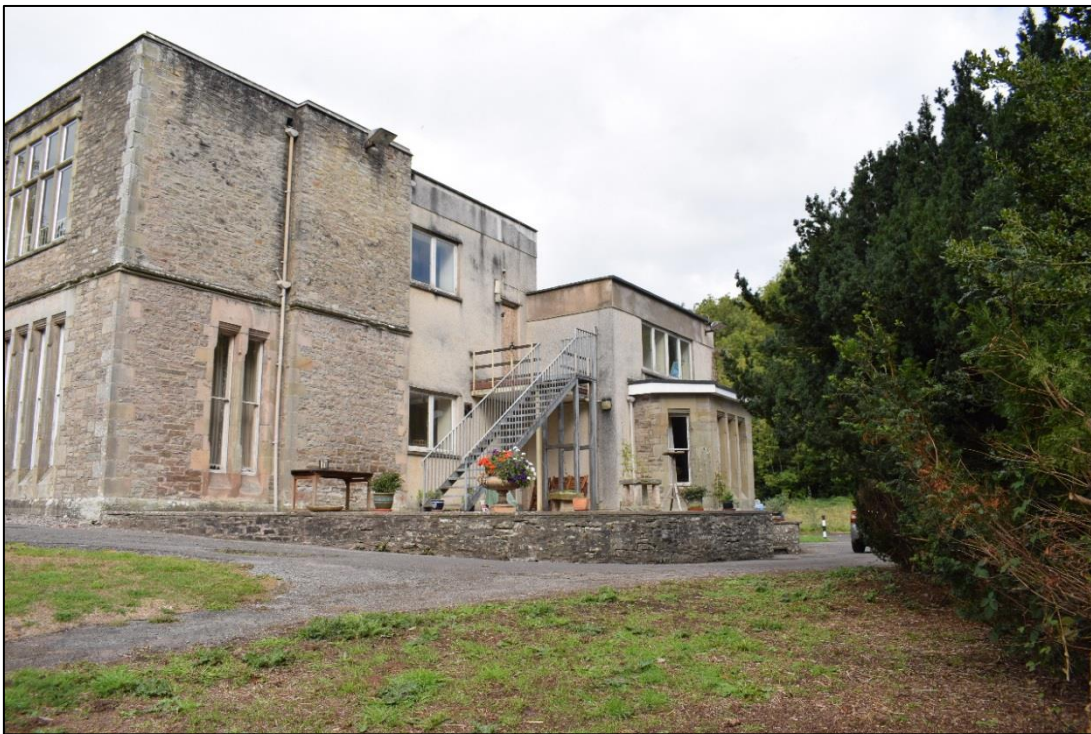
Fig. 17: Eastern end of Bronllys Hall, showing the cement rendered replacement for the part of the hall that was lost to a fire. The bay window is original. CPAT 4537-0013
