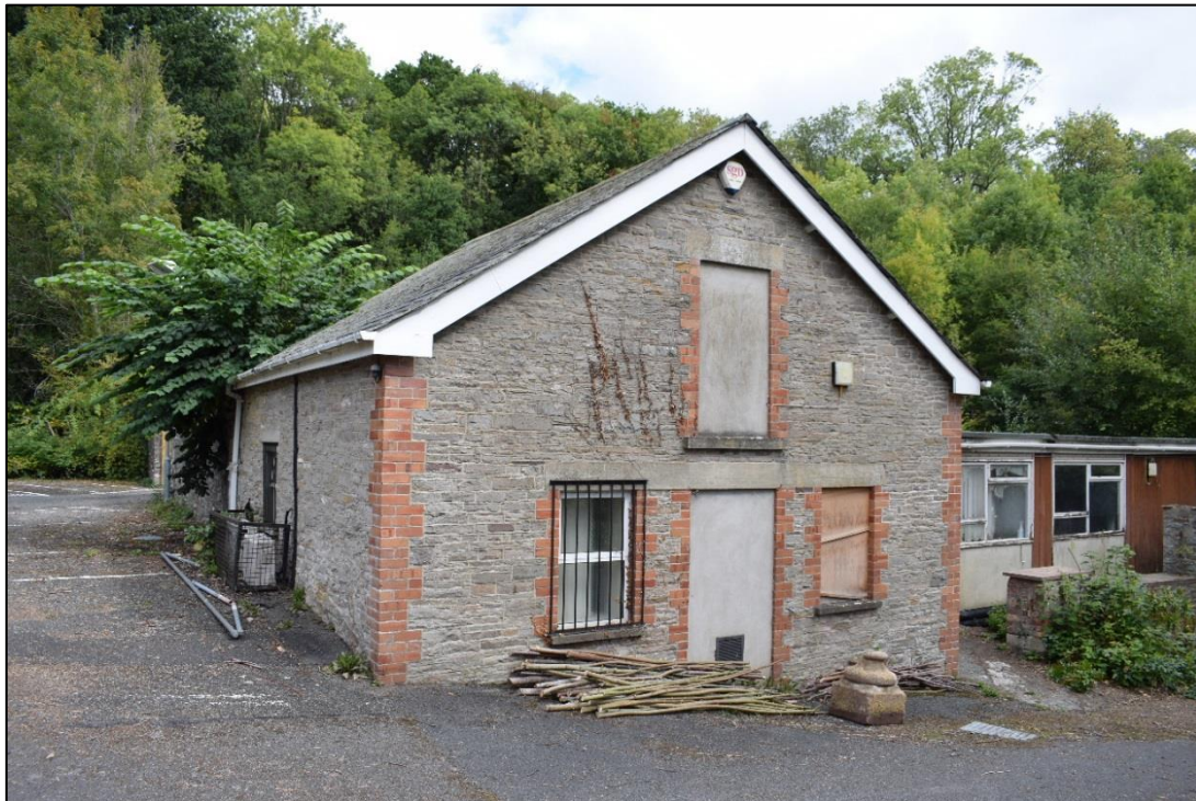
Fig. 49: The coach house at the south-west corner of the walled garden. CPAT 4537-0052
