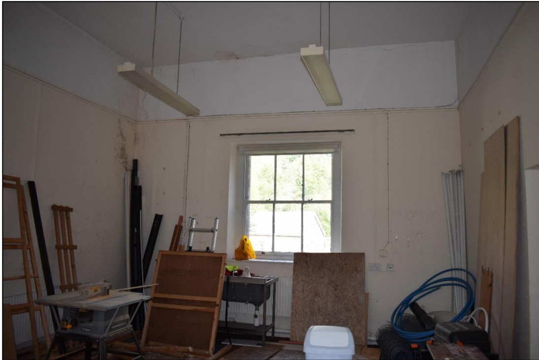
Fig. 32: Typical interior view of a room on the ground floor of the 19 th -century extension to the north of the western end of the historic core (Fig. 11, G19). CPAT 4537-0149
