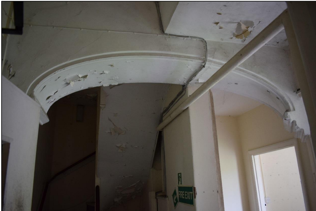
Fig.39: The skewed arch providing access to the 19 th -century wing to the north of the western end of the historic core (Fig. 12, F9). CPAT 4537-0098
