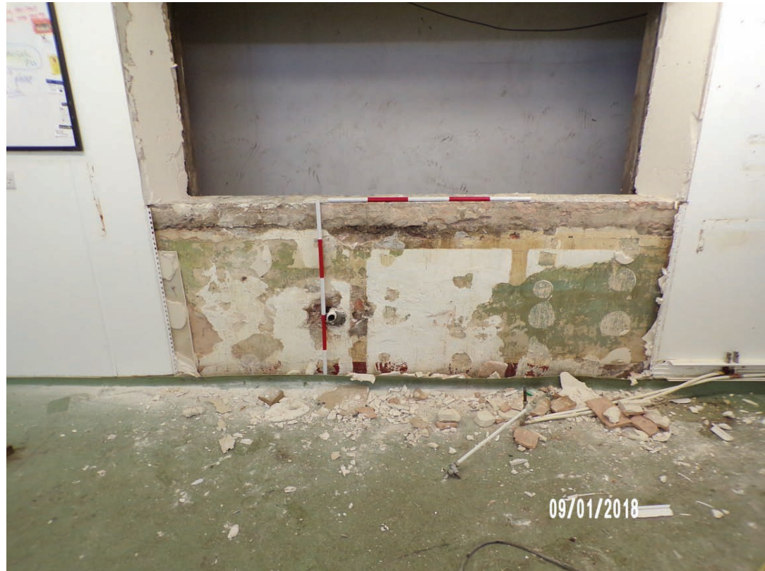
Showing architectural detail of internal face of kitchen wall beneath window opening with sink and plasterboard removed
