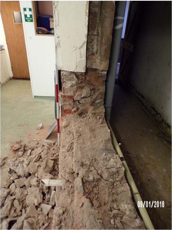
Reason for image: Showing internal brick skin butting against earlier 18/19th Century masonry wall of kitchen
