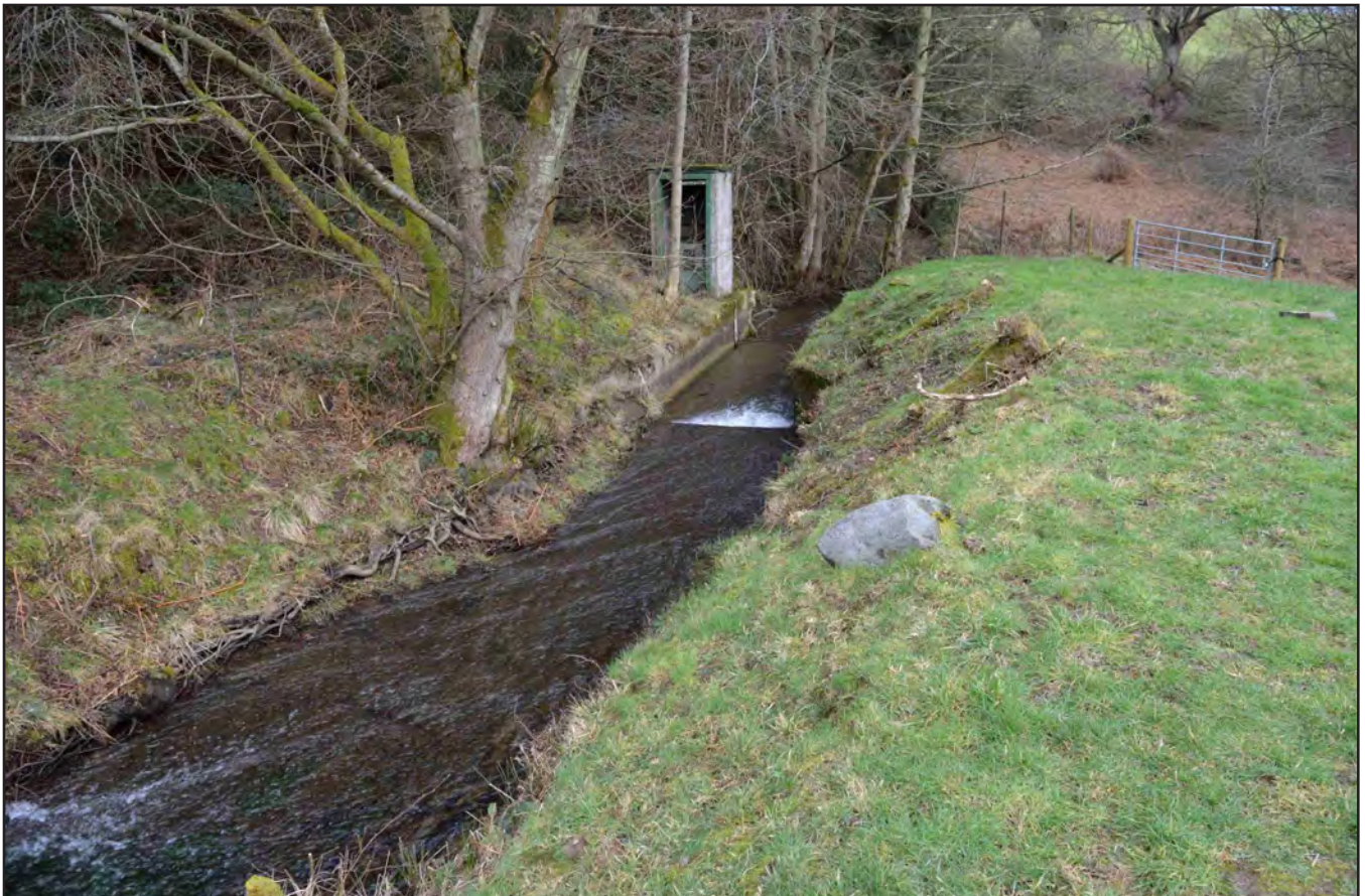
Plate 06: Concrete spillway leading to Nant Gain; no scale (archive reference: G2597_010)
