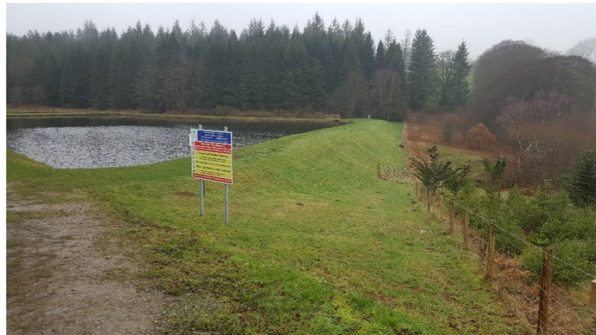
View along the downstream face of Cilcain No. 2 embankment
