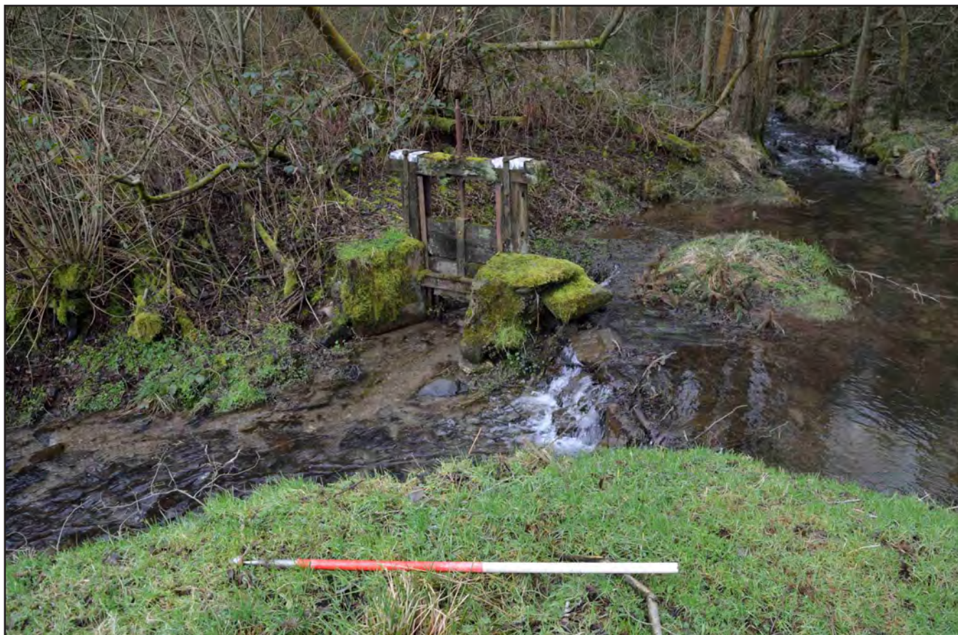
Plate 11: Obsolete sluice gate, Cilcain 1; scale 1x1m (archive reference: G2597_021)
