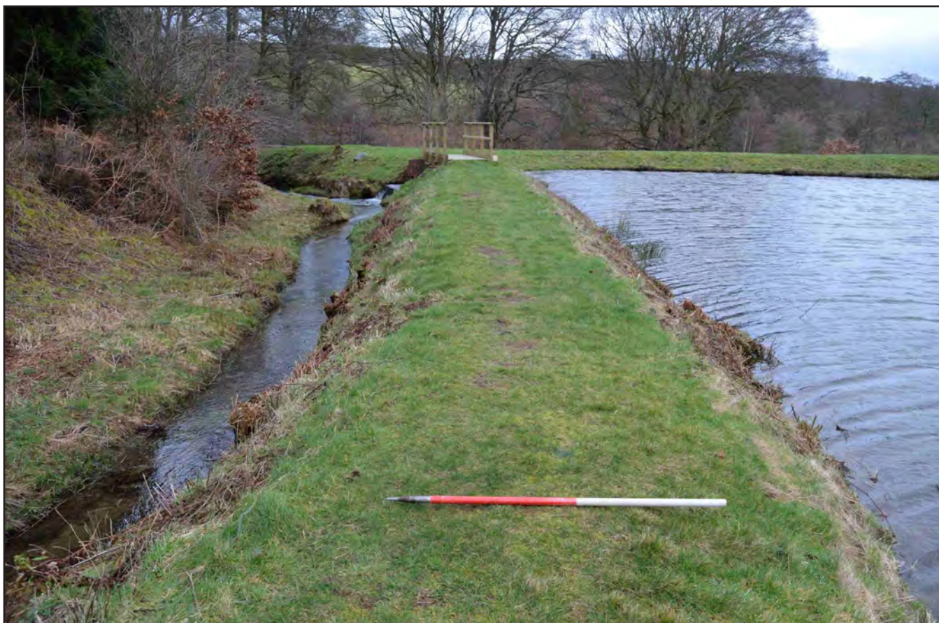
Plate 08: Nant Gain routed alongside bank to spillway; scale 1x1m (archive reference: G2597_012)
