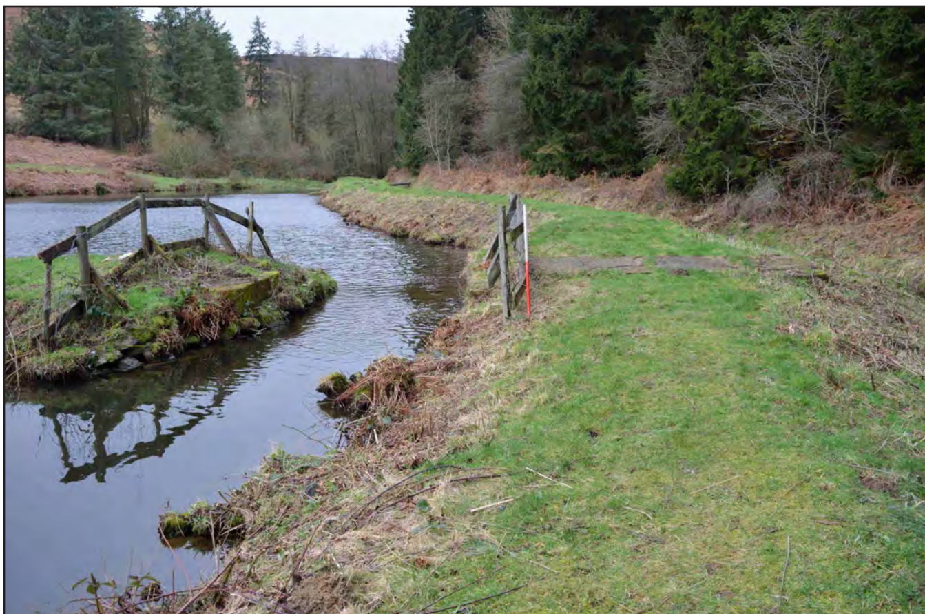
Plate 10: Concrete reinforcement to embankments; scale 1x1m (archive reference: G2597_015)
