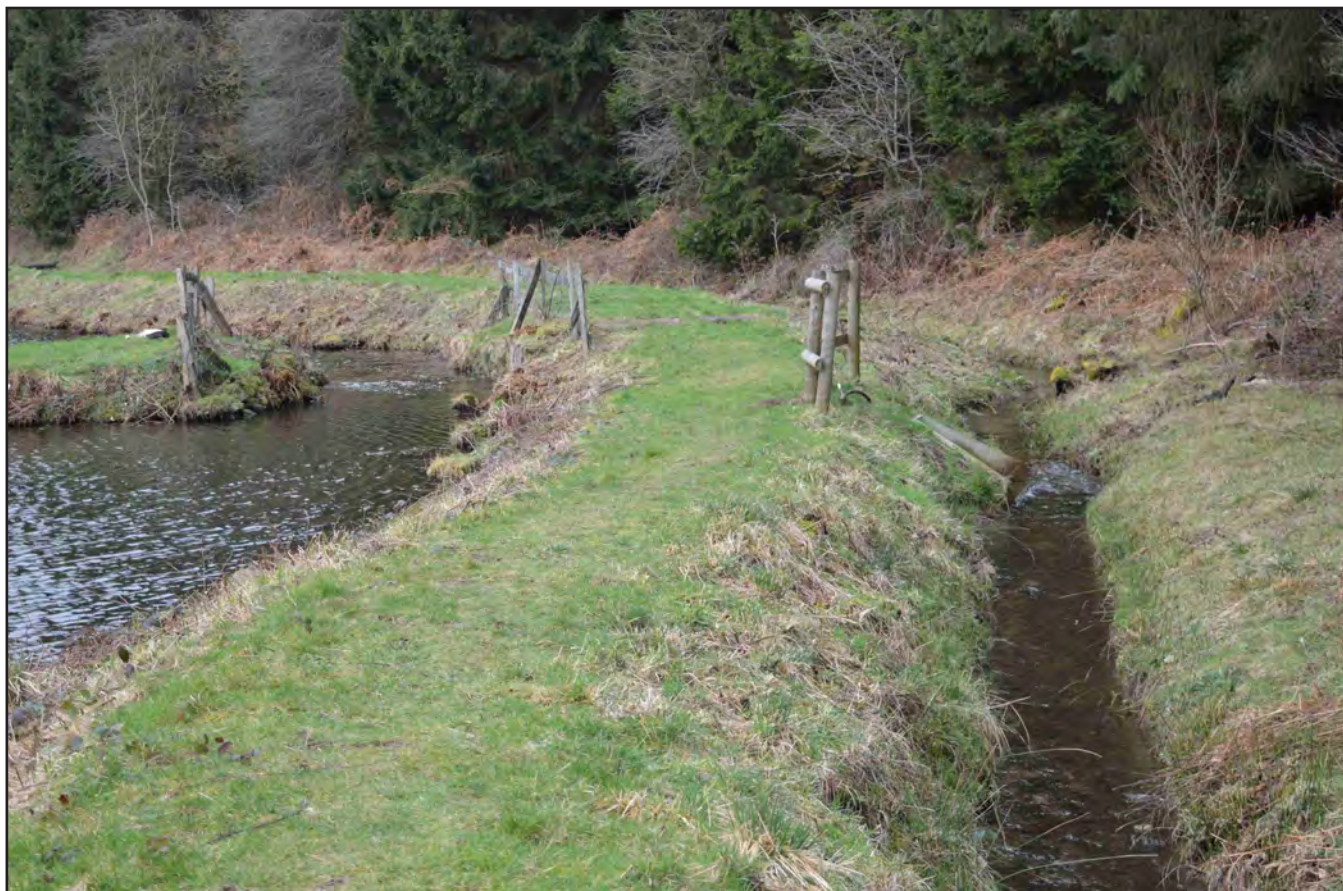
Plate 09: Secondary overflow near to central dividing bank; no scale (archive reference: G2597_014)
