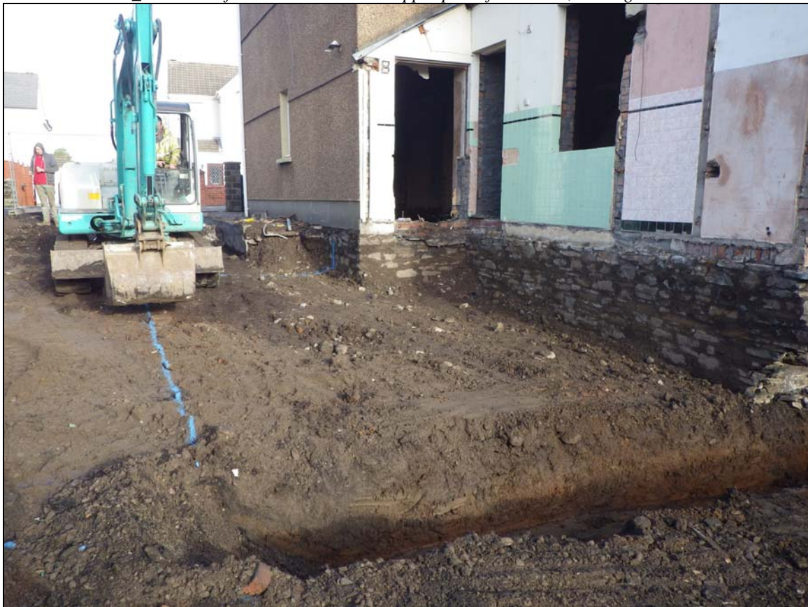
Plate 4: CSL2013_104: After excavation of southernmost foundation trench, looking northeast.
