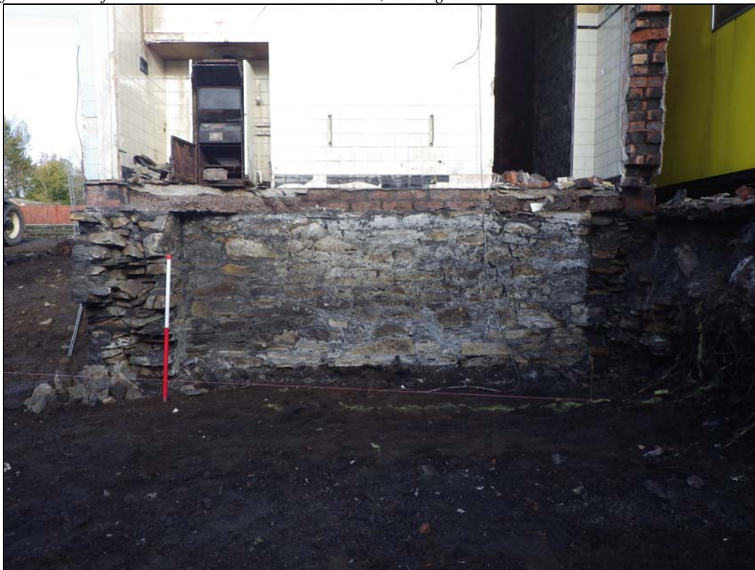
Plate 2: CSL2013_102: Detail of the foundations of the house, looking north northwest.
