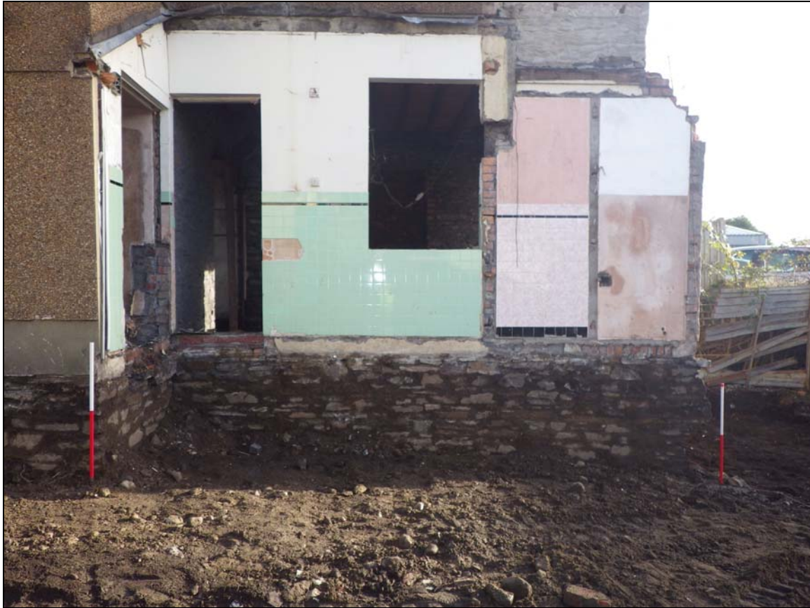
Plate 3: CSL2013_103: Stone foundations and brick upper part of the house, looking east northeast.
