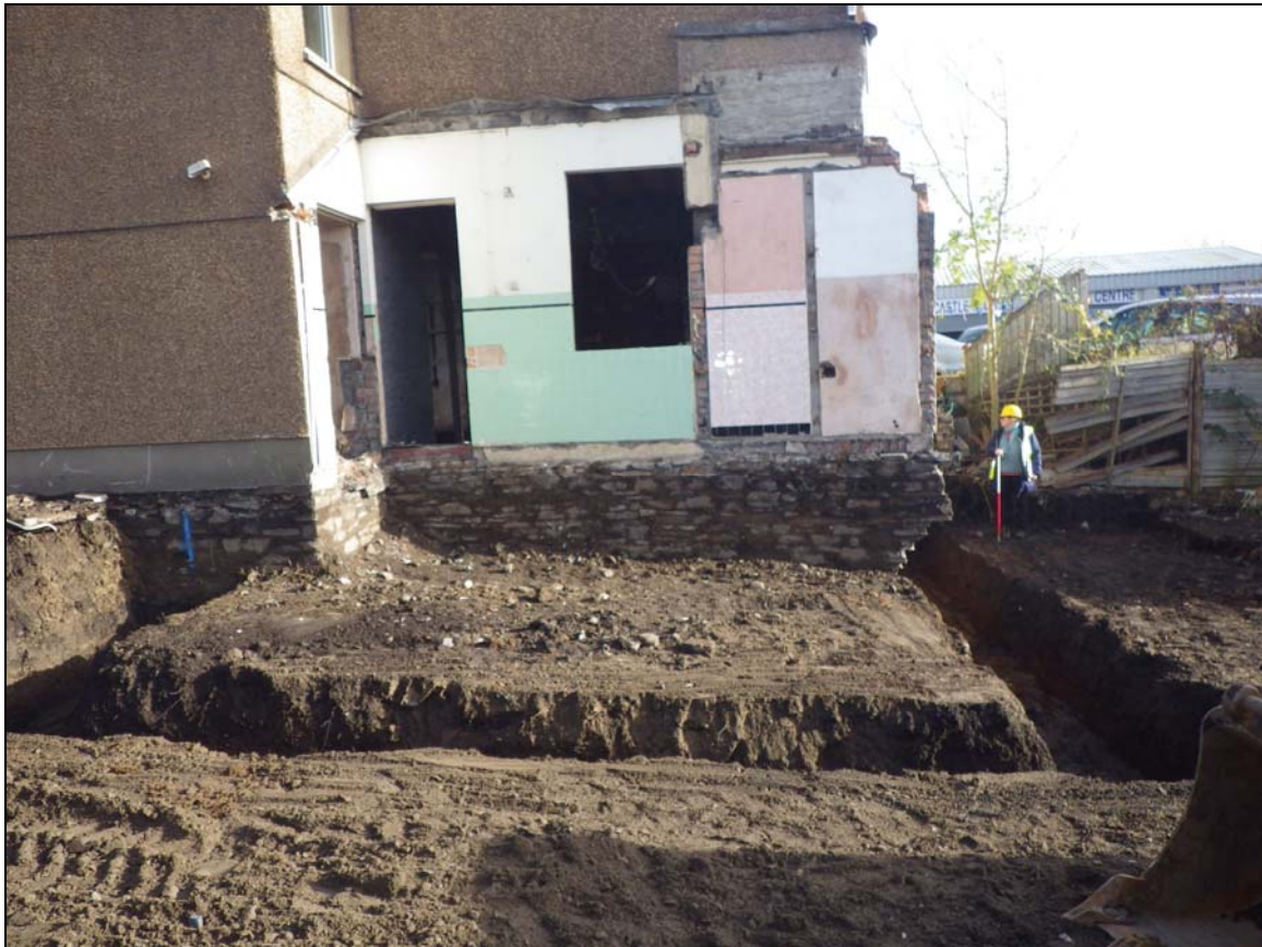
Plate 5:CSL2013_105: Excavated foundation trenches, looking east northeast.
