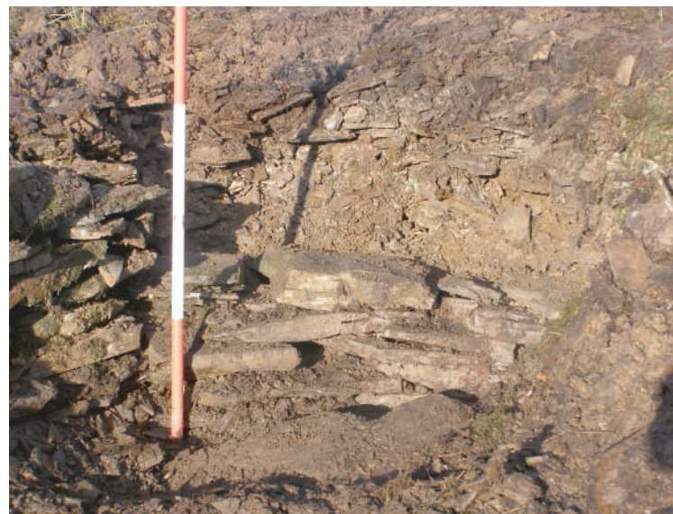
Plate 10. Detail of stone revetting during removal in area of southern Quarry pit No. 1.
