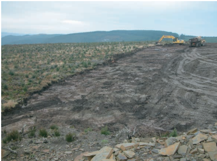
Plate 15. Working shot during stripping for area of cuts 8-10. Looking eastward.
