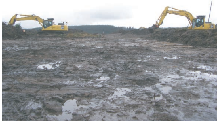
Plate 1. Working shot during top soil stripping whilst widening trackway
