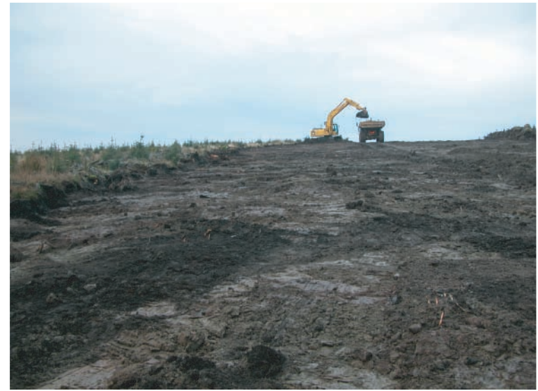
Plate 16. Working shot during stripping for area of cuts 8-10. Looking eastward.
