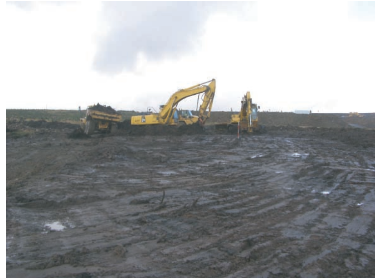
Plate 2. Working shot during excavation of lagoon area. Looking north.
