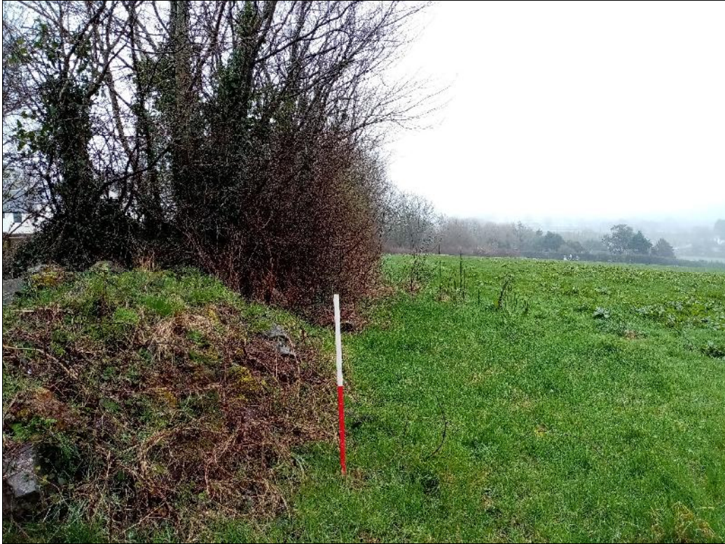
Plate 5: RBW2021_005 From the gateway in the northwest corner of the field looking east-northeast along the field boundary. The vegetation covered rubble to the left of the ranging rod is probably the remains of a stone gatepost removed in recent years so the gateway could be widened.
