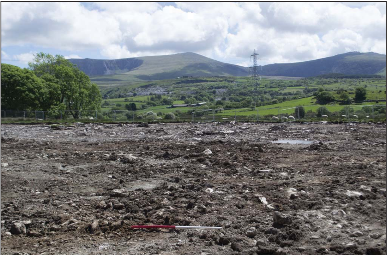
Plate 8: General Site Looking SE From Corner of BT Compound; scale 1x1.0m (archive reference: G2688_211).
