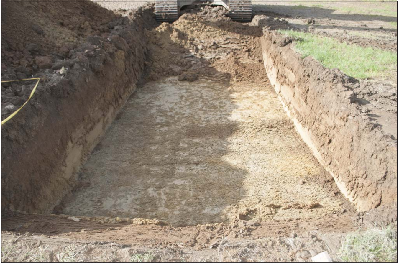
Plate 40: View of Test Pit 3 after excavation to full depth of 1.2m showing glacial clay; scale not used; view from E (archive reference: G2589_157).
