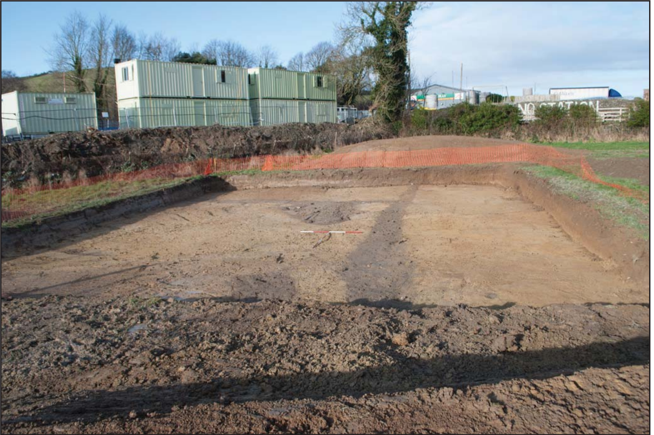
Plate 01: Mitigation excavation area post-machining, scale 2x2m (archive ref: G2589_066).
