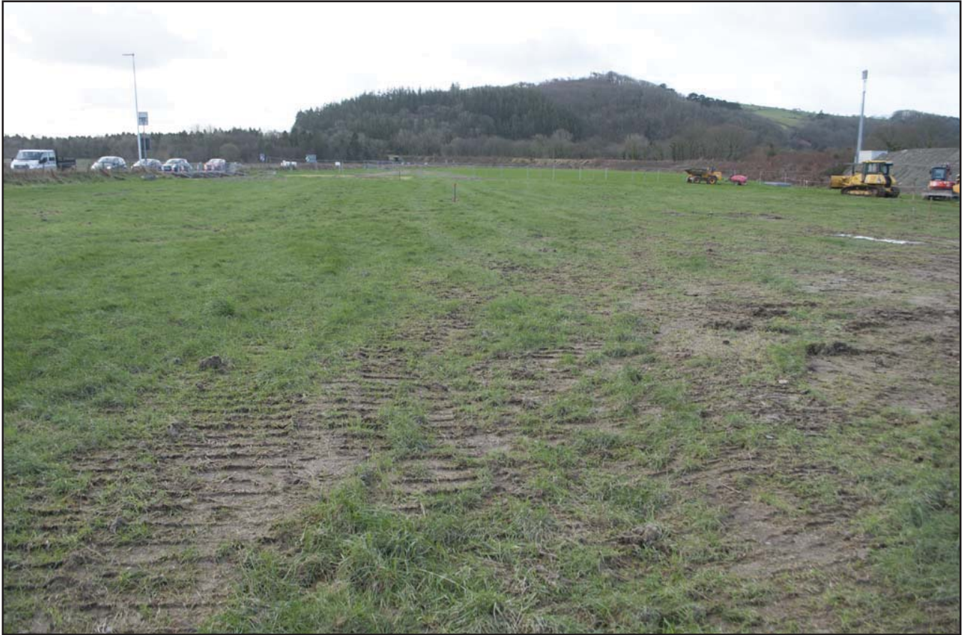
Plate 26: General view of the location of new site entrance before the commencement of work; scale 1x1m; view from NE (archive reference: G2589_112).
