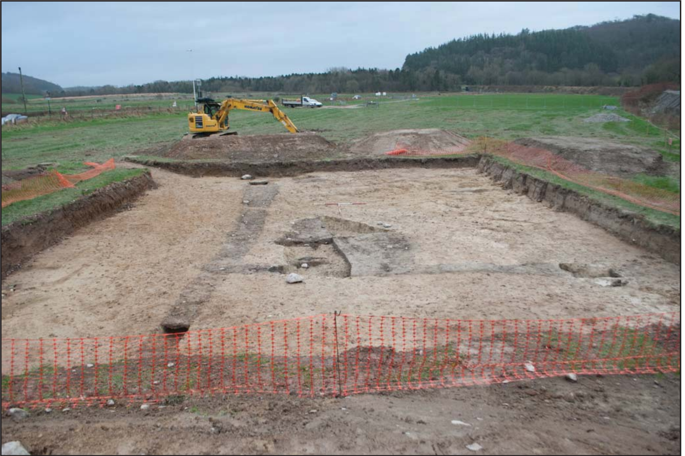
Plate 25: Mitigation area post-excavation, viewed from the north, scale 2x2m (archive ref: G2589_110).
