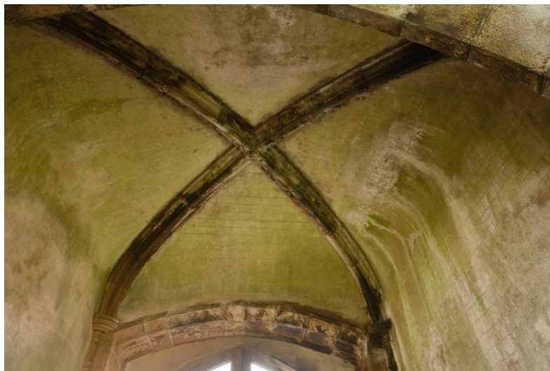
Figure 15. Quadrupartite vault in the passage of the lower stage.
