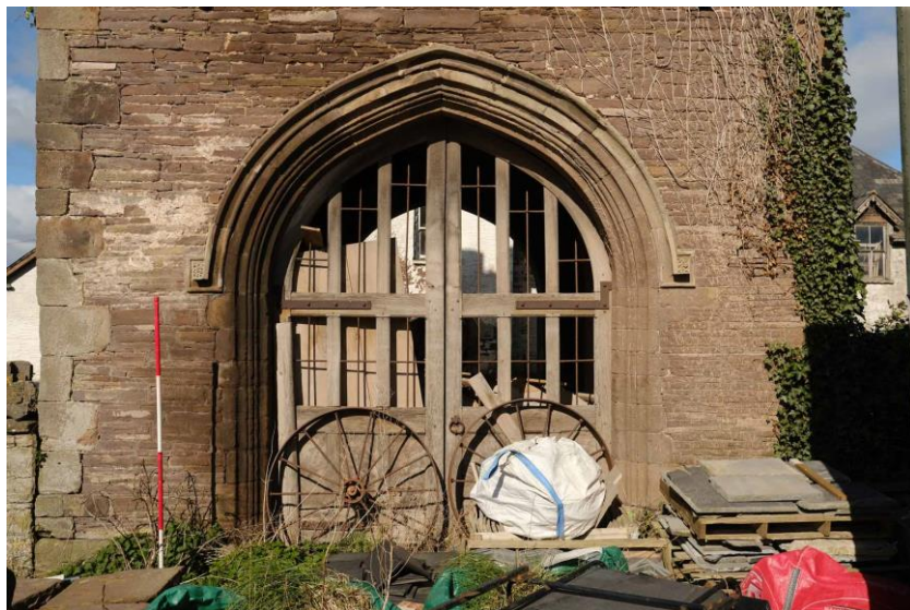
Figure 9. Double gates in south-east front.
