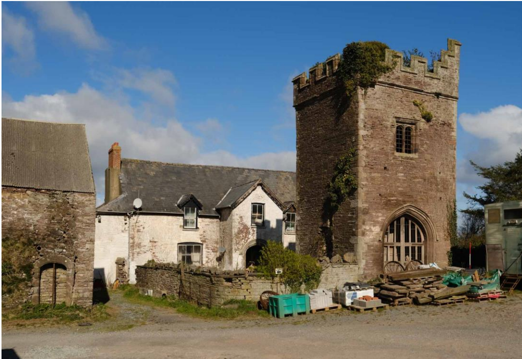
Figure 8. South-east (front) and south-west fronts, with garden wall and farmhouse in the background.
