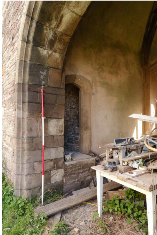
Figure 12. Arch in north-west front.
