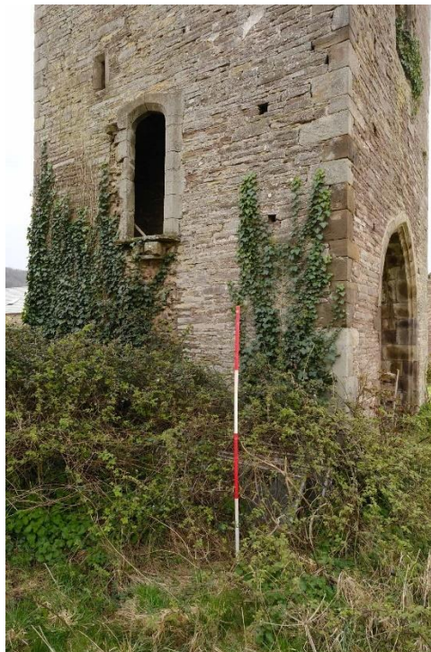
Figure 13. Doorway, stair light, and scar of original forecourt wall in north-east front.
