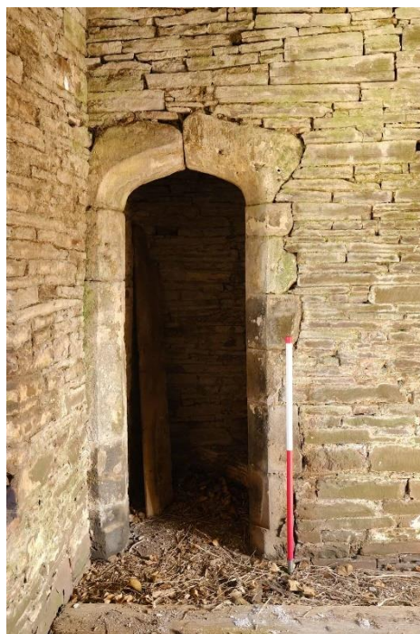
Figure 16. Doorway to stair from upper stage to parapet.
