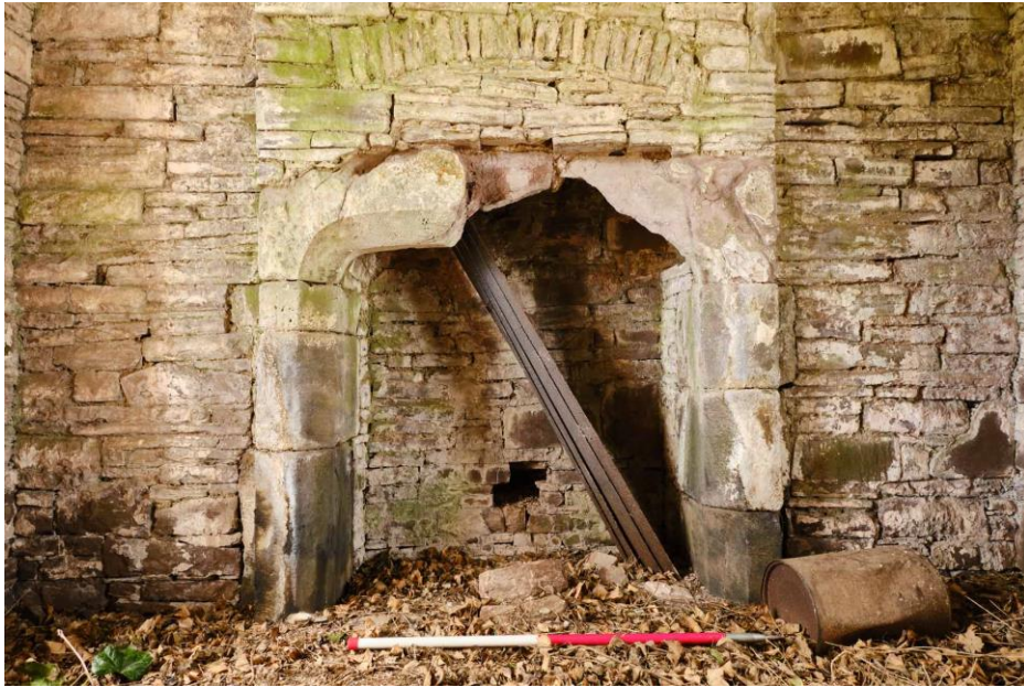
Figure 17. Fireplace in the upper stage.
