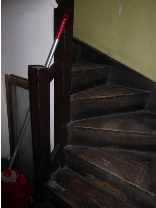
Figure. 53 Foot of attic staircase
