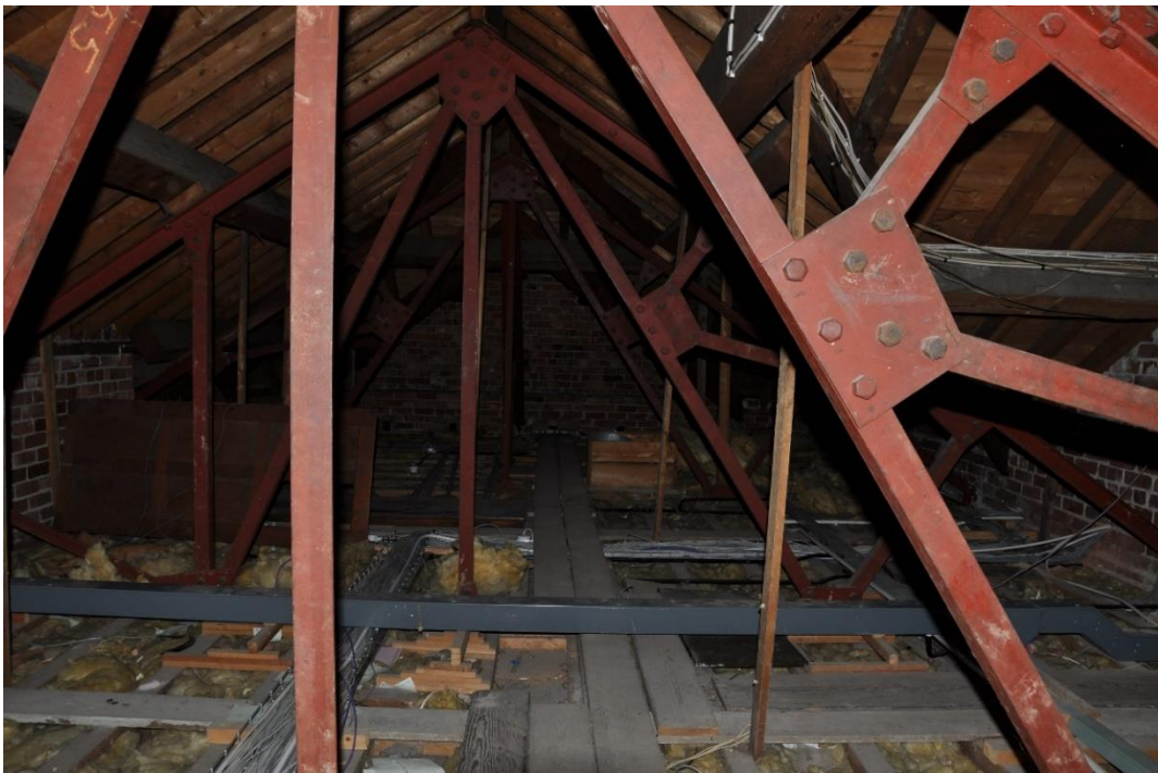
Figure. 55 Steel trusses to the attic over the 1931 block © Lovelock Mitchell Architects
