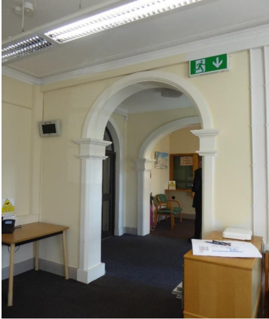
Figure 21. Arched openings to entrance hall.
