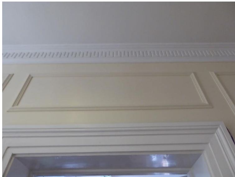
Figure. 45 Detail of panelling and frieze to room adjoining former Clerk's Office
