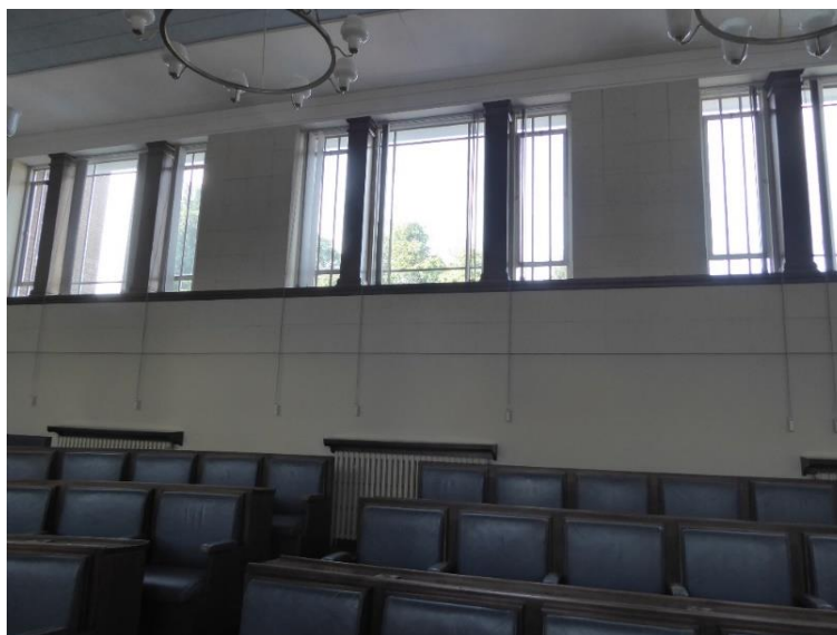
Figure 36. Council Chamber high level windows
