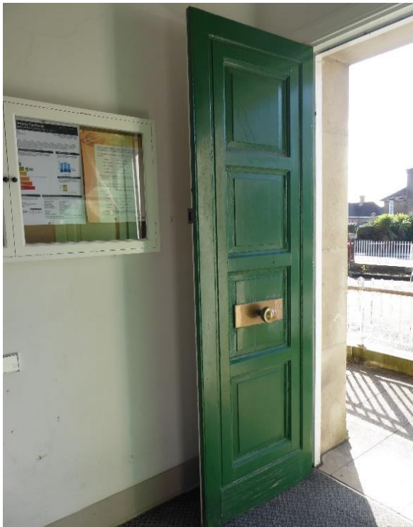
Figure 19. Outer entrance doors.
