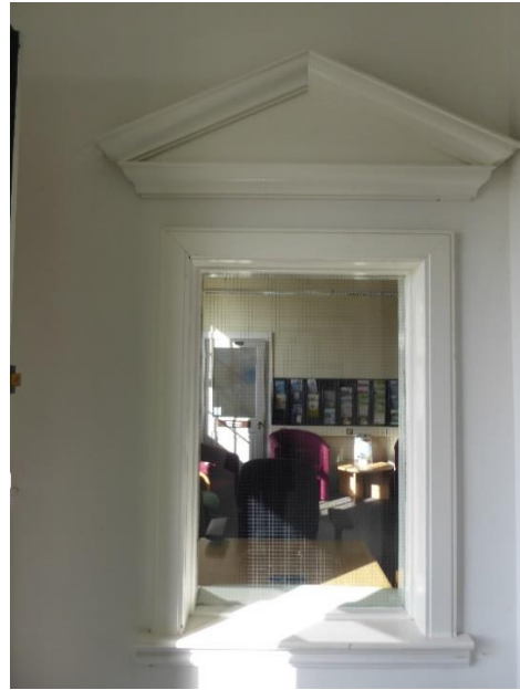
Figure 22. Former reception hatch.
