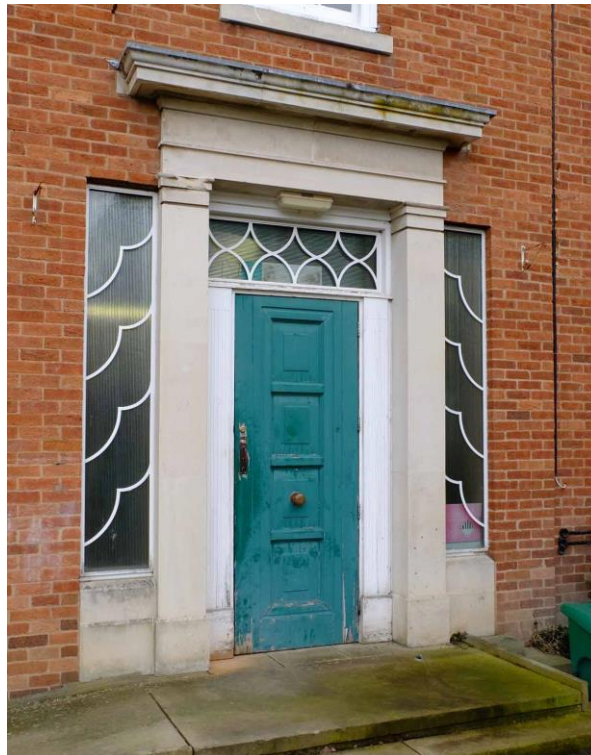
Figure 16. Doorway in the secondary wing.
