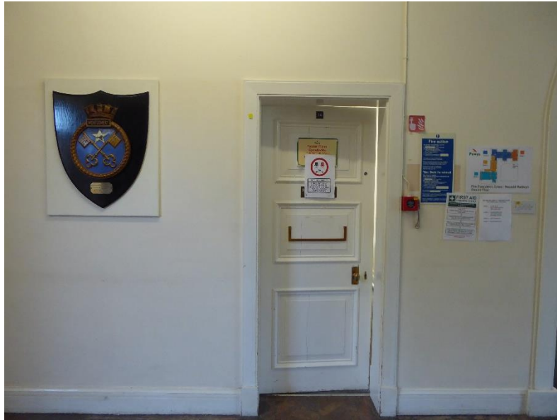
Figure 31. Example of 3-panel door in staircase hall, this one into the Members Video Conferencing Room
