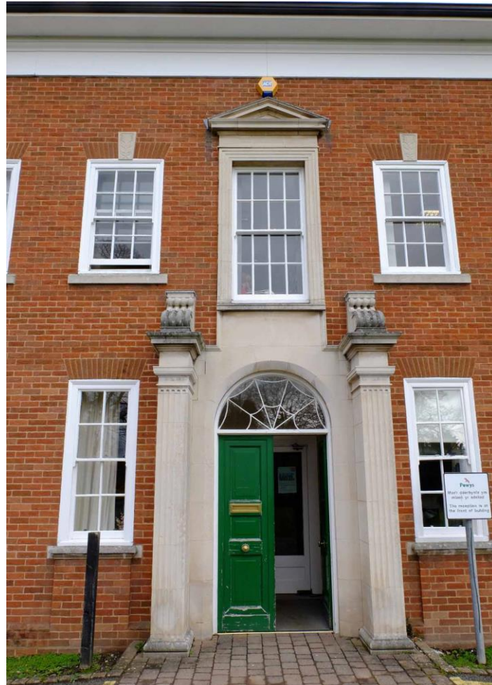
Figure 17. Entrance to the council suite.
