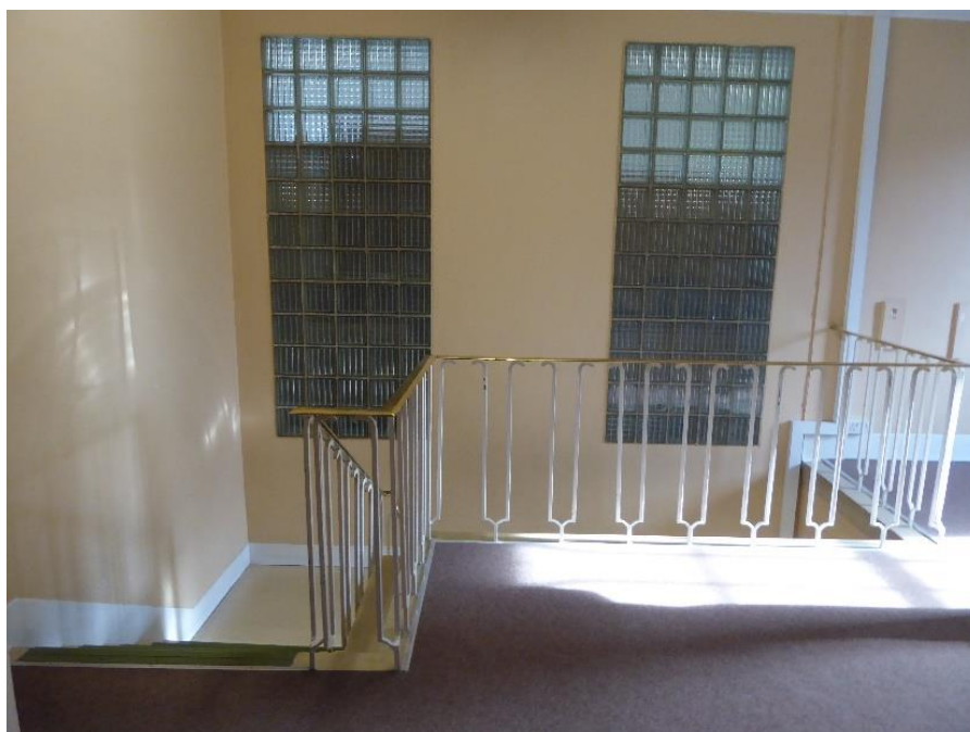
Figure. 48 1938 Staircase windows and 1 st floor landing
