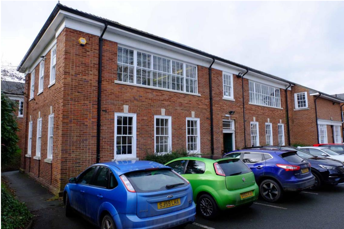
Figure 13. Rear (north-east) wall.
