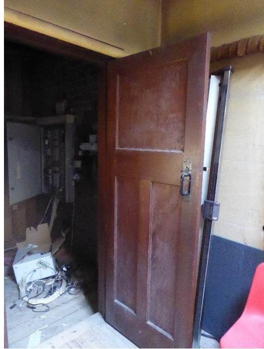
Figure 54 Attic door and door furniture
