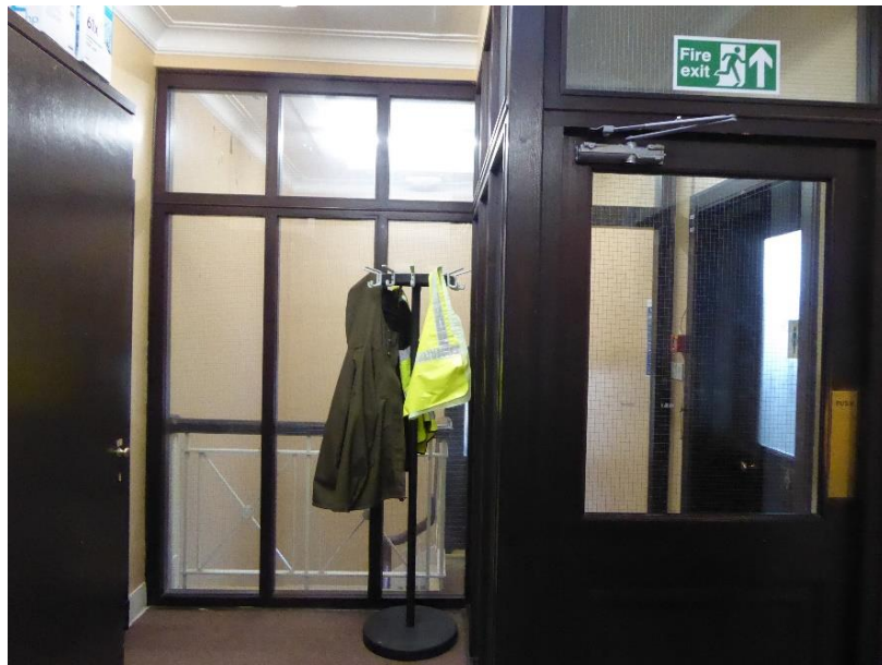
Figure. 41 1 st floor landing in 1931 block showing modern enclosure of staircase
