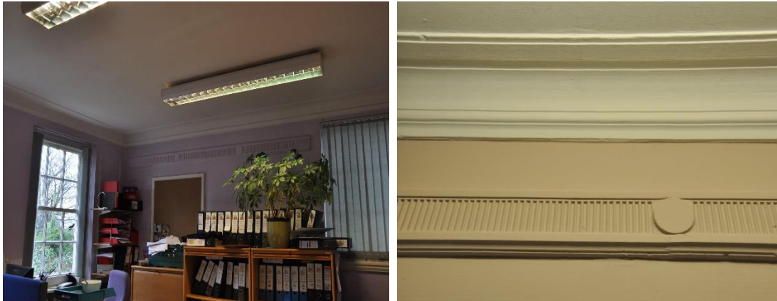
Figures 46 and 47 1 st floor surviving sections of neo-classical frieze to centre of south-east elevation in 1938 phase © Lovelock Mitchell Architects
