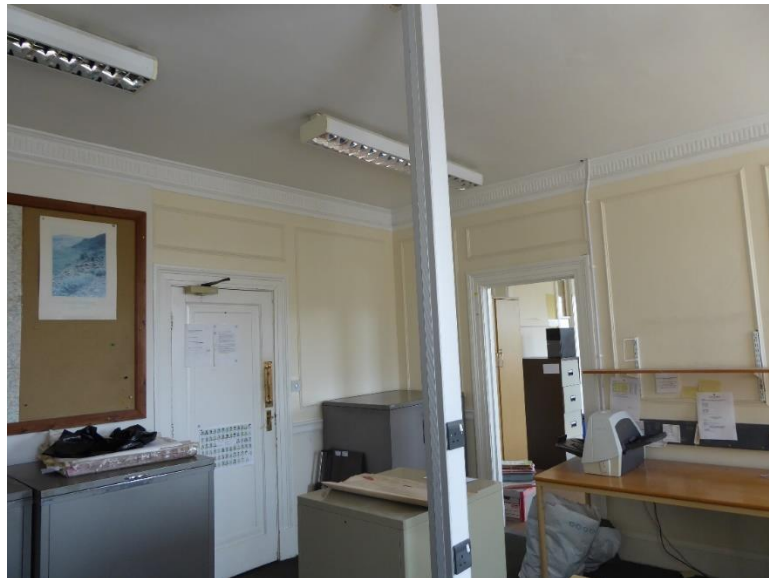
Figure. 44 Adjoining room to former Clerk's Office
