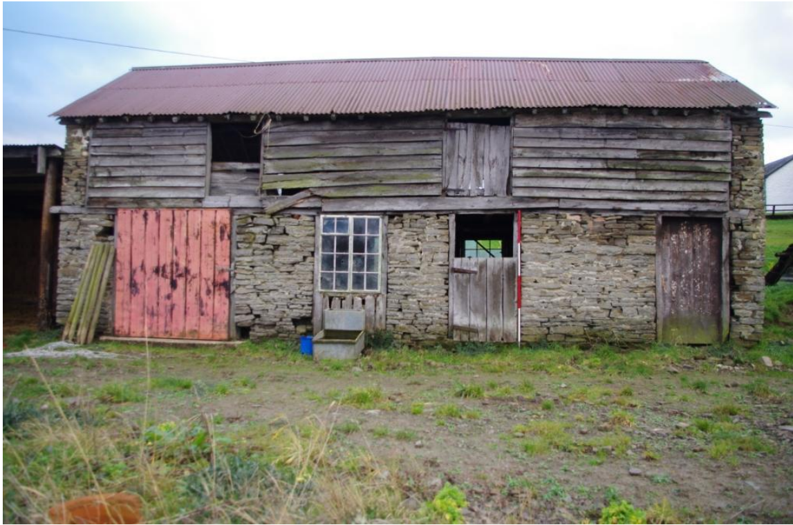
Figure 3 Principal Elevation, General View (Looking South East).
