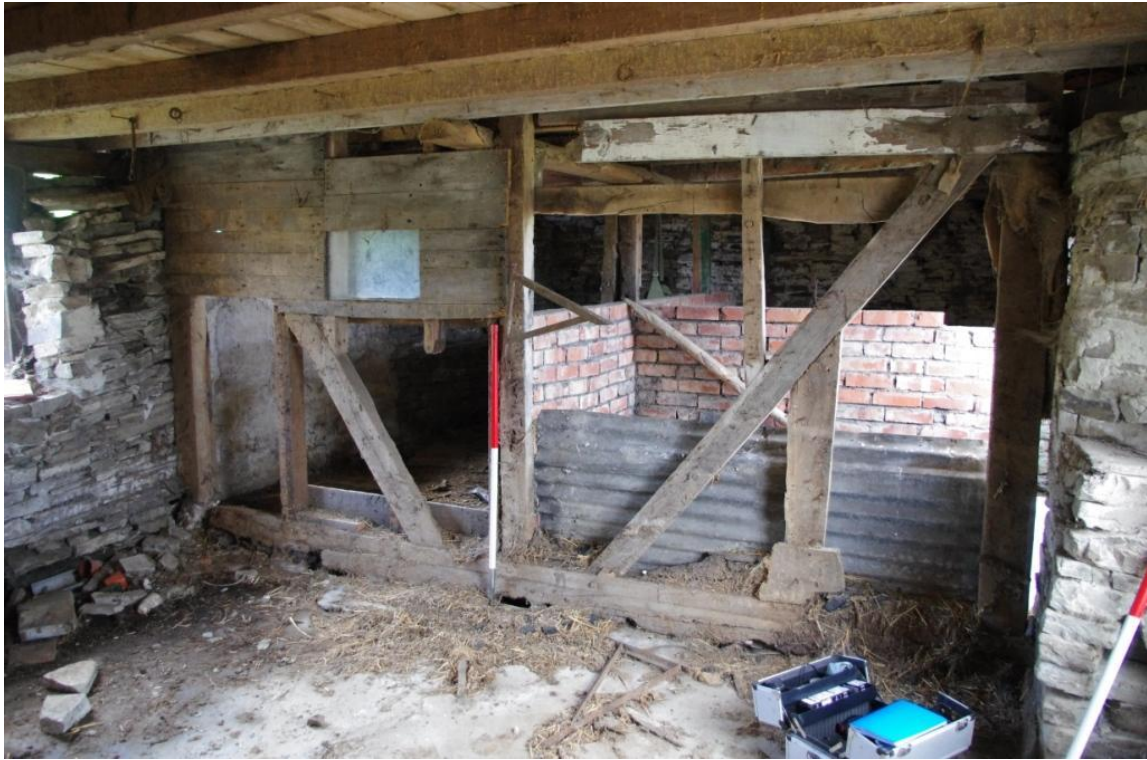
Figure 7 A (2) Cross Frame (Looking South – South West).
