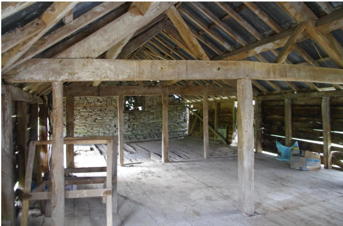
Figure 8 A (4) General View (Looking West).
