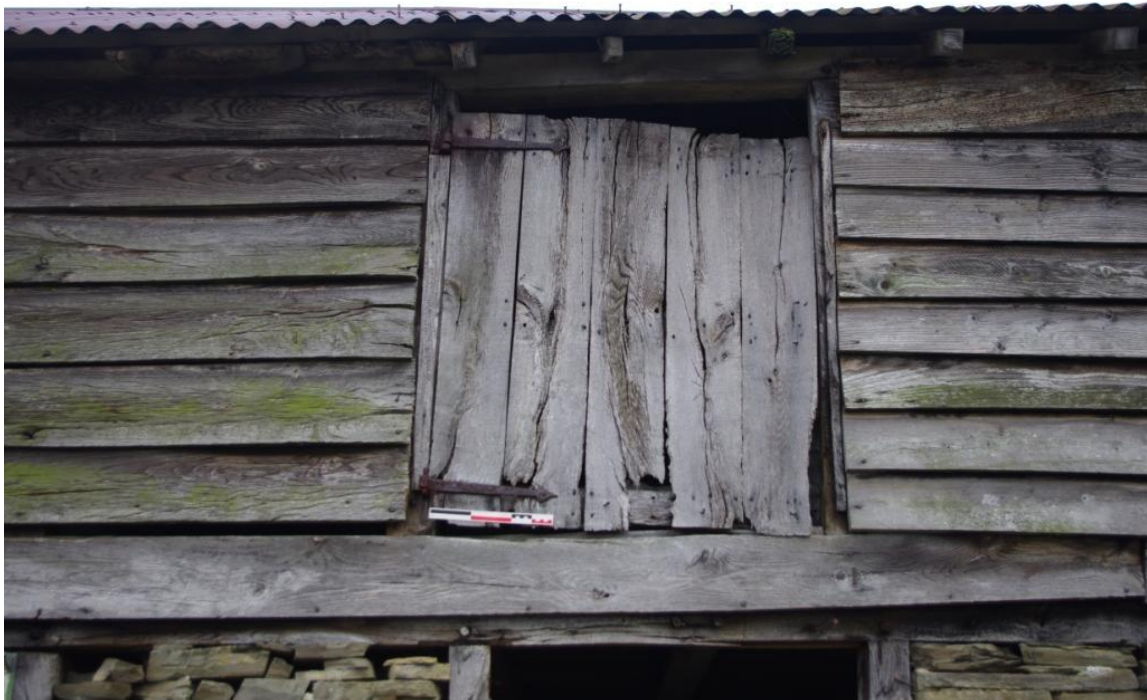
Figure 6 Pitching Door on Principal Elevation, Showing Potentially 17th Century Hinge (Looking South East).
