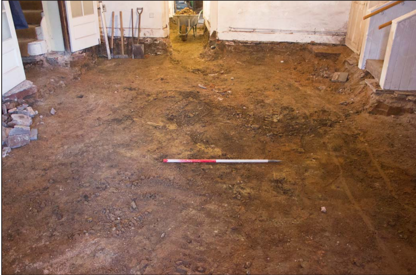
Plate 15: Post excavation shot of Entrance Hall, Argoed Hall, Mynydd Isa, Mold, Flintshire - from the east - scale 1.00m
