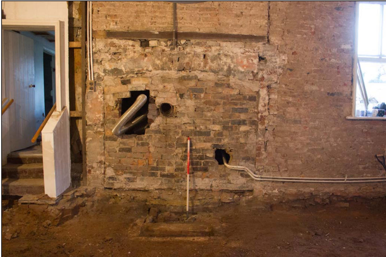
Plate 20: Former fireplace, Northern elevation in Entrance Hall, Argoed Hall, Mynydd Isa, Mold, Flintshire - from the south - scale 1.00m
