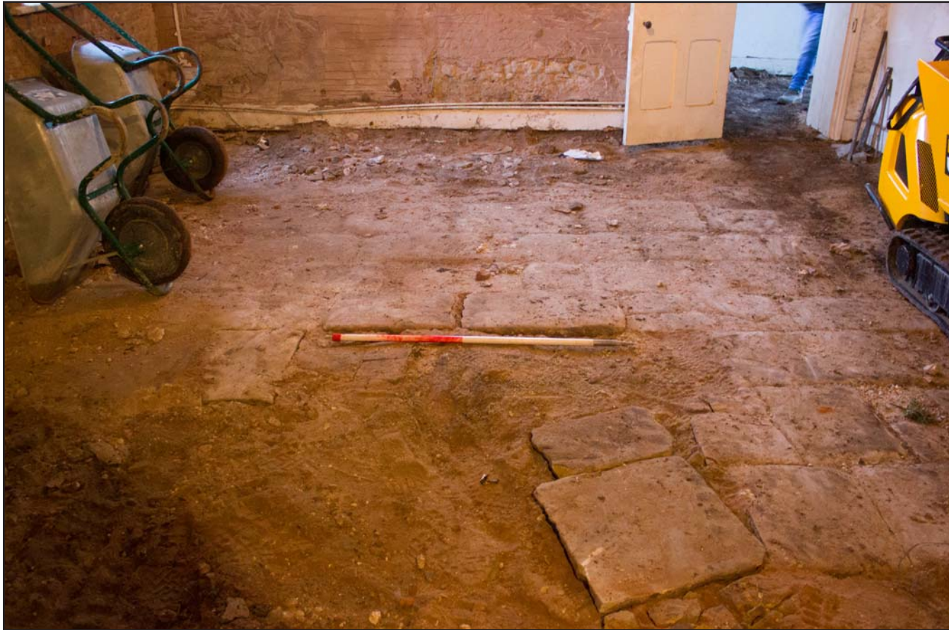
Plate 06: Pre removal of Flagstones in Entrance Hall, Argoed Hall, Mynydd Isa, Mold, Flintshire - from the west - scale 1.00m
