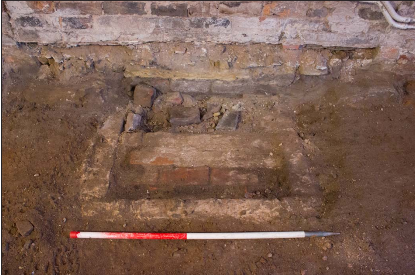
Plate 21: Blocked up access to Basement, to south of fireplace located on the northern elevation, Entrance Hall, Argoed Hall, Mynydd Isa, Mold, Flintshire - from the south - scale 1.00m
