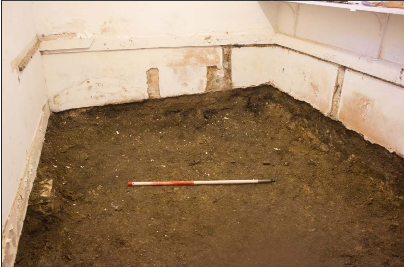
Plate 02: Post excavation shot of Pantry, Argoed Hall, Mynydd Isa, Mold, Flintshire - from the southwest - scale 1.00m
