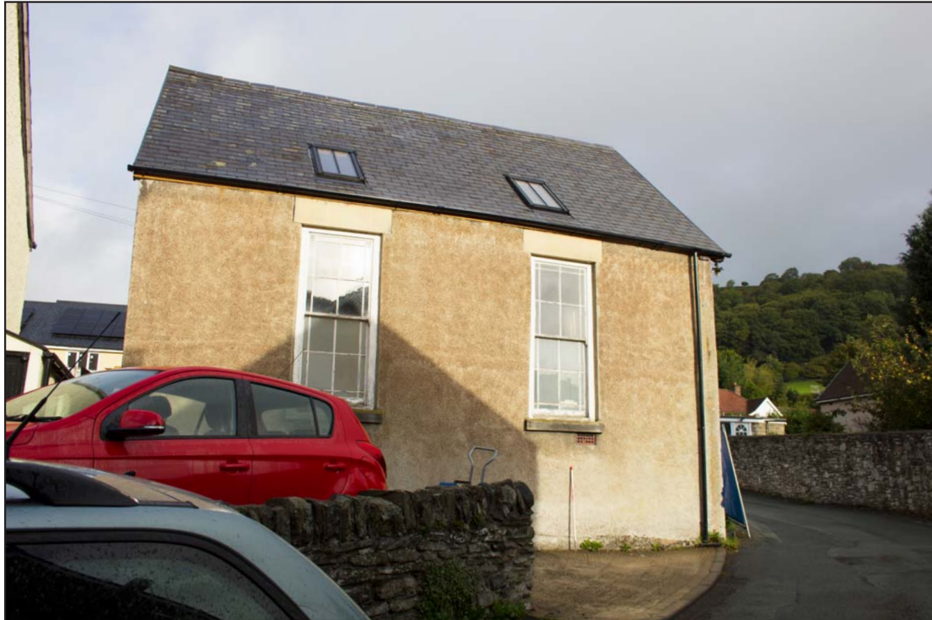
Plate 05: Oblique shot of southwest and southeast external elevations of Capel Sion, Pontfadog, Llangollen - from the south/southeast - 1.00m scale
