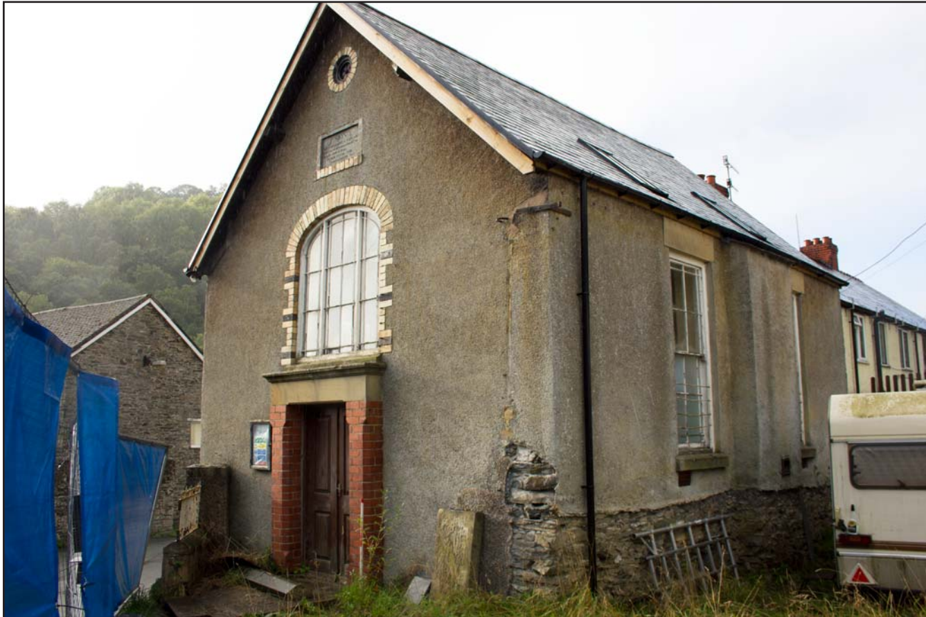
Plate 11: Oblique shot of northwest and northeast external elevations of Capel Sion, Pontfadog, Llangollen - from the north - 1.00m scale
