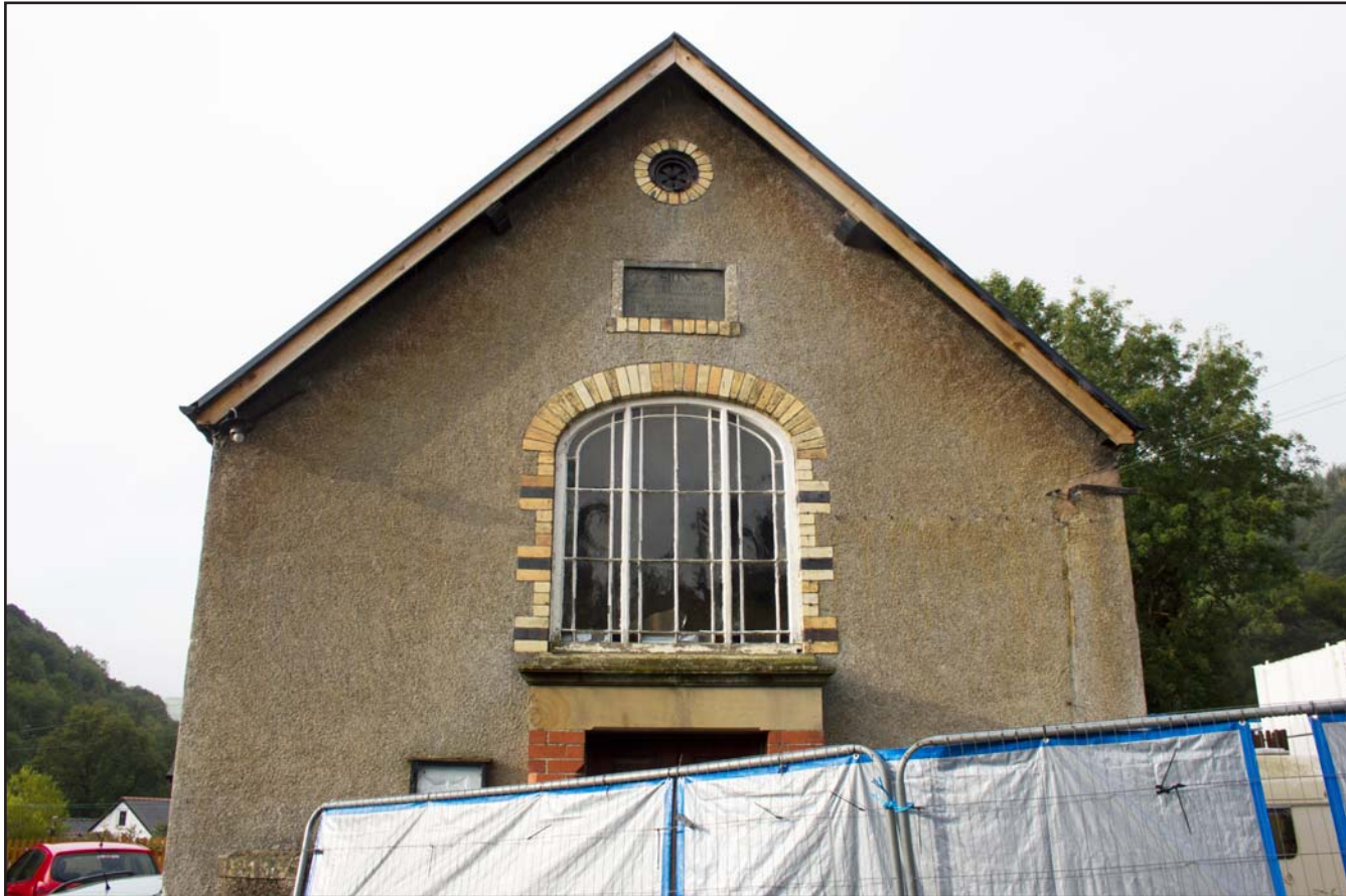
Plate 09: Framed shot of northeast external elevation of Capel Sion, Pontfadog, Llangollen - from the northeast - 1.00m scale
