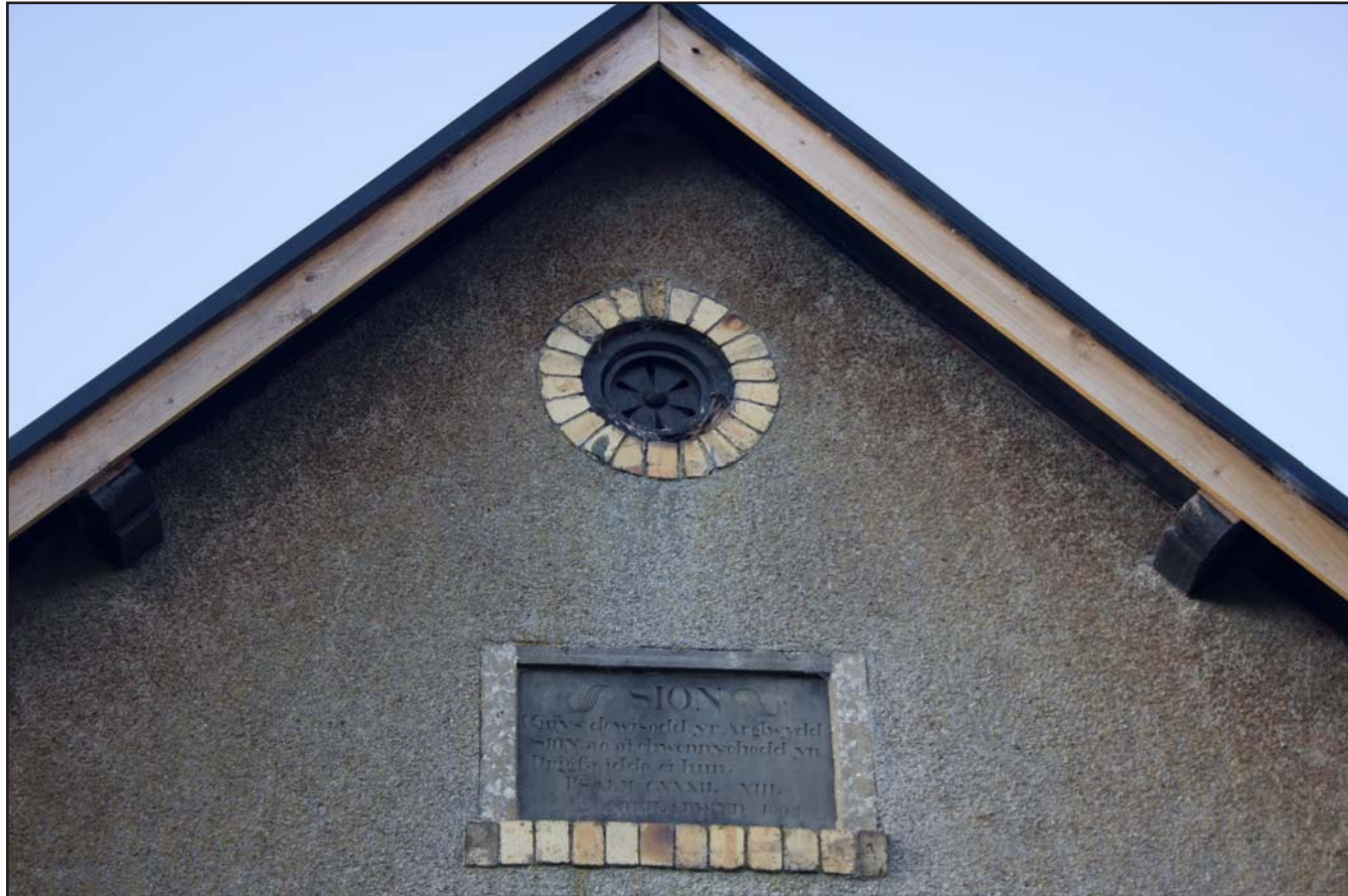
Plate 14: Slate plaque located above doorway on northeast external elevation of Capel Sion, Pontfadog, Llangollen - from the northeast - no scale
