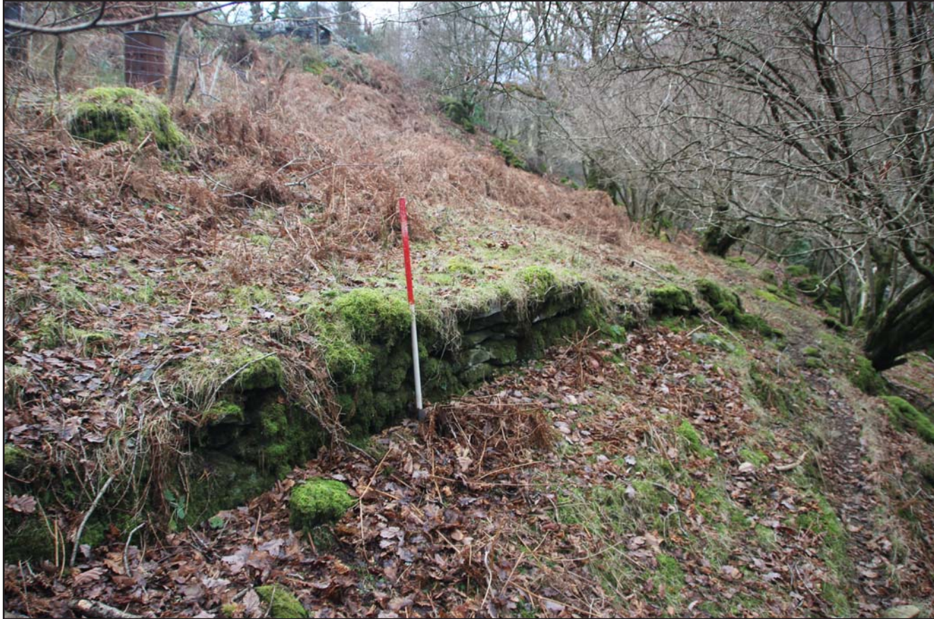
Plate 17: Section of walling (feature 2), from the south. Scale 1.0m.
