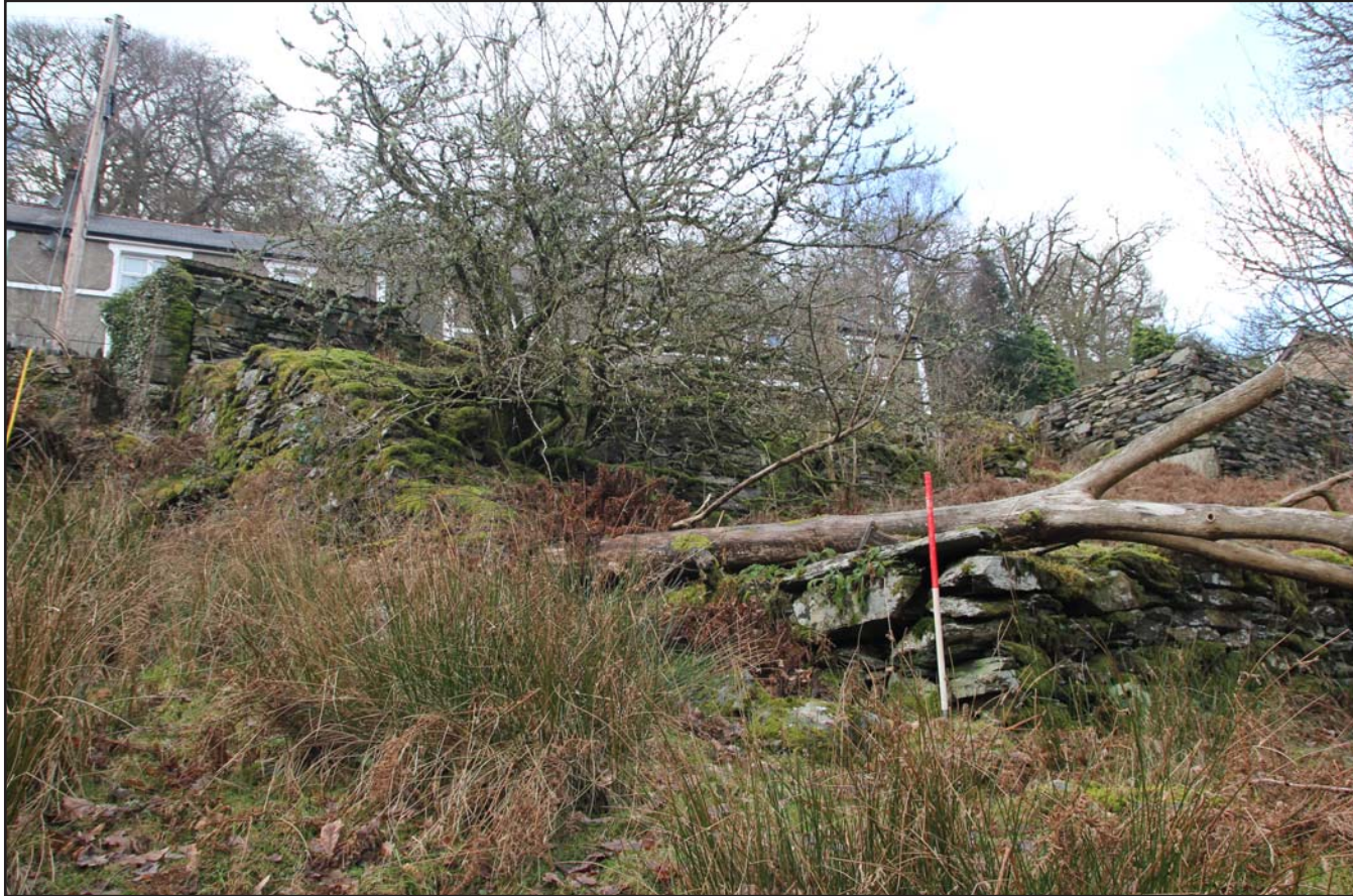
Plate 28: Incline terminus (feature 7), from the southeast. Scale 1.0m.
