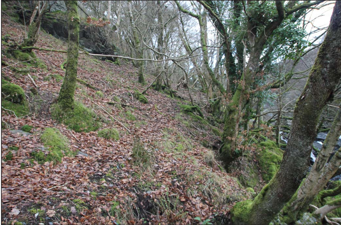
Plate 05: Proposed location of new penstock and cable tunnels terminus, from the southeast.
