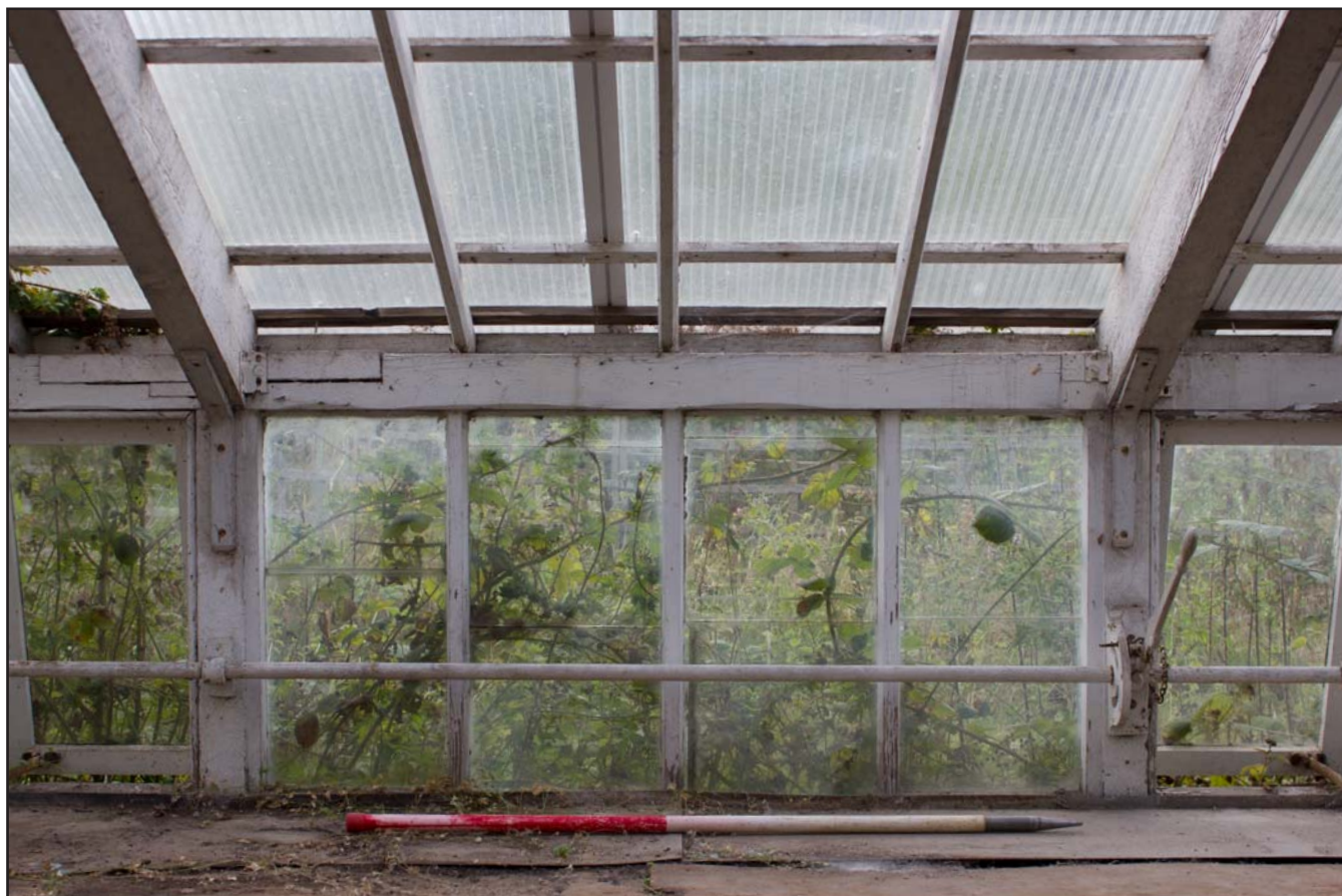
Plate 32: Example of opening casement window in North western glasshouse (showing lever mechanism), Poor Clare's Monastery, Upper Aston Hall Lane, Hawarden, Flintshire - from the northeast - scale 1m
