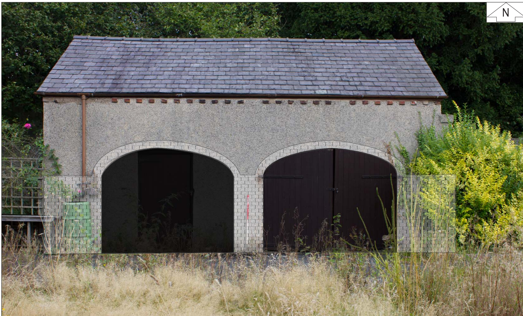
Figure 09. Mock up of the south western elevation of the Cart Shed depicting how the original facade would have appeared with two double cart doors. Scale 1m.
