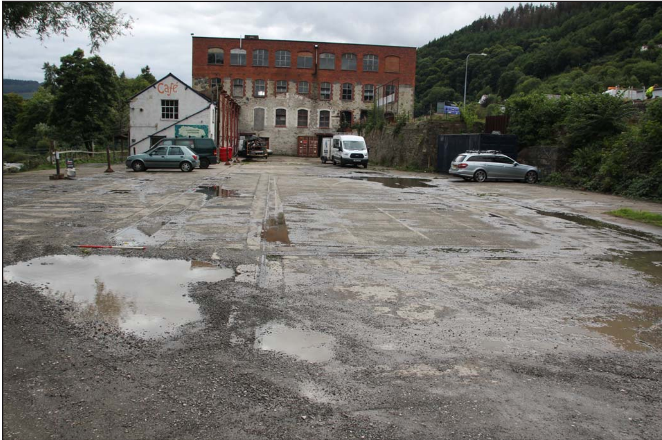
Plate 04: Mile End Mill showing narrow gauge railway tracks (feature 2), from the north. Scale 1.0m.
