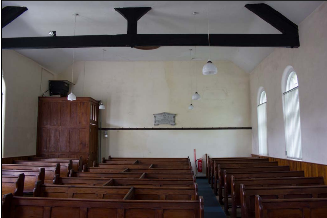
Plate 22: Ffrwd Chapel first floor chapel, from the north. Scale 1.0m.
