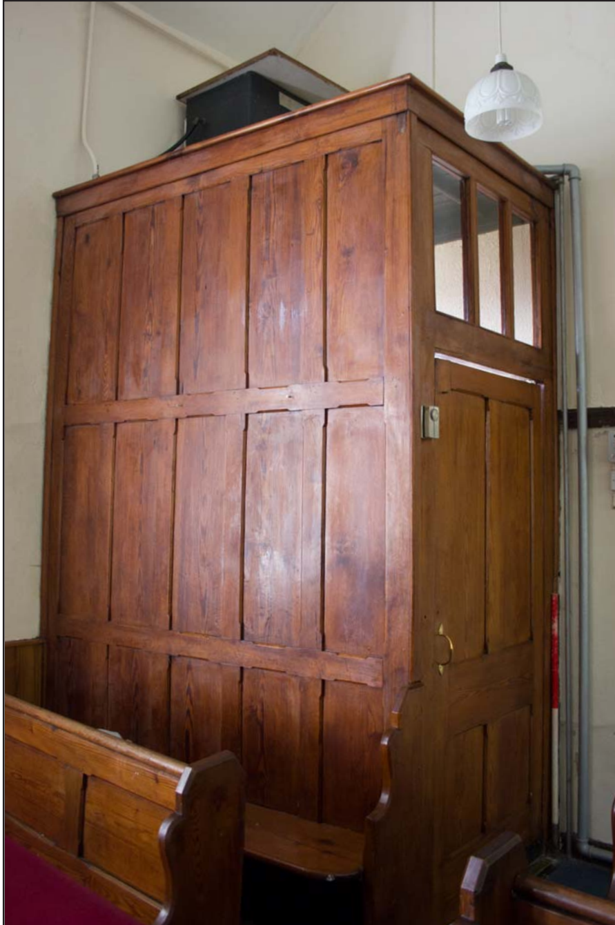
Plate 31: Ffrwd Chapel first floor chapel east elevation (south side) showing porch wood panelling, from the northwest. Scale 1.0m.
