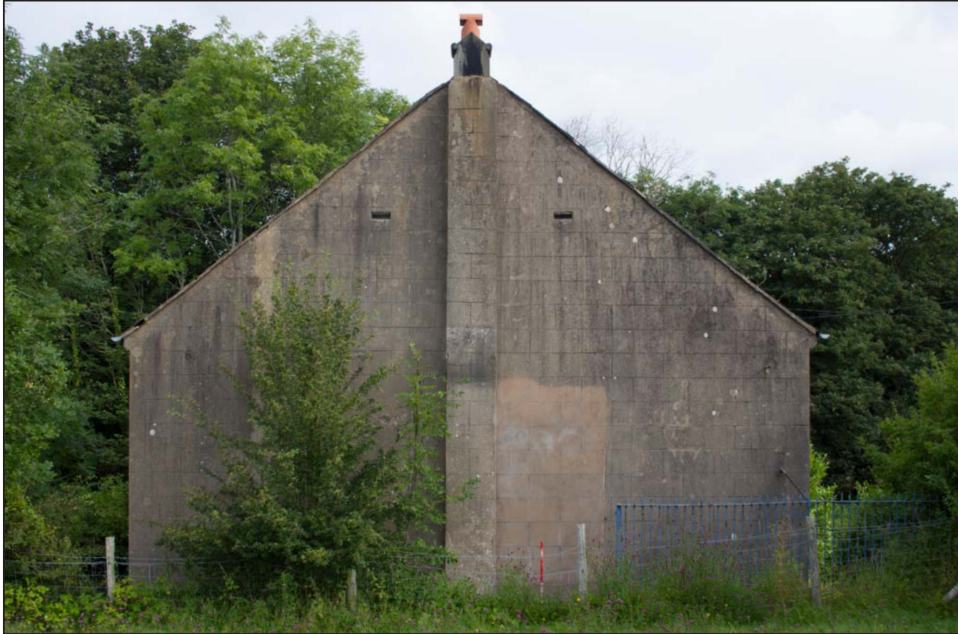
Plate 09: Ffrwd Chapel south facing external elevation, from the south. Scale 1.0m.
