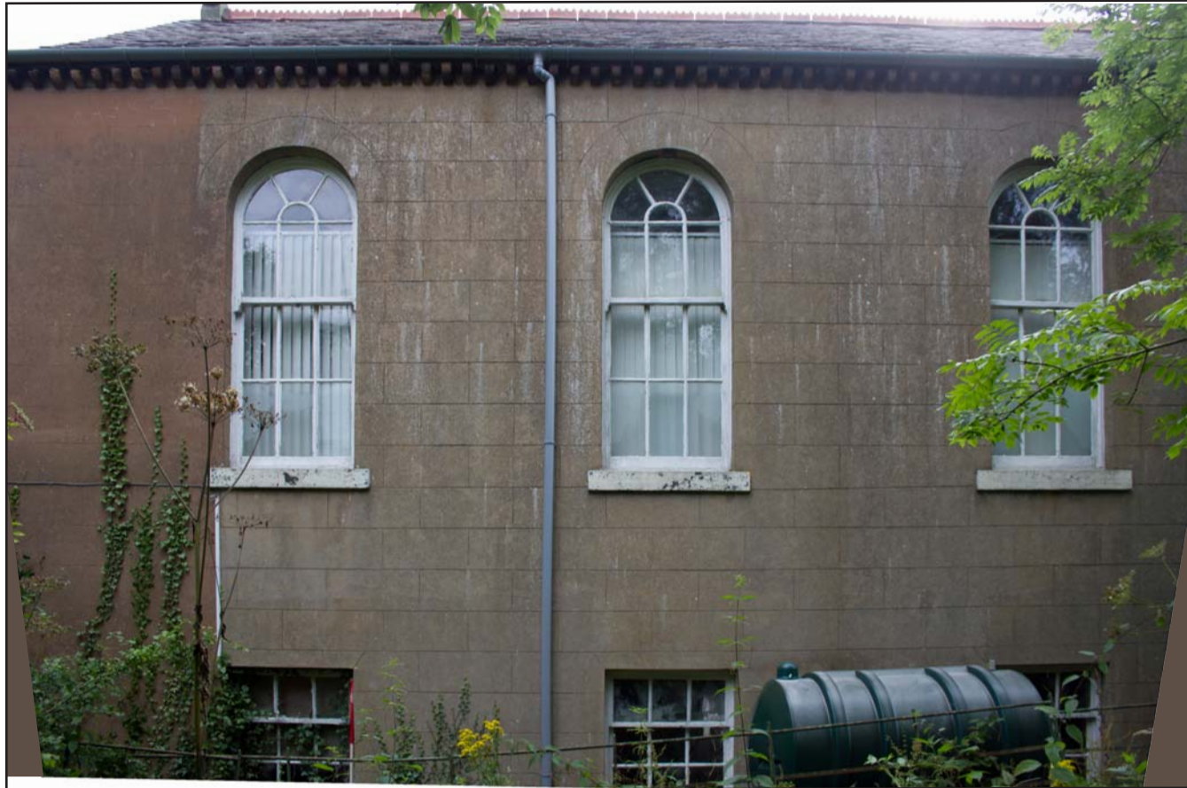
Plate 11: Ffrwd Chapel west facing external elevation, from the west.
