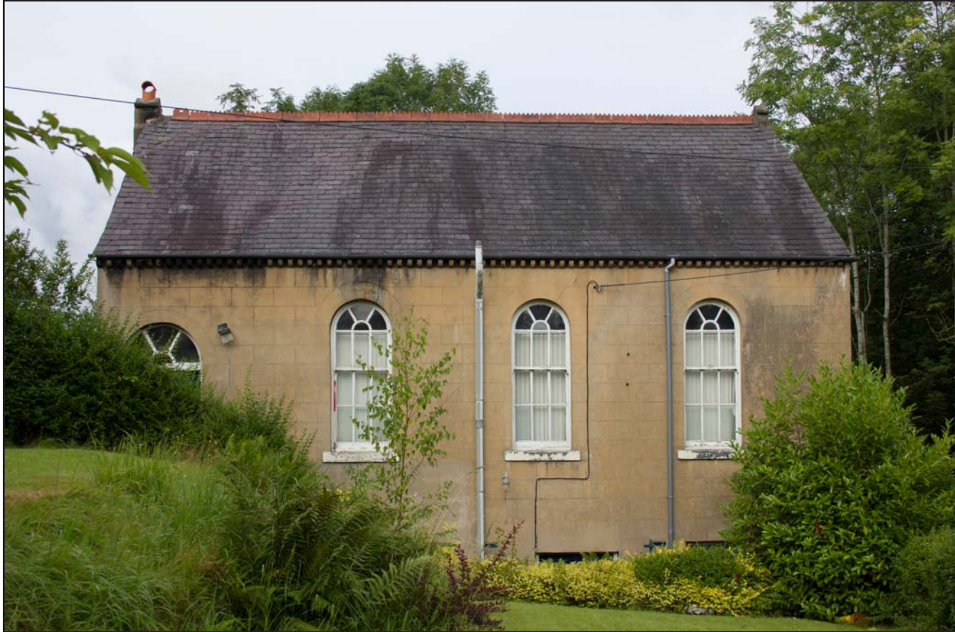
Plate 06: Ffrwd Chapel east facing external elevation, from the east. Scale 1.0m.
