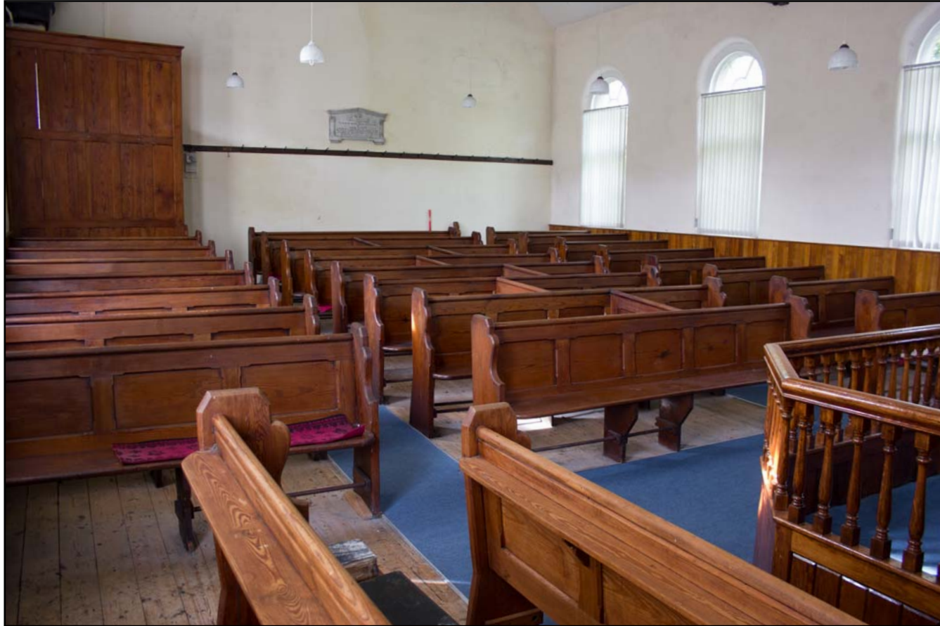
Plate 24: Ffrwd Chapel first floor chapel, from the northeast. Scale 1.0m.
