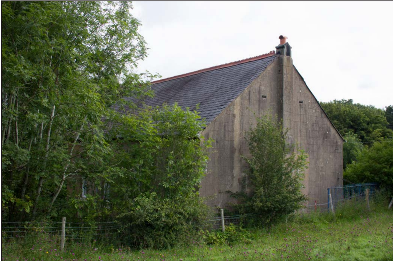
Plate 10: Ffrwd Chapel south and west facing external elevations, from the southwest. Scale 1.0m.
