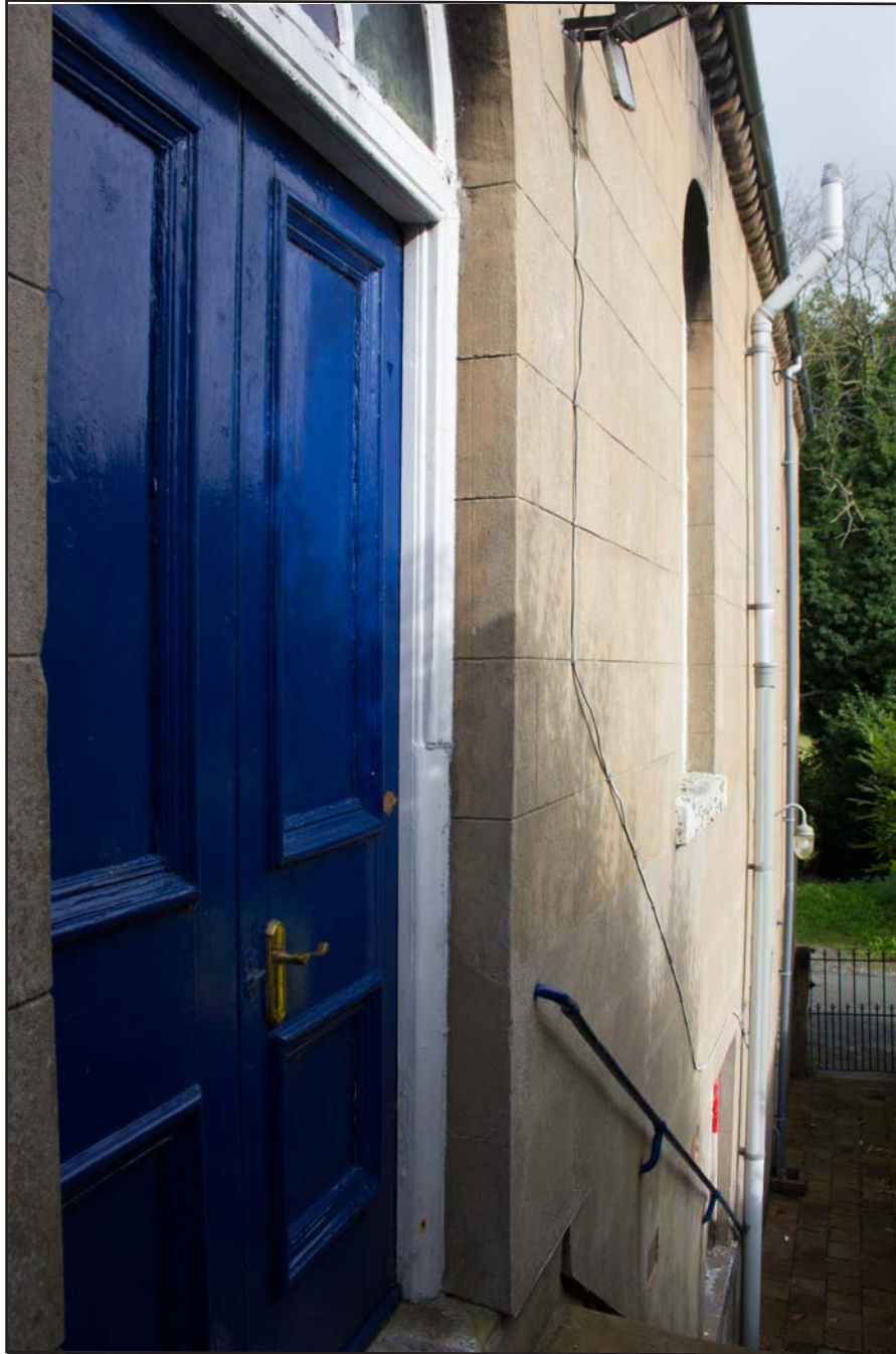
Plate 07: Ffrwd Chapel east facing external elevation, from the southeast. Scale 1.0m.
