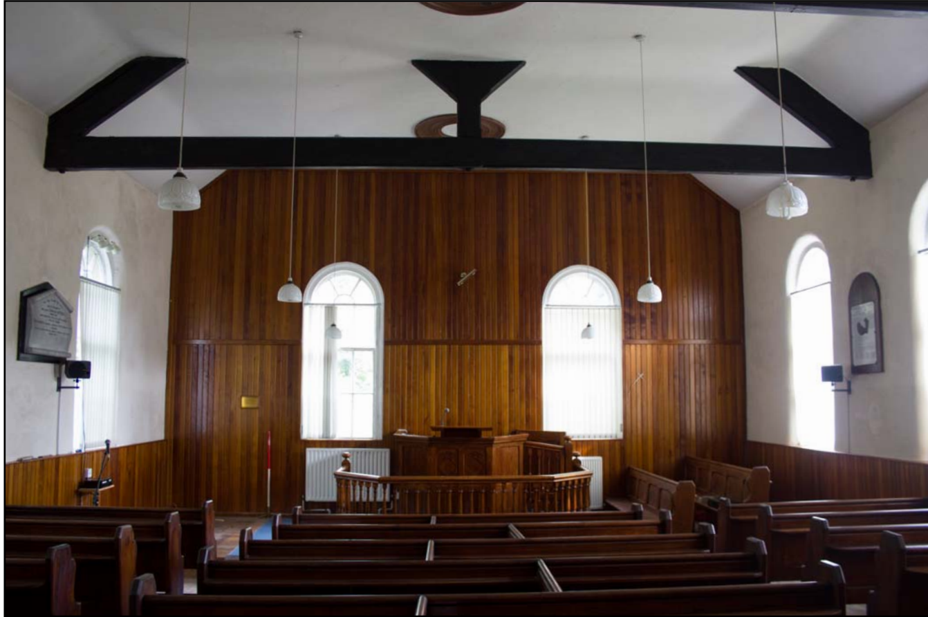
Plate 21: Ffrwd Chapel first floor chapel, from the south. Scale 1.0m.
