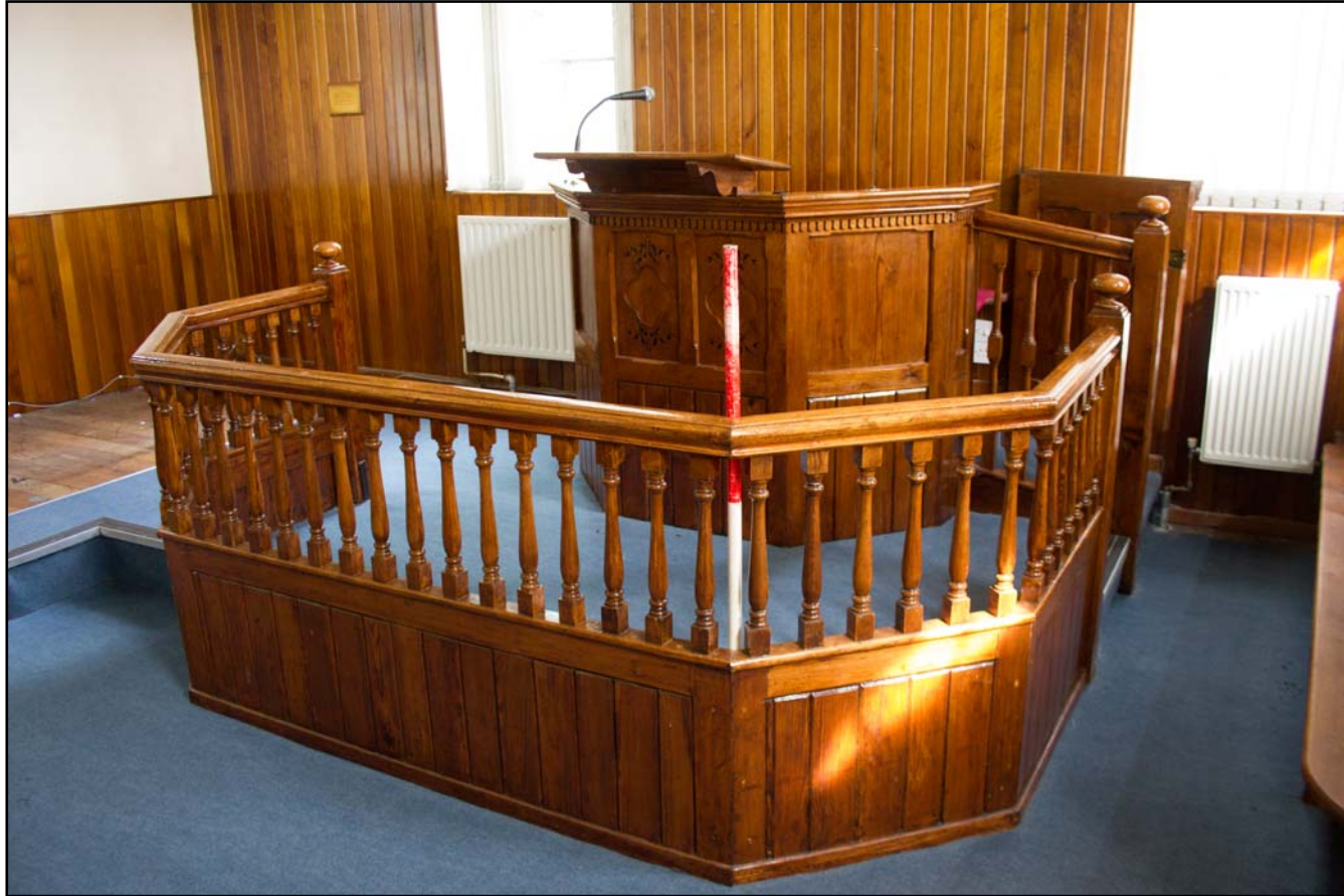
Plate 27: Ffrwd Chapel first floor chapel showing pulpit, from the southeast. Scale 1.0m.
