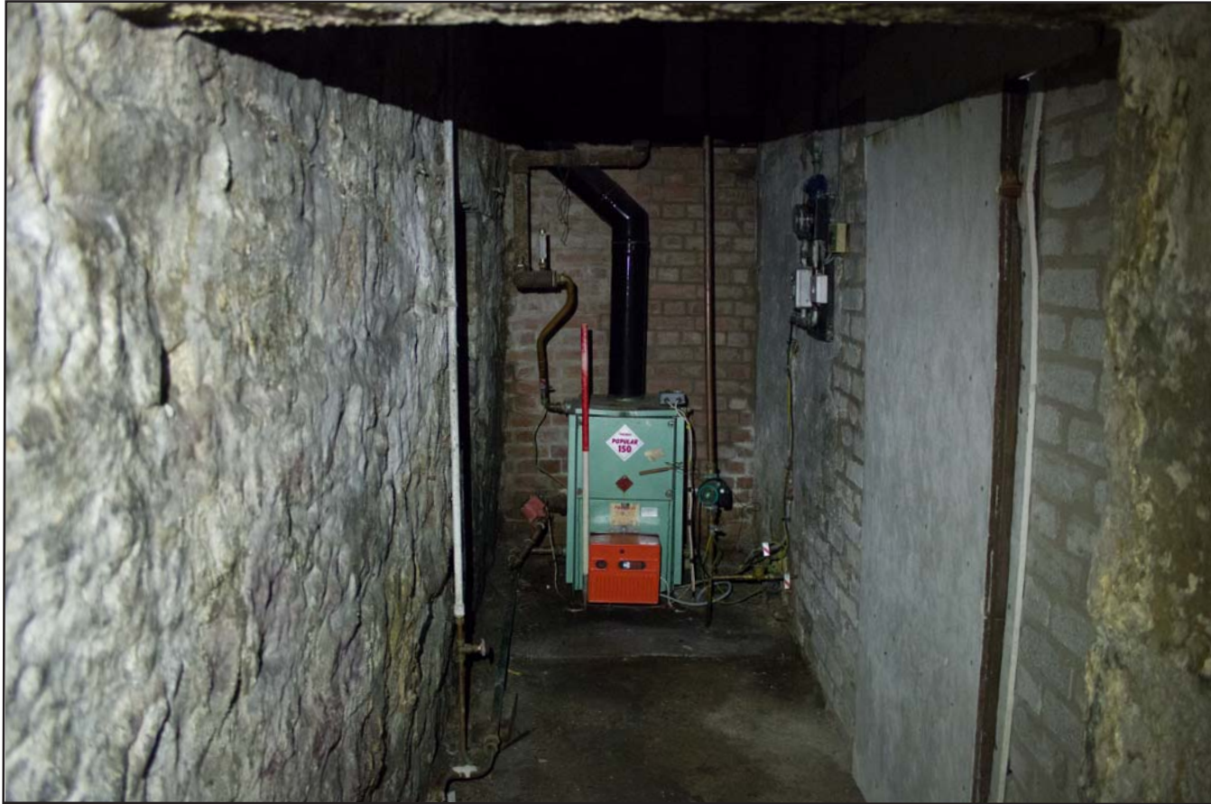
Plate 18: Ffrwd Chapel ground floor Boiler Room, from the east. Scale 1.0m.
