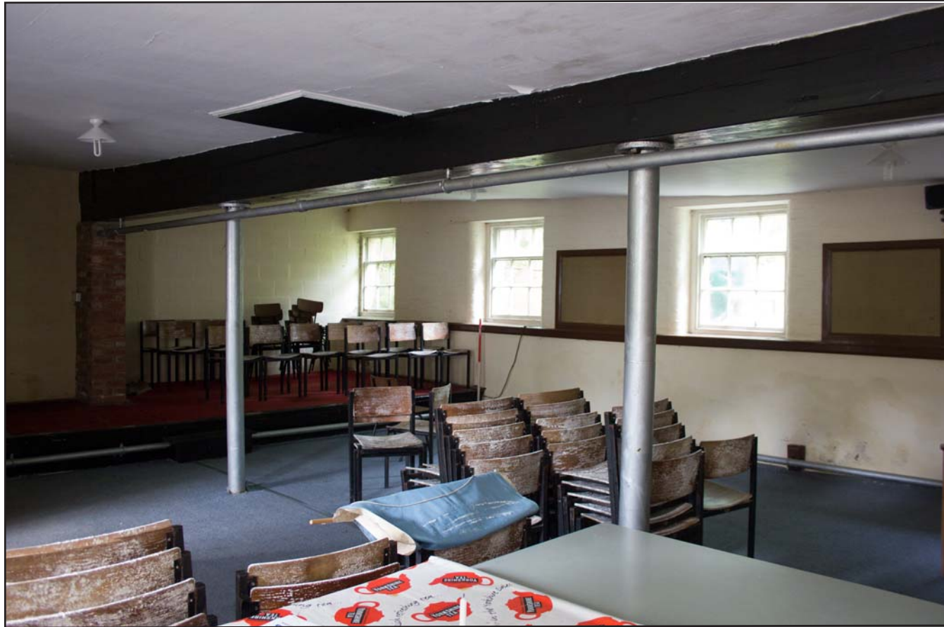
Plate 15: Ffrwd Chapel ground floor Meeting Hall, from the northeast. Scale 1.0m.
