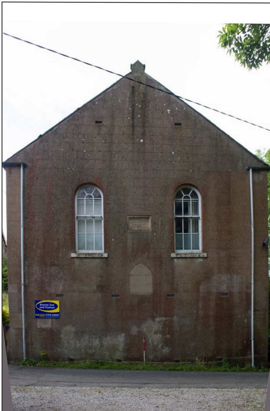
Plate 01: Ffrwd Chapel north facing external elevation, from the north. Scale 1.0m.
