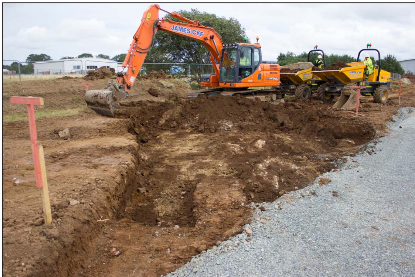
Plate 29: Reduced dig into redeposited clay layer (102) Access Road (B) estate road shot in plan, Parc Bryn Cefni, Llangefni, Ynys Môn - from the northwest - scale 1m
