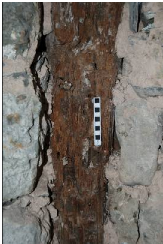
Plate 12: Pegs for a mortice and tenon joint in the external post
