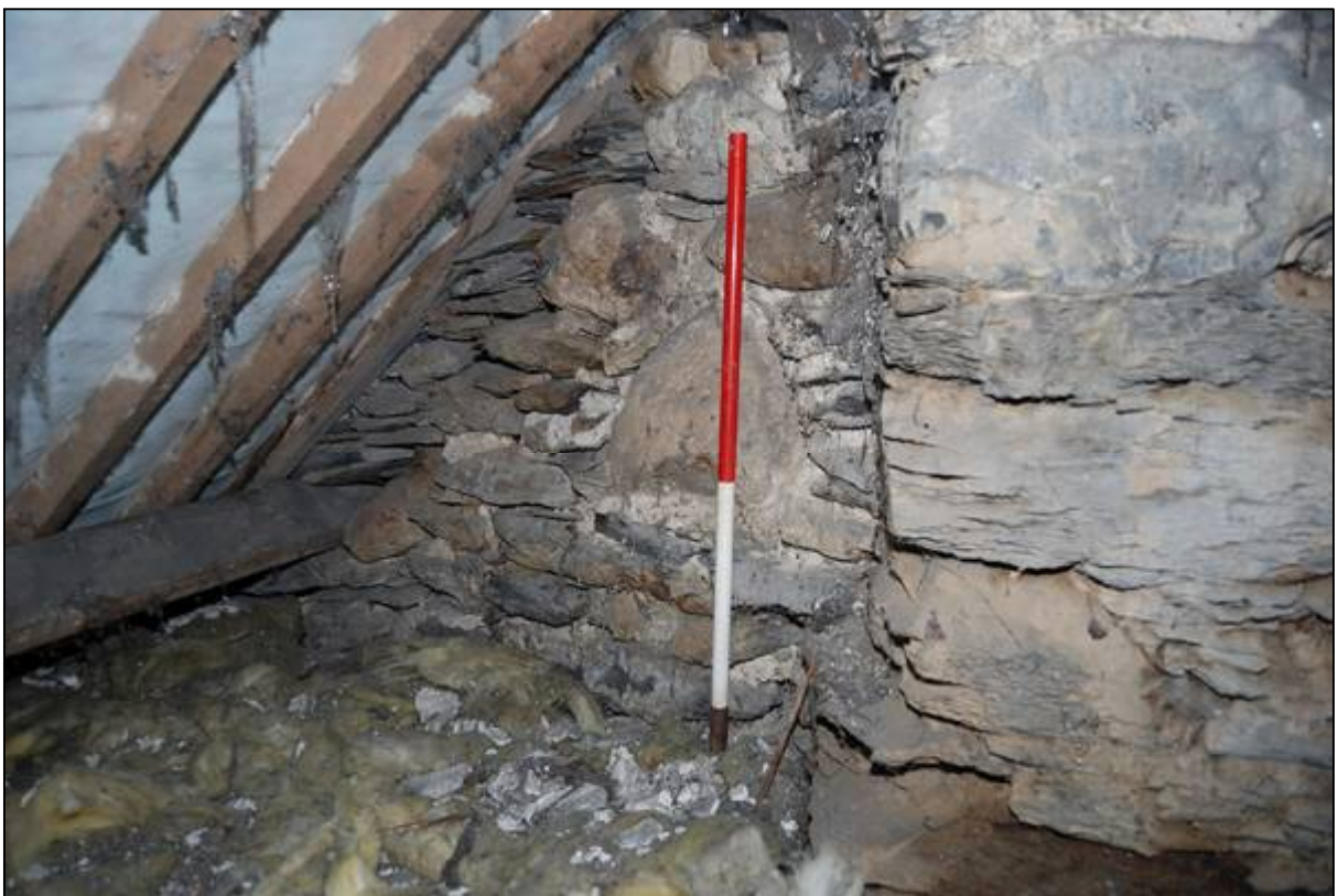
Plate 64: Diagonal wall adjacent to the northern chimney in the main range
