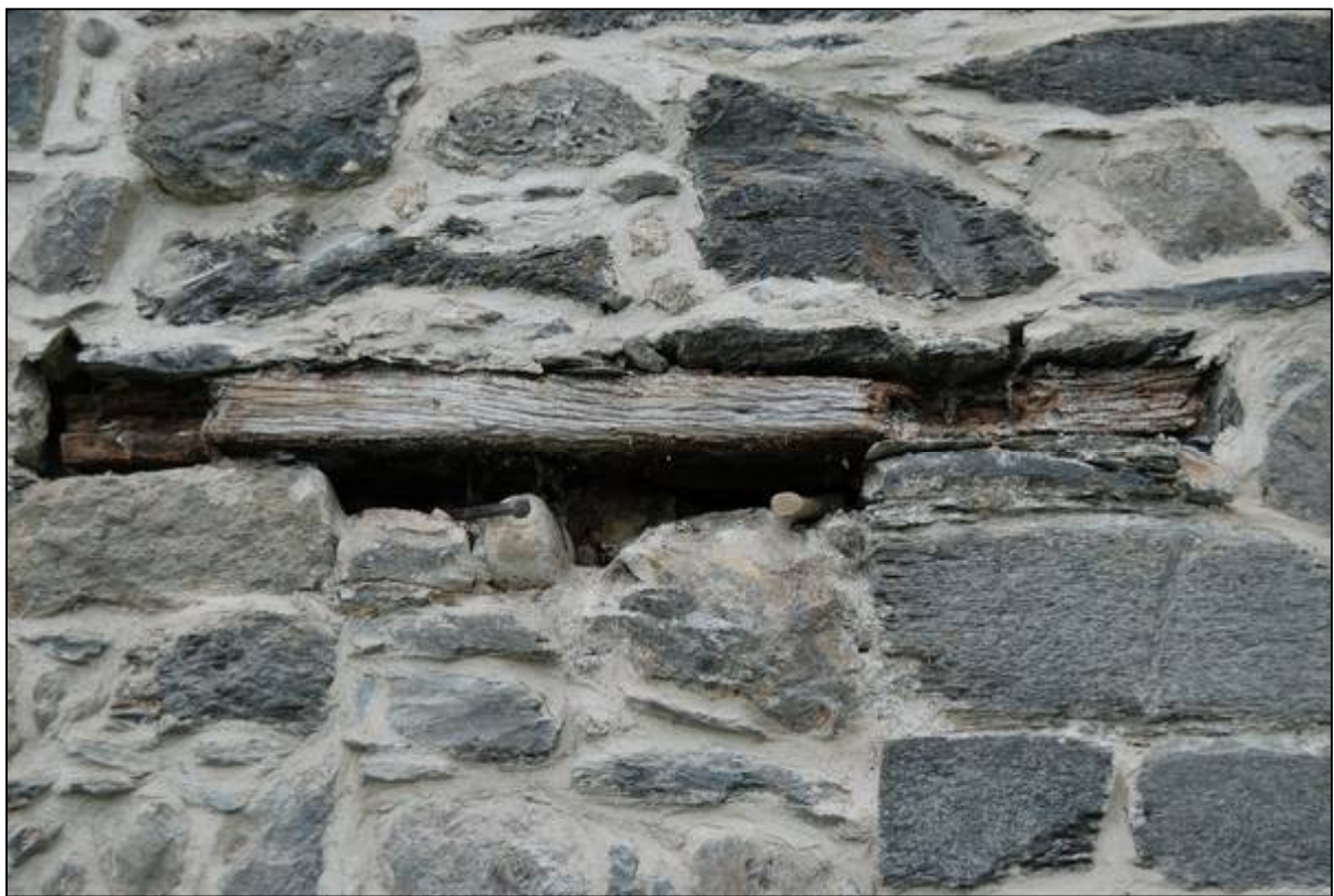
Plate 18: Lintel above the blocked doorway
