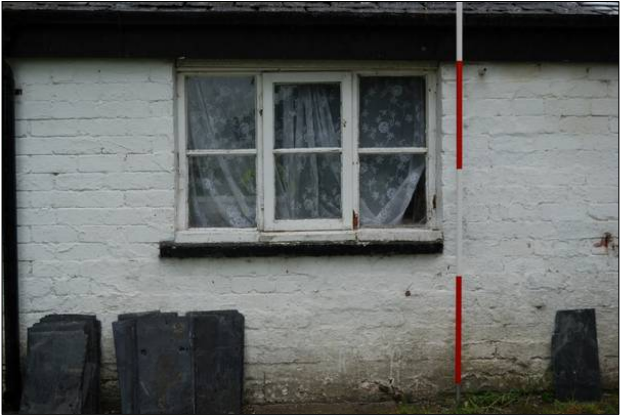
Plate 33: Detail of the scullery window
