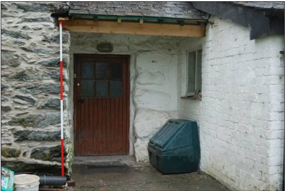
Plate 30: The kitchen door
