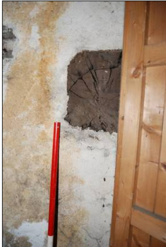
Plate 58: End of the bressumer in cupboard in Bedroom 4
