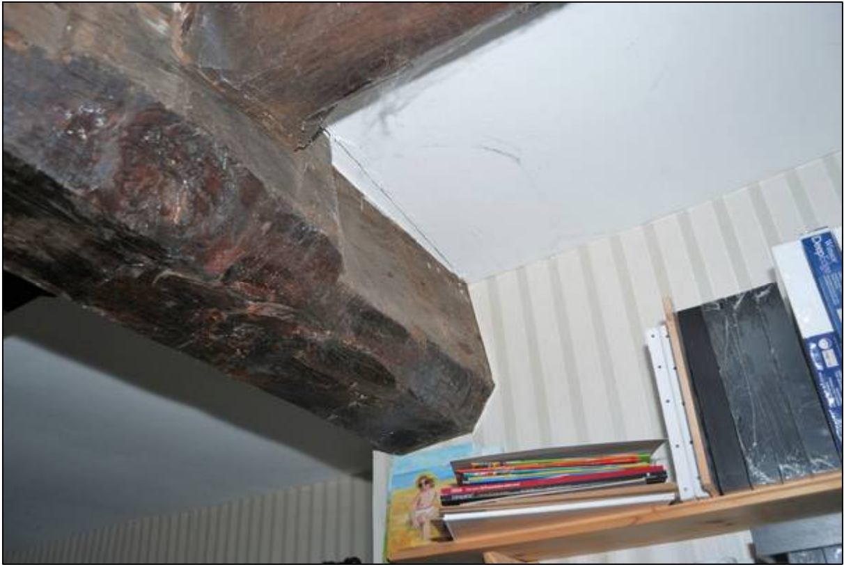
Plate 51: The reduced width of the transverse beam in the parlour
