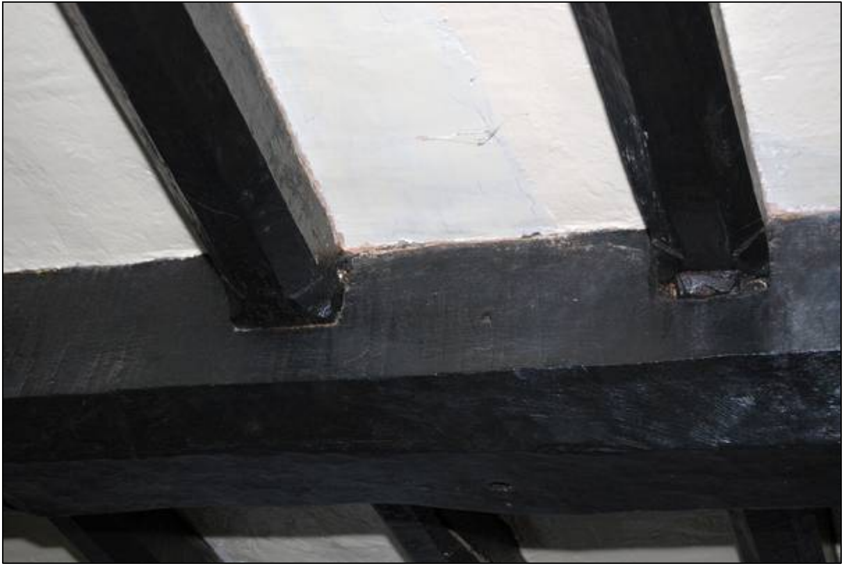
Plate 47: Joists in the hall
