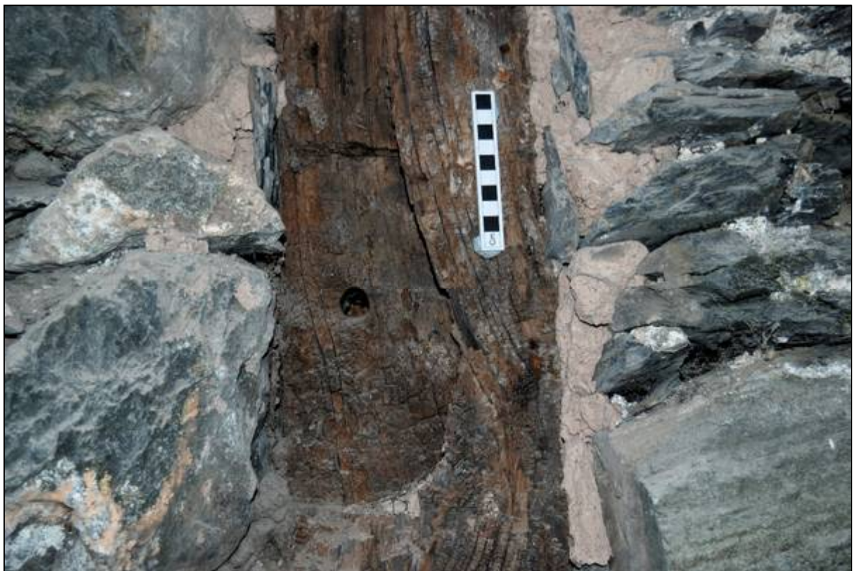
Plate 10: Mortice for a diagonal brace in the external post
