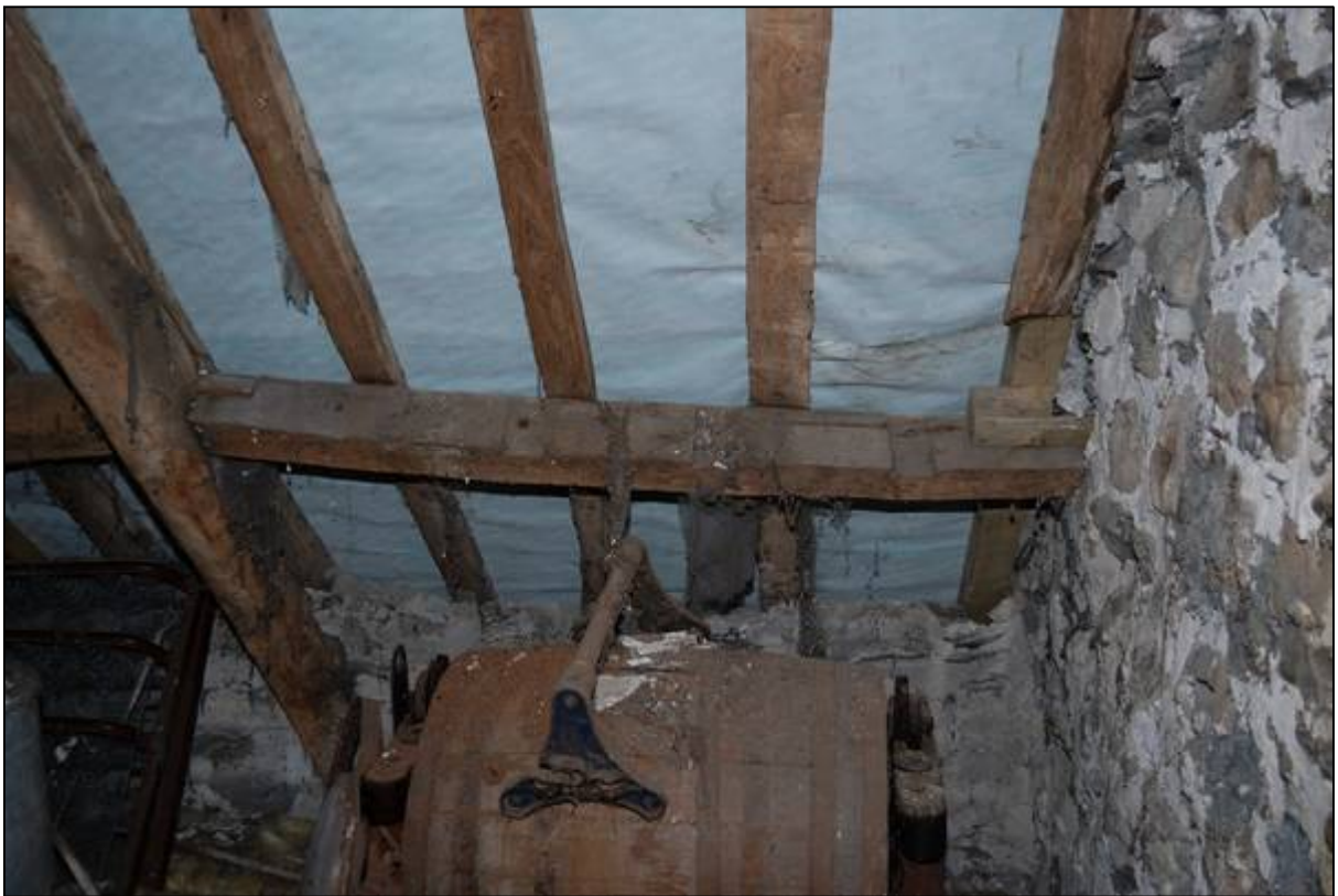
Plate 70: The replaced segment of the lower southern purlin
