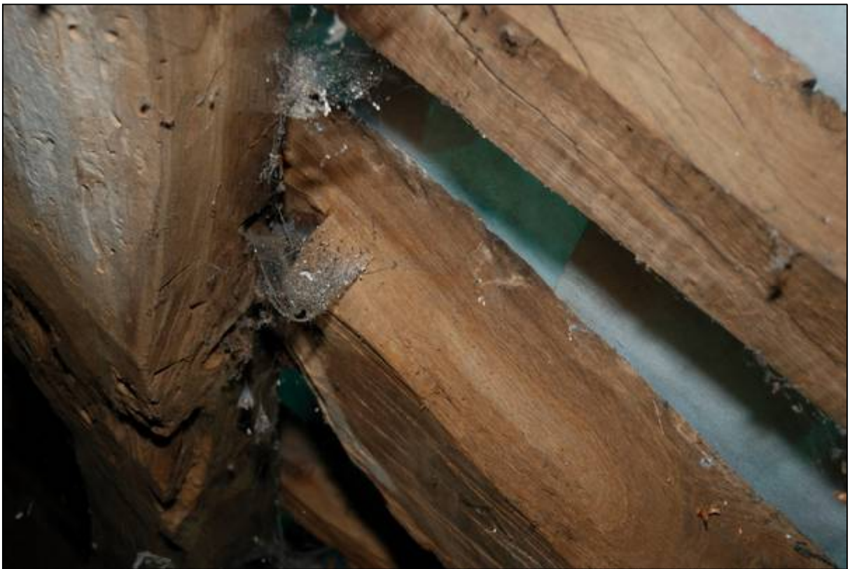
Plate 72: Relationship between the enlarged rafter and the top purlin
