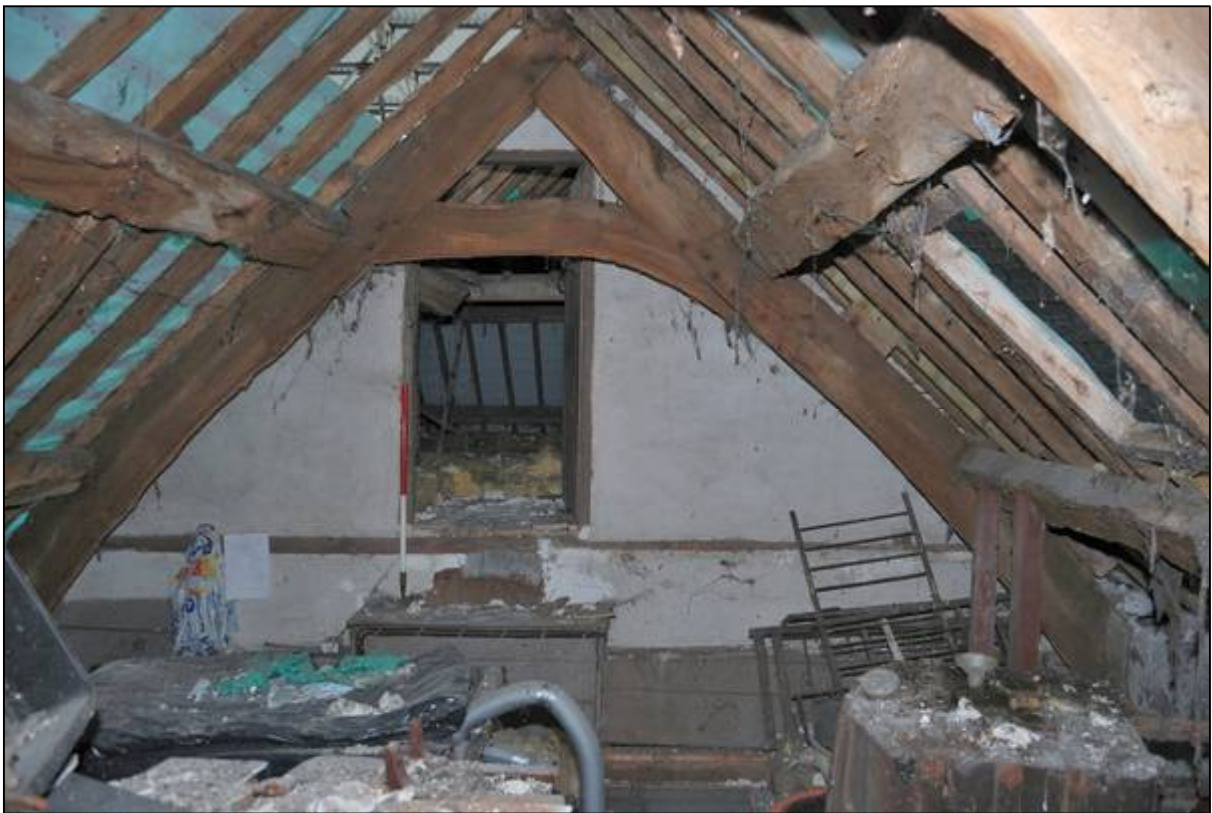
Plate 66: Truss 2 looking east
