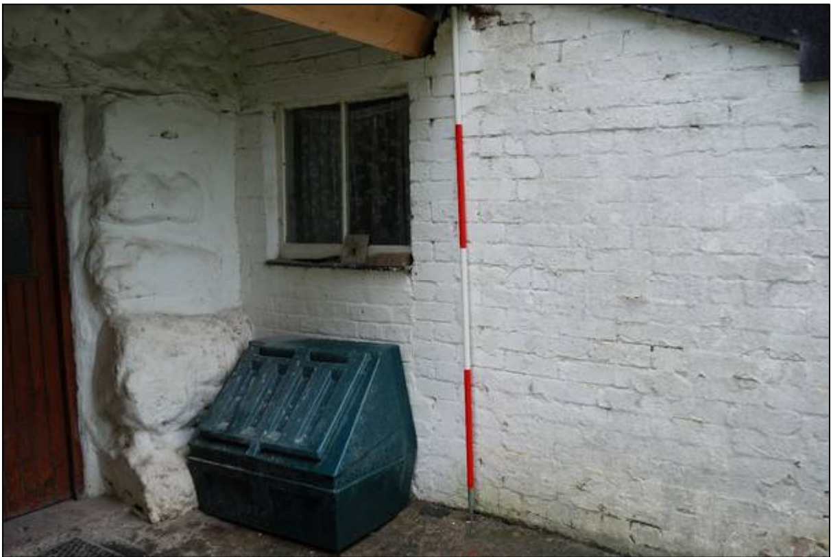
Plate 32: Blocked doorway in the scullery
