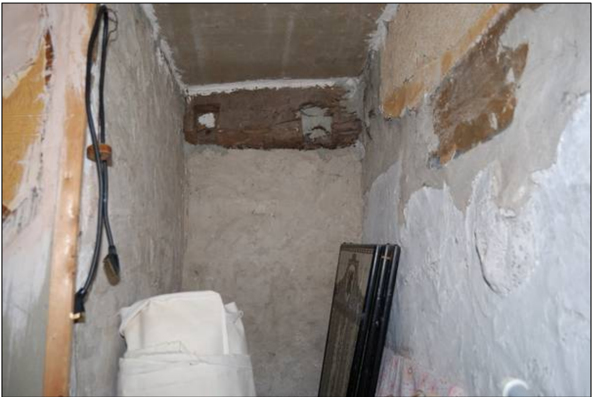
Plate 48: Beam exposed in the below stairs cupboard
