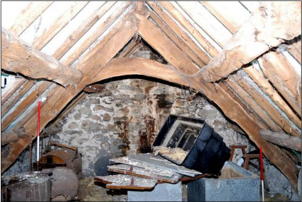
Plate 67: Truss 1, looking west
