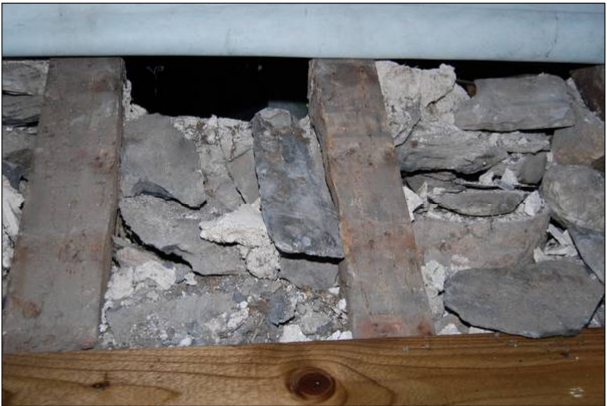
Plate 28: Moss slates resting on top of the wall of the “Kitchen Range”
