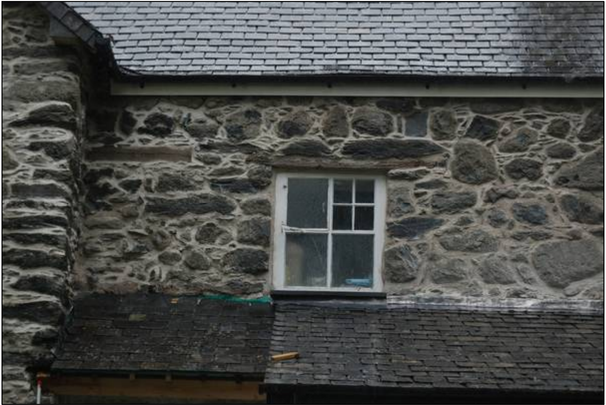
Plate 23: First floor window in the northern elevation of the “Kitchen Range”
