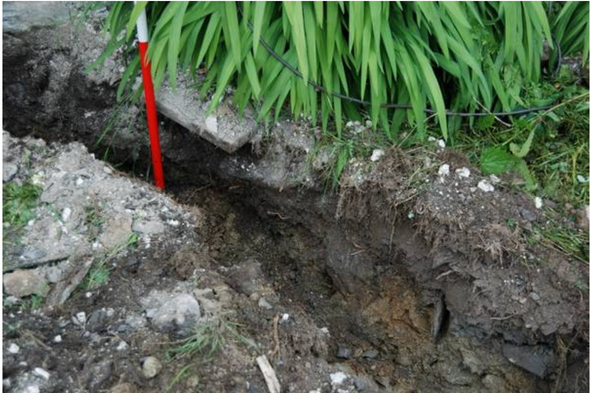
Plate 73: Context 3, foundation trench for the house
