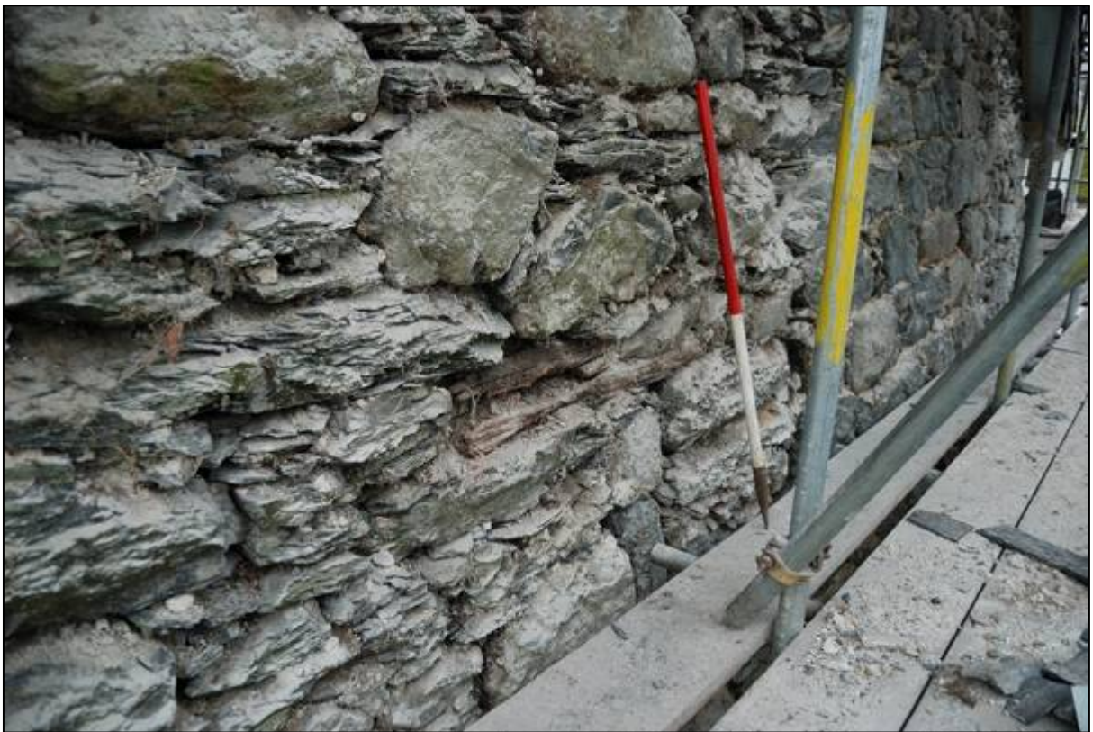
Plate 22: Timber in the northern gable of the main range
