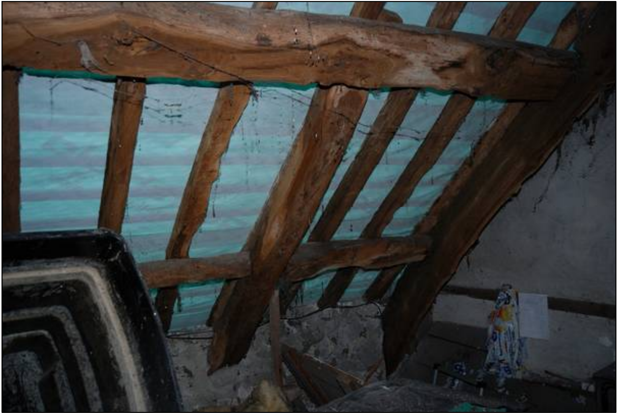
Plate 71: Possible fragment of a truss in the kitchen range
