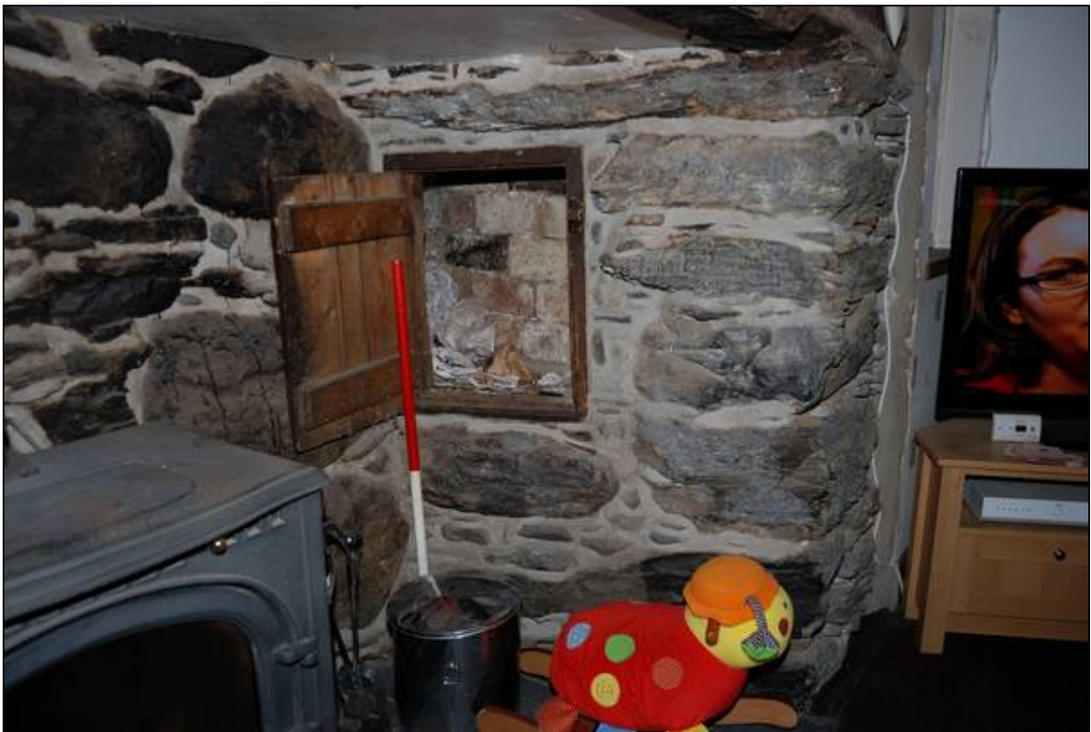
Plate 42: Opening in the side of the hearth
