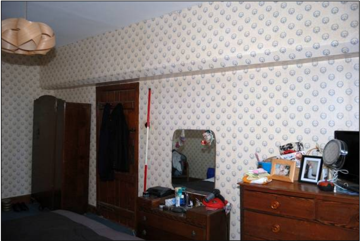
Plate 55: Probable transverse beam in Bedroom 1
