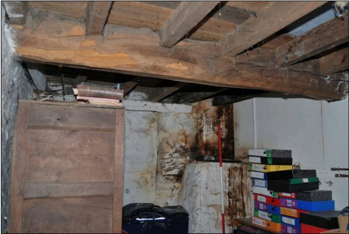
Plate 61: Beam in the store room
