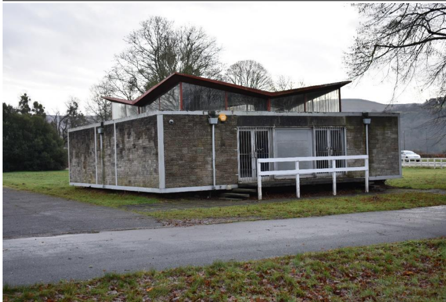
Fig. 15 Building 1 – Museum, Phase 3. Photo CPAT 4720-0004
