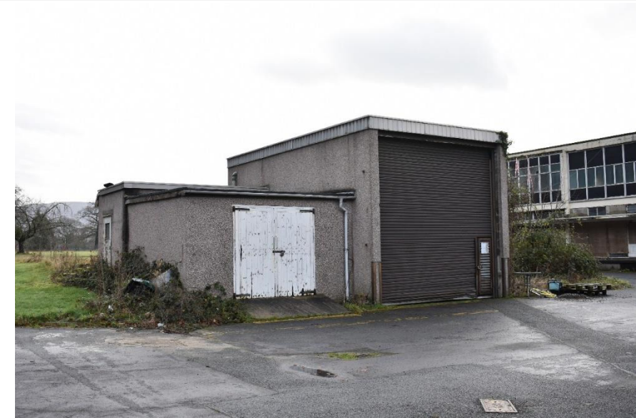
Fig. 29 Building 15 – Store, Phase 3. Photo CPAT 4720-0023
