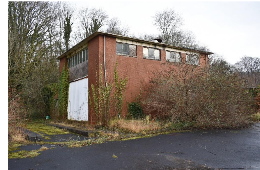
Fig. 20 Building 6 – Boiler House, Phase 3. Photo CPAT 4720-0029
