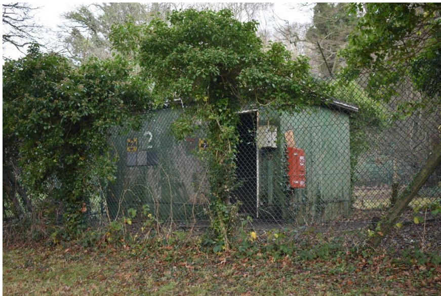
Fig. 30 Building 16 – Ammo Store, Phase 3. Photo CPAT 4720-0025
