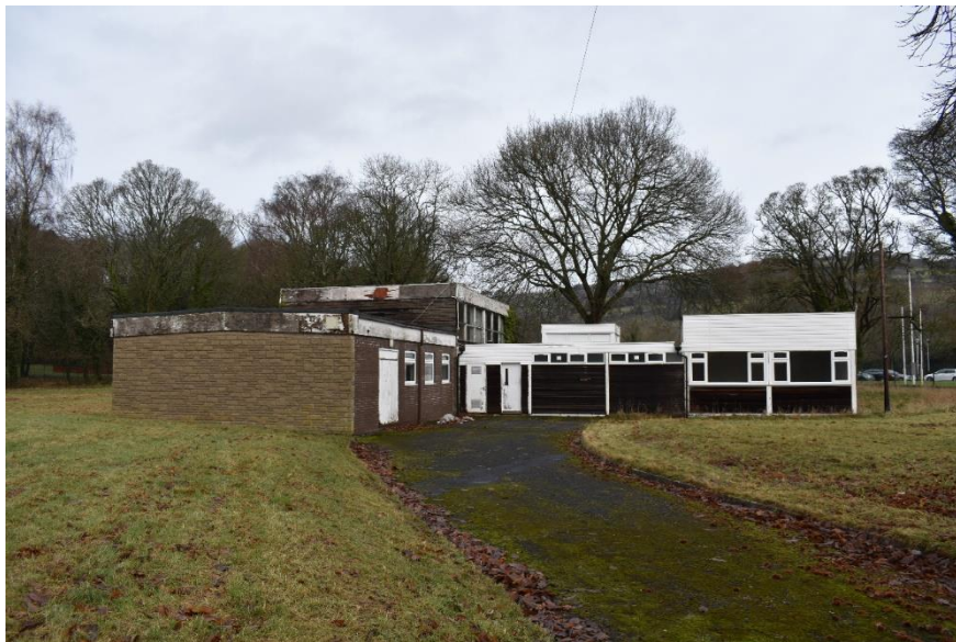
Fig. 24 Building 10 – Hang Gliding Centre, Phase 4. Photo CPAT 4720-0043
