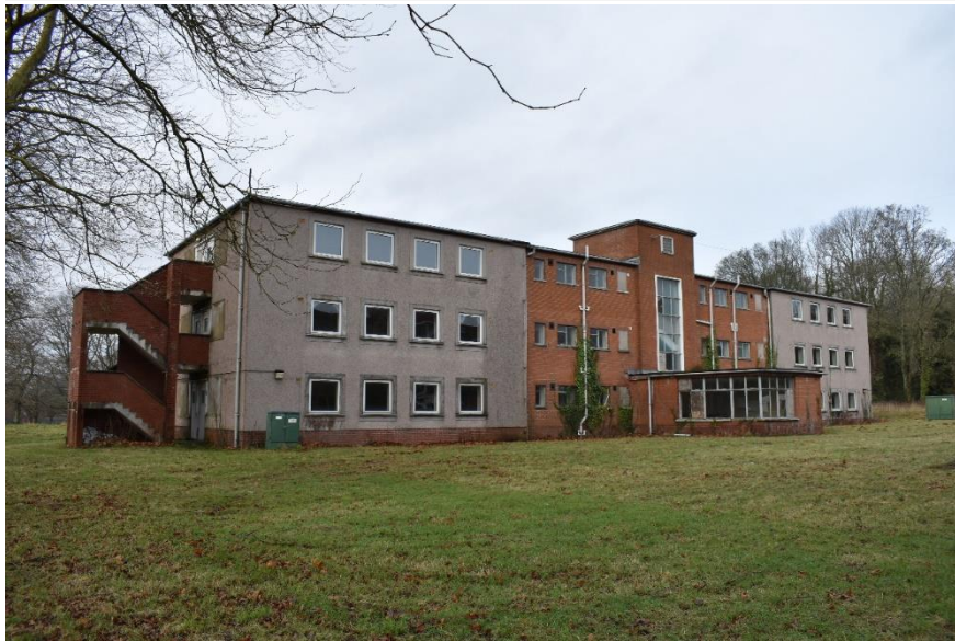
Fig. 21 Building 7 – Accommodation Block, Phase 3. Photo CPAT 4720-036
