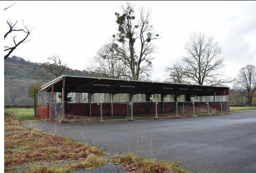
Fig. 16 Building 2 – Review Shelter, Phase 2? Photo CPAT 4720-0006
