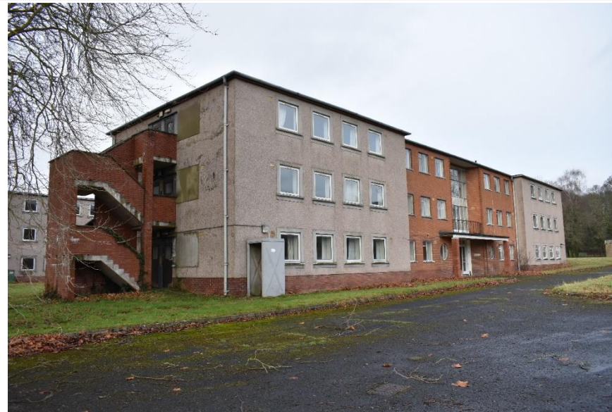
Fig. 22 Building 8 – Accommodation Block, Phase 3. Photo CPAT 4720-0038
