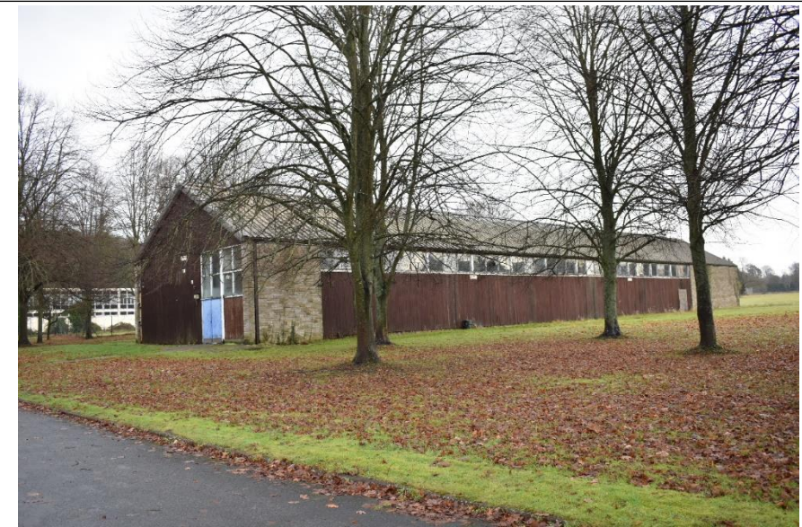
Fig. 17 Building 3 – Gymnasium, Phase 3. Photo CPAT 4720-0010
