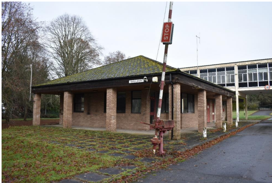
Fig. 18 Building 4 – Guard Room, Phase 4. Photo CPAT 4720-0017
