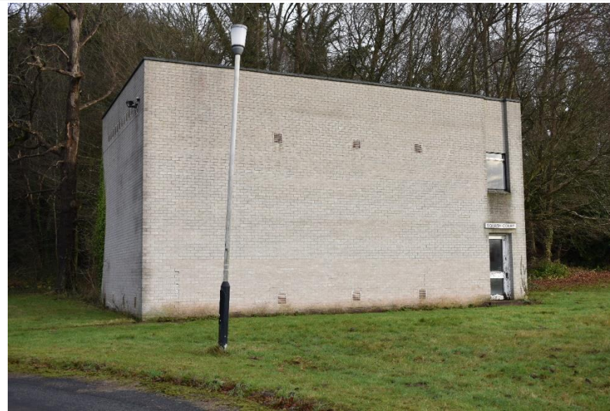
Fig. 28 Building 14 – Squash Court, Phase 4. Photo CPAT 4720-0027
