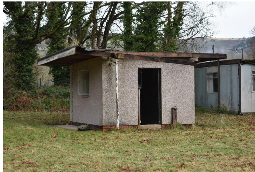
Fig. 25 Building 11 – ‘Gas Chamber’, Phase 4. Photo CPAT 4720-0045
