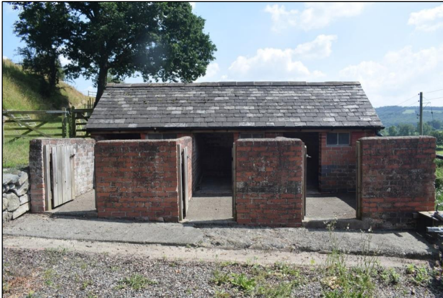
Fig. 3 Pigsty, viewed from the west Photo CPAT 4935-003
