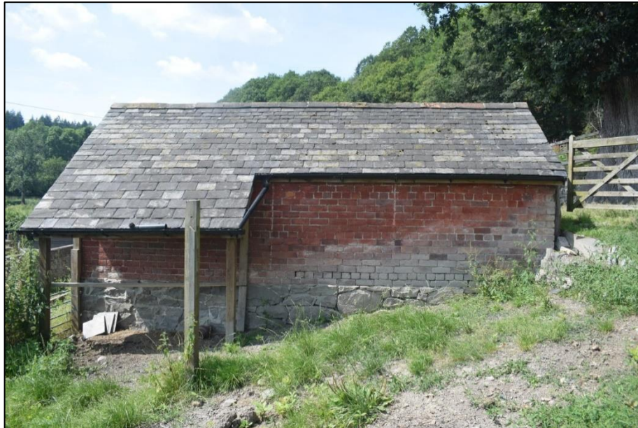
Fig. 4 East elevation of the pigsty Photo CPAT 4935-006
