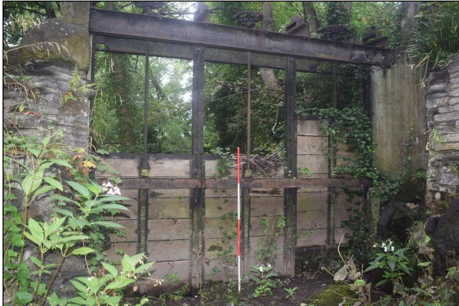
Fig. 9 The sluice gate, viewed from the east Photo CPAT 4948-013
