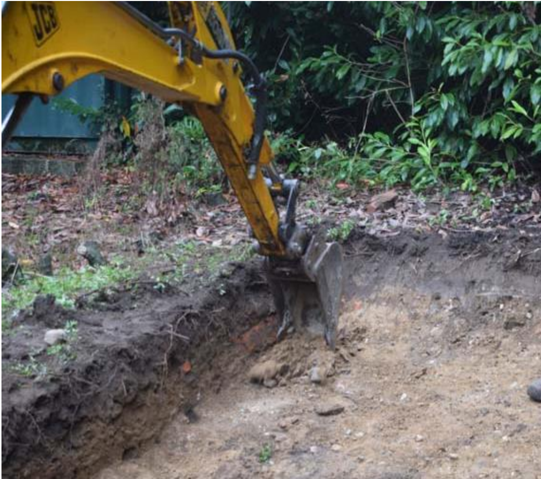
Figure 6 toothed bucket penetrating compact layer beneath brick surface. Photo CPAT 4954-0006
