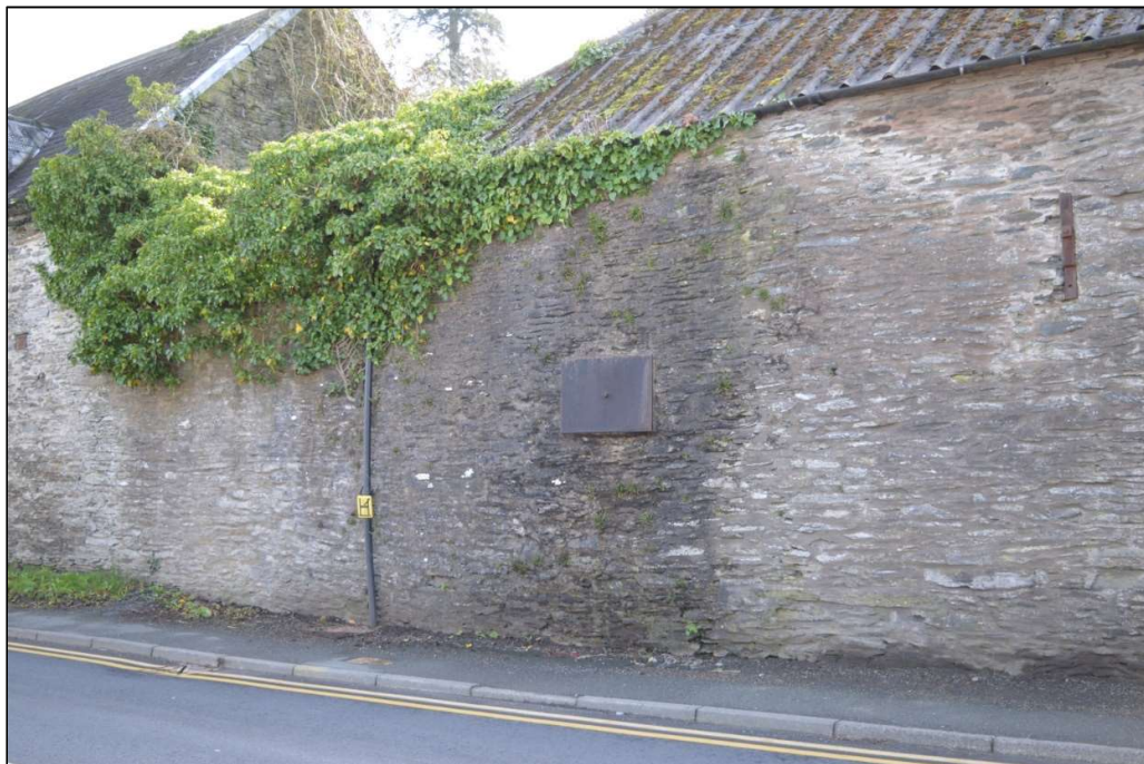
Fig. 15: Two examples showing where iron bars have been inserted to tie the wall, here bowed outwards, to the rest of the building. Taken from the west. CPAT 4902-0053
