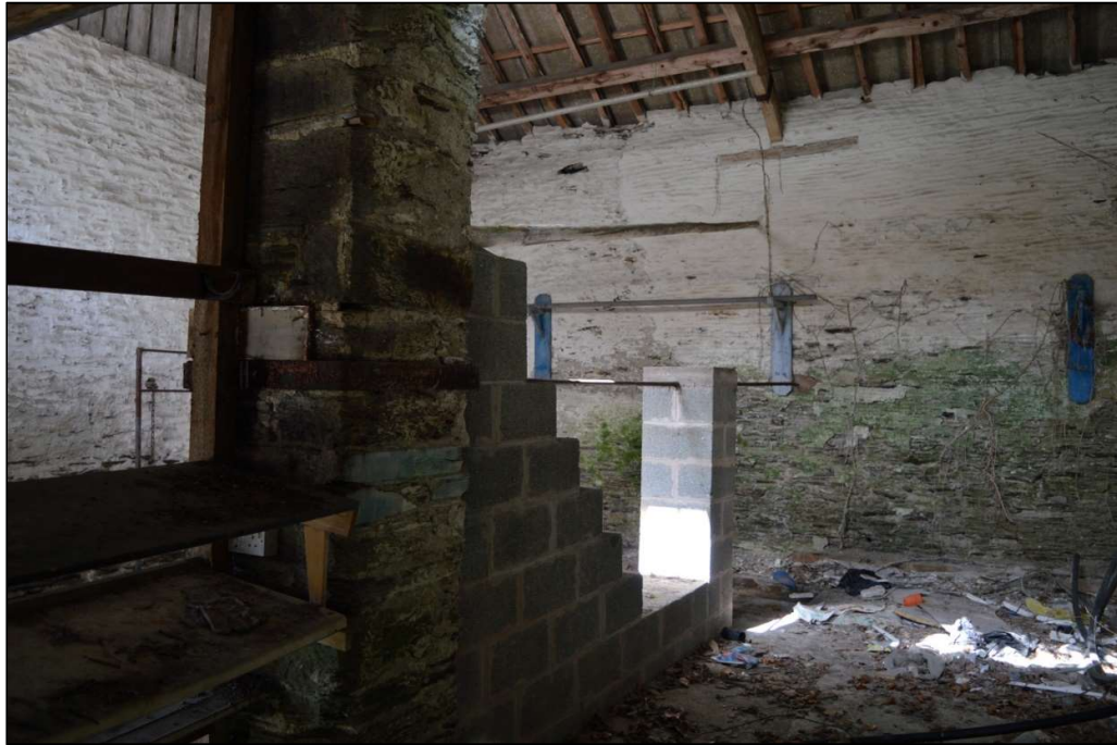
Fig. 16: The two open bays at the north-east end of the building, showing the inserted iron bar and block-built structure. CPAT 4902-0058
