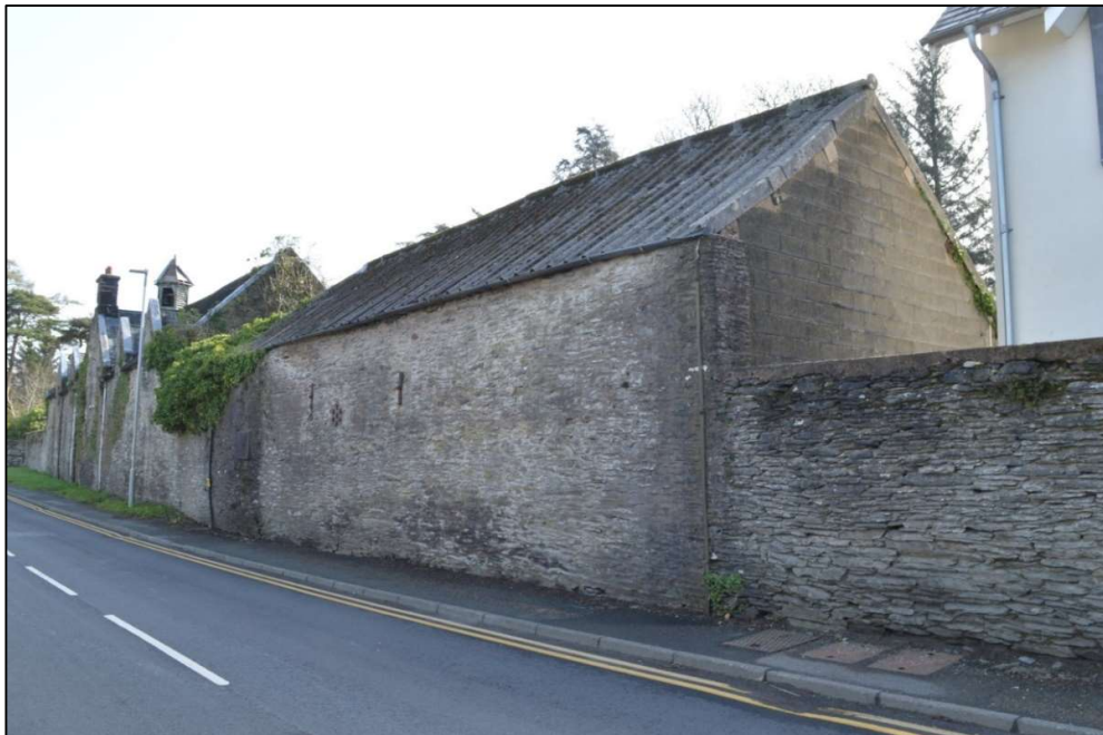
Fig. 10: The building from the west, showing the modern block wall where the south-west end has been removed. CPAT 4902-0045
