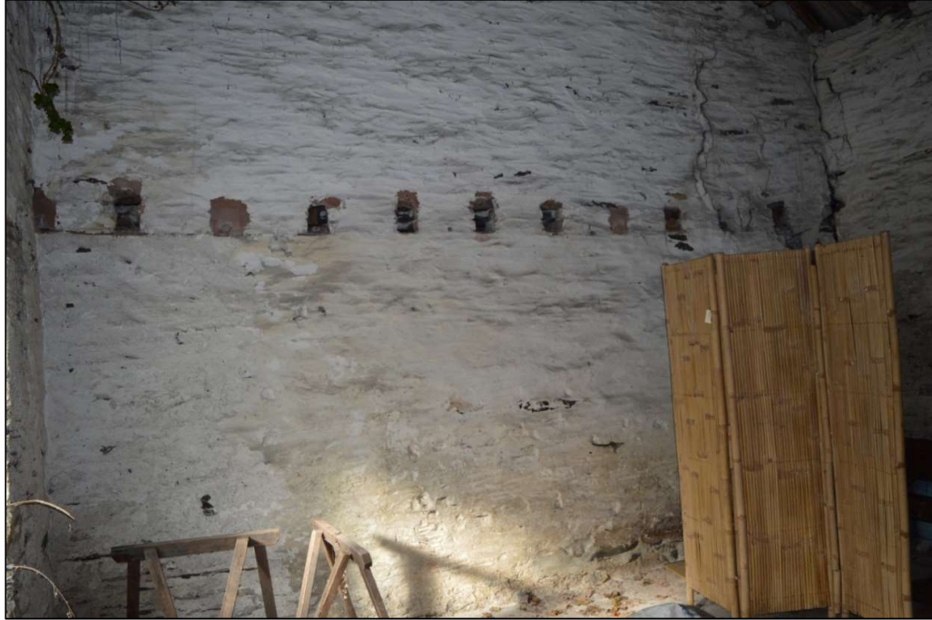
Fig. 11: The slots for timber joists on the inside of the south-west wall of the building indicating that there had been a first floor room. CPAT 4902-0011
