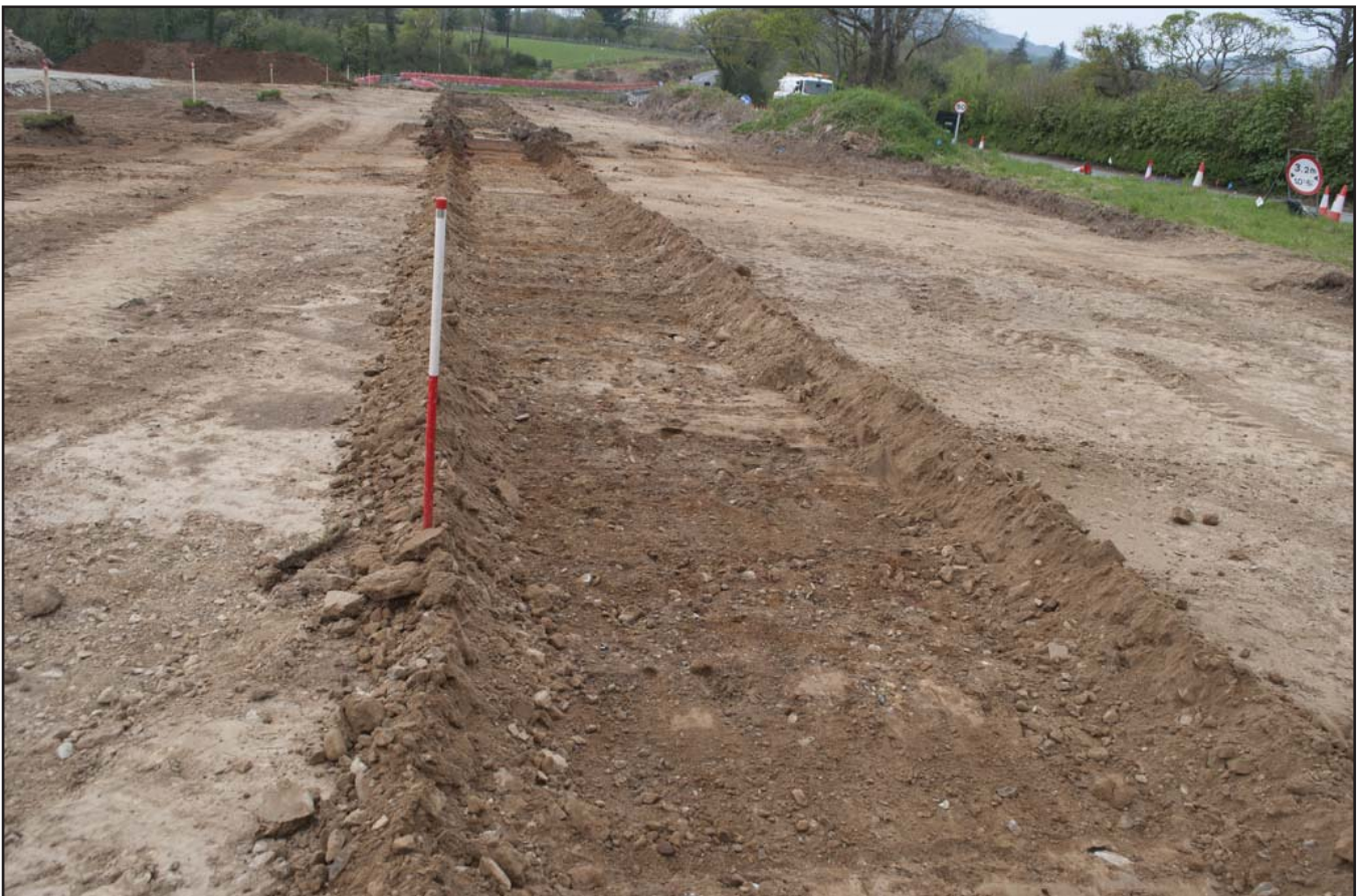
Plate 12: General view along trench showing the former gravel pit (PRN90073; Feature 1); scale 1x1m; view from SW (archive reference: G2716_014).
