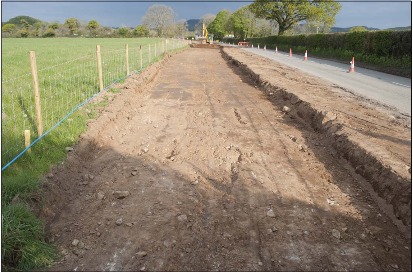
Plate 11: View of topsoil stripping of the Efailnewydd link road section; scale not used; view from SW (archive reference: G2716_011).
