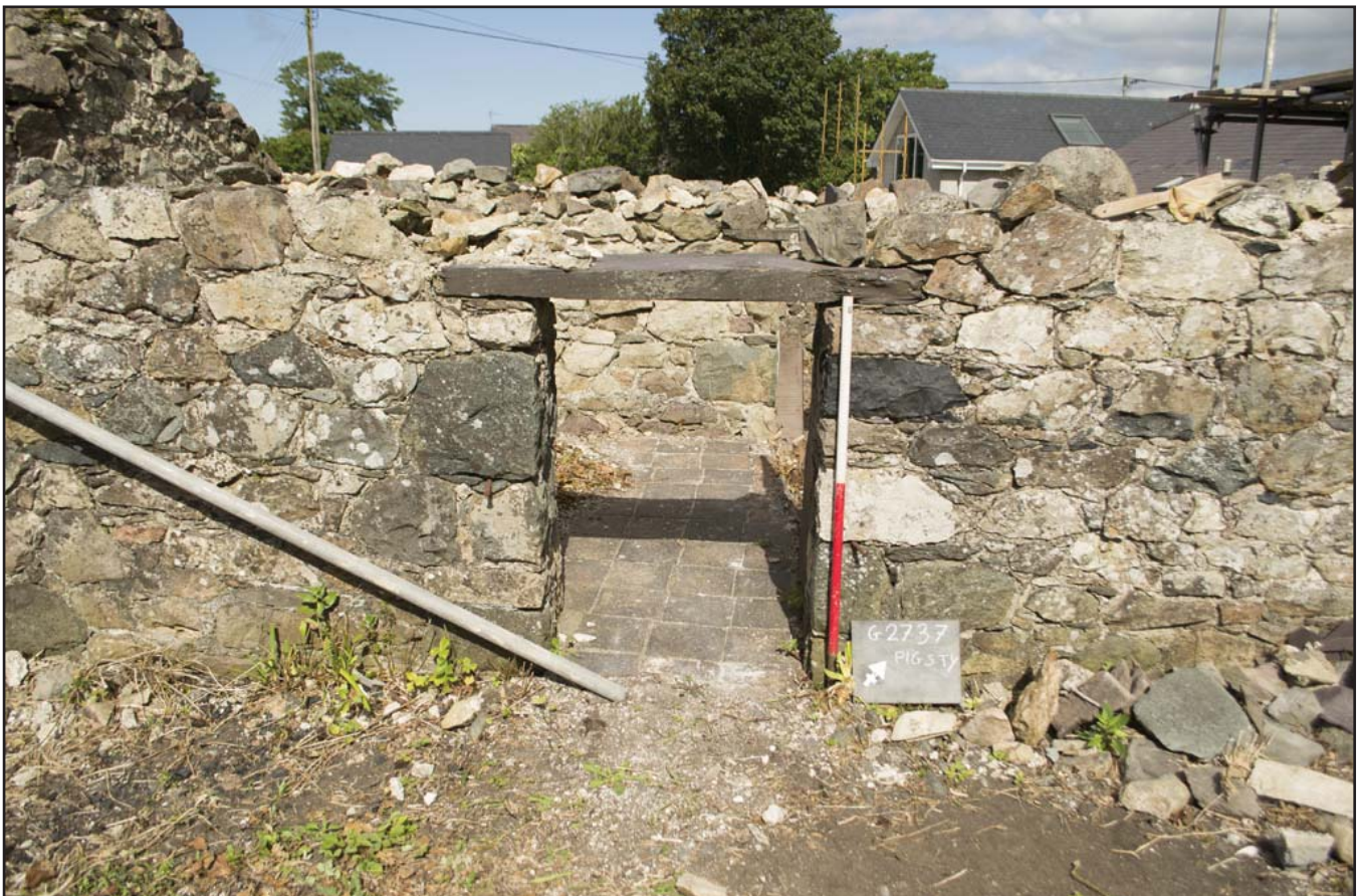
Plate 10: View of doorway with slate slab lintel between Rooms 2 and 3; scale 1x1m; view from ESE (archive reference: G2736_014).
