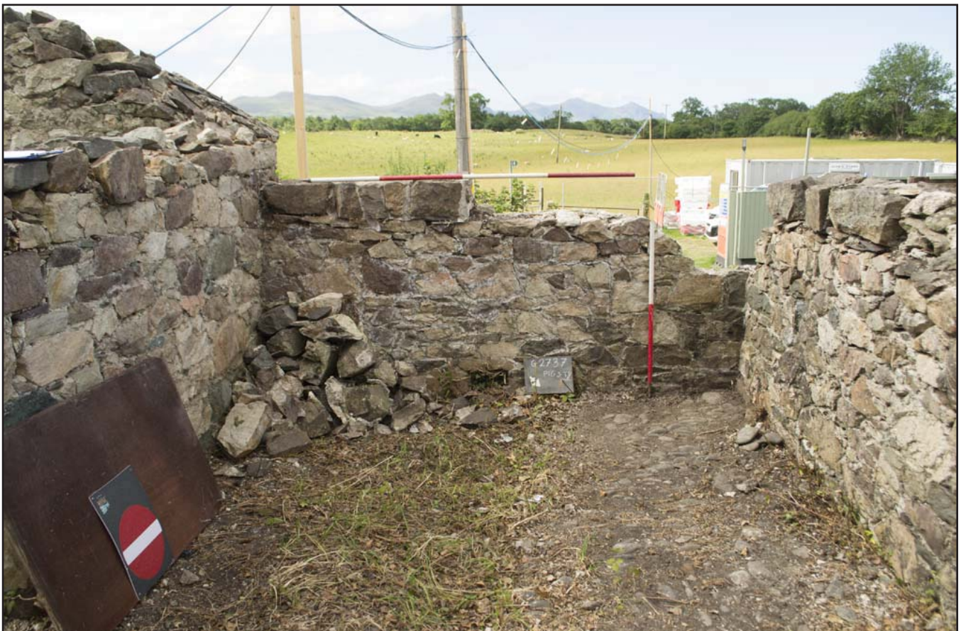
Plate 16: Interior view of pigsty (Room 4); scale 1x2m & 1x1m; view from NNE (archive reference: G2736_020).
