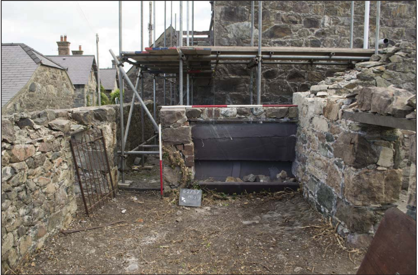
Plate 17: Interior view of pigsty showing slate pig trough (Room 4); scale 1x2m & 1x1m; view from SSW (archive reference: G2736_021).
