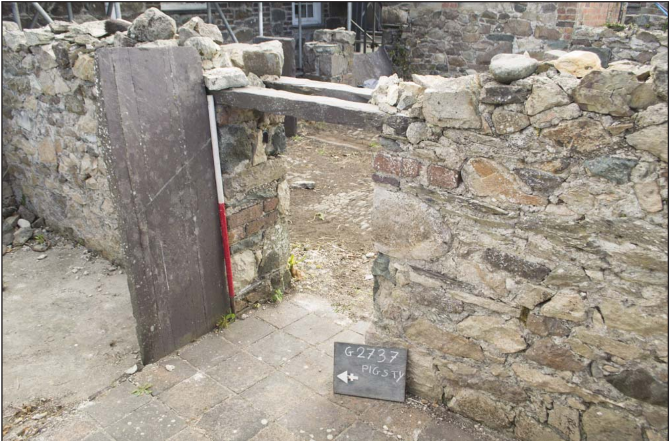
Plate 11: View of doorway between Rooms 2 and 3 showing slate lintel and slate slab orthostat; scale 1x1m; view from W (archive reference: G2736_017).
